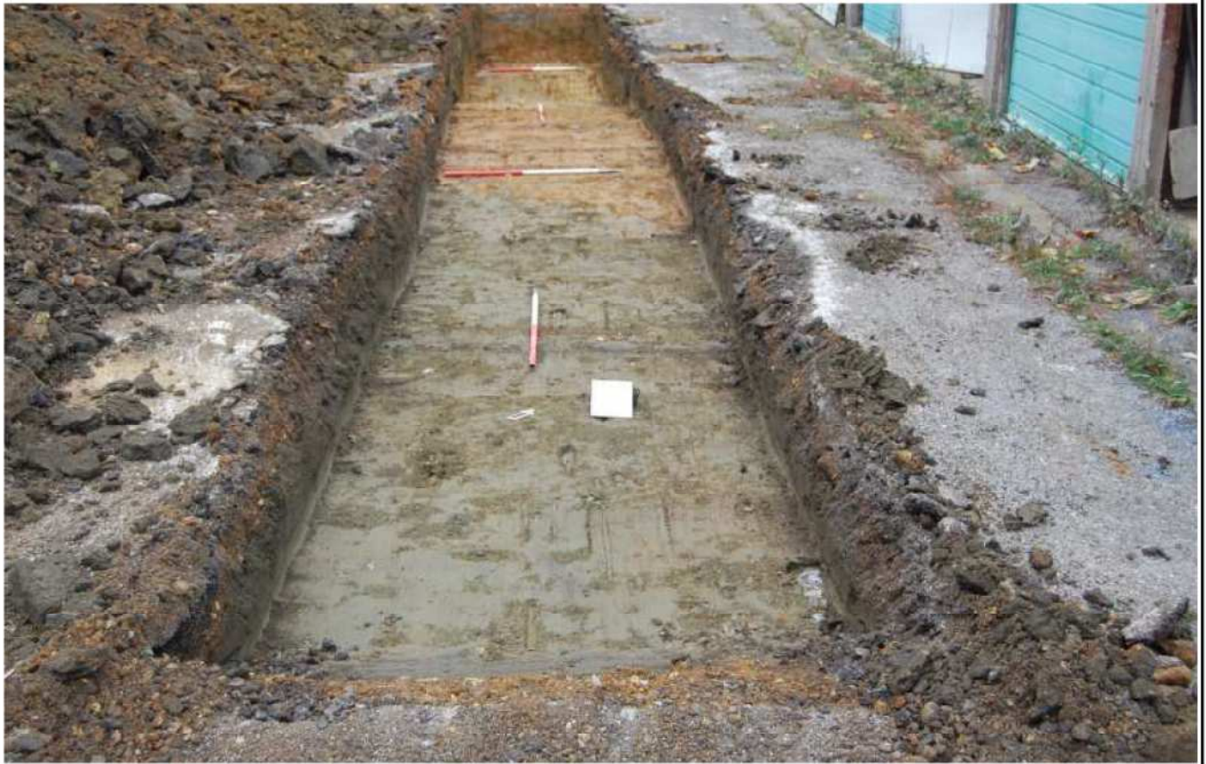
Plate 1: Trench 1, looking north-west
