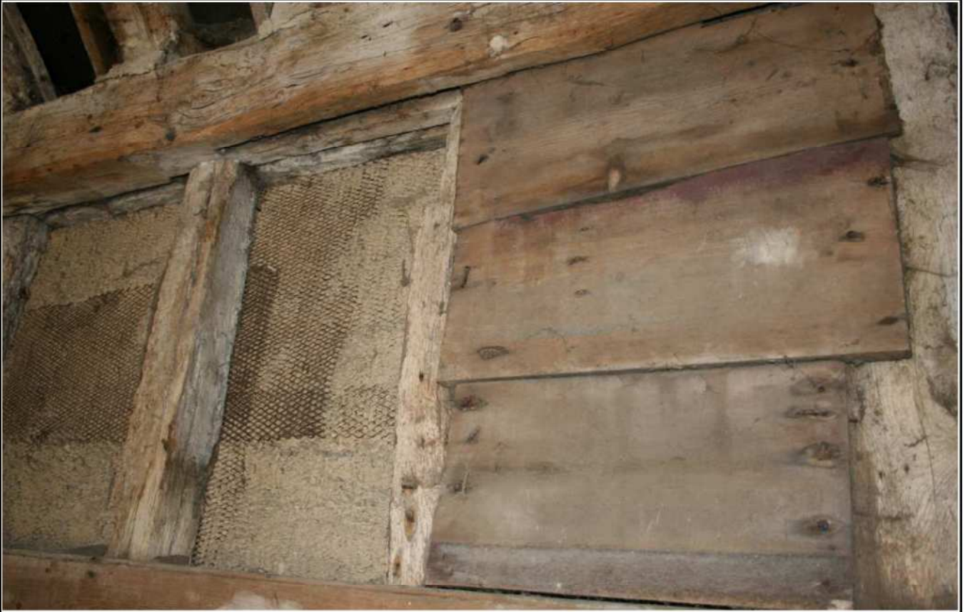
Plate 19: Upper floor, blocked window and groove for shutter, west elevation, Bay 2
