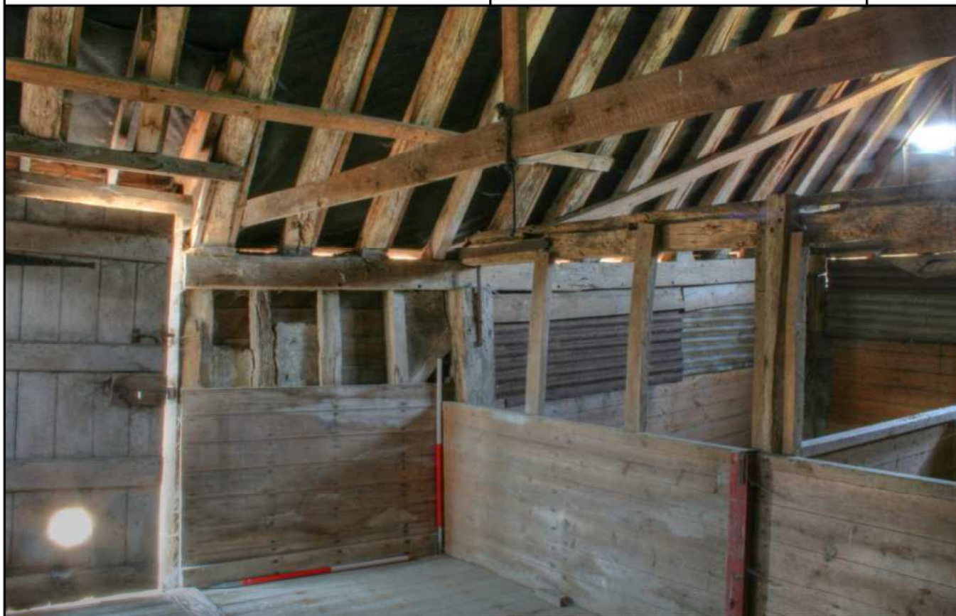
Plate 21: Upper floor, partition between Bays 1 & 2, looking NW
