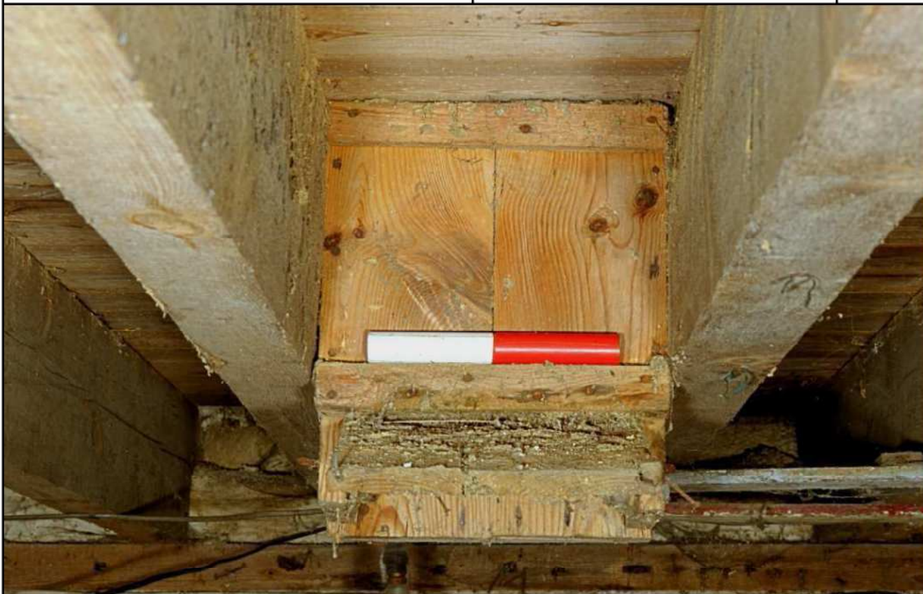
Plate 13: Ground floor, north grain chute
