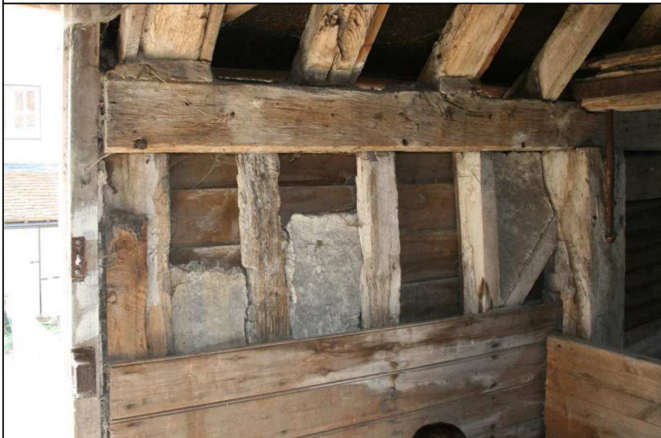
Plate 18: Upper floor, plaster panels in west elevation, Bay 2
