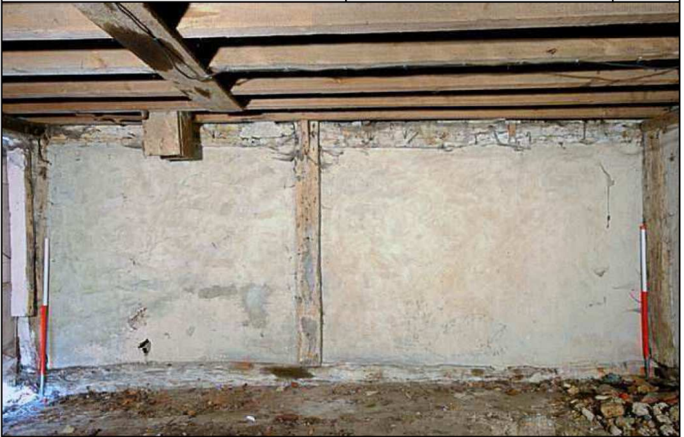
Plate 9: Ground floor, north interior elevation
