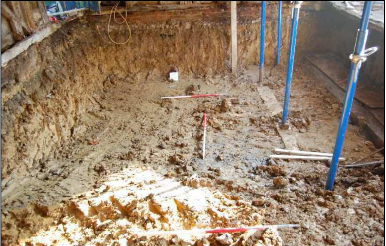
Plate 27: Granary after ground reduction, looking south
