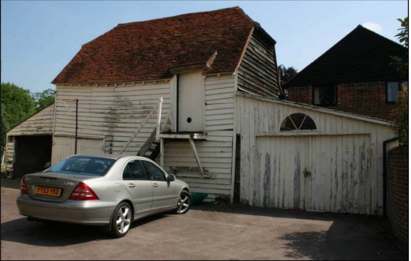
Plate 1: Granary, west exterior elevation, looking north-east
