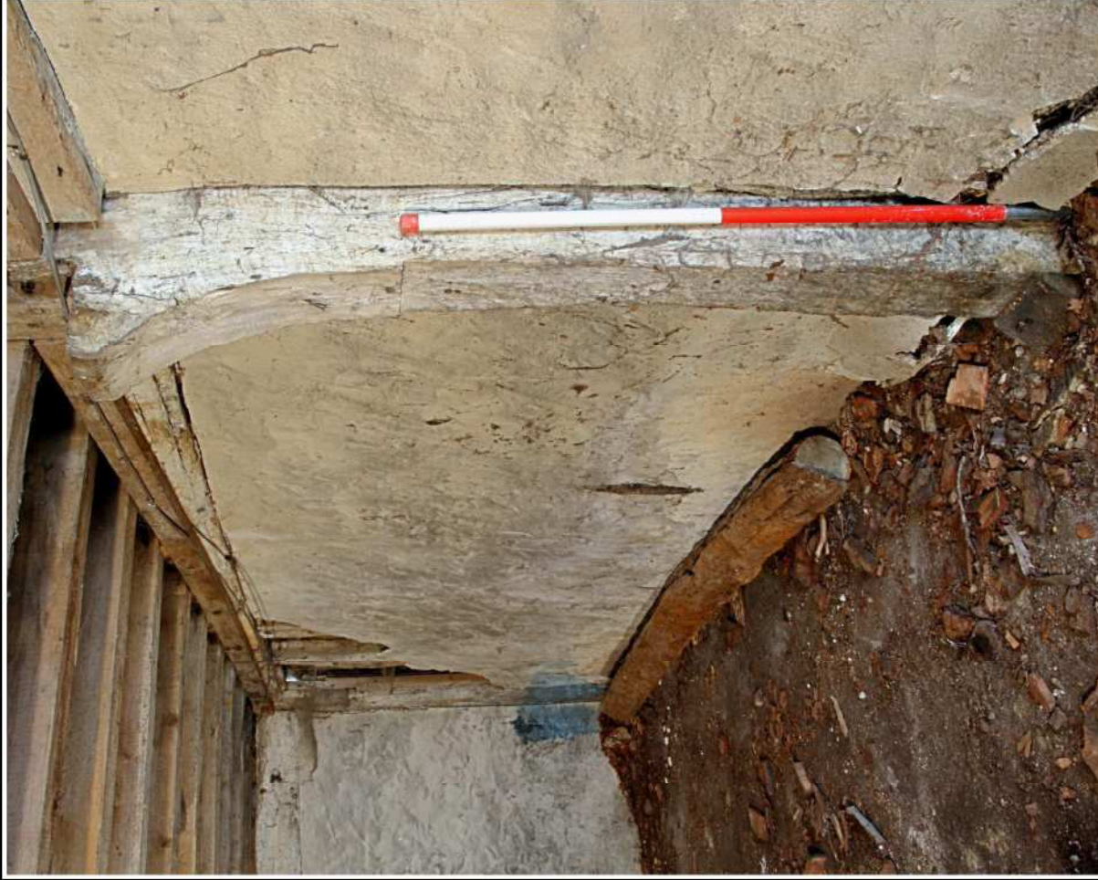
Plate 12: Detail of west middle post
