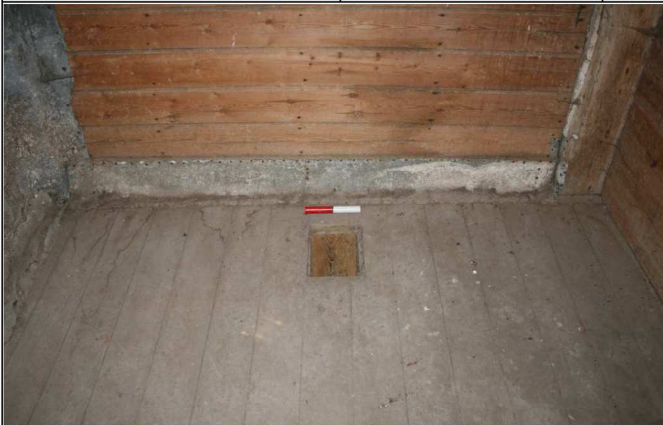
Plate 23: Upper floor, Bay 1, chute in western grain bin
