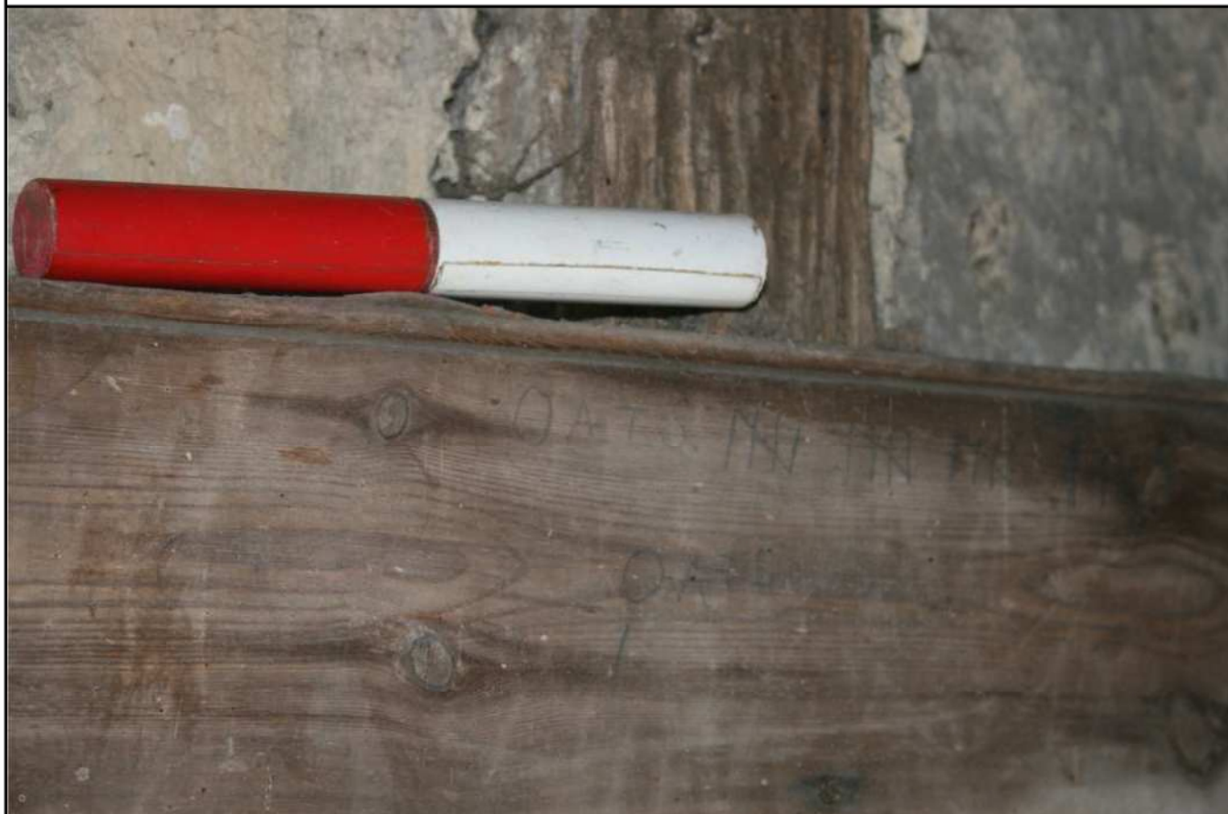
Plate 26: Upper floor, pencilled tally, W elevation, Bay 2
