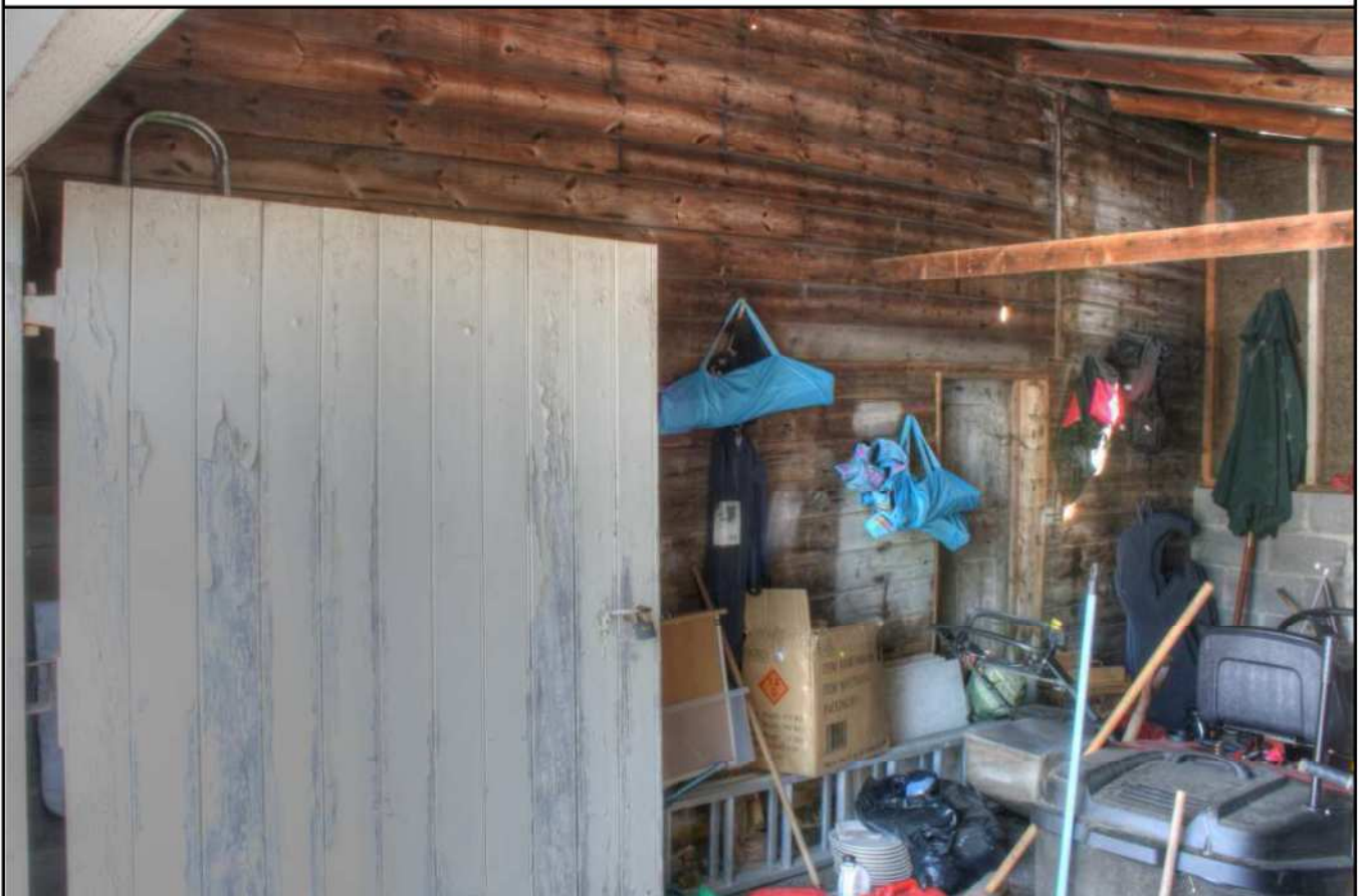
Plate 6: Southern lean-to, detail of granary south wall
