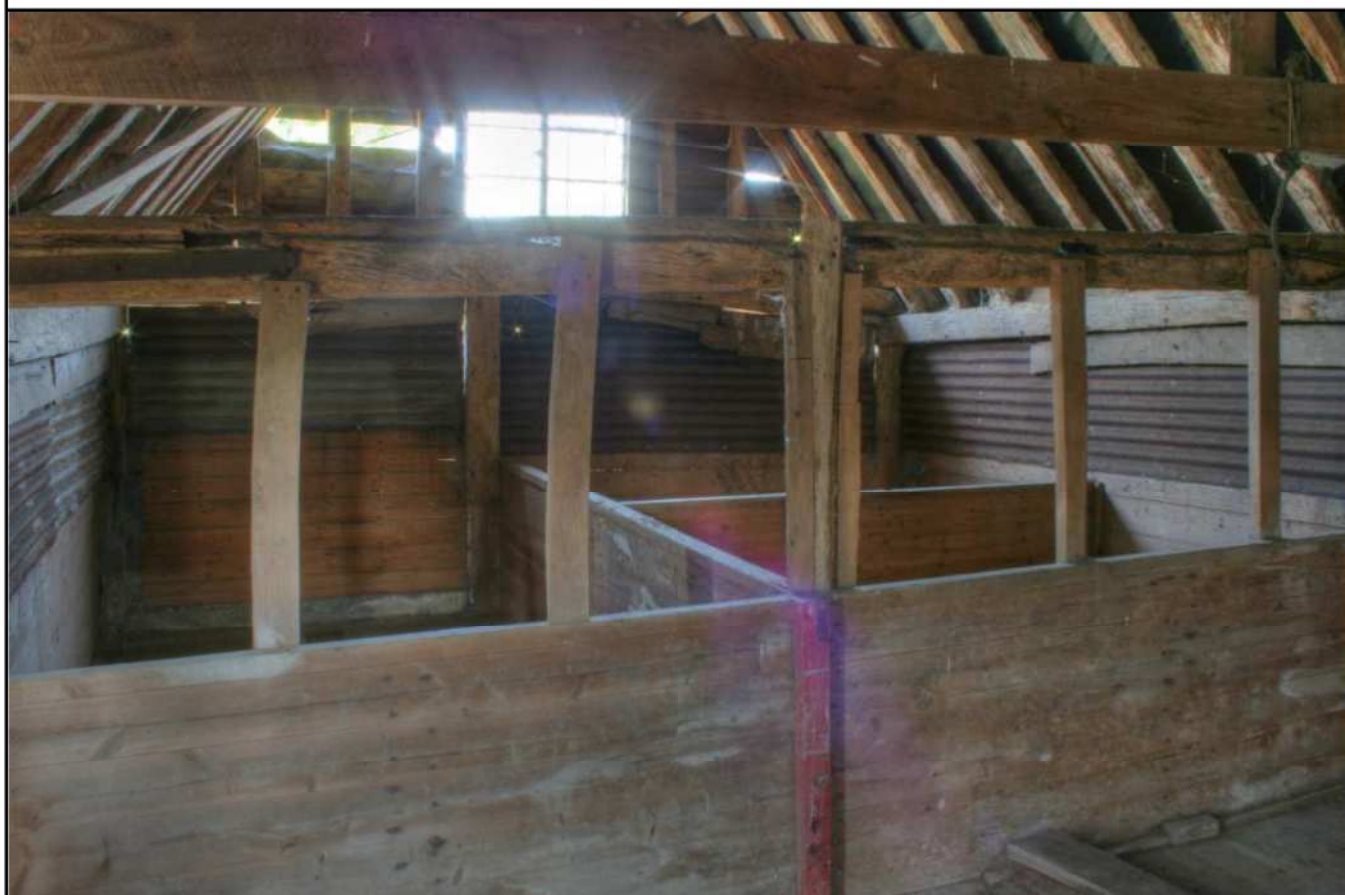
Plate 22: Upper floor, grain bins in Bay 1, looking NE
