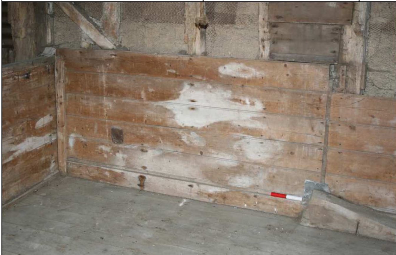
Plate 25: Upper floor, possible southern grain bin, E elevation Bay 2
