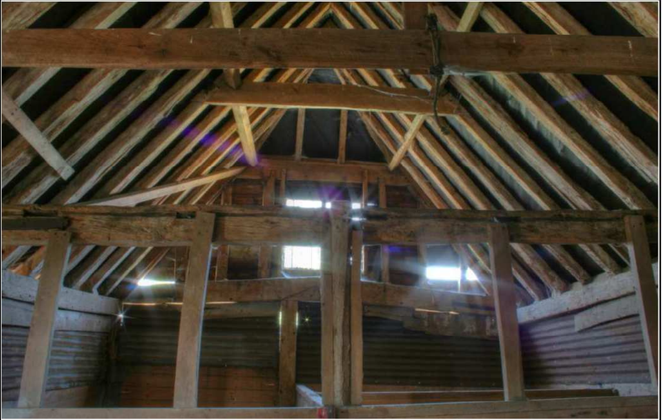
Plate 15: Upper floor, roof structure, looking north
