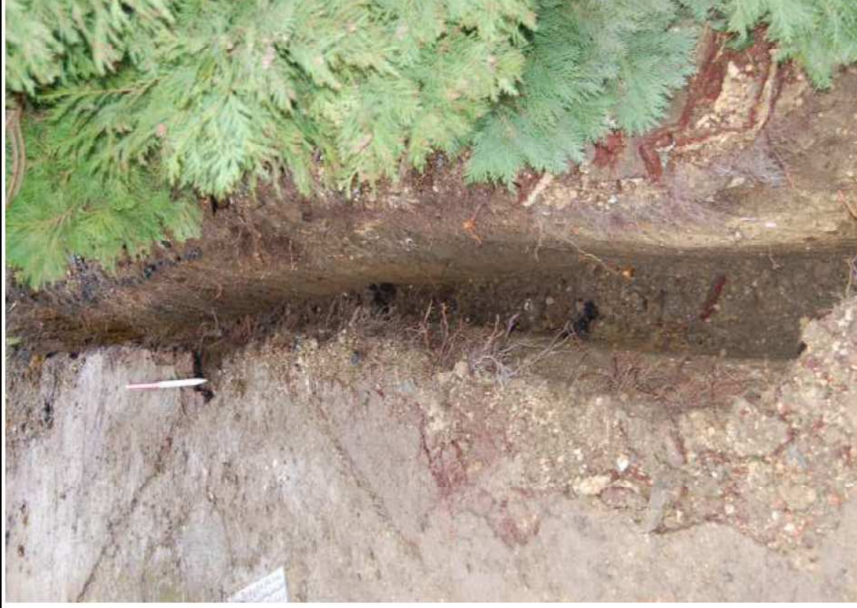
Plate 32: Drainage trench to N of Granary, looking N
