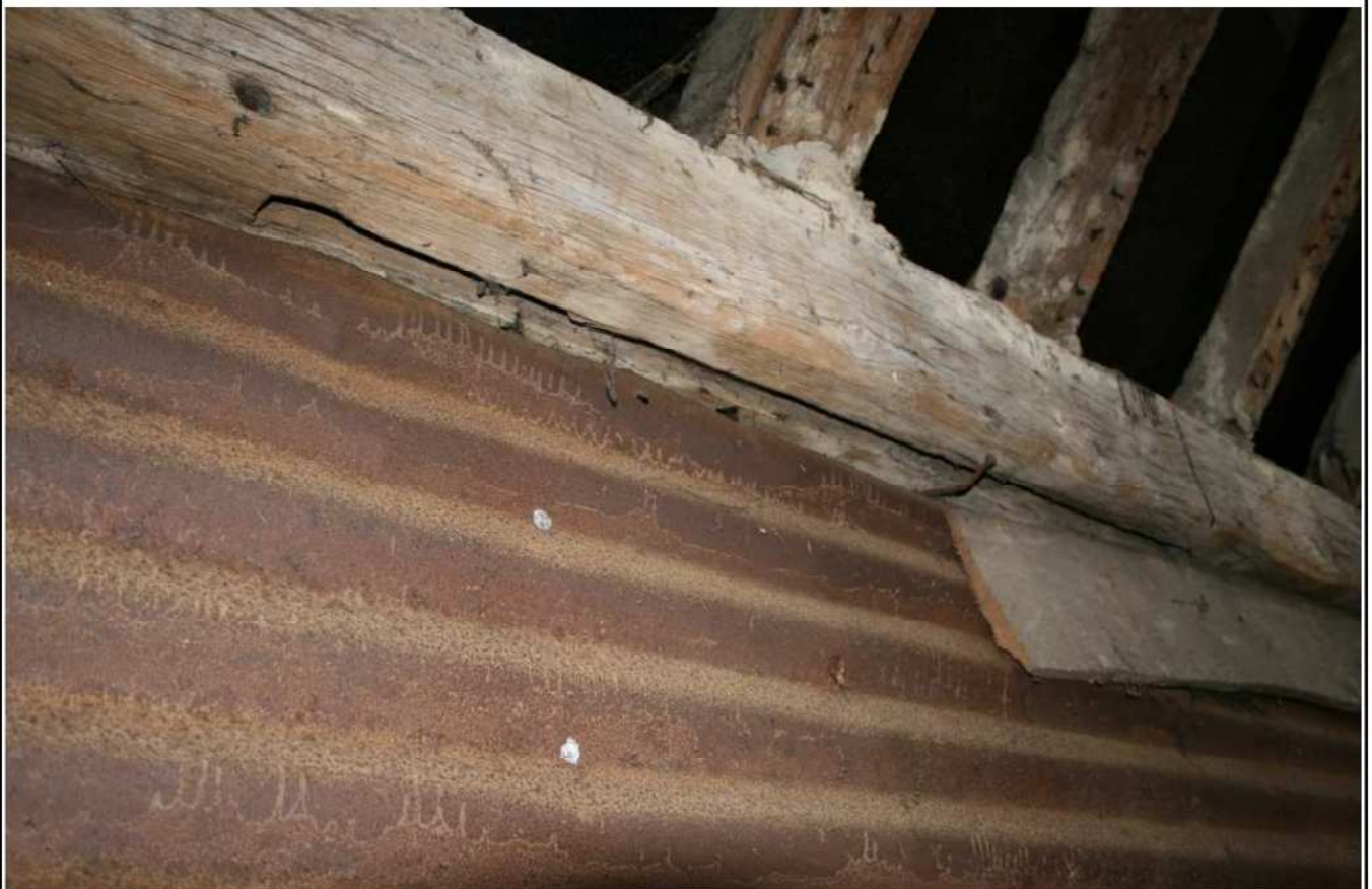
Plate 20: Upper floor, groove for shutter, east elevation, Bay 1
