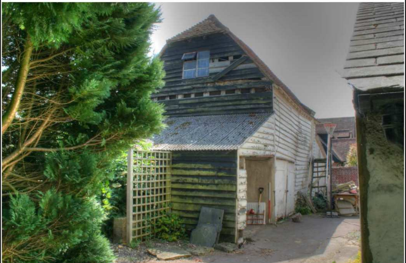
Plate 4: North exterior elevation, looking south
