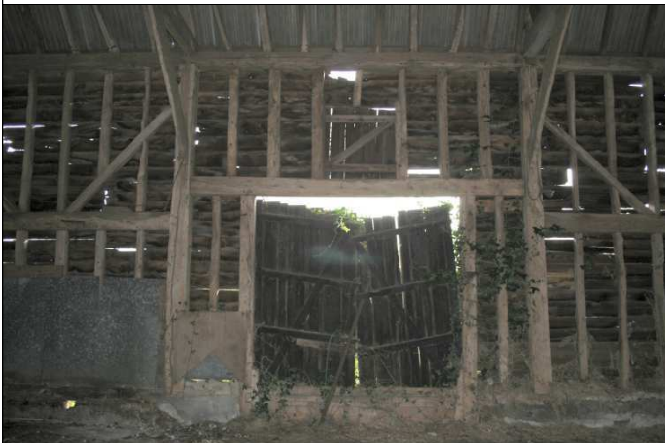
Plate 8: South interior elevation, doorway, looking south
