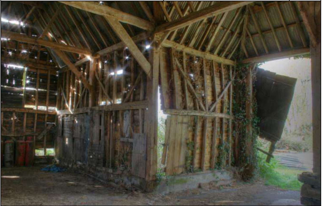
Plate 11: North interior elevation, and west elevation to porch, looking north-west
