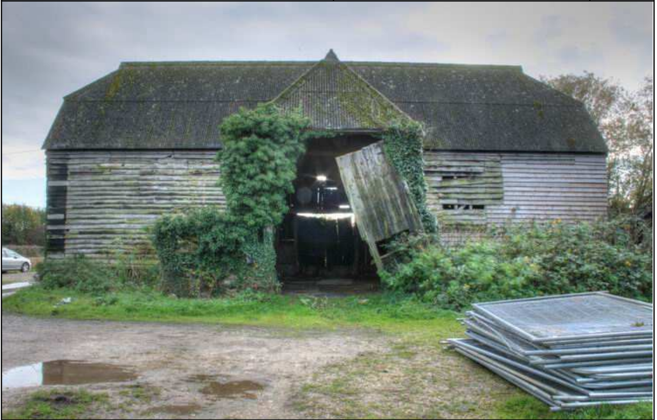
Plate 3: North exterior elevation, looking south
