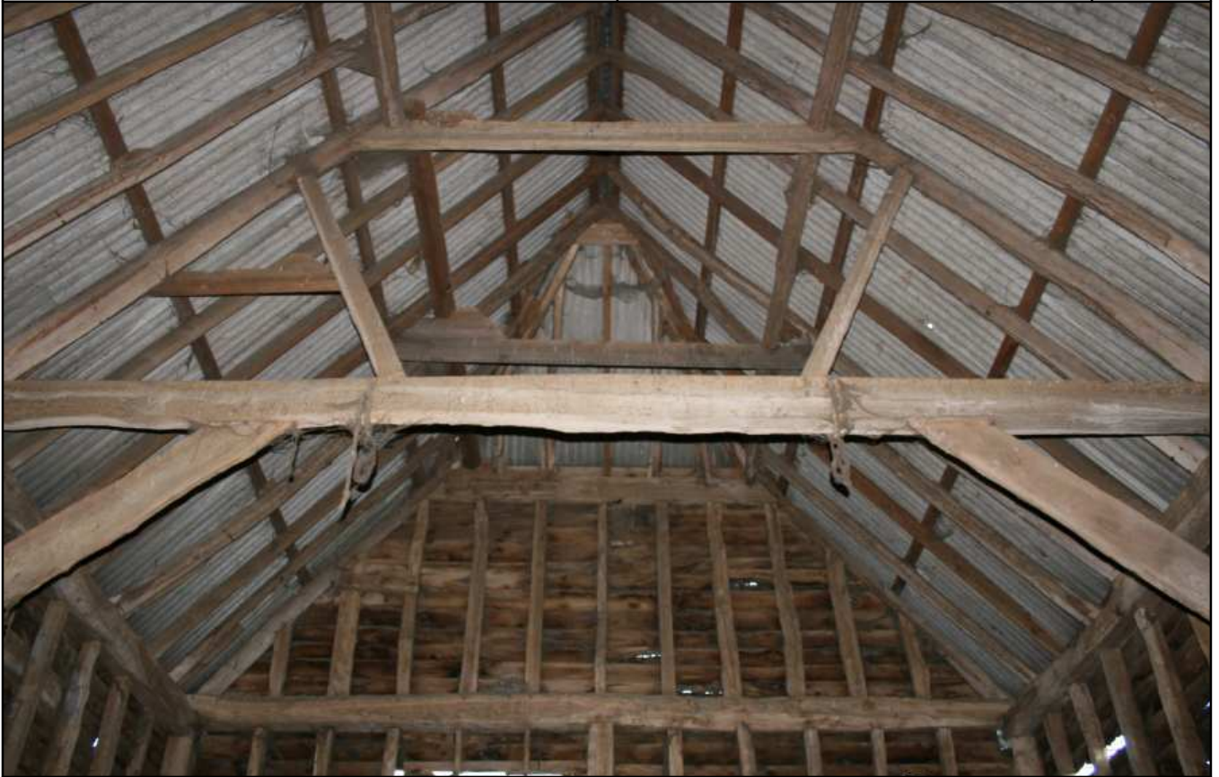
Plate 13: Roof structure, looking east
