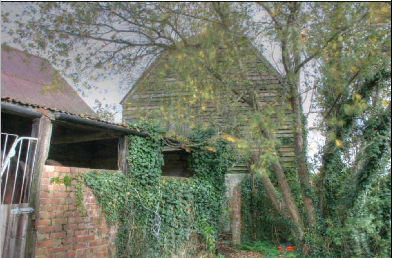
Plate 4: West exterior elevation, looking east
