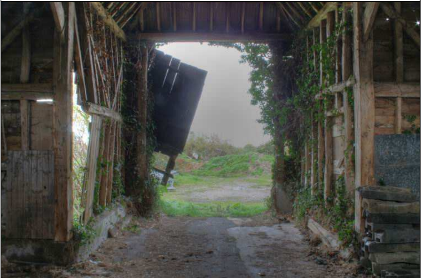
Plate 10: North interior elevation, looking north through porch
