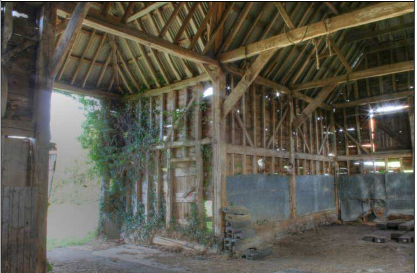
Plate 12: North interior elevation & east elevation to porch, looking north-east
