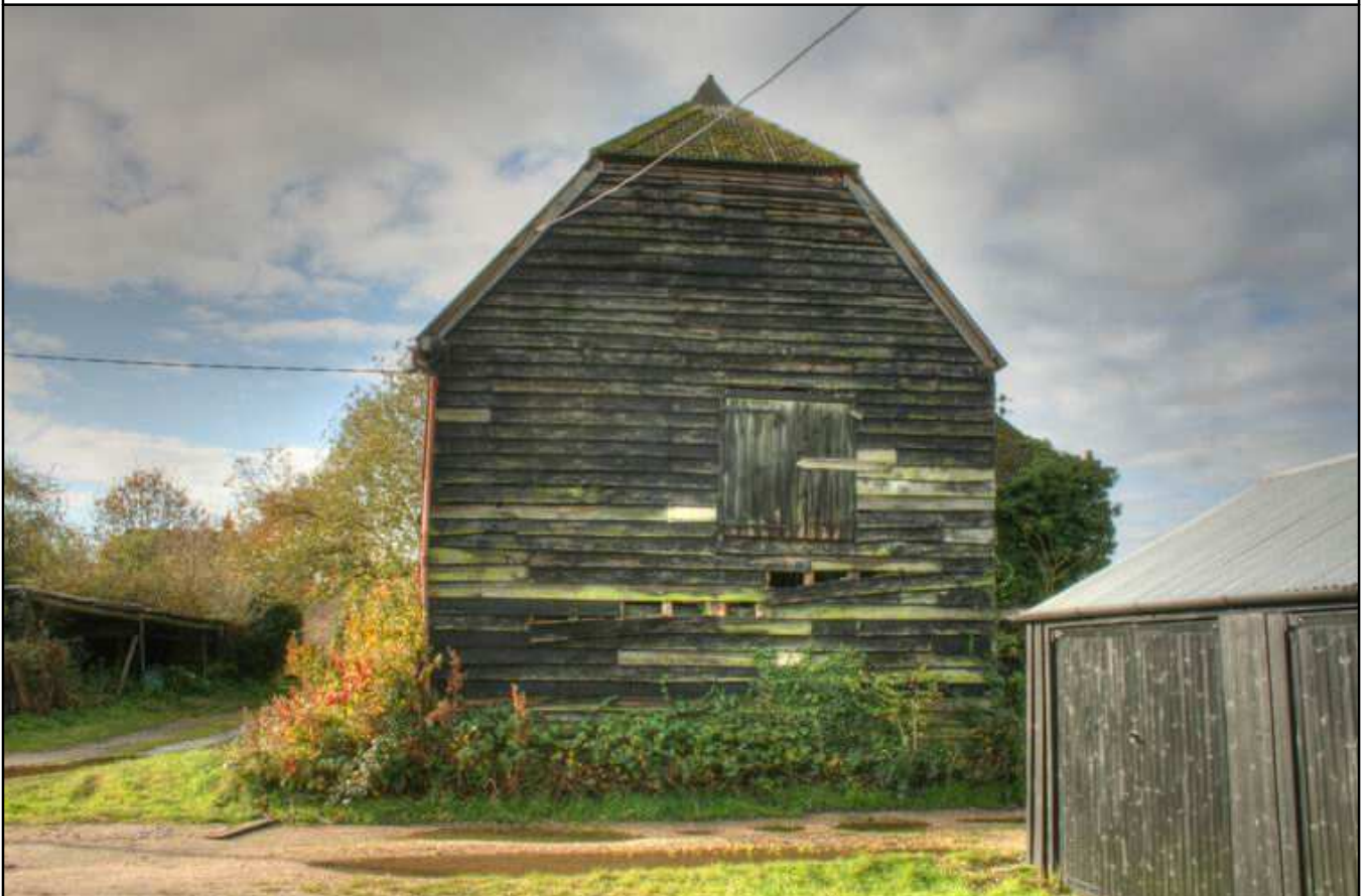
Plate 2: East exterior elevation, looking west
