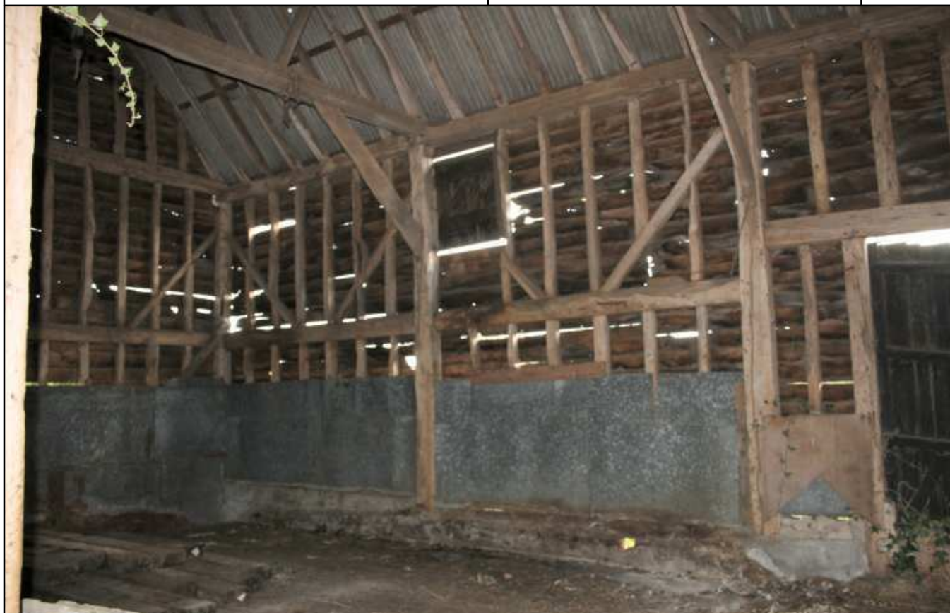
Plate 7: Southern and eastern interior elevations, looking south-east
