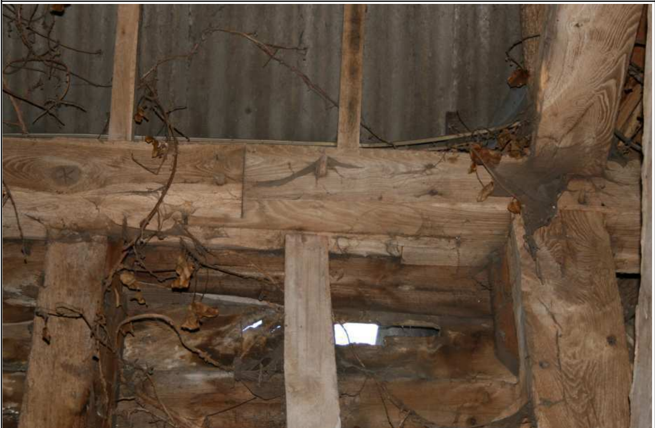
Plate 14: Sample scarf joint in wall plate
