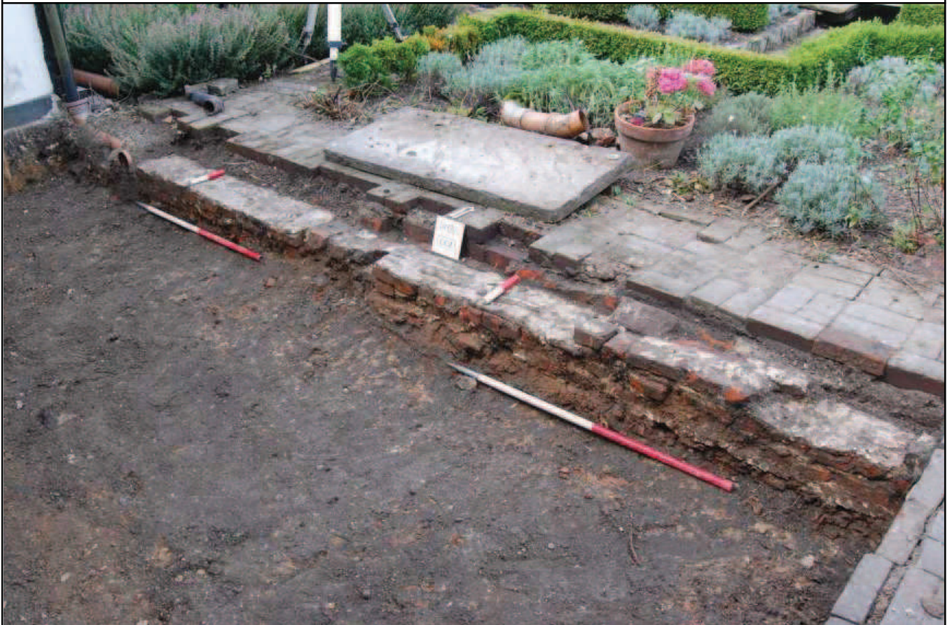
Plate 2: Wall [002], looking north-west
