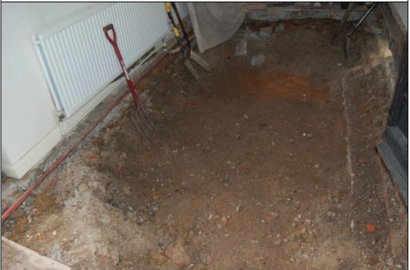
Plate 6: General shot of interior showing wall foundations and floor makeup
