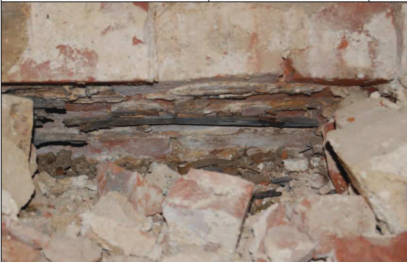
Plate 21: Vault [103], detail of wooden lining at the west end
