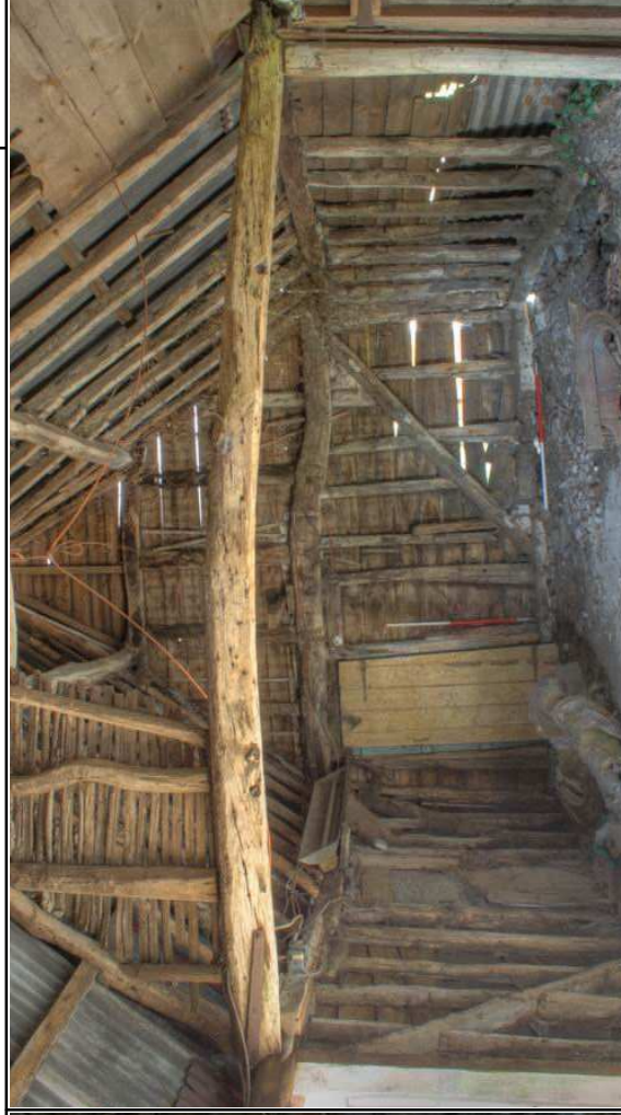
Plate 38: Block 4, detail of possible original middle truss
