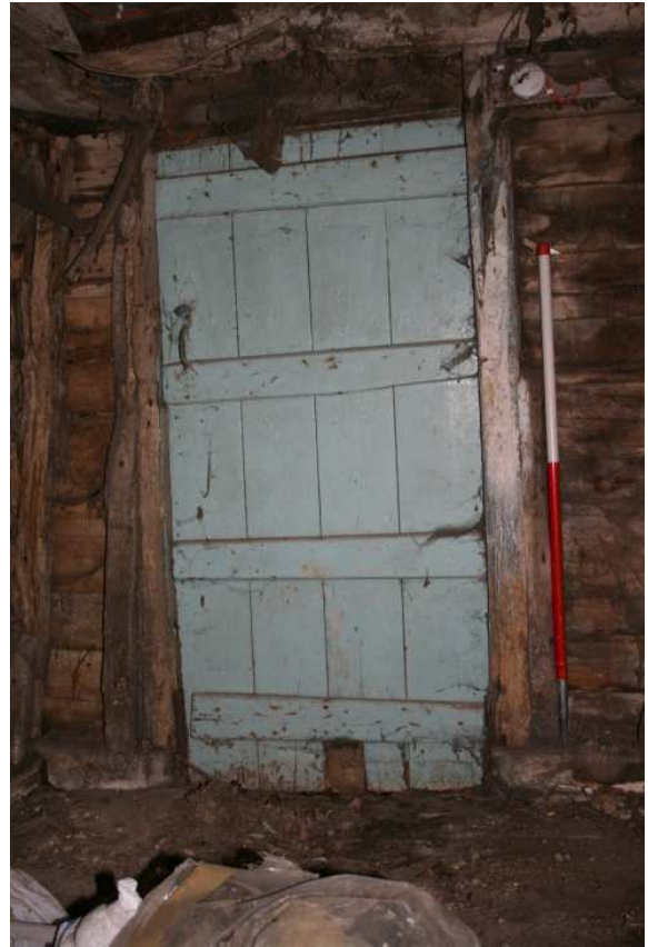
Plate 34: Block 4, S elevation, ledged & boarded door
