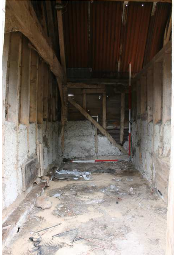
Plate 16: Block 3, looking west
