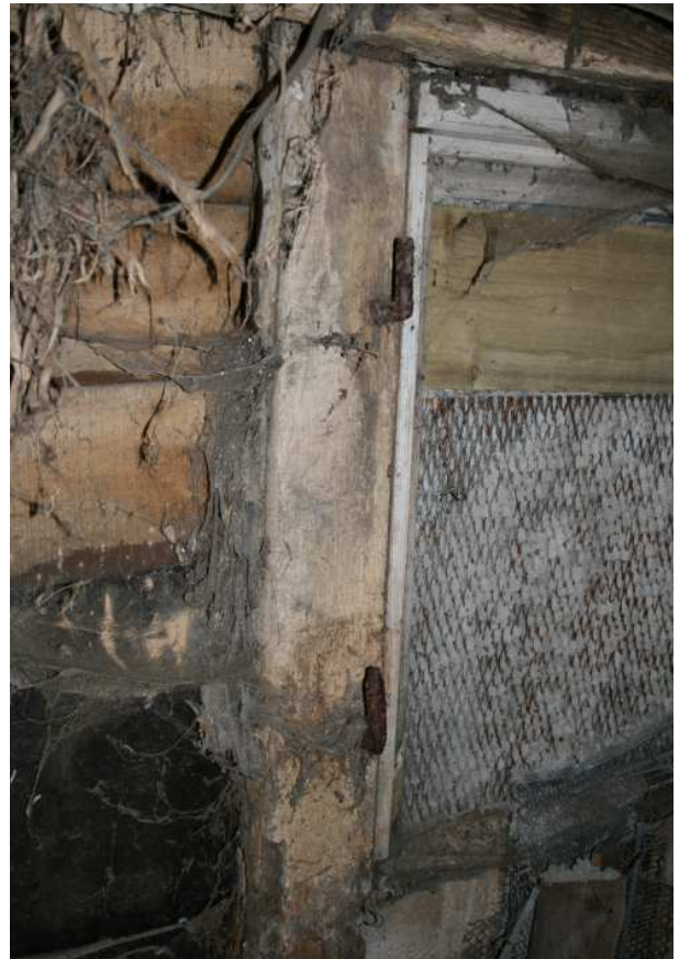
Plate 36: Block 4, hinge detail, blocked window, Bay 2 E elevation
