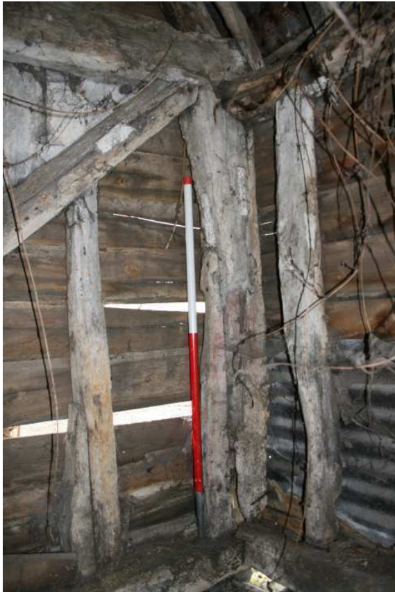
Plate 33: Block 4, SE corner post, Bay 2
