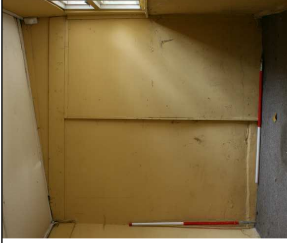
Plate 44: Block 5, N interior elevation, looking N
