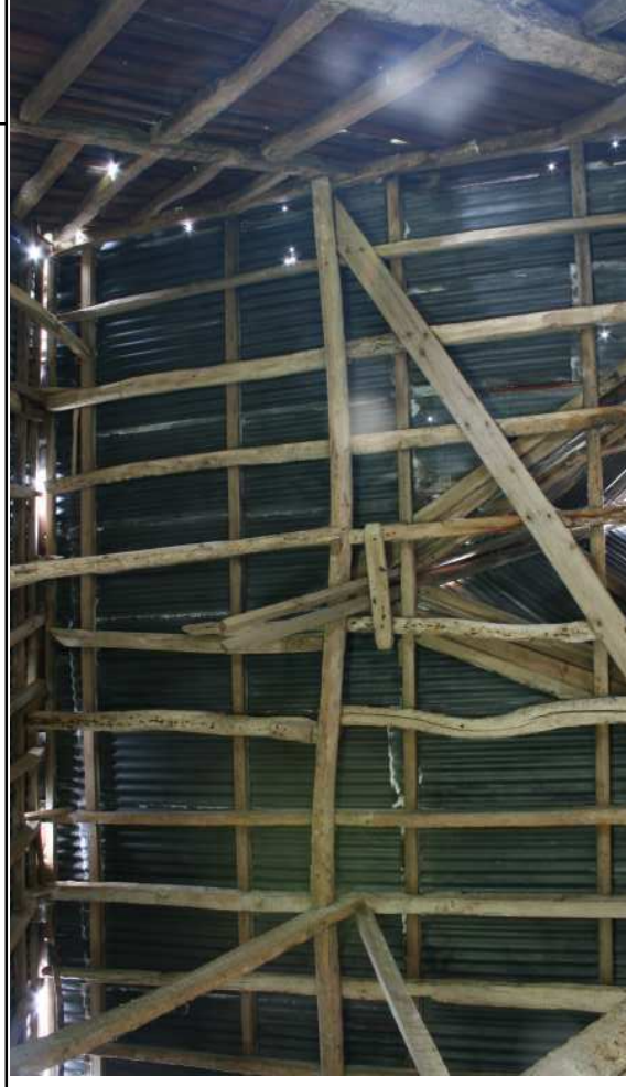
Plate 18: North Barn, roof structure S elevation, Bay 1
