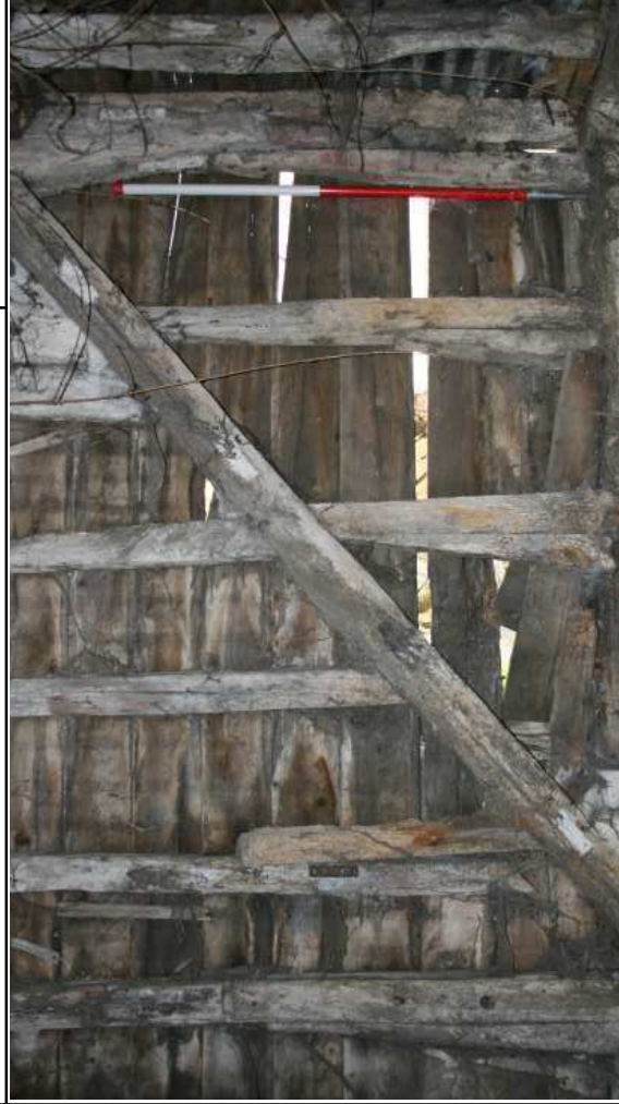
Plate 37: Block 4, Bay 2, detail of re-used brace in S elevation
