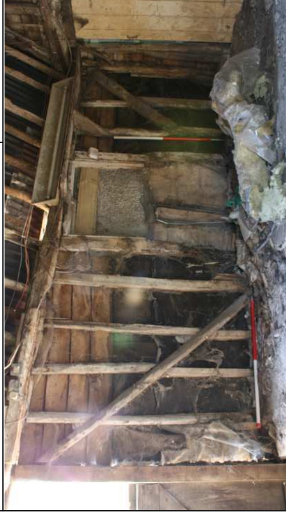
Plate 41: Block 4, Bay 2 W interior elevation, looking SW
