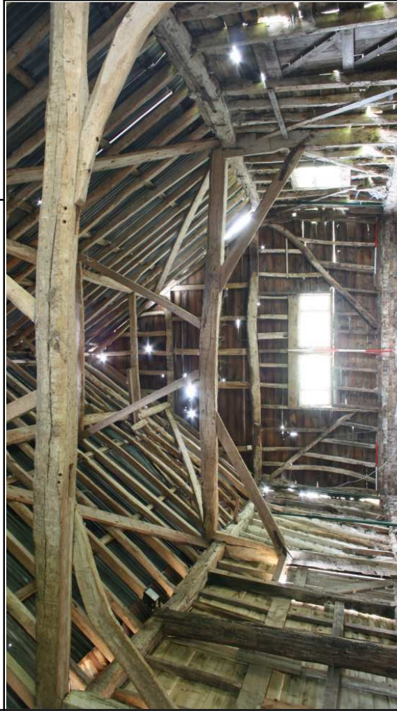
Plate 5: North Barn, W interior elevation, looking W
