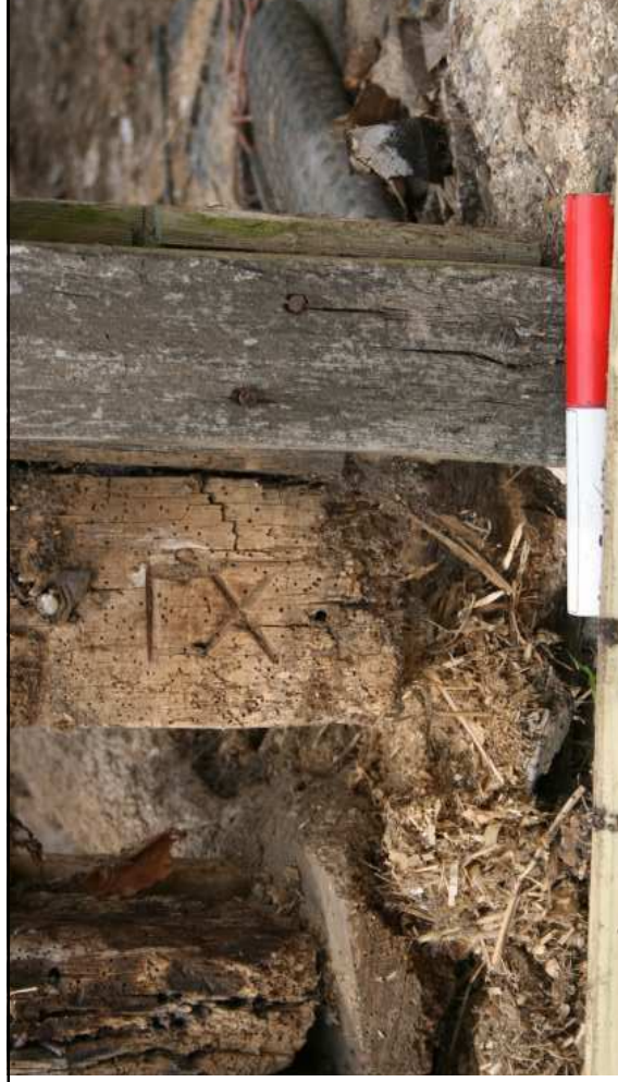
Plate 47: Block 4, detail of carpenter's mark, base of SE corner post
