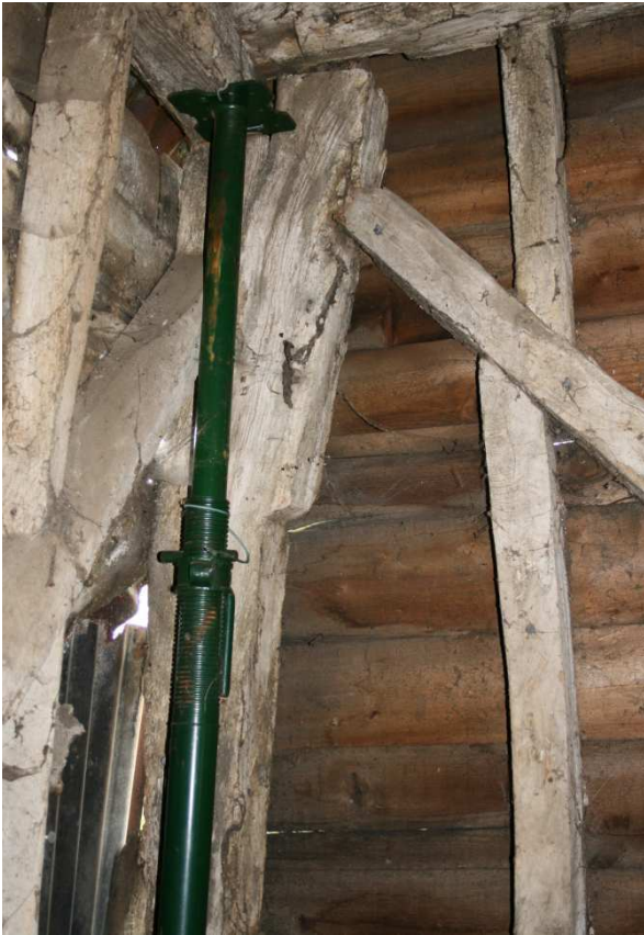
Plate 13: North Barn, detail of SW corner post
