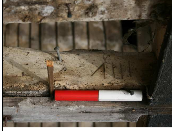
Plate 48: Block 1, detail of carpenter's mark on N door jamb
