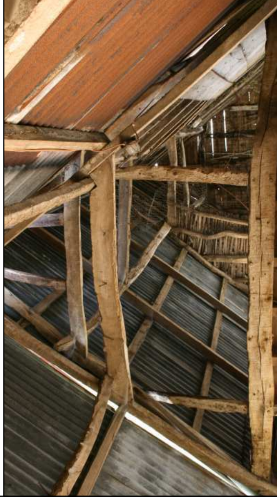
Plate 31: Block 3, detail of roof structure at junction of Blocks 3 & 4
