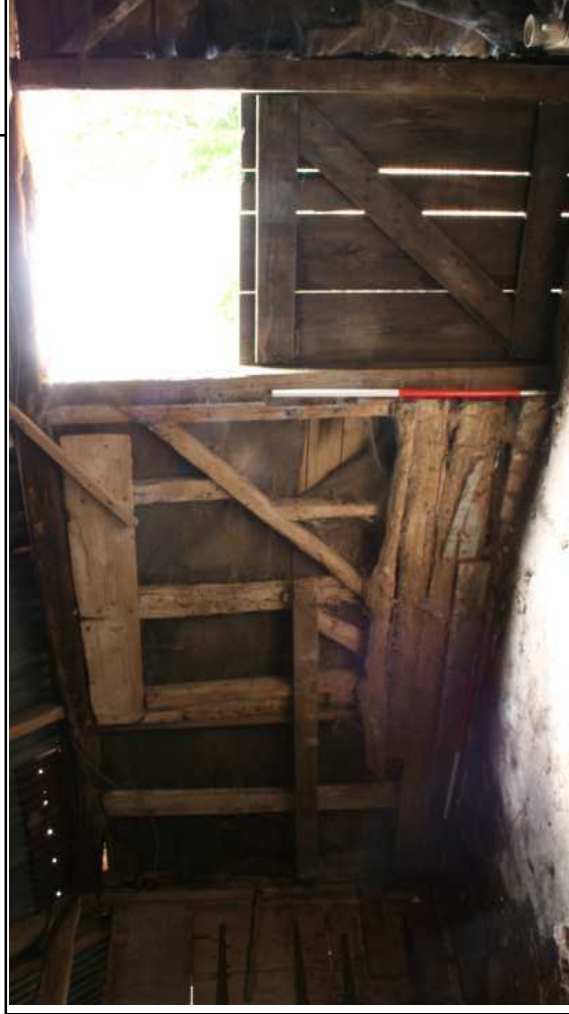
Plate 42: Block 4, Bay 1, E interior elevation, looking NE
