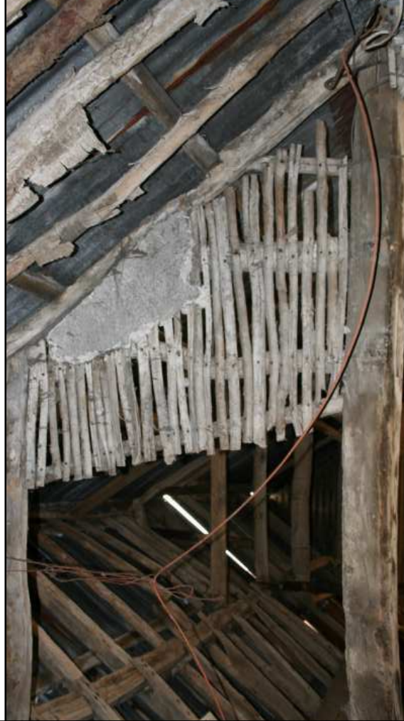
Plate 39: Block 4, lath & plaster partition between Bays 1 & 2, looking N
