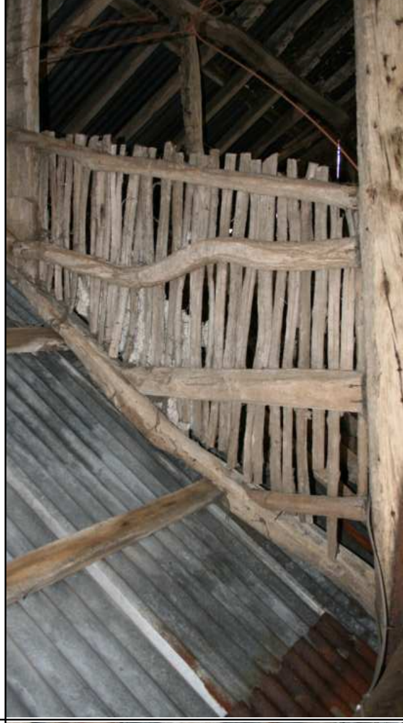
Plate 40: Block 4, lath & plaster partition, looking S
