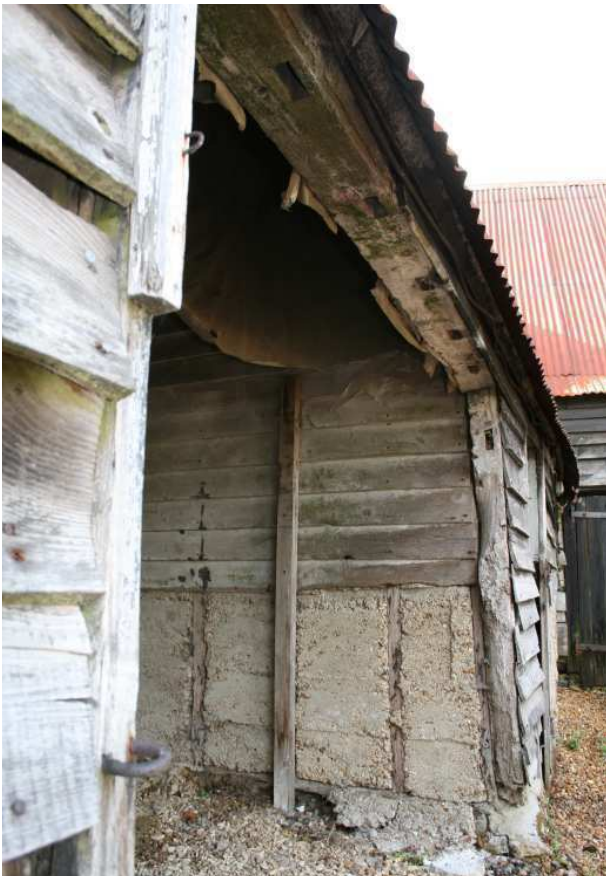
Plate 15: Block 2, detail of mortice holes in underside of E wall plate
