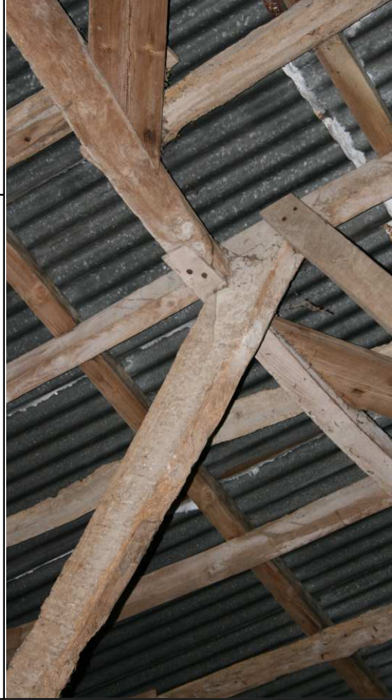
Plate 17: North Barn, S elevation roof structure, detail of junction between purlin & collar
