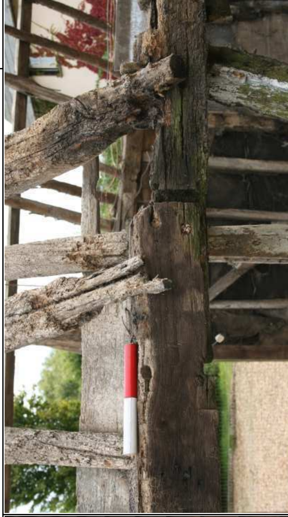
Plate 46: Block 4, detail of W wall plate, visible after removal of cladding
