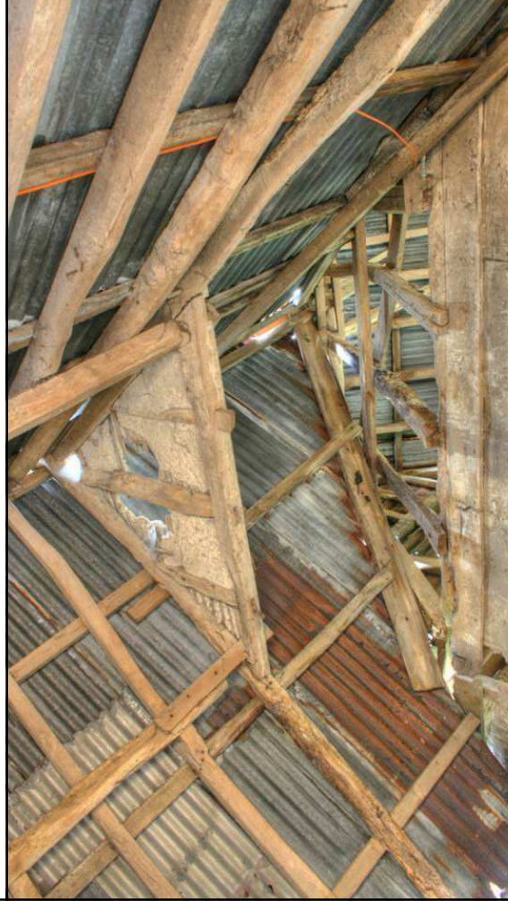
Plate 27: Block 1, floating panel above collar
