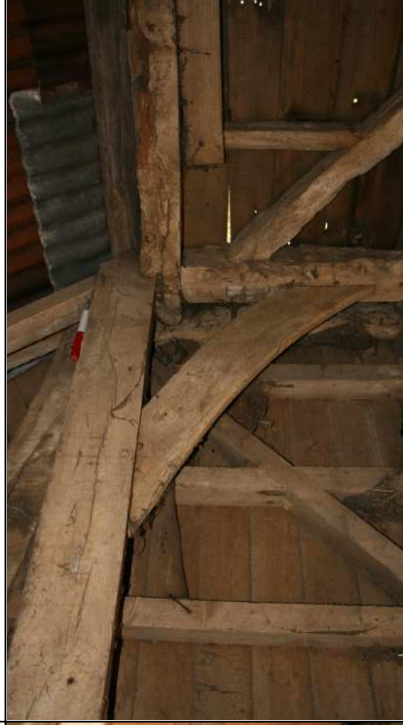
Plate 32: Block 3, detail of the truss between Blocks 3 & 4
