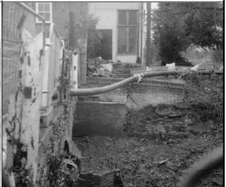
Frame 6: Retaining wall, island side, S of bridge
