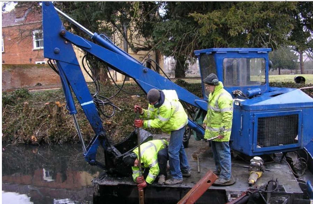
Plate 3: Setting the core sampler in the SW arm of the moat
