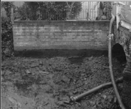
Frame 7: Retaining wall, land side, S of bridge
