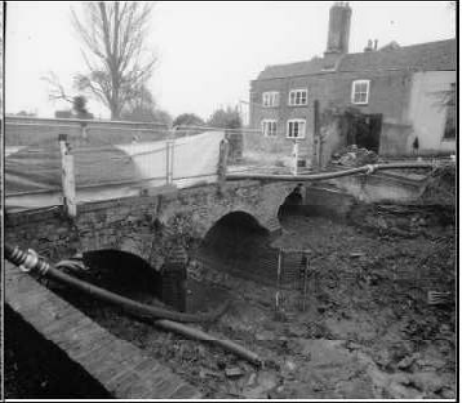
Frame 3: Bridge S elevation, looking NE
