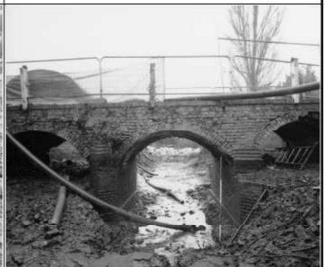
Frame 12: Bridge, S elevation, looking NW
