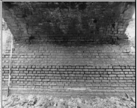
Frame 9: E pier, W elevation, detail of brickwork
