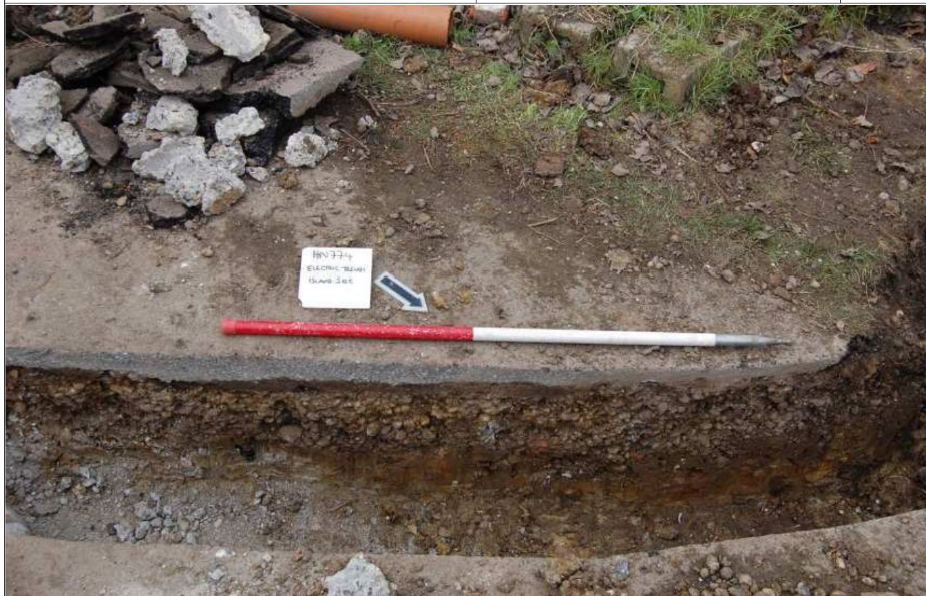
Plate 17: Island side service trench, looking SW
