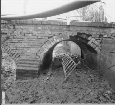
Frame 1: E arch of bridge, S elevation
