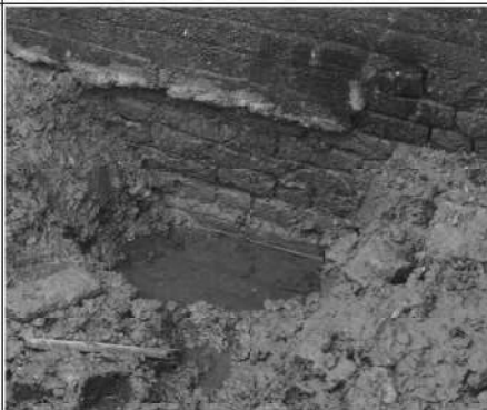
Frame 8: Earlier bricks, retaining wall, land side, S of bridge
