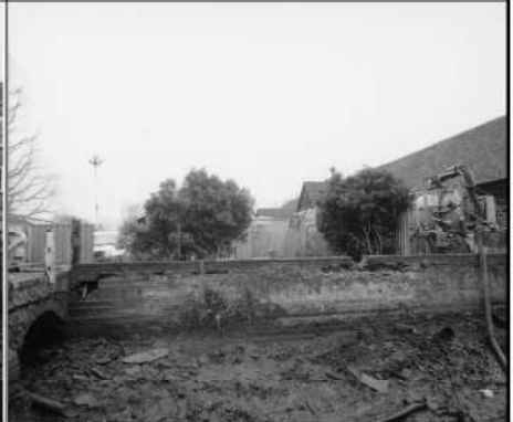
Frame 6: Retaining wall, land side, N of bridge
