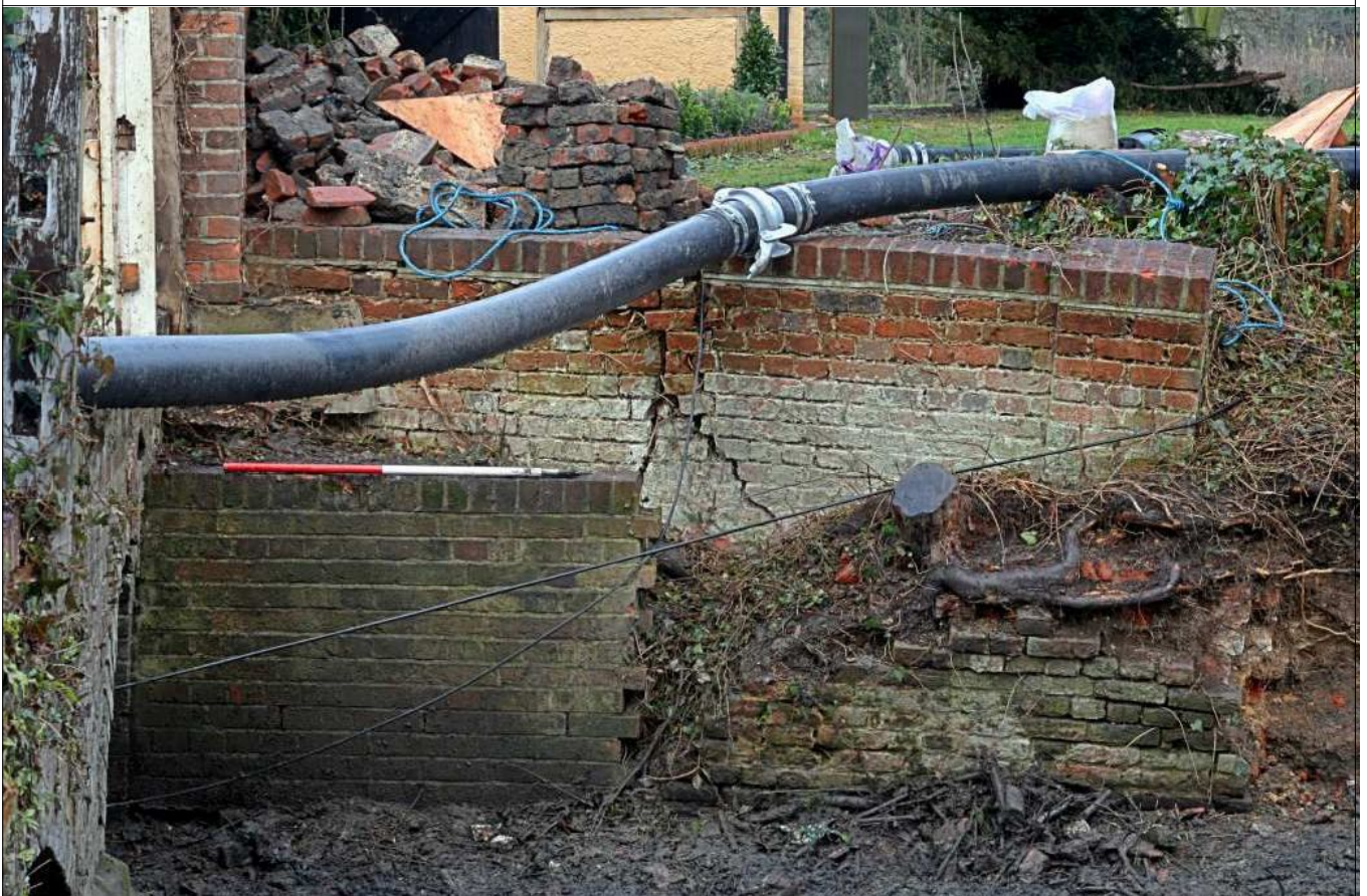
Plate 14: Retaining wall to N of bridge on island side
