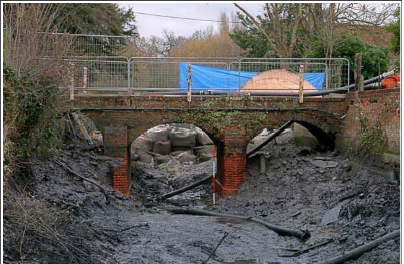
Plate 8: North-west elevation of the bridge, looking SE
