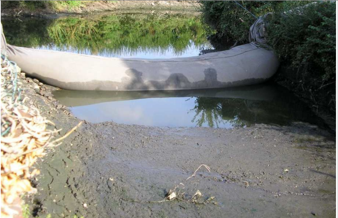
Plate 5: Water-filled barrage at NW end of SW arm of the moat
