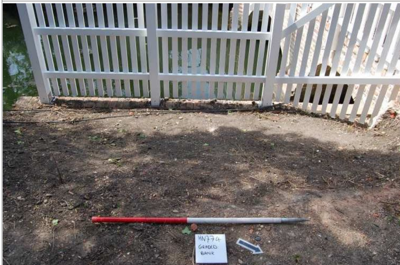
Plate 18: Graded bank to S of bridge on the island side, looking SW
