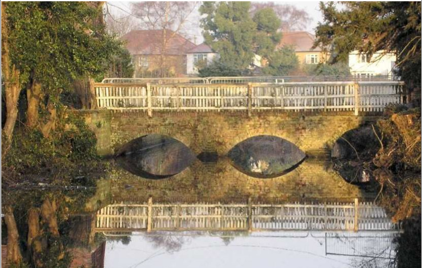
Plate 7: South-east elevation of the bridge before restoration, looking NW
