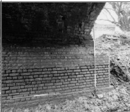
Frame 11: E pier, W elevation, detail of brickwork, view SE
