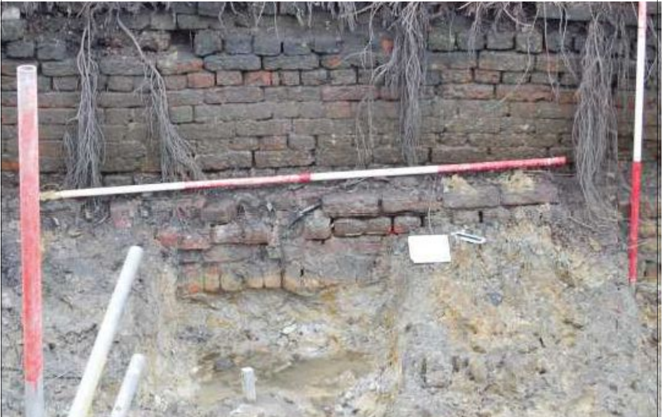
Plate 13: Earlier wall footings below late 19th century retaining wall to island side
