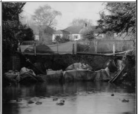
Frame 12: Bridge, S elevation, looking NW
