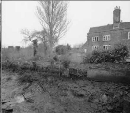
Frame 5: Moat bank, island side, N of bridge
