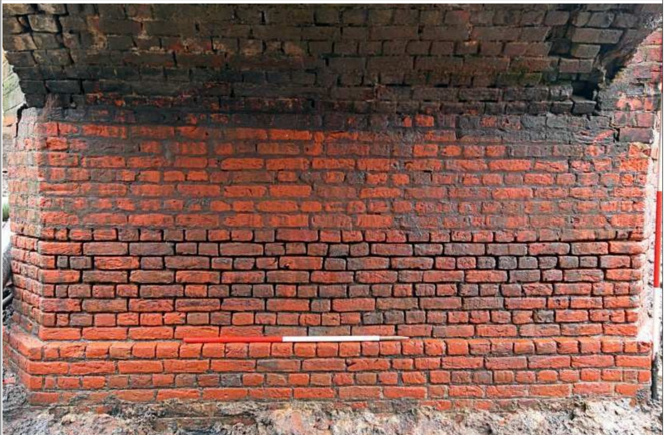
Plate 10: Western pier, E elevation, detail of brickwork
