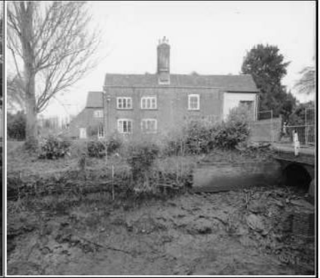
Frame 3: View of manor & retaining wall, island side, N of bridge
