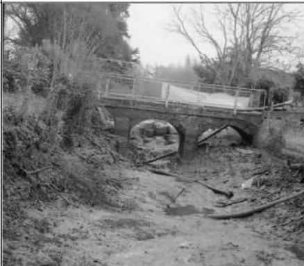
Frame 5: Bridge, N elevation, looking SE
