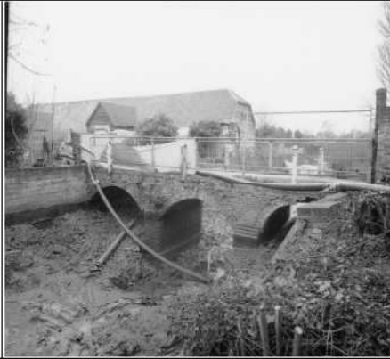
Frame 2: Bridge S elevation, looking SW
