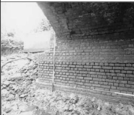
Frame 10: E pier, W elevation, detail of brickwork, view NW
