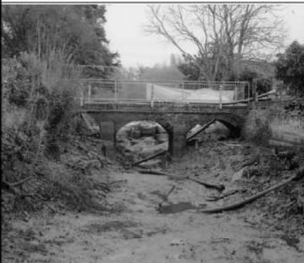
Frame 4: Bridge, N elevation, looking SE
