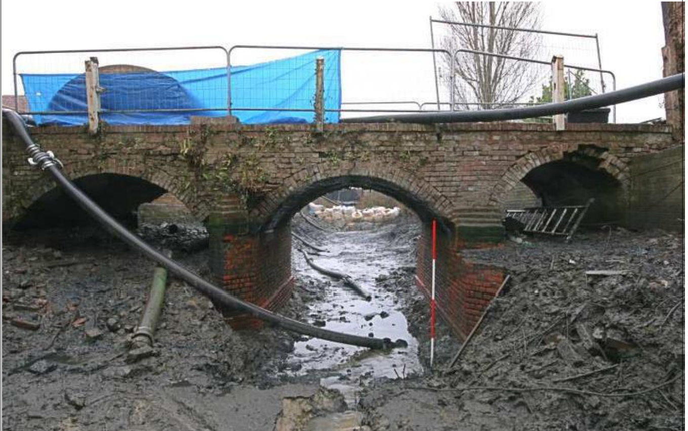
Plate 9: South-west elevation of the bridge, looking NE
