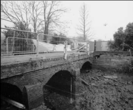
Frame 7: Bridge, N elevation, looking SW
