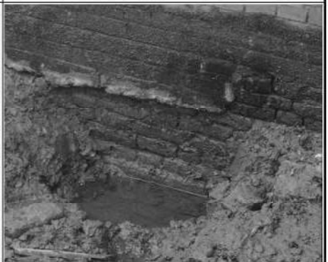
Frame 9: Earlier bricks, retaining wall, land side, S of bridge
