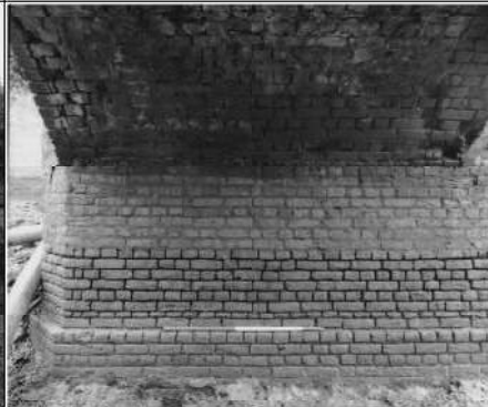
Frame 8: West pier, E elevation, detail of brickwork
