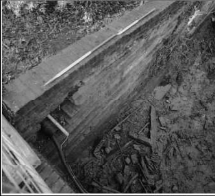
Frame 1: Retaining wall, land side, N of bridge
