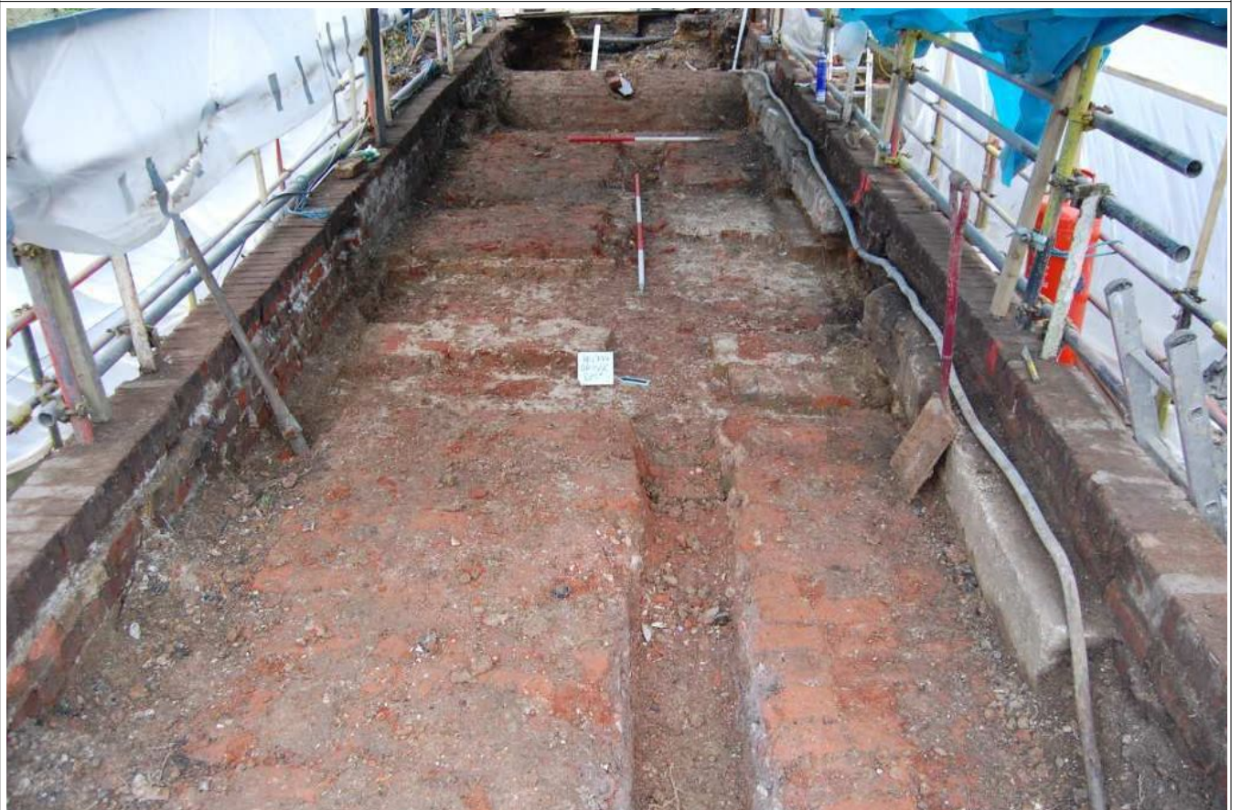
Plate 12: bridge deck following the removal of the surfacing materials, looking NE
