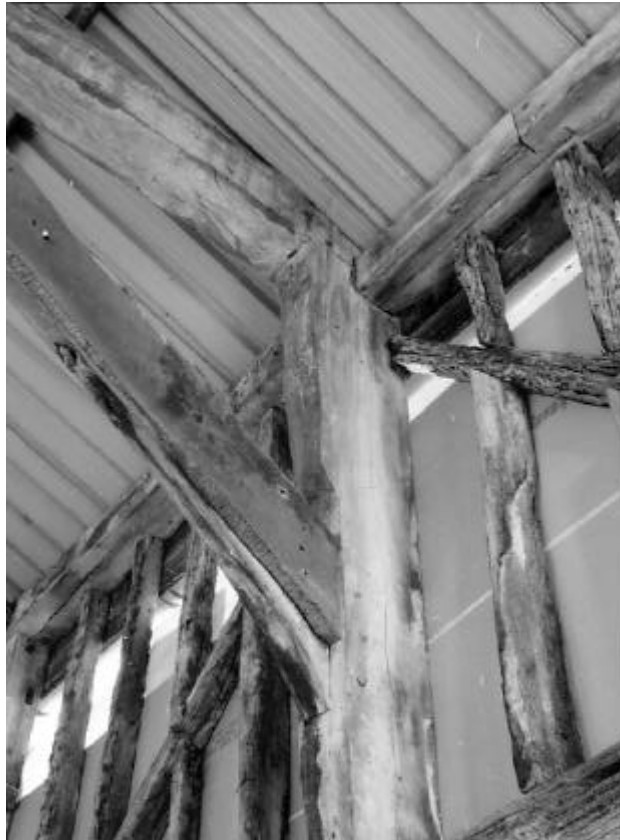
Bay 3, south elevation: edge-halved & bridle-butted scarf joint
