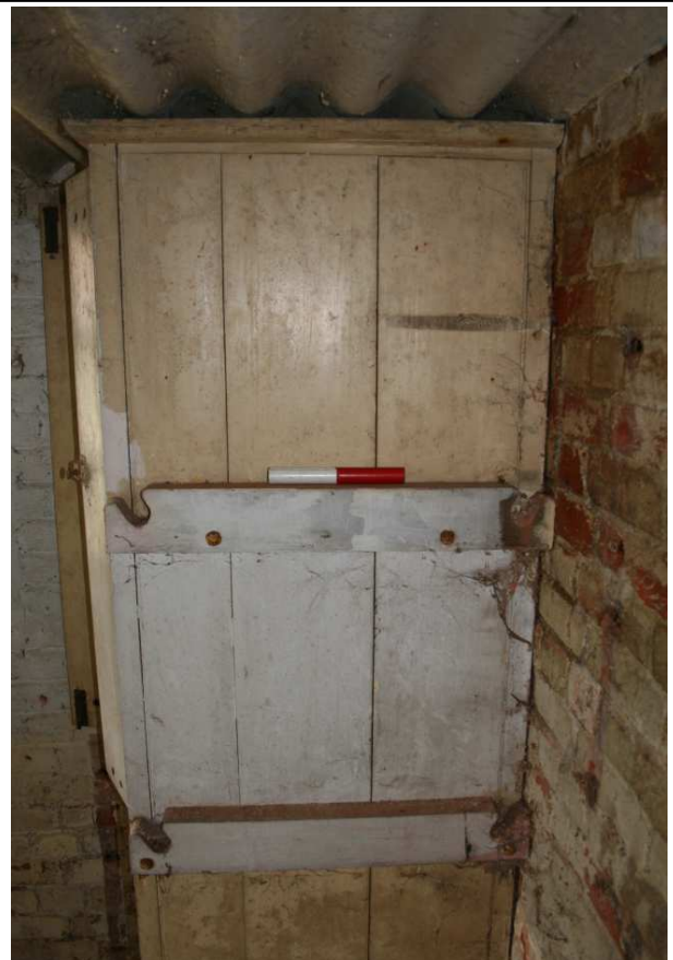
Plate 32: Air-raid shelter: detail of wooden slats, W side of built-in cupboard
