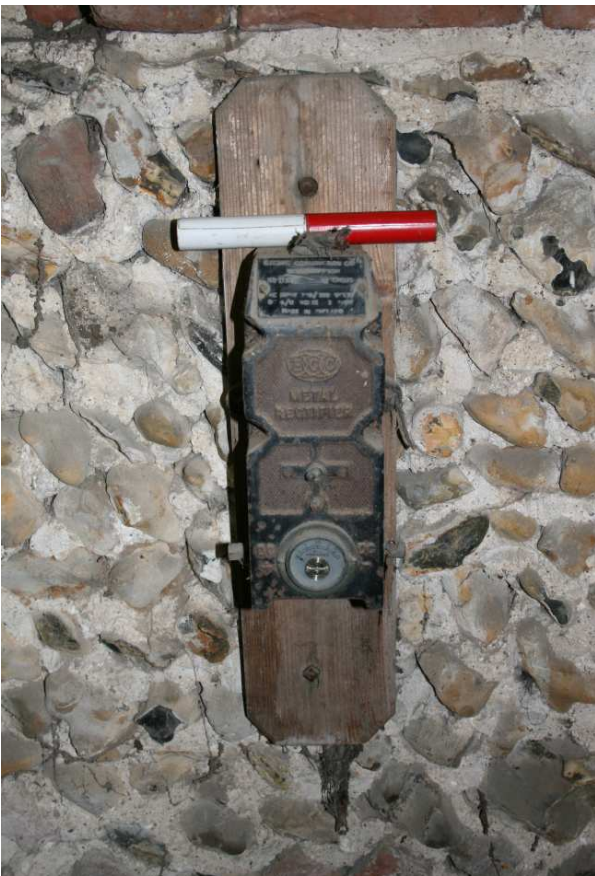
Plate 31: Barn: S elevation, ECC metal rectifier in Bay 3
