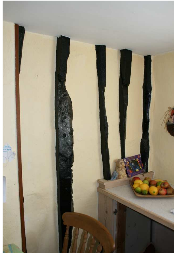
Plate 12: Cottage, kitchen, S elevation W end, showing exposed timber framing
