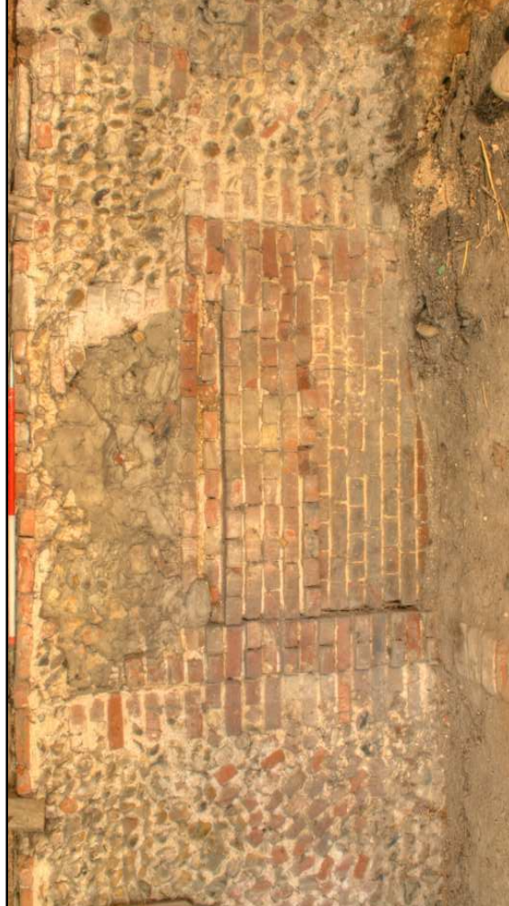
Plate 23: Barn: S elevation, detail of blocked opening in Bay 4
