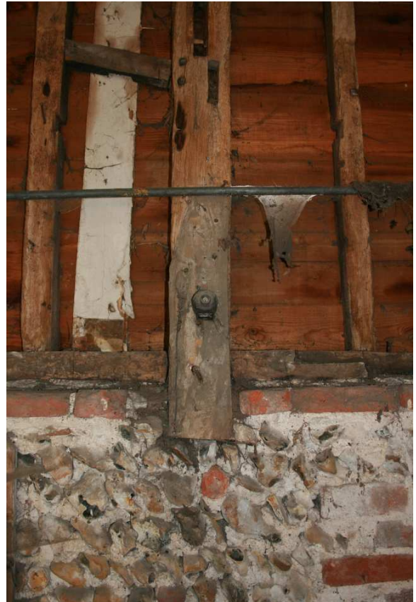
Plate 30: Barn: S elevation, detail of base of post between Bays 3 & 4
