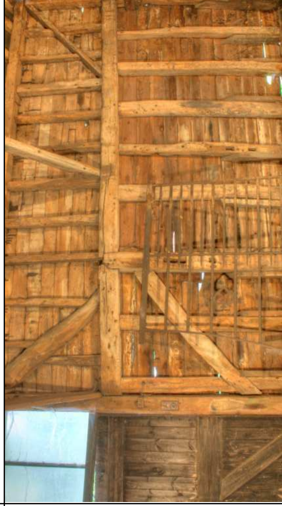
Plate 20: Barn, N elevation to E of doorway, looking N
