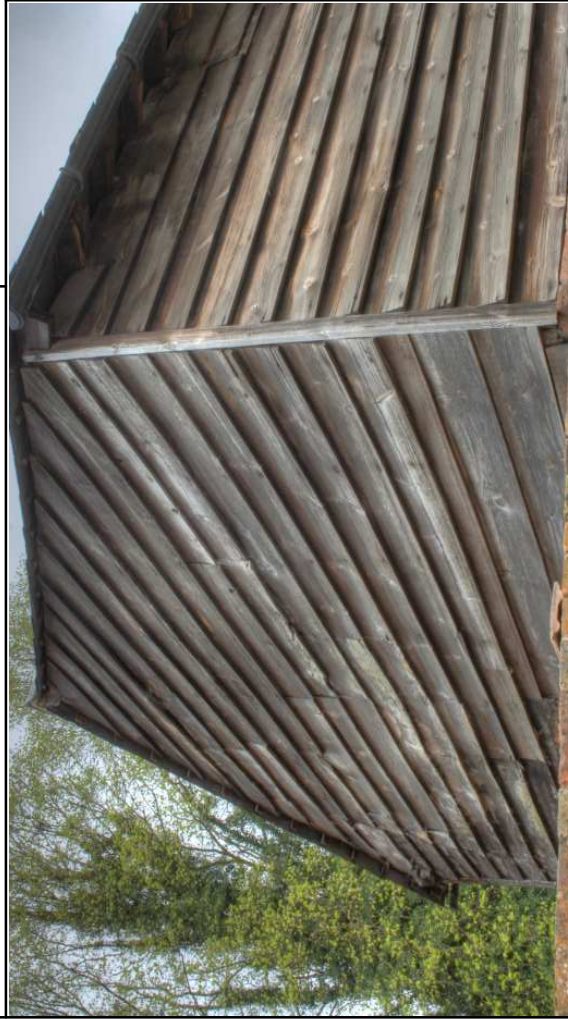
Plate 13: Barn, west elevation gable, looking SE
