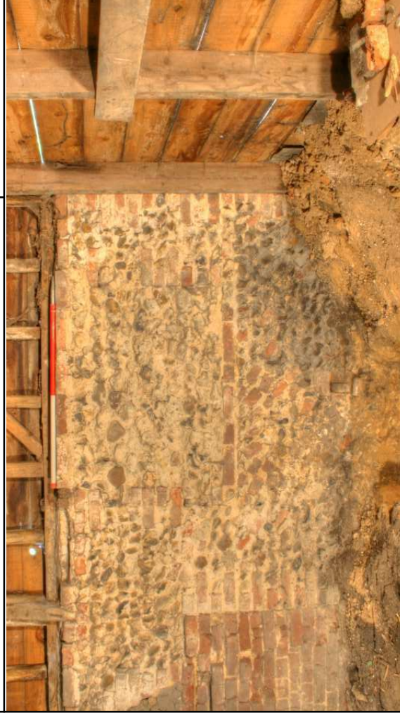
Plate 25: Barn, S elevation, detail of blocked opening in Bay 5
