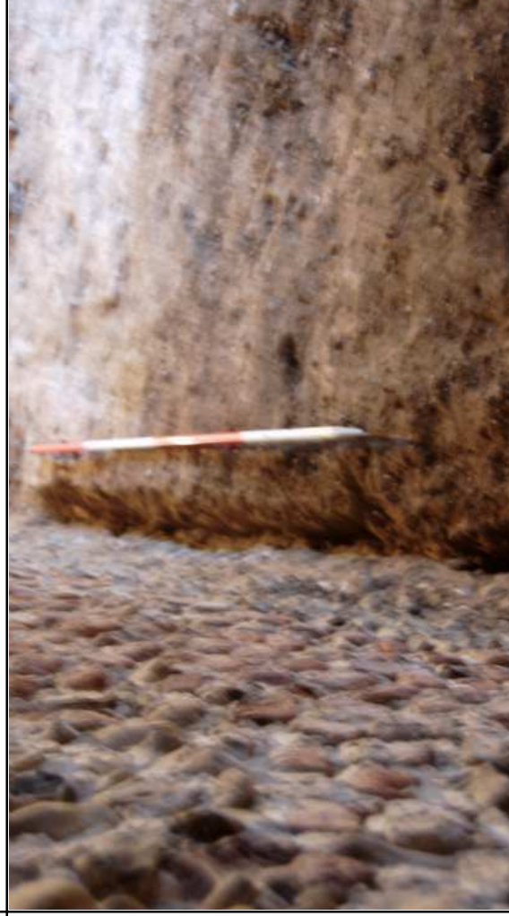
Plate 42: Air-raid shelter: detail of the floor & E wall, showing evidence for demolished blast wall
