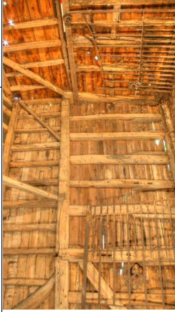
Plate 21: Barn, N & E elevations, looking NE
