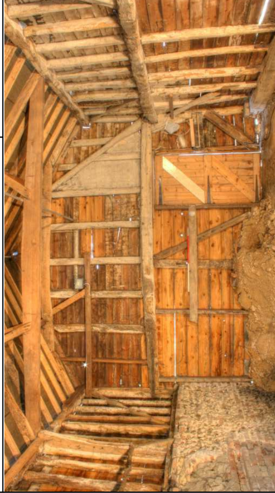
Plate 17: Barn, west interior elevation, looking W
