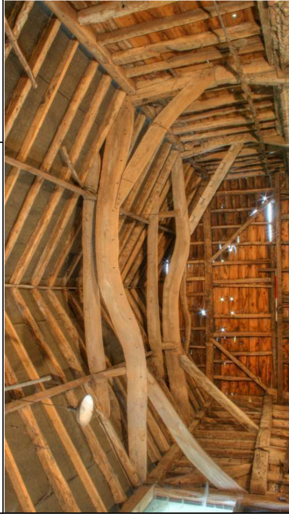
Plate 33: Barn: roof structure looking east
