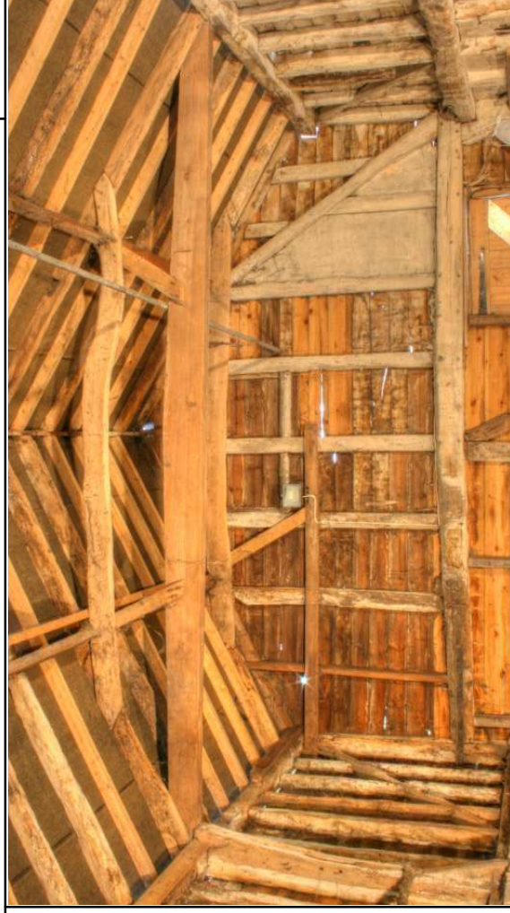
Plate 34: Barn: roof structure looking west
