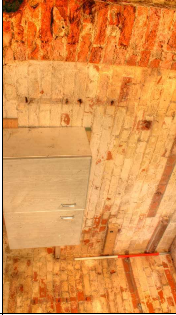
Plate 40: Air-raid shelter: E interior elevation
