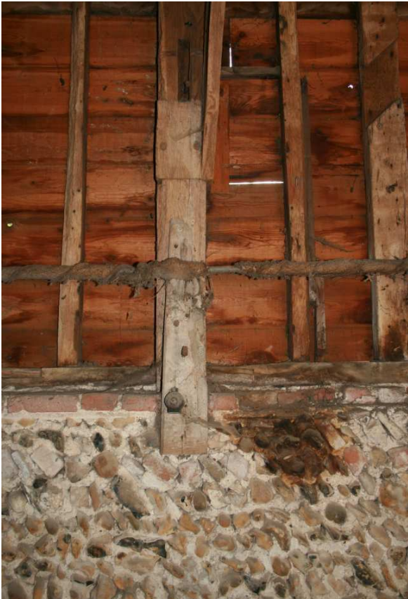
Plate 29: Barn: S elevation, detail of base of post between Bays 1 & 2
