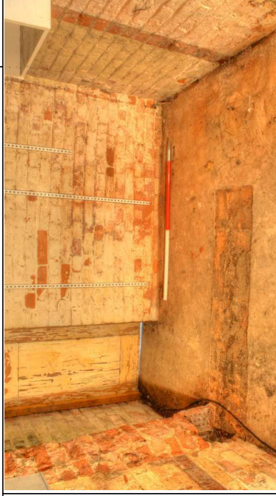
Plate 42: Air-raid shelter: detail of the floor & E wall, showing evidence for demolished blast wall
