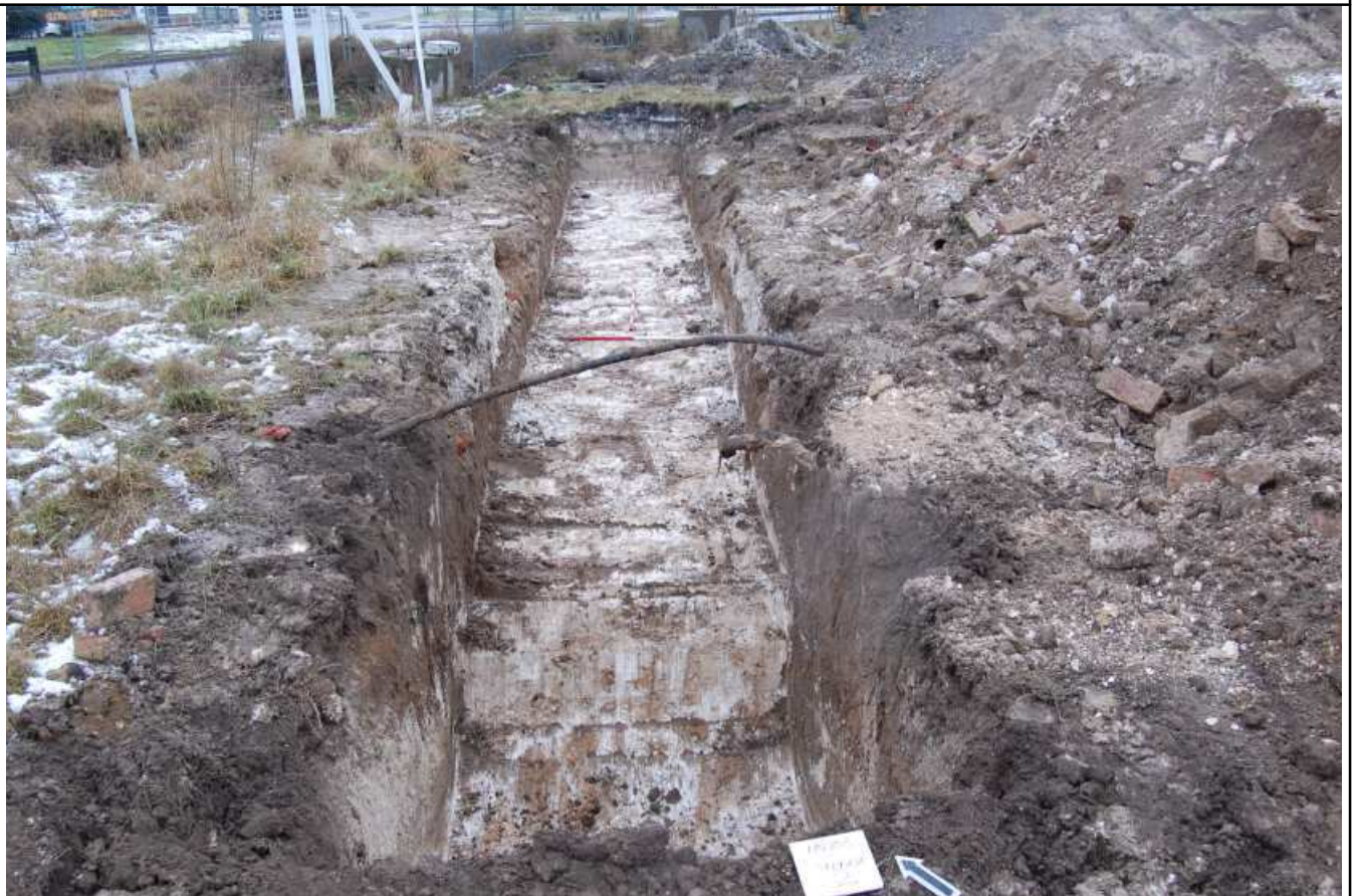
Plate 2: Trench 7, looking north-east
