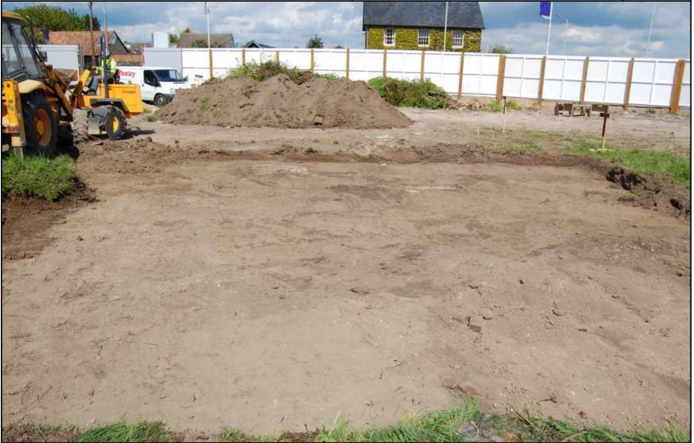
Plate 3: Topsoil stripping, southern end of site, looking north
