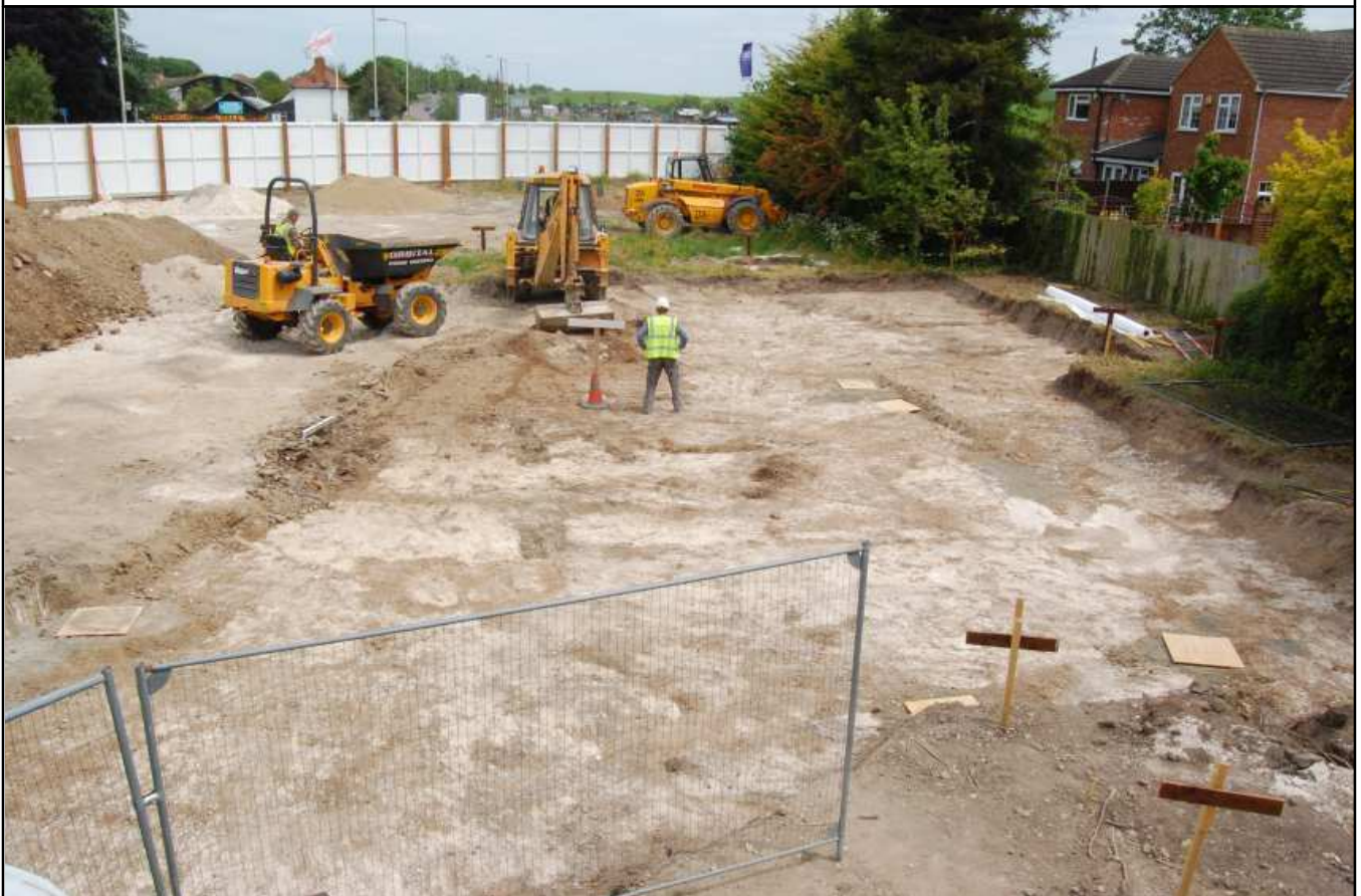
Plate 4: Ground reduction in car park area
