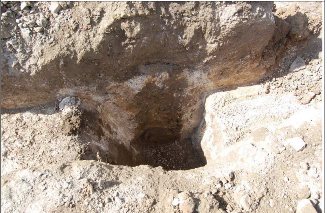
Plate 12: Well in footings trench, Plots 7-12
