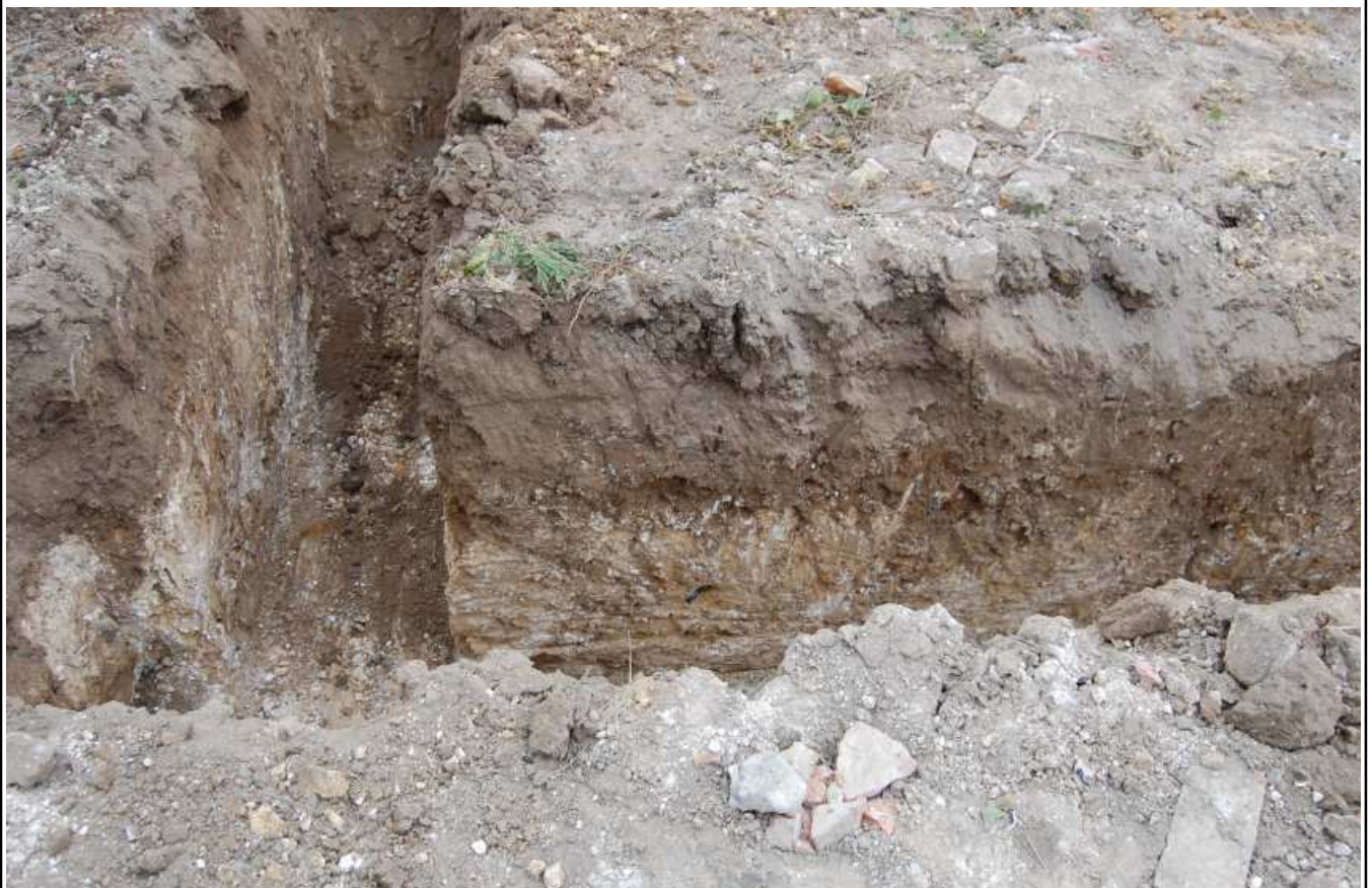
Plate 10: Sample section, footings trench Plots 13-14
