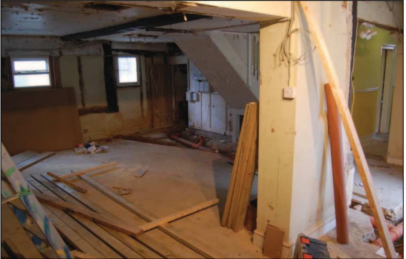
Plate 5: Interior shot, looking west, showing location of removed walls
