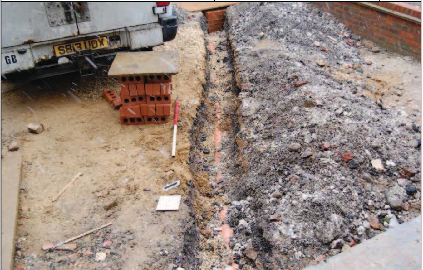
Plate 9: Exterior drainage trench, looking NE
