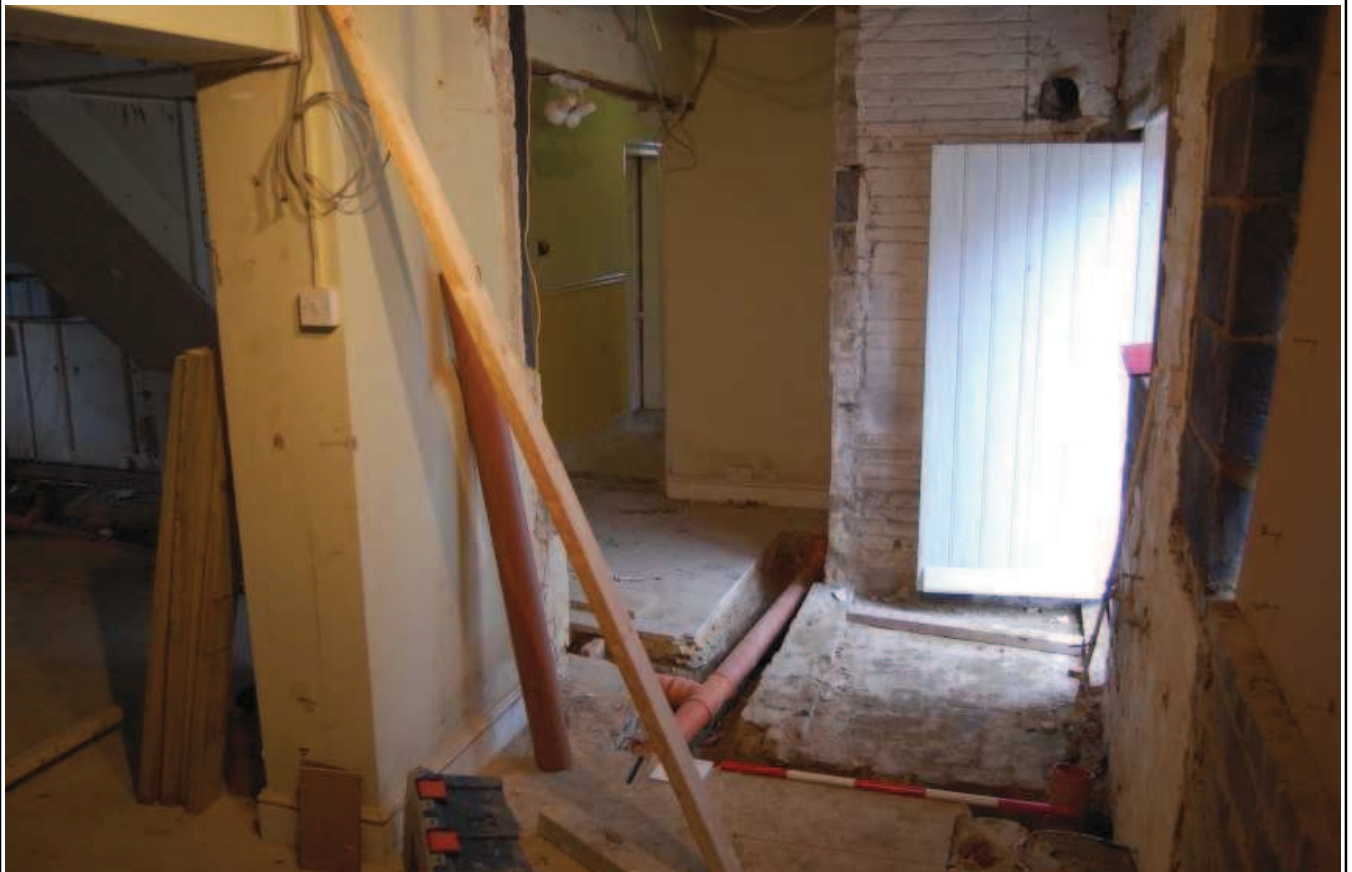
Plate 4: Interior shot, looking N showing location of walls removed
