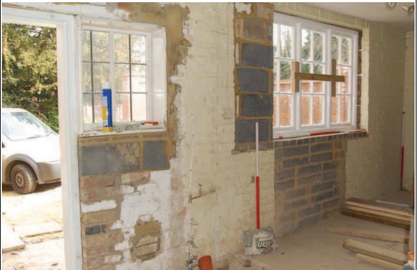
Plate 8: Former lobby & recess, east interior elevation, looking SE
