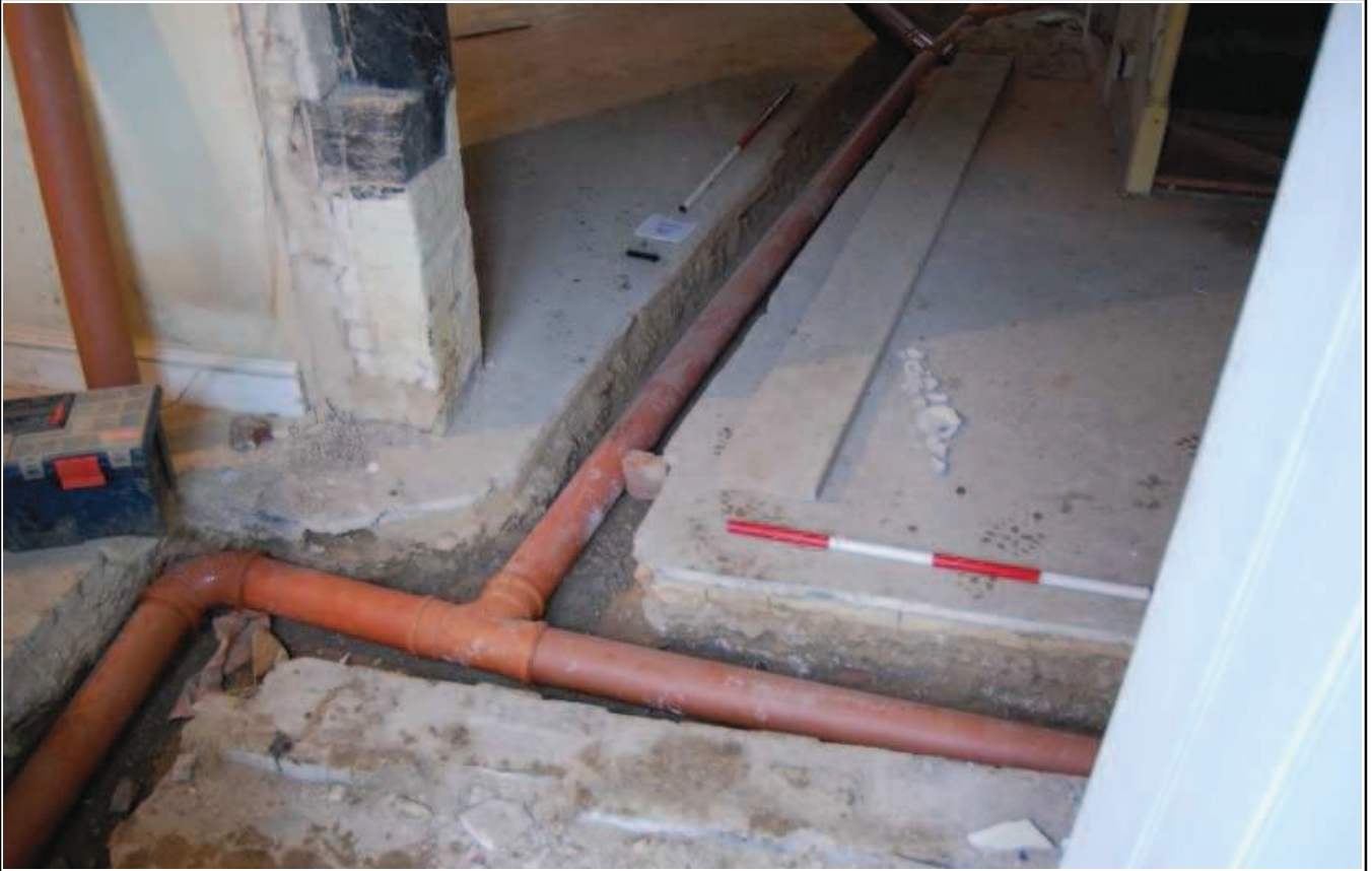
Plate 11: Interior service trenches, central area, showing concrete floor above brick floor
