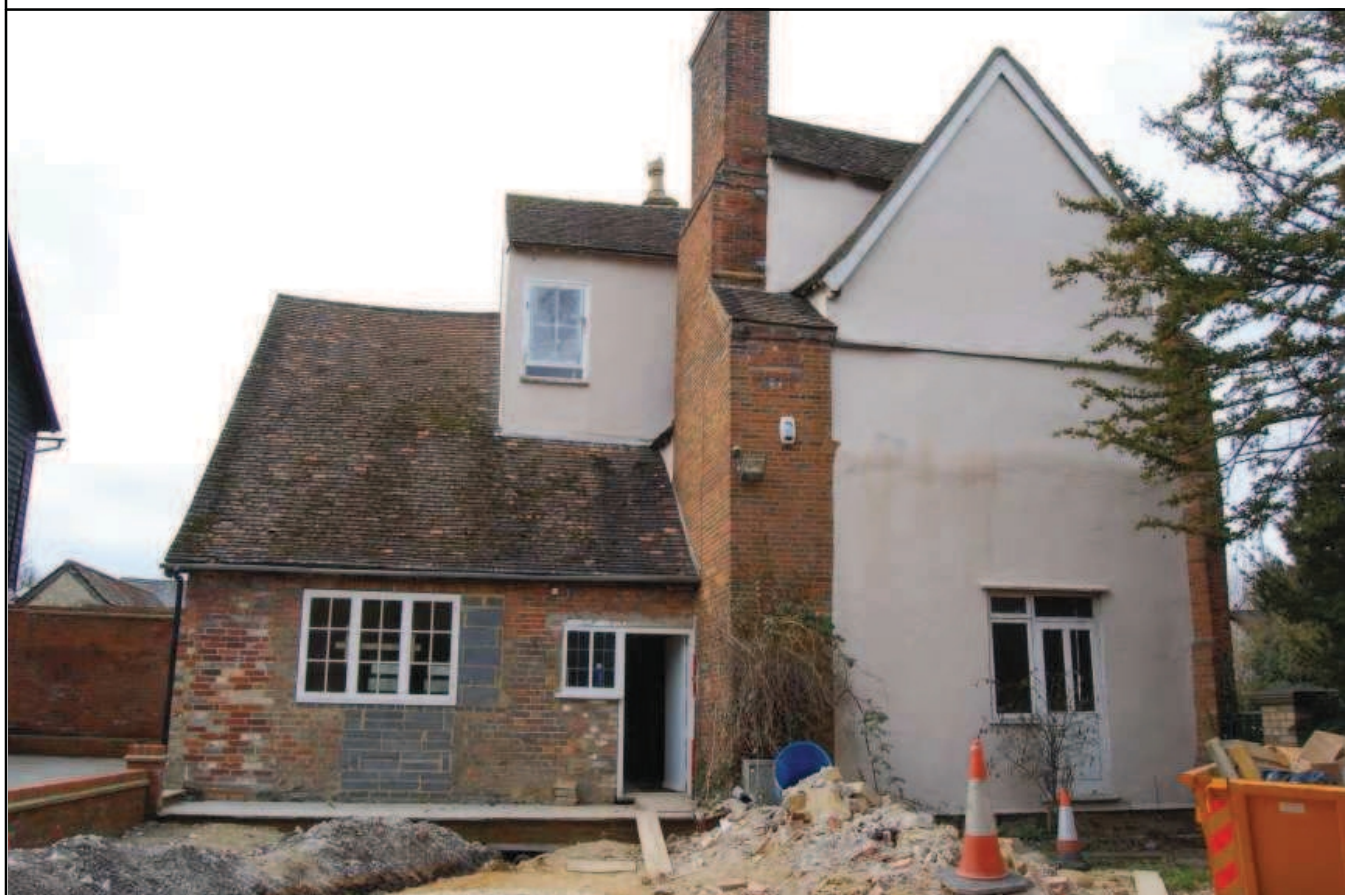
Plate 2: East exterior elevation
