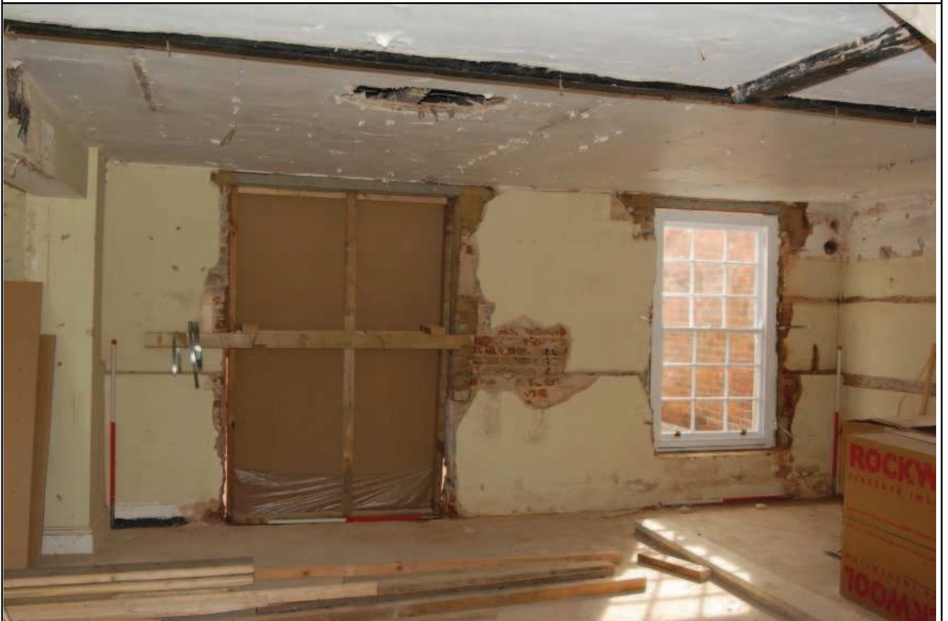
Plate 6: South interior elevation, looking south
