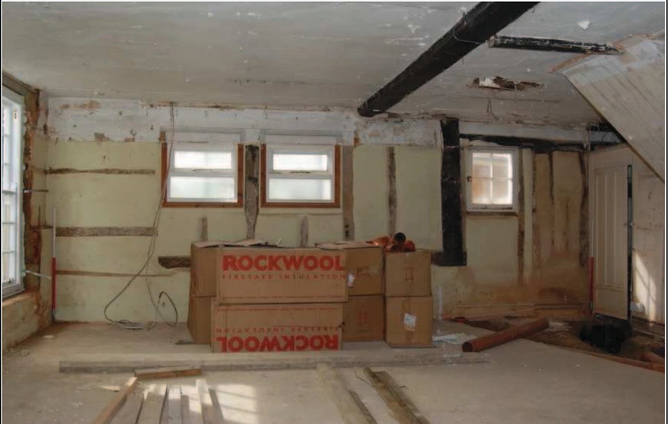
Plate 7: West interior elevation, looking west
