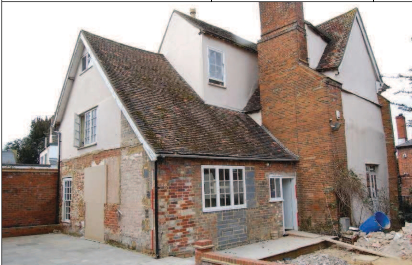
Plate 1: South and east exterior elevations
