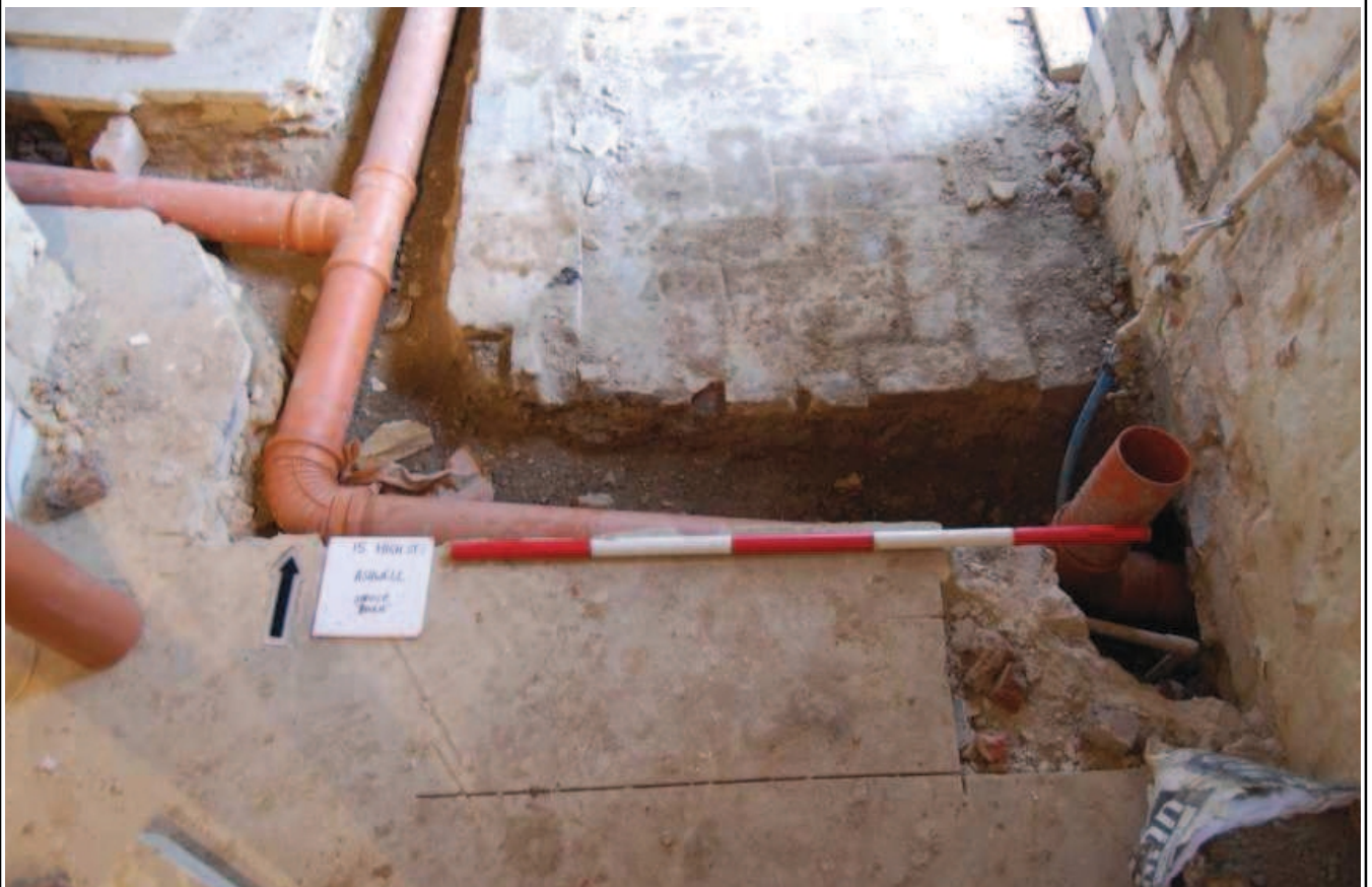
Plate 12: Interior service trenches, former lobby and recess, showing brick floor
