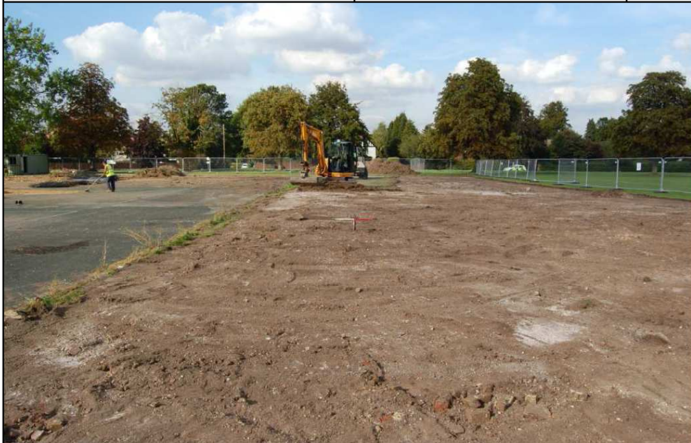
Plate A1: Rubble deposit after removal of topsoil, looking north.
