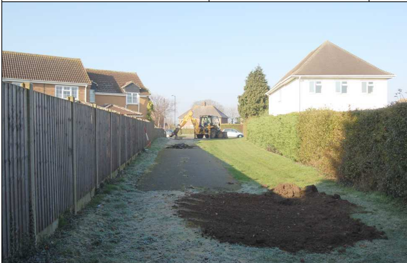
Plate 1: General site view, looking west.
