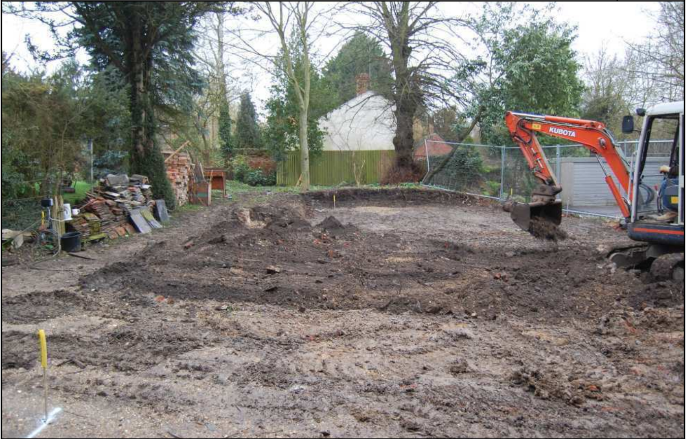
Plate 1: General site view, looking north.
