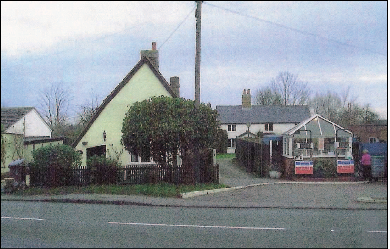
Plate 1: Forecourt and kiosk, prior to demolition, looking north. (Courtesy of Attfield and Jones Architects)
