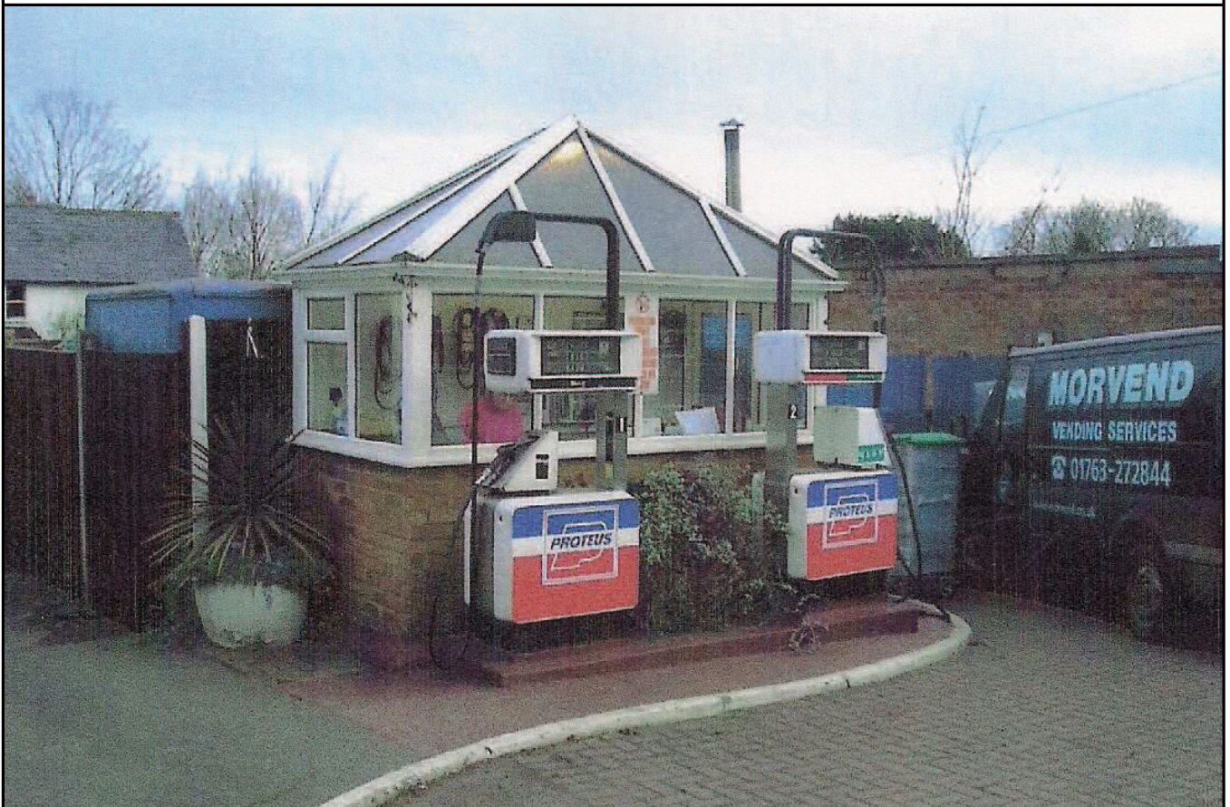
Plate 4: Kiosk and petrol pumps, prior to demolition, looking northeast. (Courtesy of Attfield and Jones Architects)
