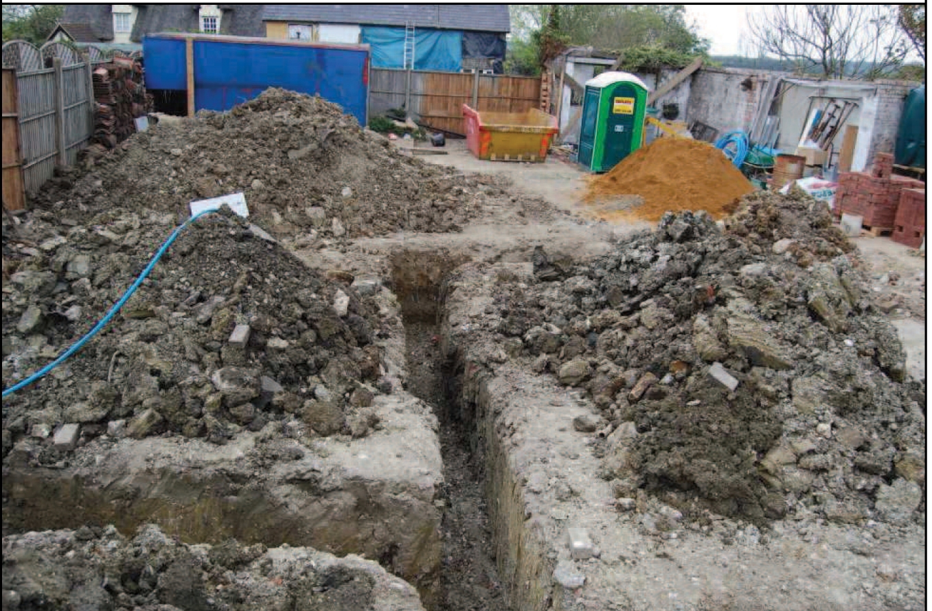
Plate 8: General site view showing groundworks, looking north.
