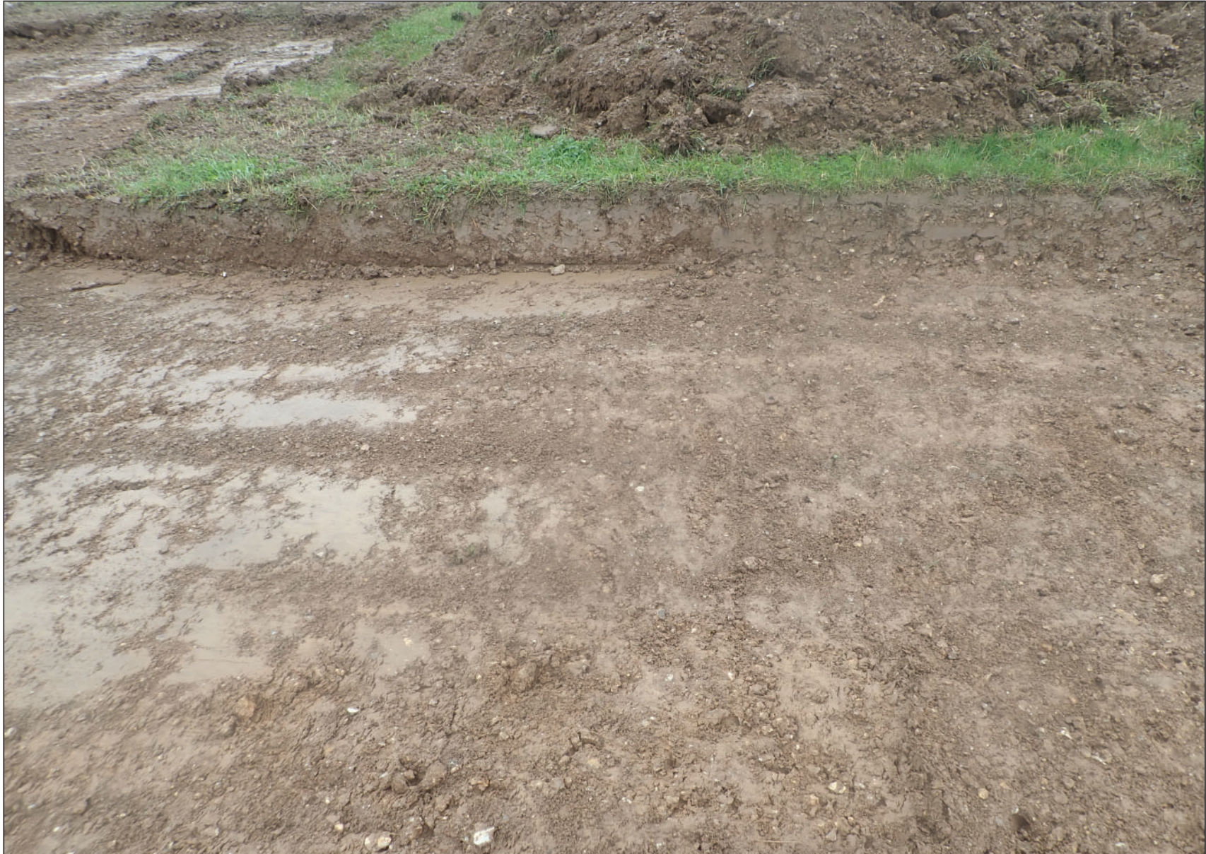
Plate 3 - Representative section through haul road showing depth of topsoil removal, looking northeast
