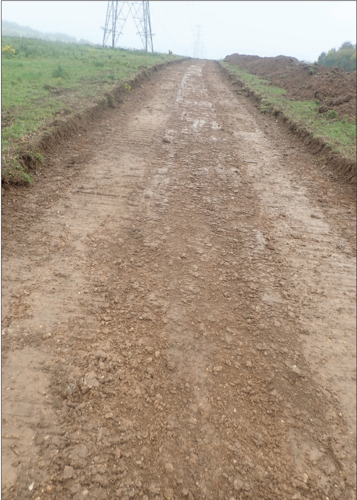
Plate 2 - Overview of haul road after topsoil removal, looking northwest
