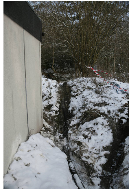
Plate 4 Trench looking east
