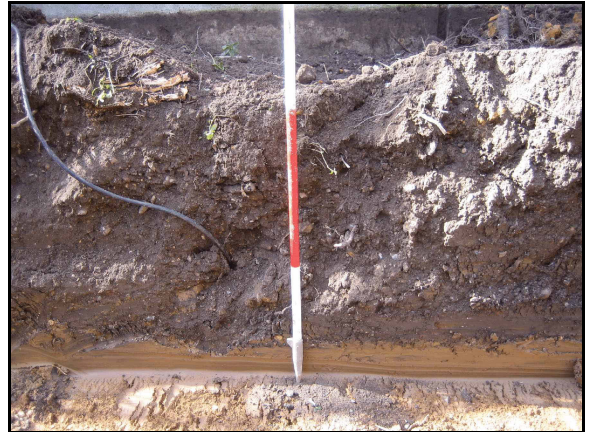
Plate 2 Trench 6: west section
