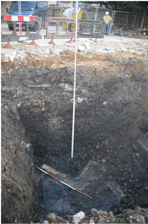
Plate 1 Trench 1: south end
