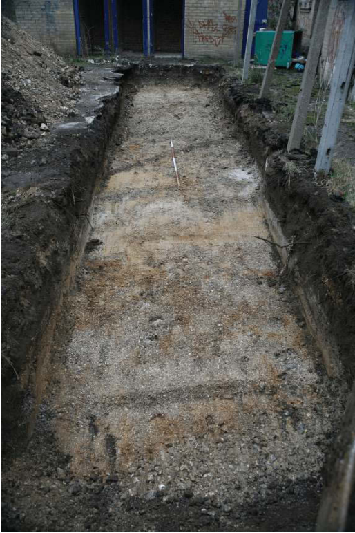
Plate 6 Tr. 4: looking east
