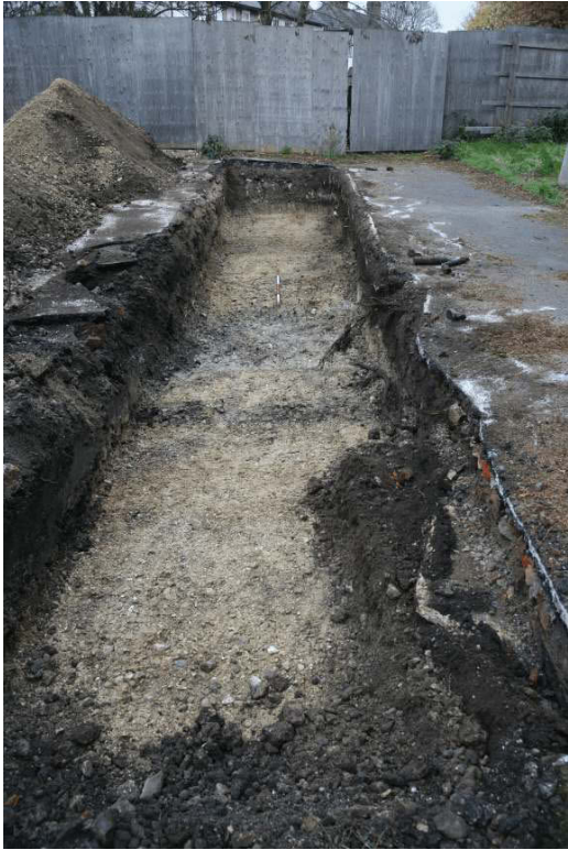
Plate 9 Tr. 5: looking east
