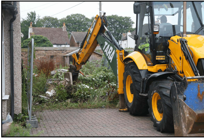
Plate 1 General view of site
