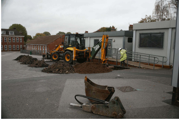
Plate 1 General view, looking north
