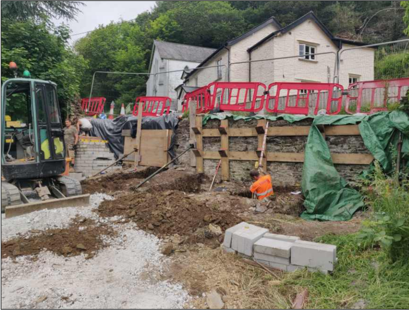
Plate 1: General working view during construction groundworks. Looking north
