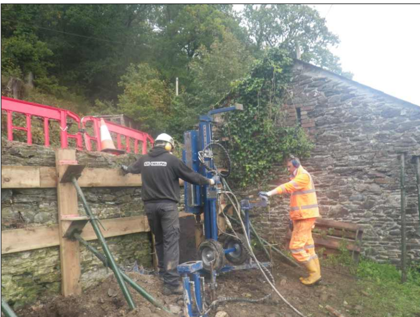
Plate 3: Working view during geotechnical investigations, looking northeast
