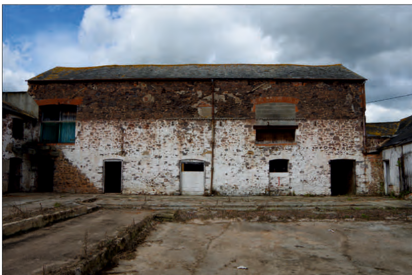
Plate 3: South elevation of north barn, looking north (1m scale)
