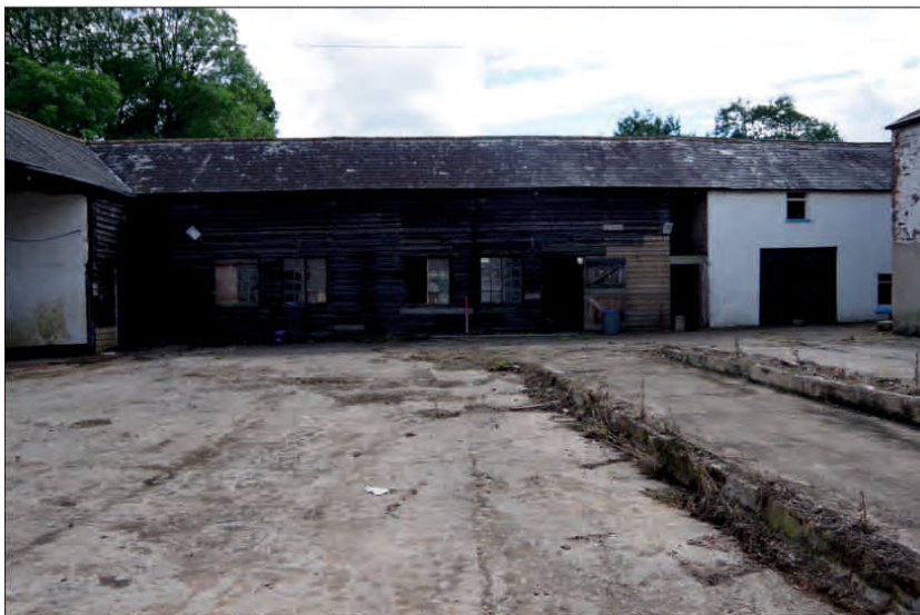
Plate 11: North elevation of south barn, looking north (1m scale)
