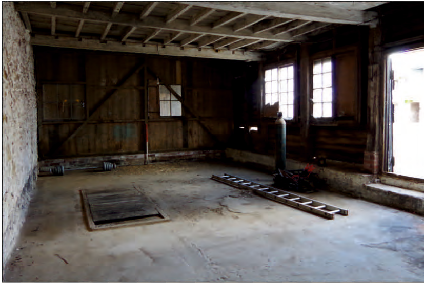
Plate 13: General view of east room on the ground floor of the south barn, looking northwest (1m scale)
