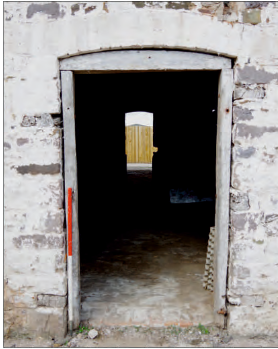
Plate 4: Peg-jointed timber door frame in south elevation of the north barn, looking north (1m scale)
