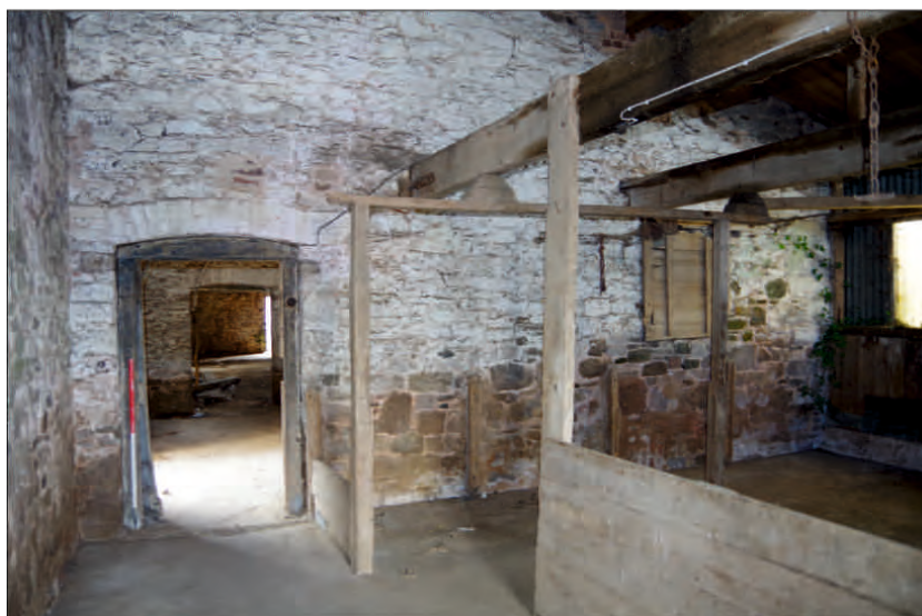
Plate 18: North elevation of west barn, looking southwest (1m scale)
