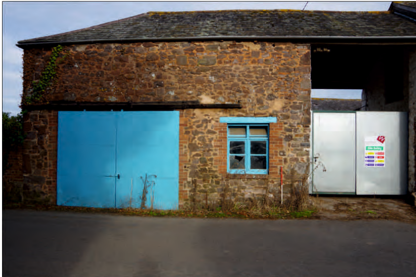
Plate 10: East elevation of south barn, looking west (1m scale)
