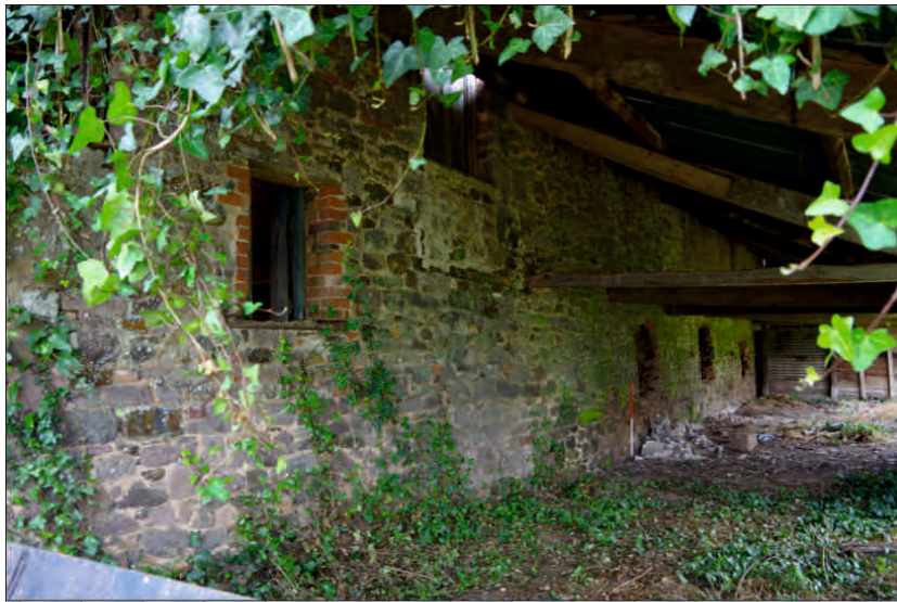
Plate 19: West elevation of west barn, looking southeast (1m scale)
