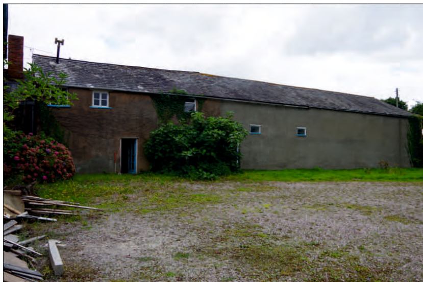
Plate 9: South elevation of south barn, looking northeast (1m scale)
