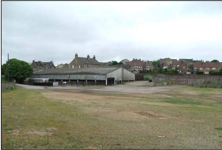
Figure 4 General view of the mart, showing open parking areas, pens and sheds. The pub is visible above the recent portal-frame sheds: looking NW
