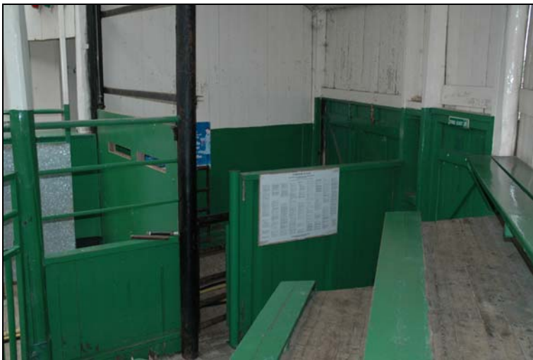
Figure 26 The exit from the ring to the raceways. The sliding door with the viewing slits slides vertically in the black frame: N
