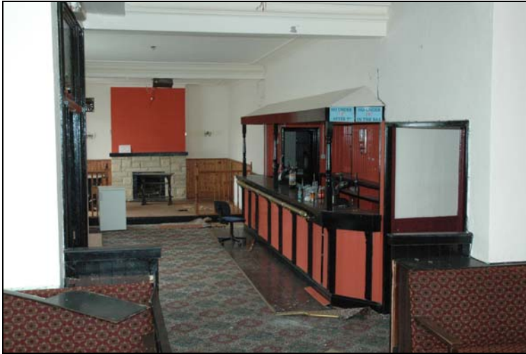
Figure 13 View along the bar. Former wall lines are visible as boxed-in joists on the ceiling: N
