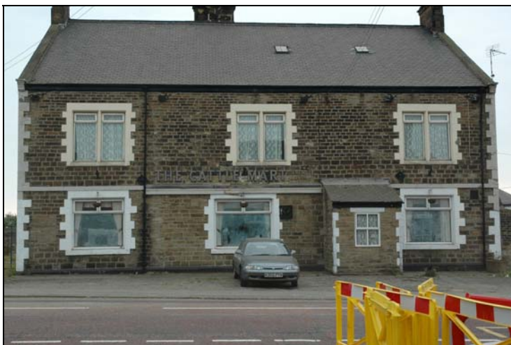
Figure 12 The front of the pub. Alterations to the ground floor windows are apparent left of the later porch: E
