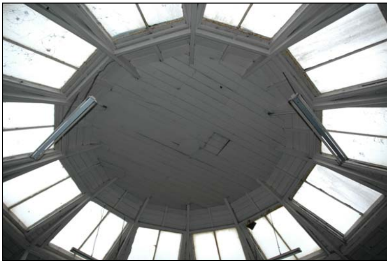
Figure 20 View of the roof of the ring
