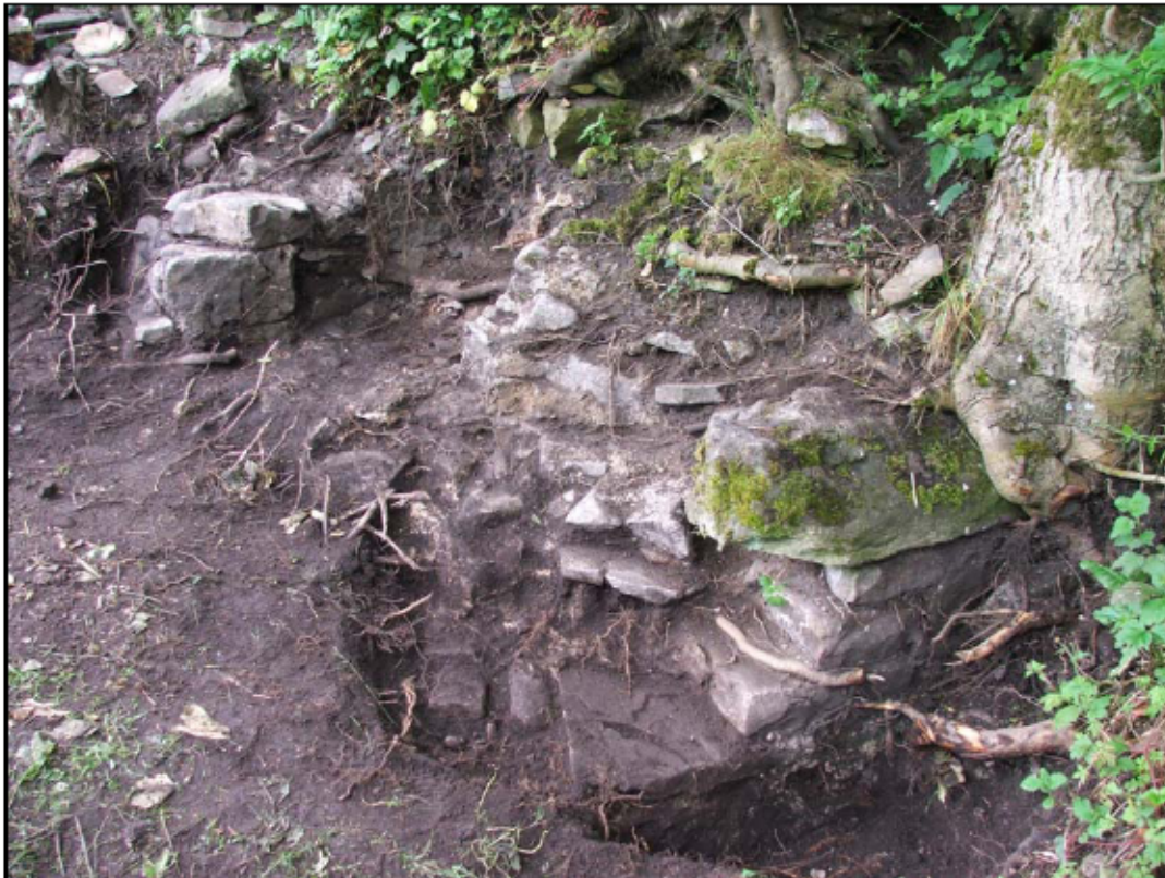
Figure 31: Masonry exposed at the base of the bank of the northern boundary lane, facing east
