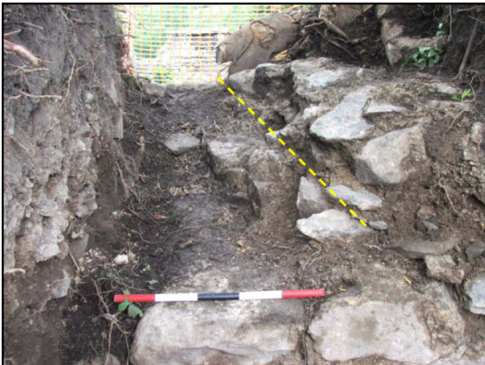
Figure 17: Wall [F66], facing west. The line of the north side of window [F55] is indicated
