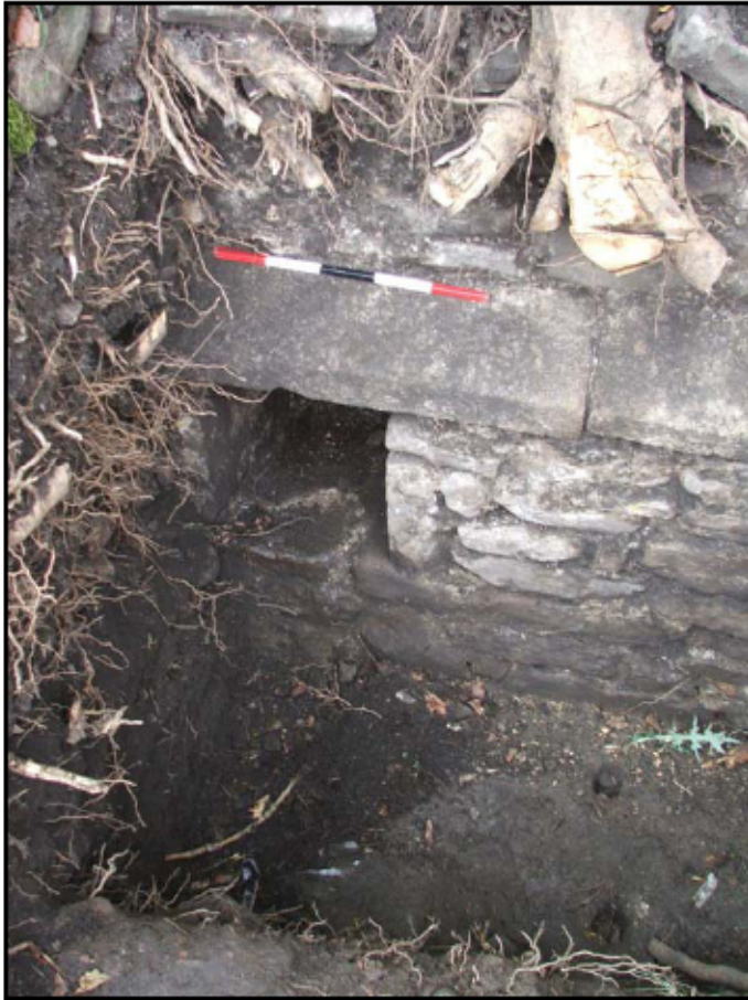
Figure 18: The west face of wall [F66], showing string course [41] and the exit of the garderobe chute [F42]
