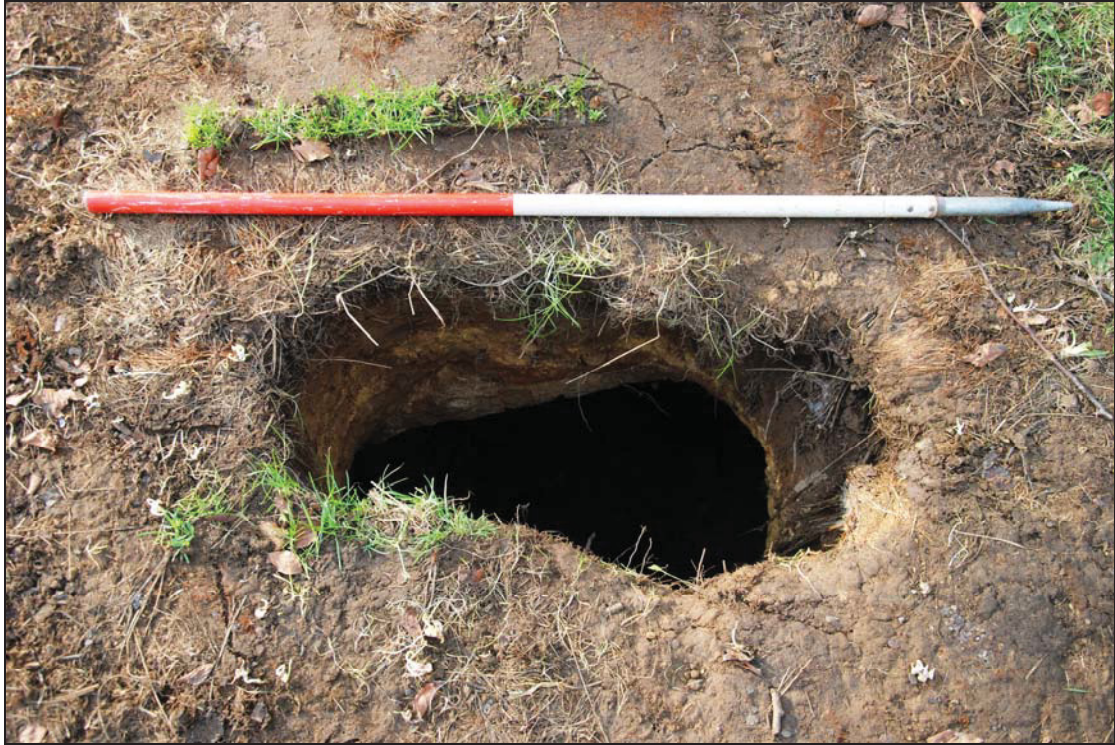
Figure 9: The hole into the 'bridge' structure at Area 1
