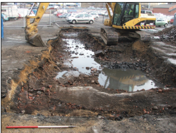
Figure 7 Concrete foundations in Trench 2 (looking east)
