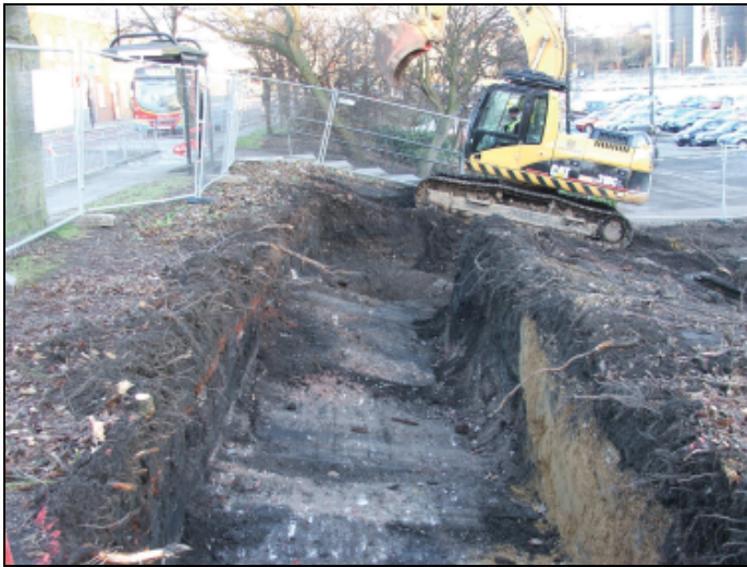
Figure 5 Made ground in Trench 1 (looking east)
