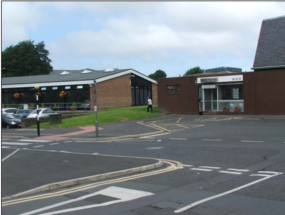
Figure 11: Raised bank south-west of Teanlowe Centre
