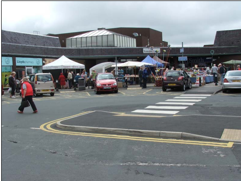
Figure 9: Teanlowe Centre, main entrance looking southeast
