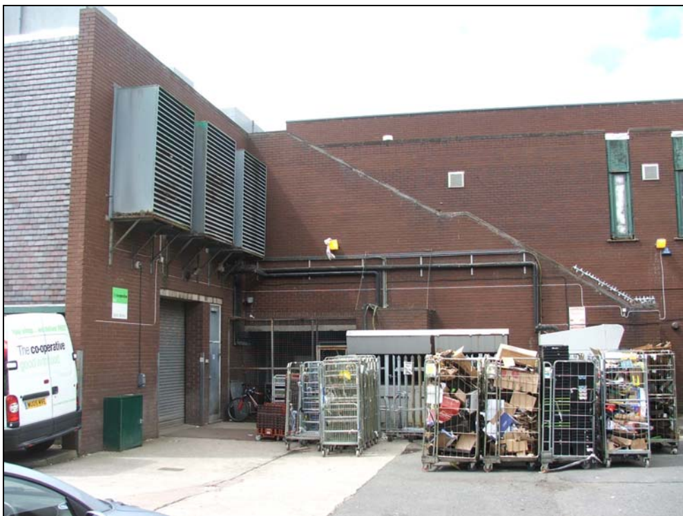
Figure 12: Service yard to east of Teanlowe Centre
