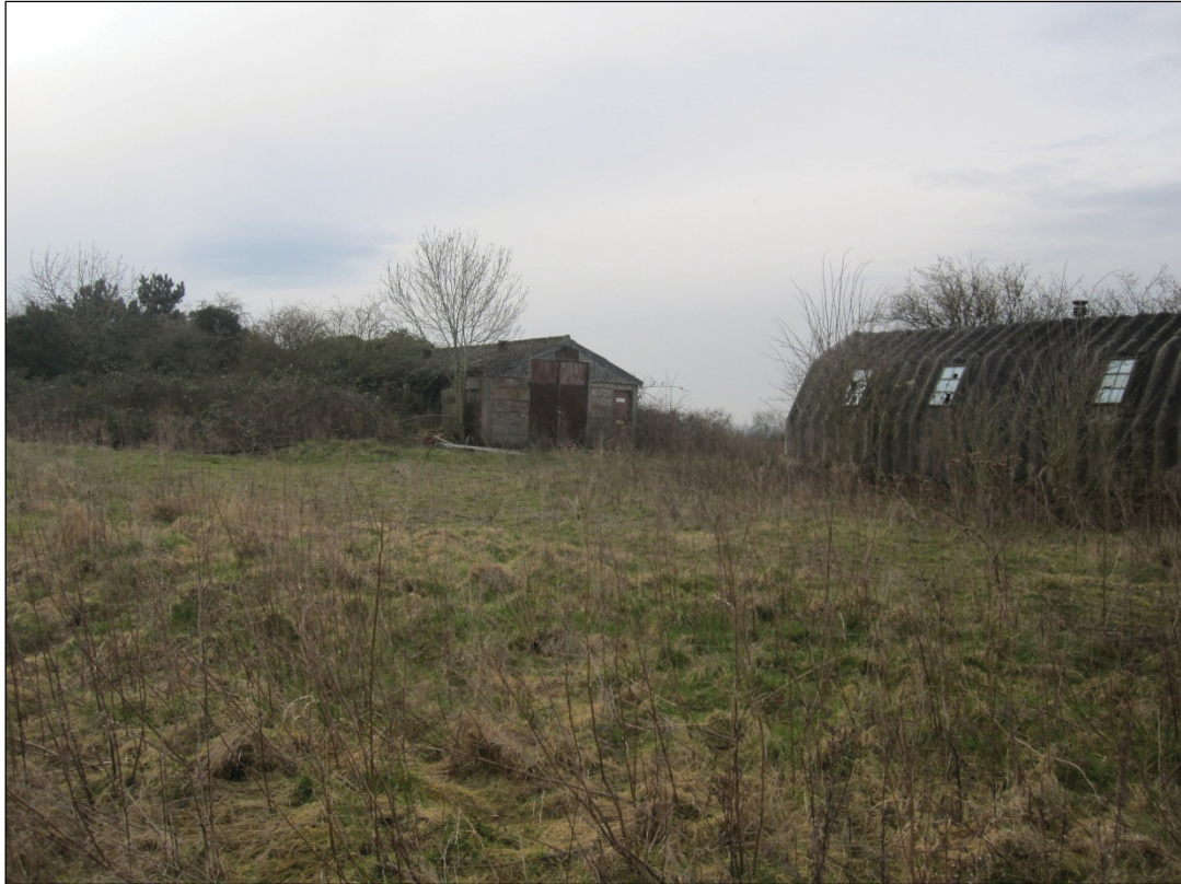
Figure 13: Huts in the centre of the site, looking south-east
