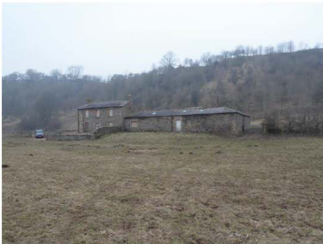
Area 4, looking NW to farm buildings
