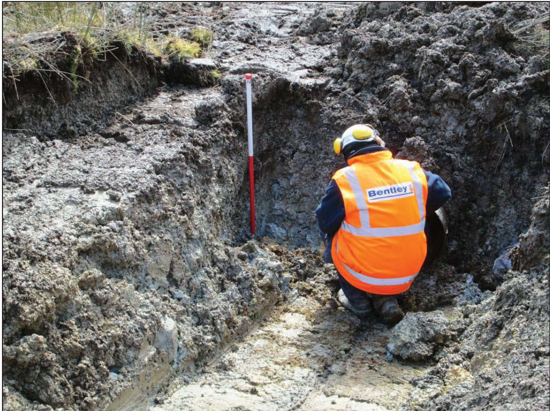
Figure 6: Excavating Chamber 3, looking north
