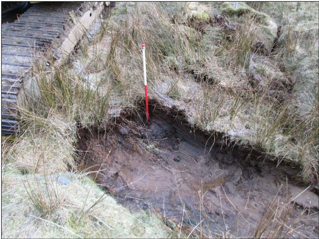
Figure 9: Excavation for the gabion basket
