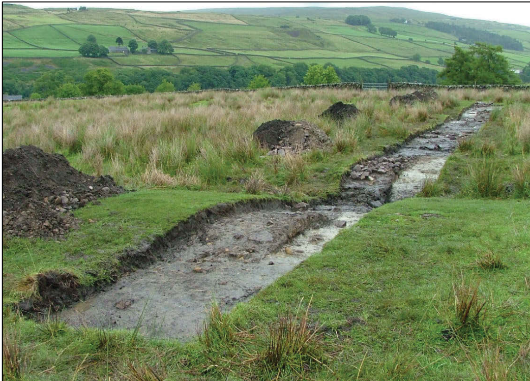
Figure 4: Trench 1, looking north
