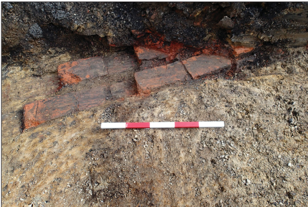
Figure 13: Trench 42, brick culvert [F43], facing east
