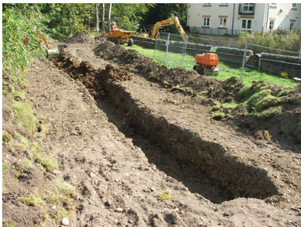
Figure 3: The monitored area during groundworks, looking south-east
