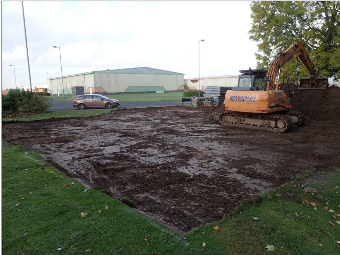
Figure 3: Topsoil strip for site compound, looking north-west
