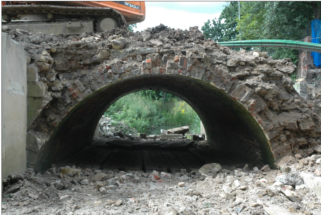
Figure 32: Main channel following the removal of stone facing, looking south-west
