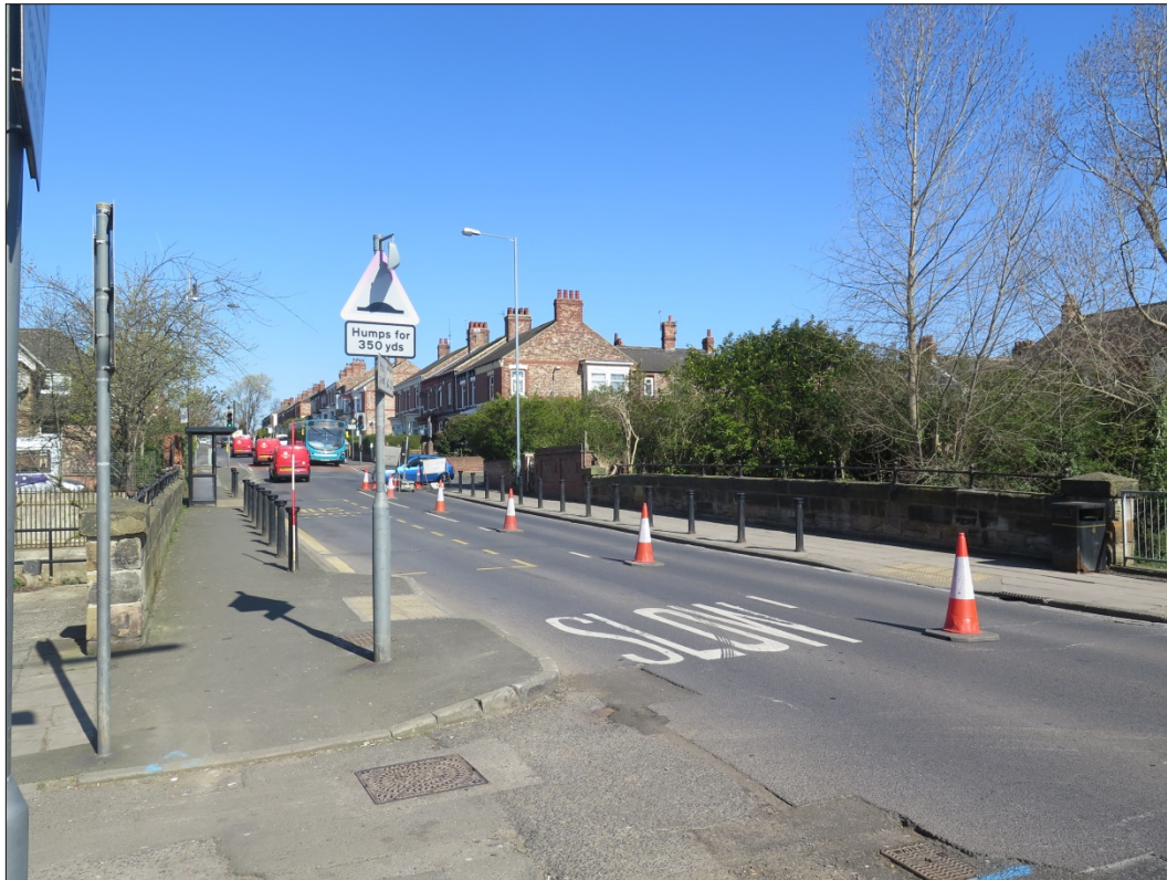
Figure 10: Oblique view across the bridge, looking north
