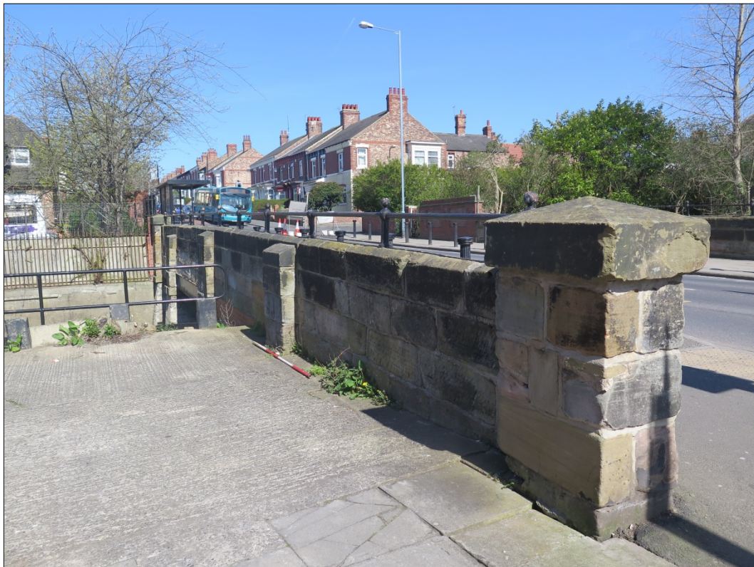
Figure 15: South-western elevation, external parapet, looking north
