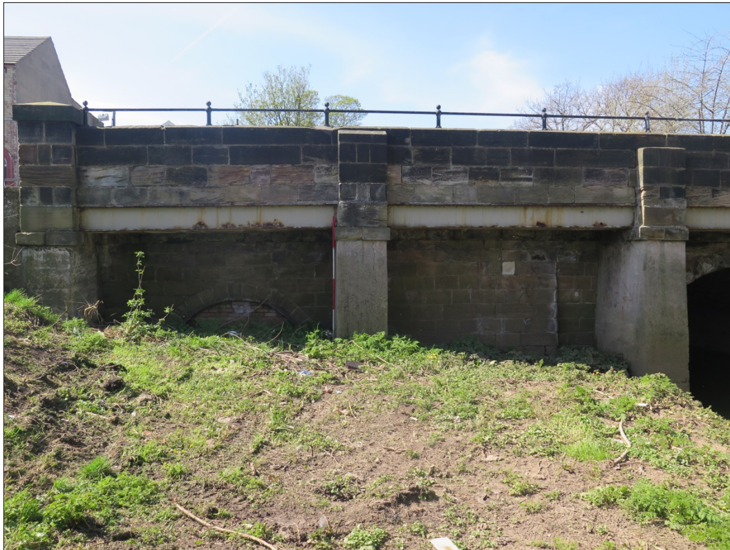
Figure 26: North-eastern elevation, detail of piers 1-3 and spans, looking south-west
