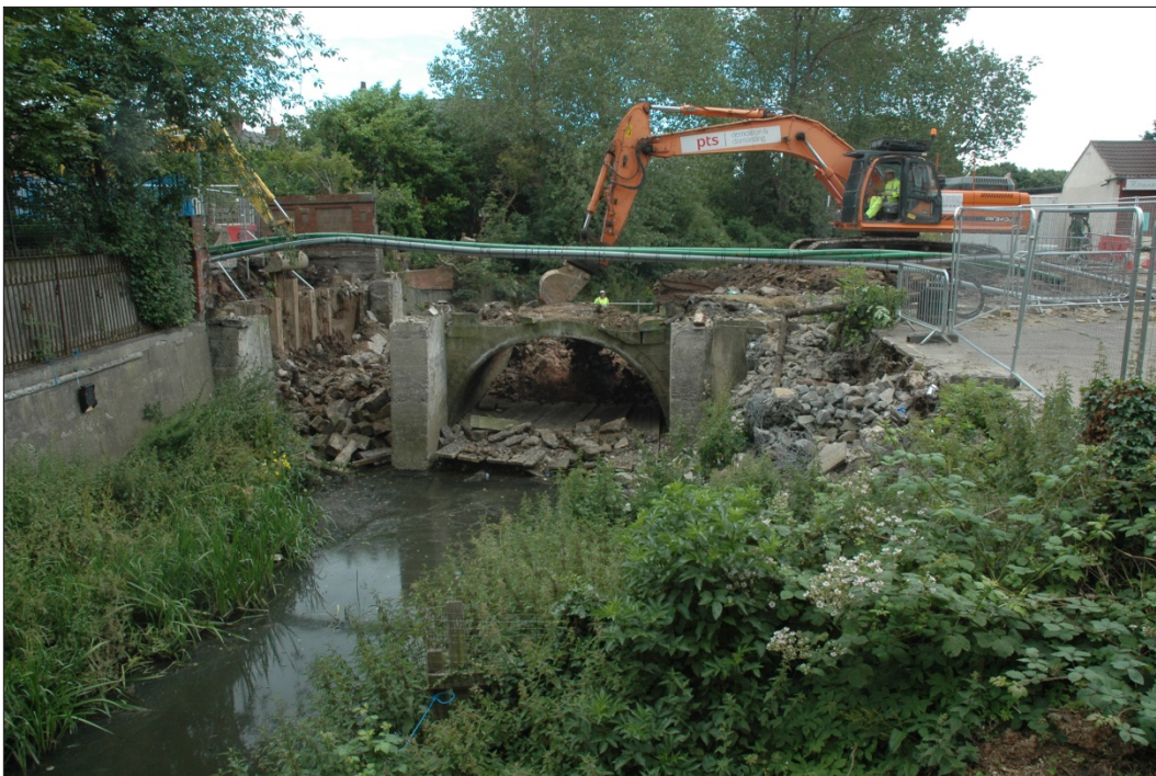
Figure 41: Demolition of the main channel, looking north-east
