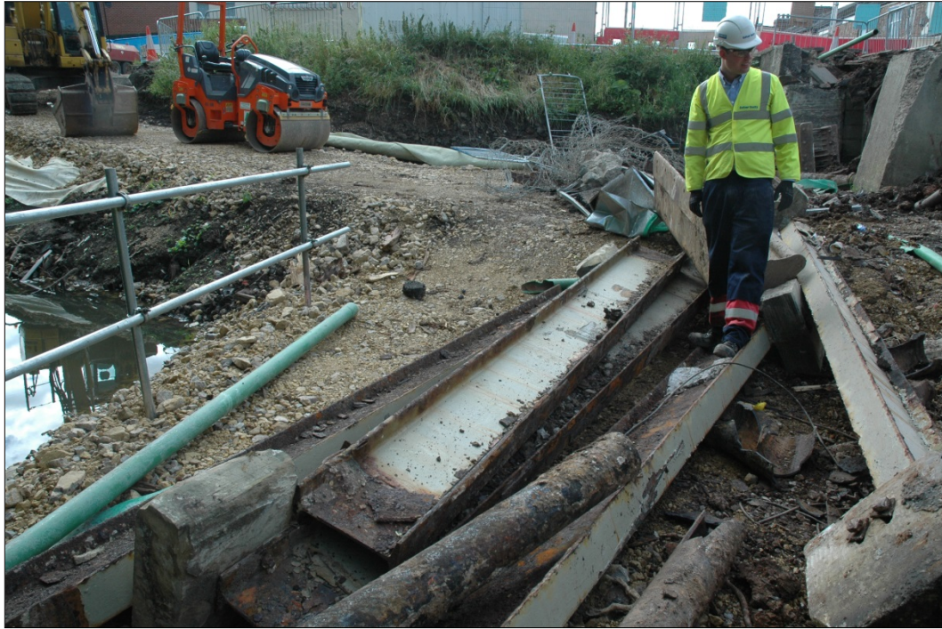
Figure 34: The steel lintels removed, looking south
