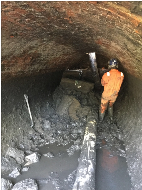
Figure 35: Southern-most channel during re-excitation, looking south-west
