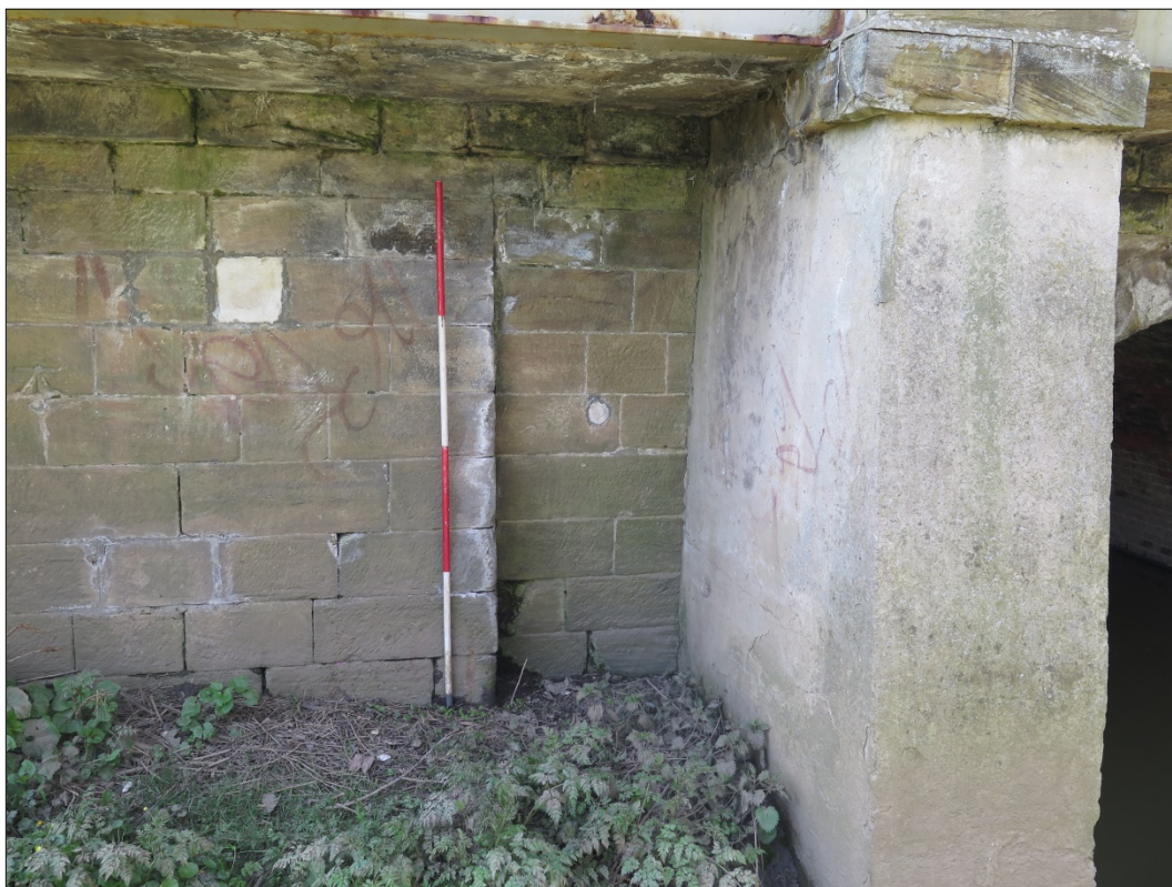
Figure 29: North-eastern elevation, detail of buttress between piers 2 and 3, looking west
