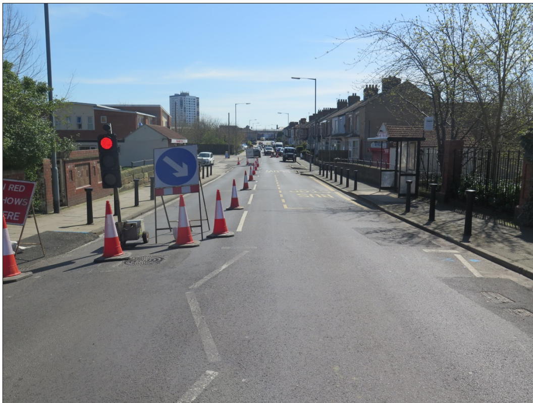
Figure 31: View across the bridge and along the Durham road, looking south-east
