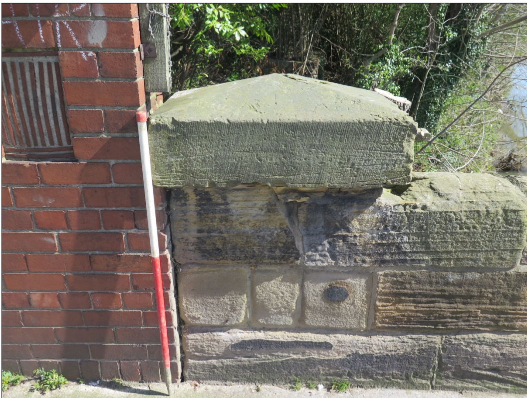
Figure 21: North-eastern pillar, looking north-east
