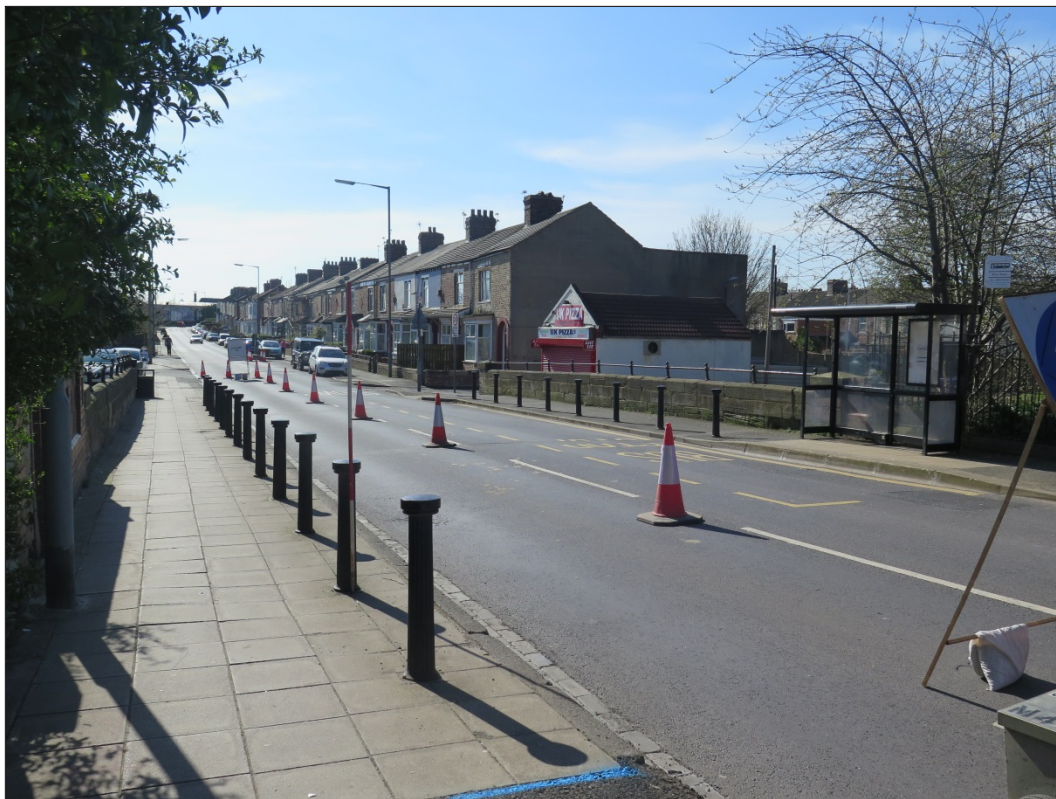
Figure 11: Oblique view across the bridge, looking south
