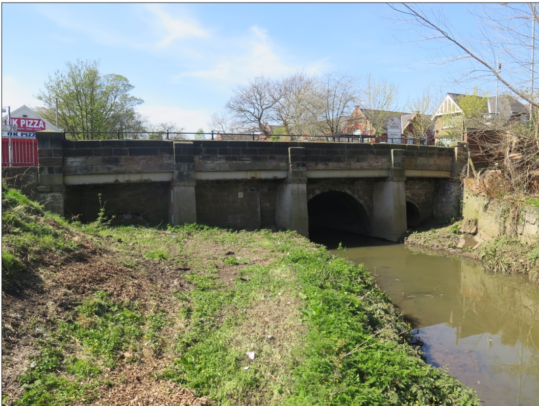
Figure 25: North-eastern elevation, looking west
