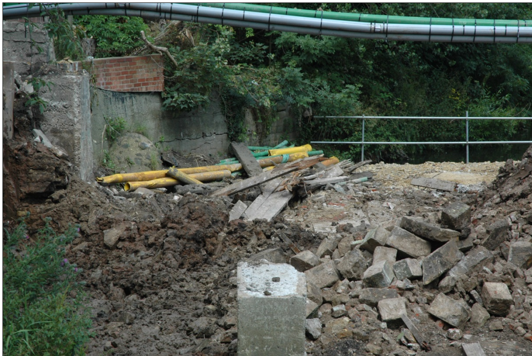
Figure 43: Wooden beams recovered from beneath the northern channel, looking north-east
