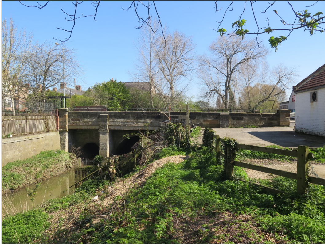
Figure 12: South-western elevation, looking north-east
