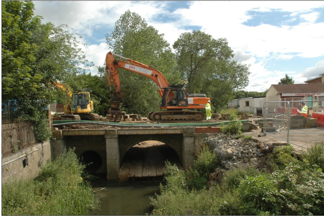
Figure 38: Removal of parapet and road surfaces, looking north-east
