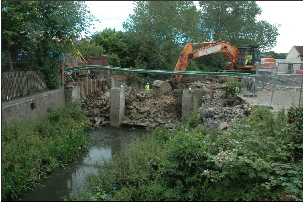
Figure 42: The main channel, following demolition, looking north-east
