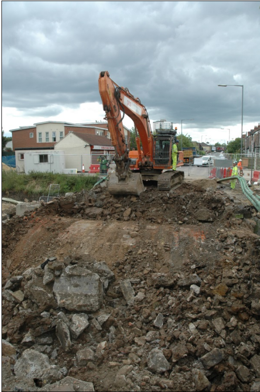
Figure 40: The excavation of the main channel, looking south-east
