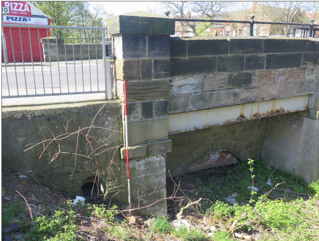
Figure 22: South-eastern pillar and concrete pier, looking west
