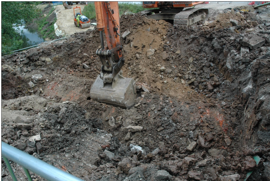
Figure 39: The excavation and demolition of the northern-most channel, looking east
