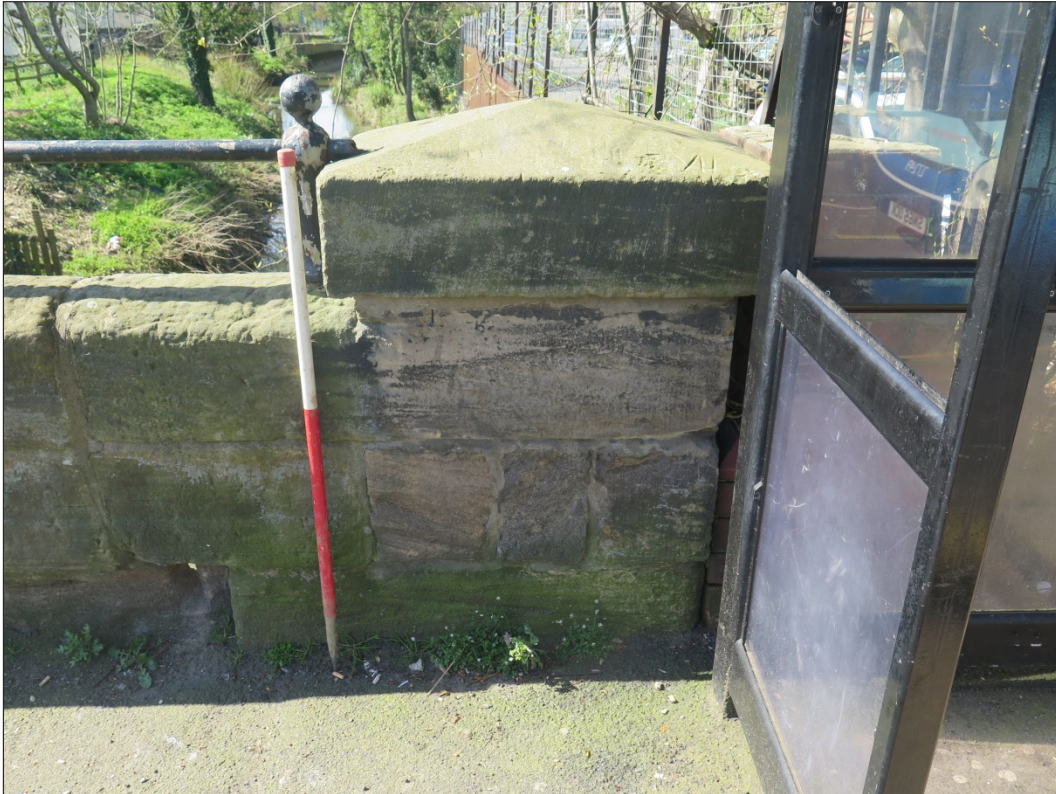
Figure 20: North-western pillar, looking south-east
