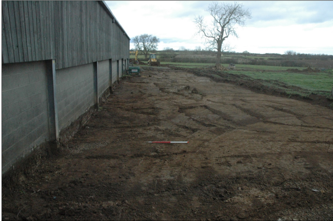
Figure 4: The western half of the site after excavation, looking north
