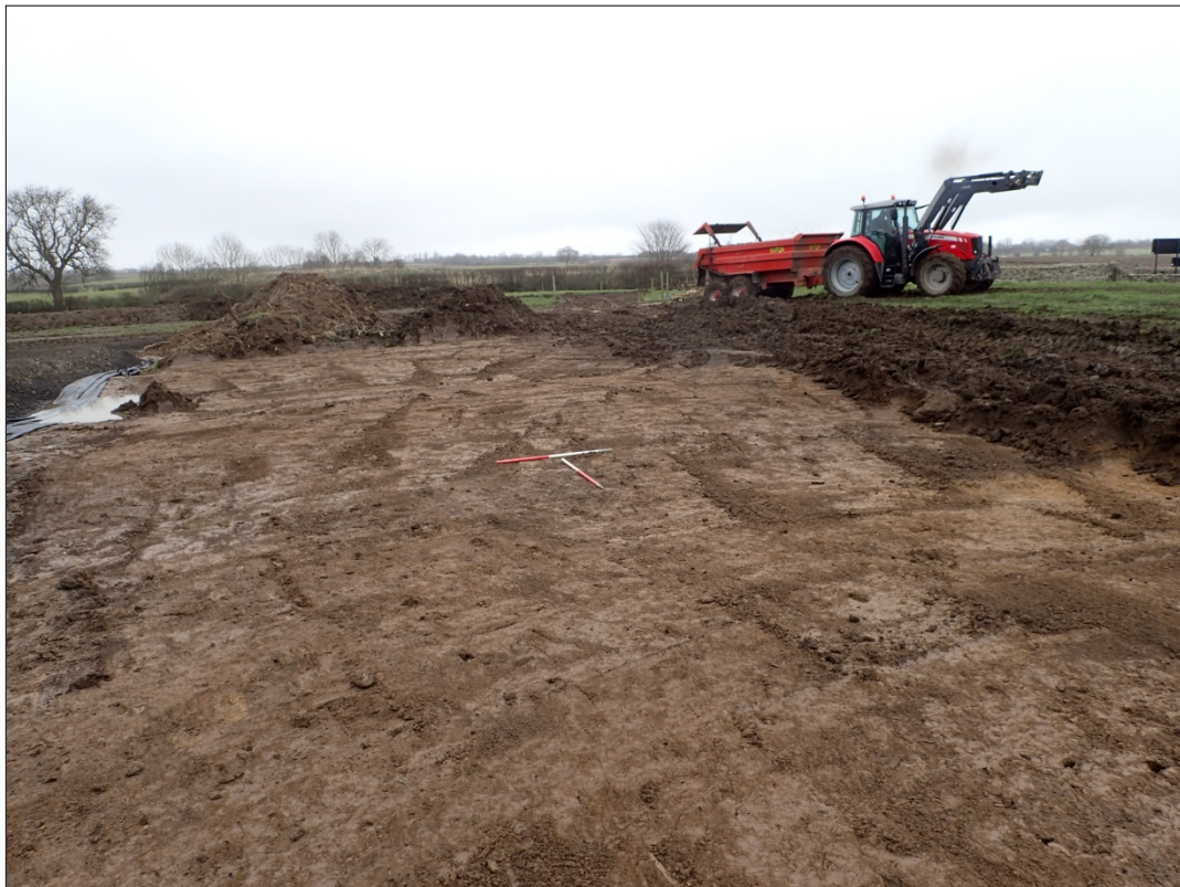
Figure 5: The eastern half of the site after excavation, looking north
