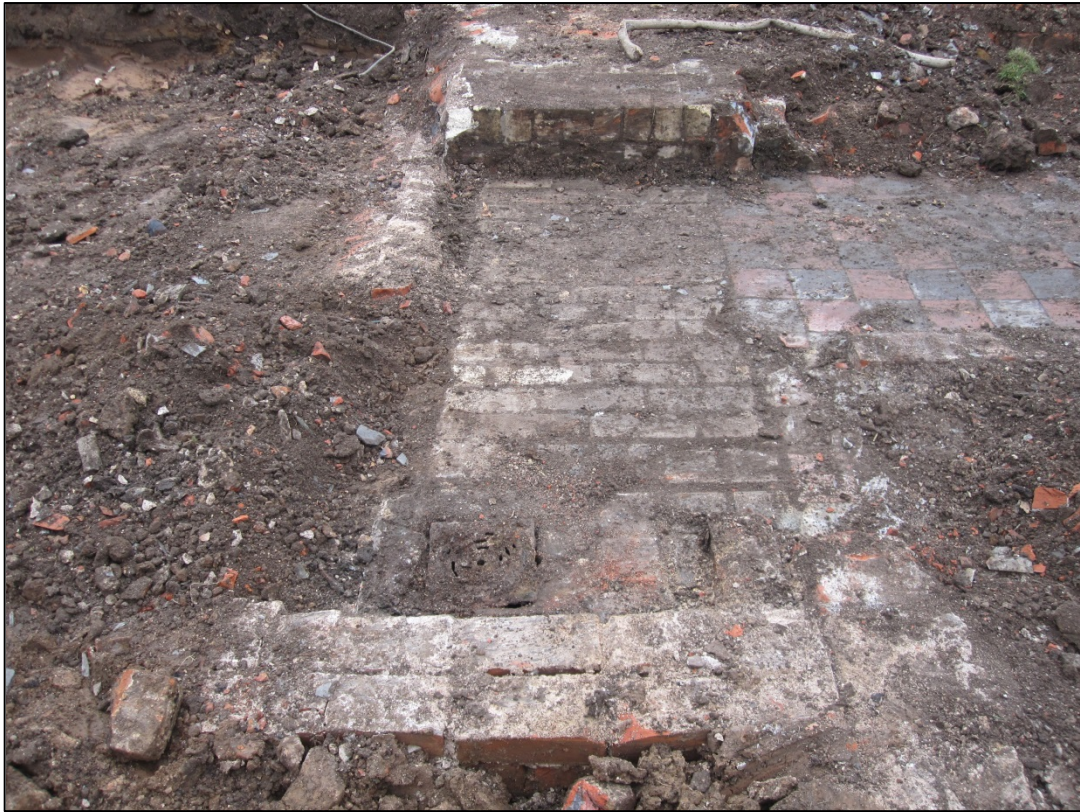
Figure 13: Brick extension at east end of west greenhouse, looking south
