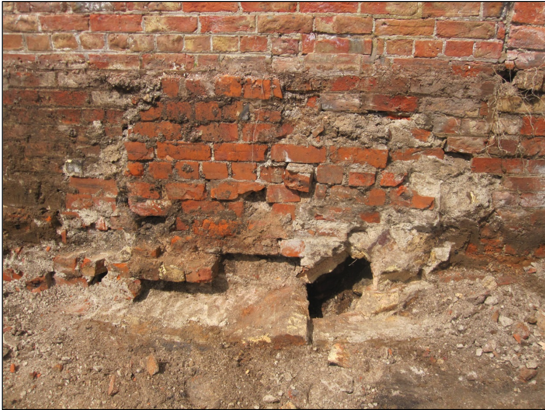
Figure 15: Heating flue F405 in annex wall, looking north
