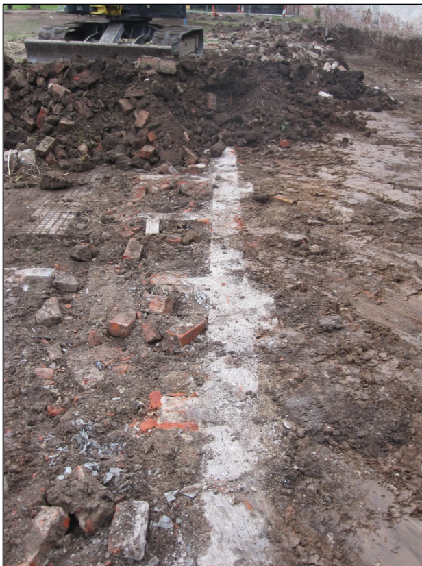
Figure 8: Wall foundation F408, looking west
