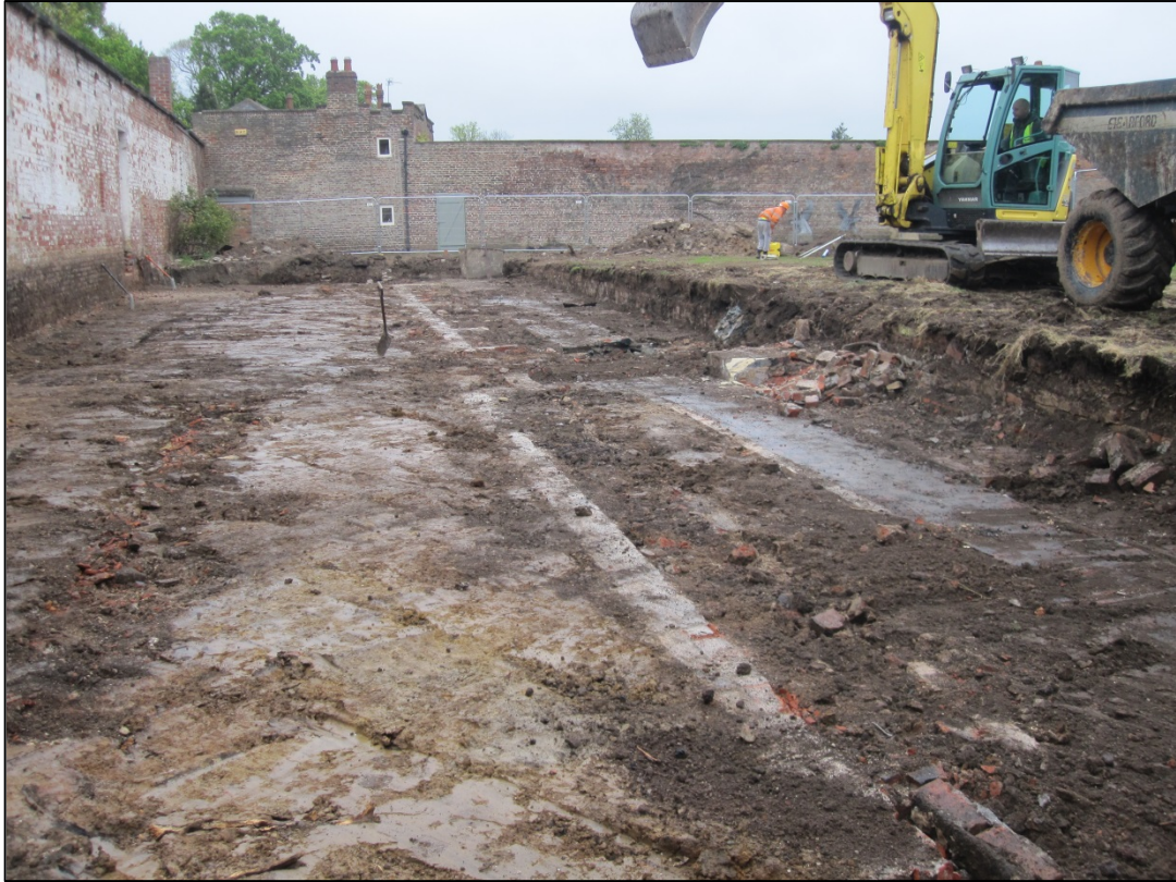
Figure 11: Western greenhouse with eastern one behind, looking east
