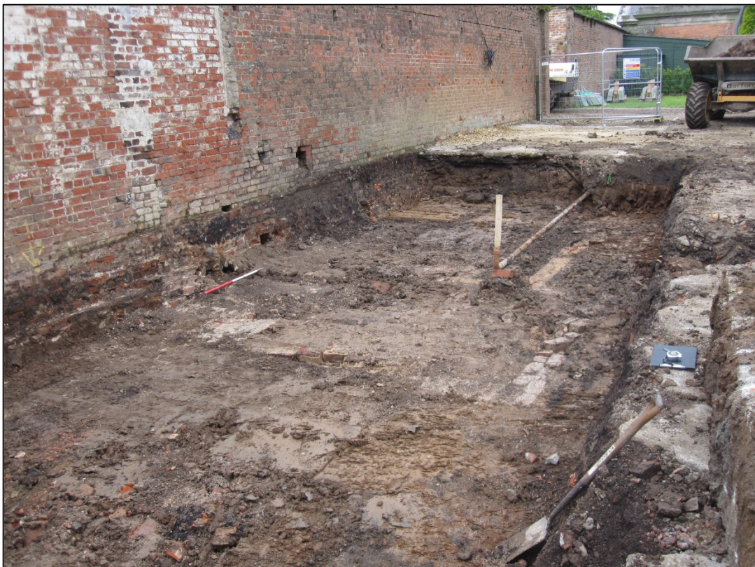
Figure 16: Cellar F512 for heating boiler, looking south-west
