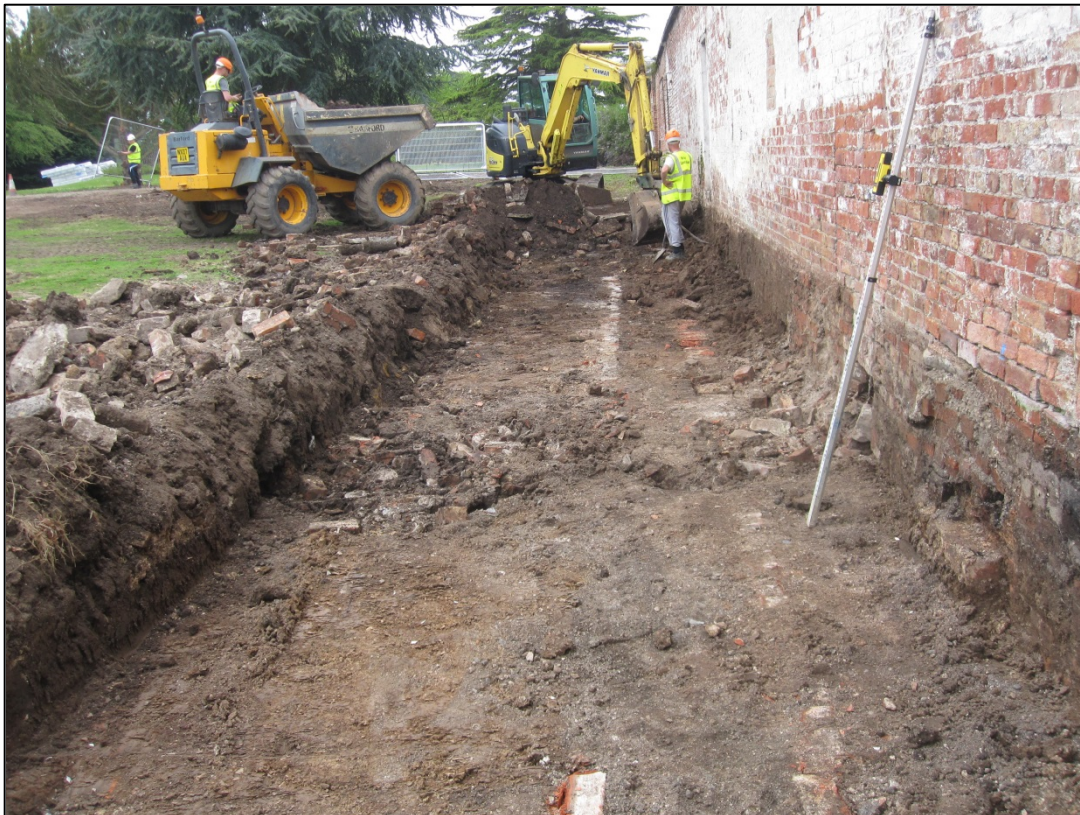
Figure 14: Parallel walls lining pipe duct 404, looking west
