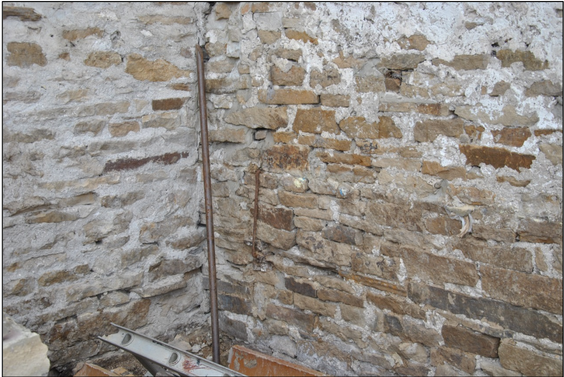
Photograph 25: An iron tethering staple (centre) attached to the internal wall, near the north corner of the southern room
