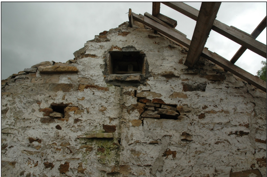
Photograph 26: The pigeon holes seen from inside the south room, with two rough recesses below
