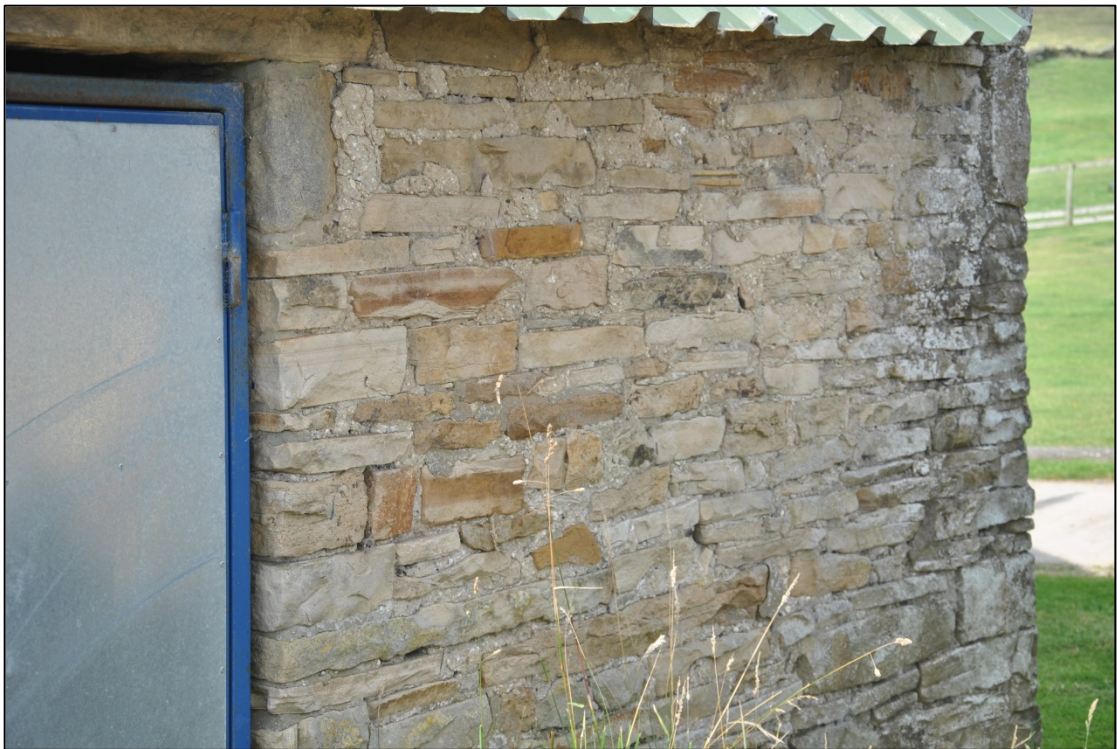
Photograph 10: The modern masonry beside the door is a good match for the greyer old stonework at the corner of the wall
