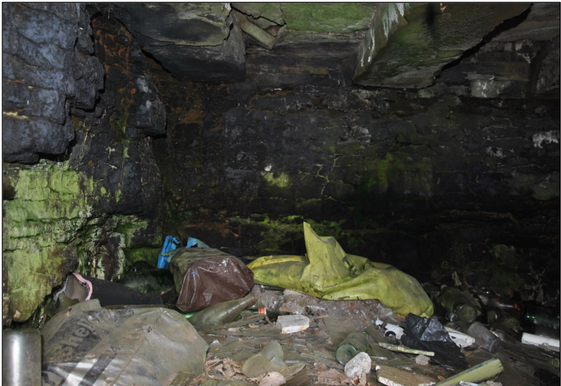
Photograph 16: The interior of the under-floor room, with what appears to be a natural stone outcrop on the left. A view looking north-east
