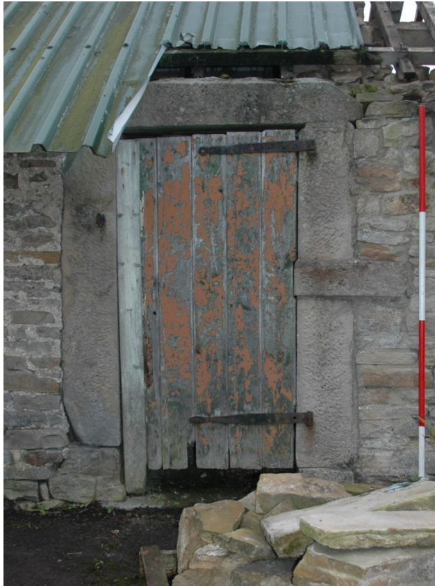
Photograph 19: Detail of the door near the middle of the north-west face
