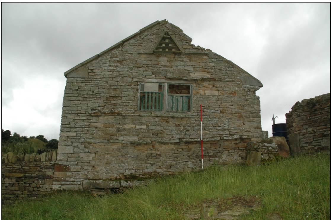
Photograph 12: The tall south-west end wall. The window is a recent insertion
