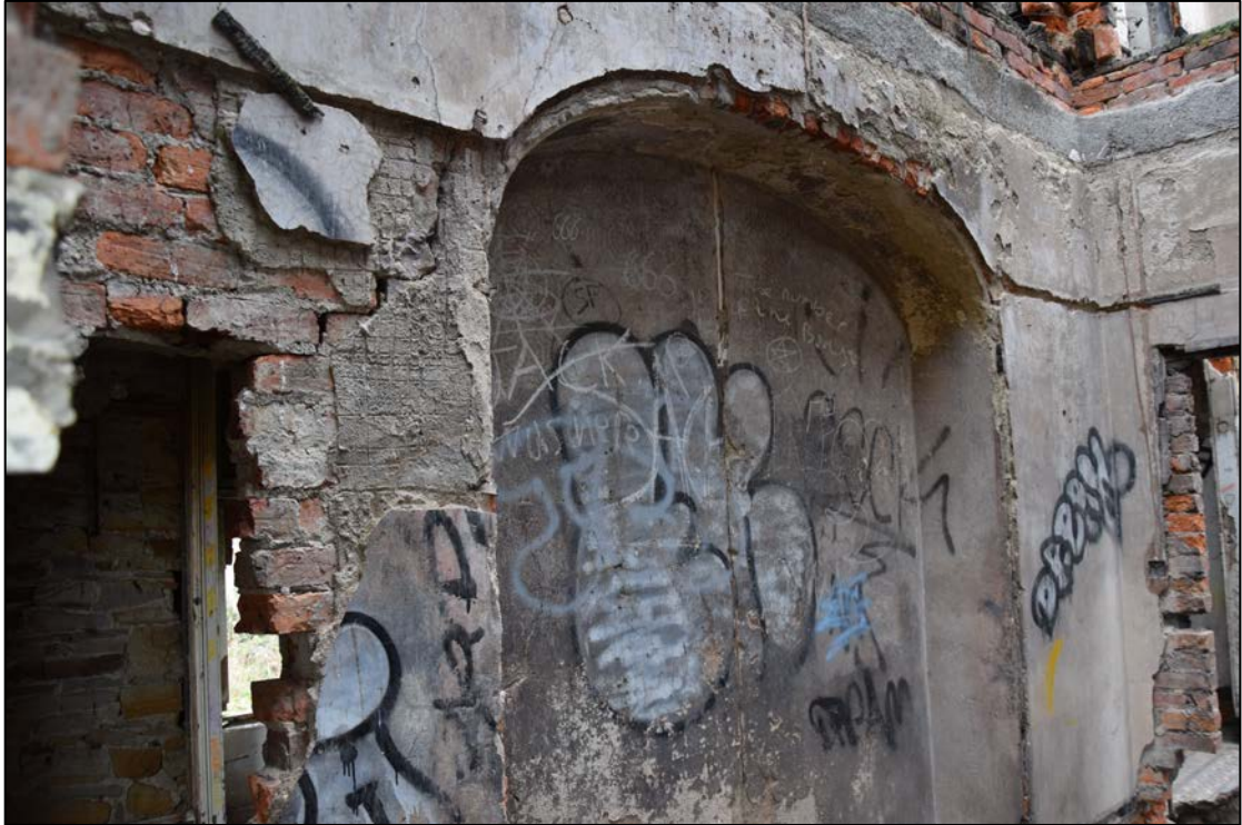
Photograph 13: Recess in the north wall of the large south-west reception room
