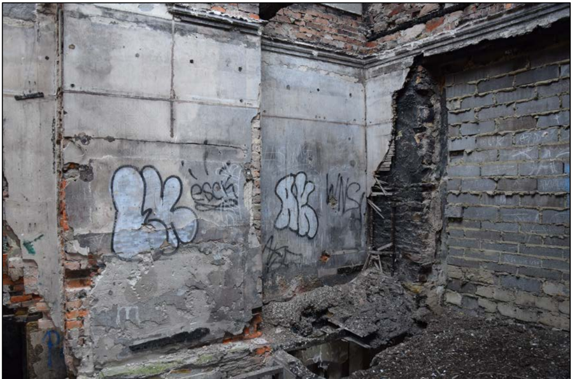
Photograph 14: The south and east wall of the room shown above. The blocked window fills most of the wall on the garden side
