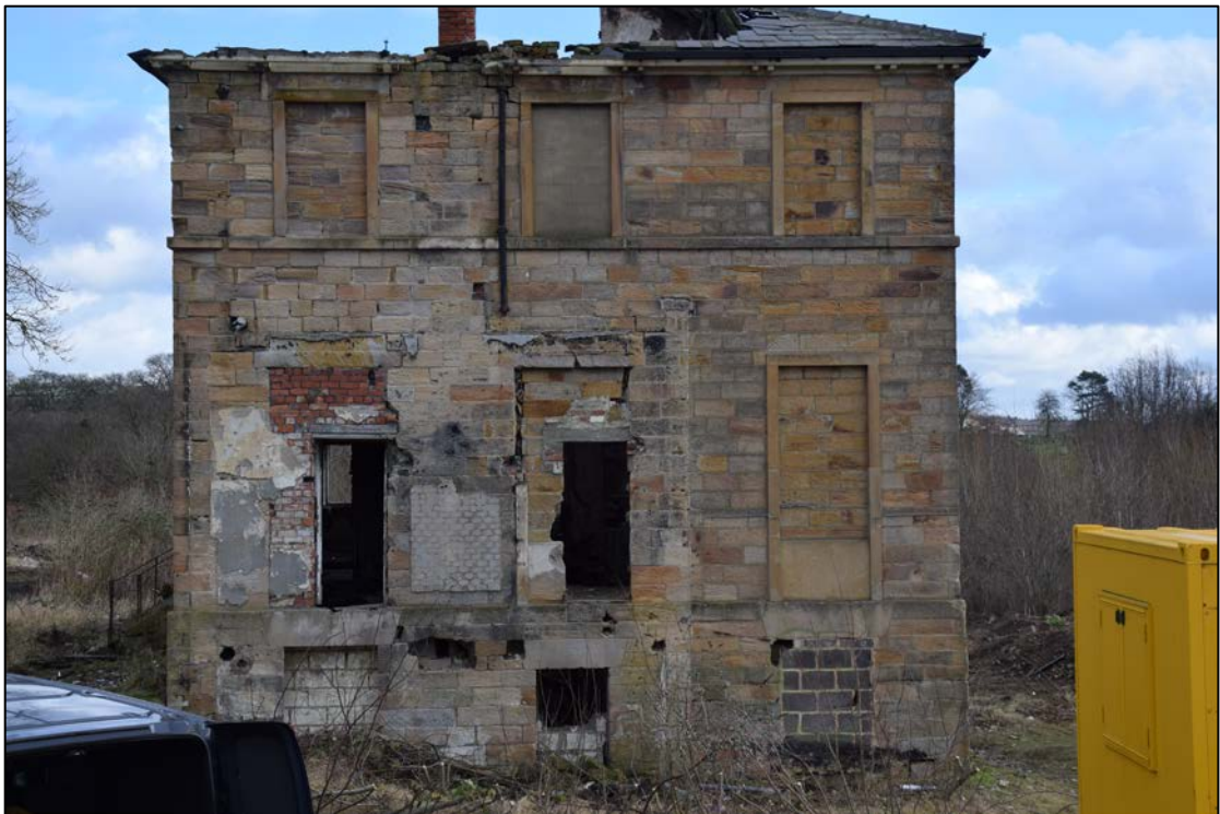
Photograph 8: The east face shows the marks of its connection with the 20th-century factory building that abutted it
