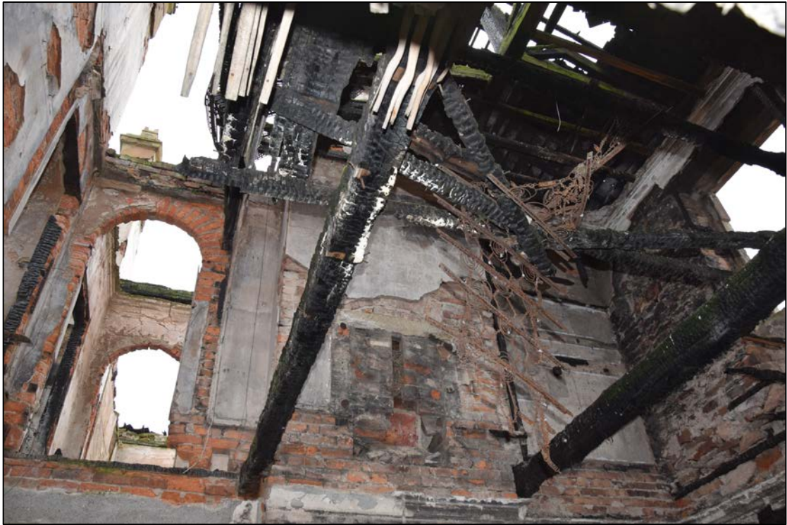
Photograph 19 (above): The south-west bedroom, seen from the floor below. A stud partition separated this room from the landing, which ran through the brick arches on either side of the staircase (left)
