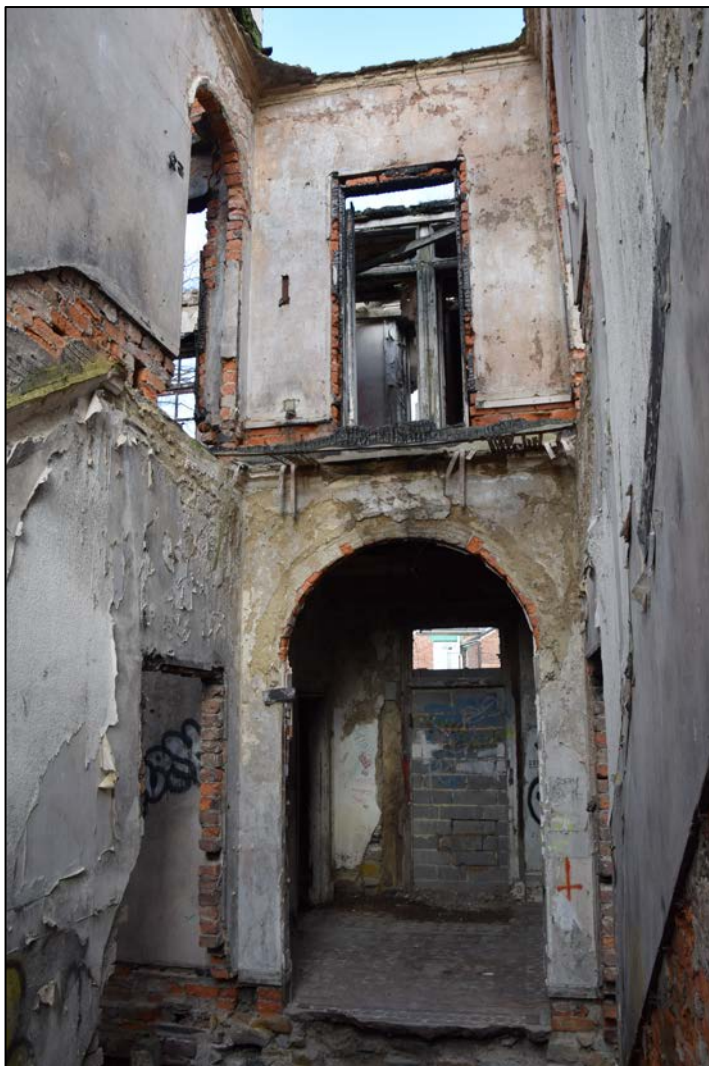
Photograph 19 (above): The south-west bedroom, seen from the floor below. A stud partition separated this room from the landing, which ran through the brick arches on either side of the staircase (left)
