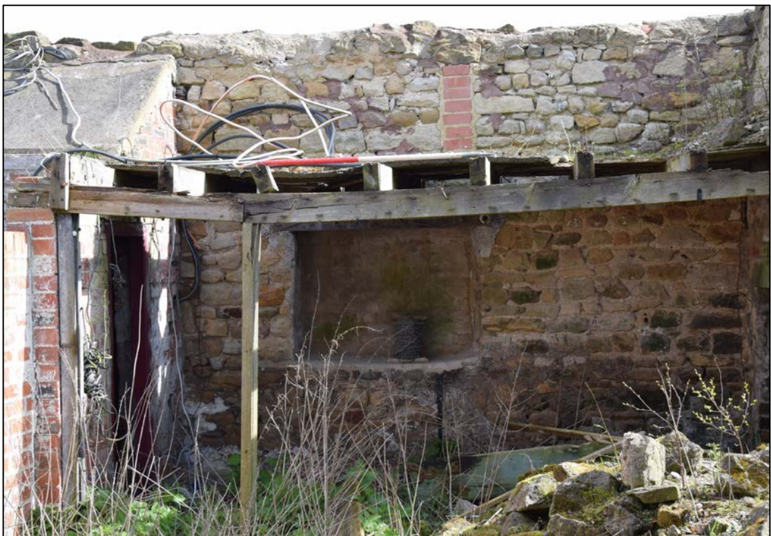
Photograph 32: The back wall of building 13, showing the door to the shed 12, a blocked window and a breather slit, and the remains of the low floor
