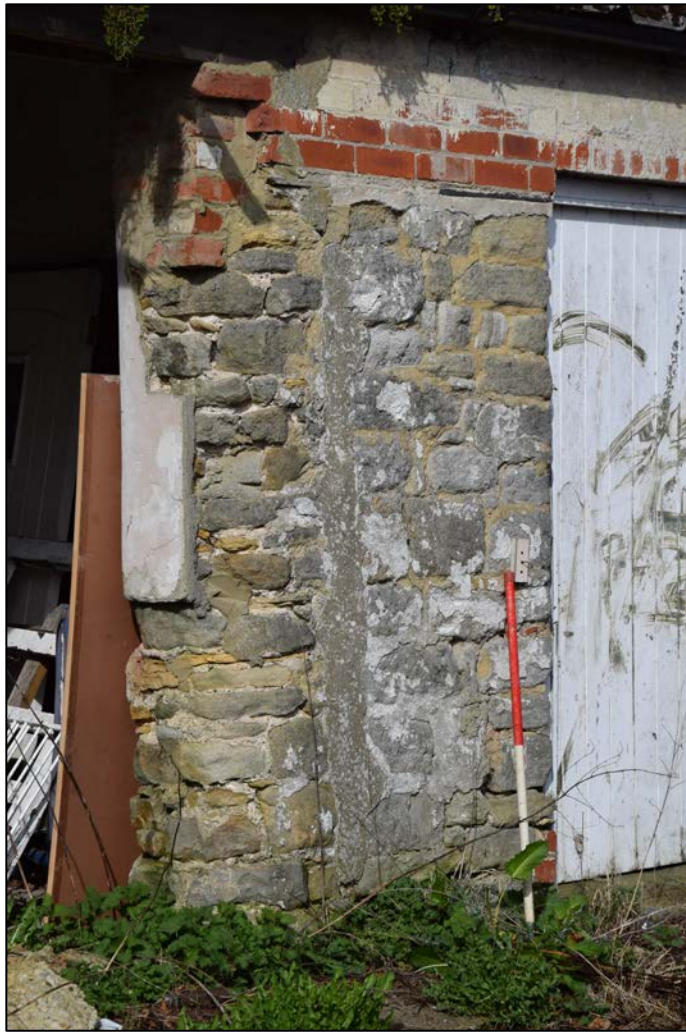
Photograph 49 (left): A cylindrical stone pier incorporated into the stone wall in the east face of building 7
