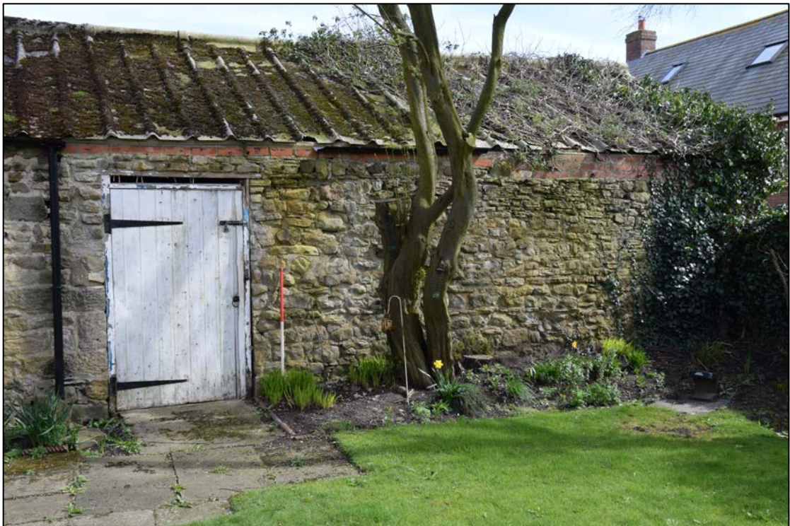
Photograph 44: Smaller, more roughly coursed rubblestone forms the west wall of building 7
