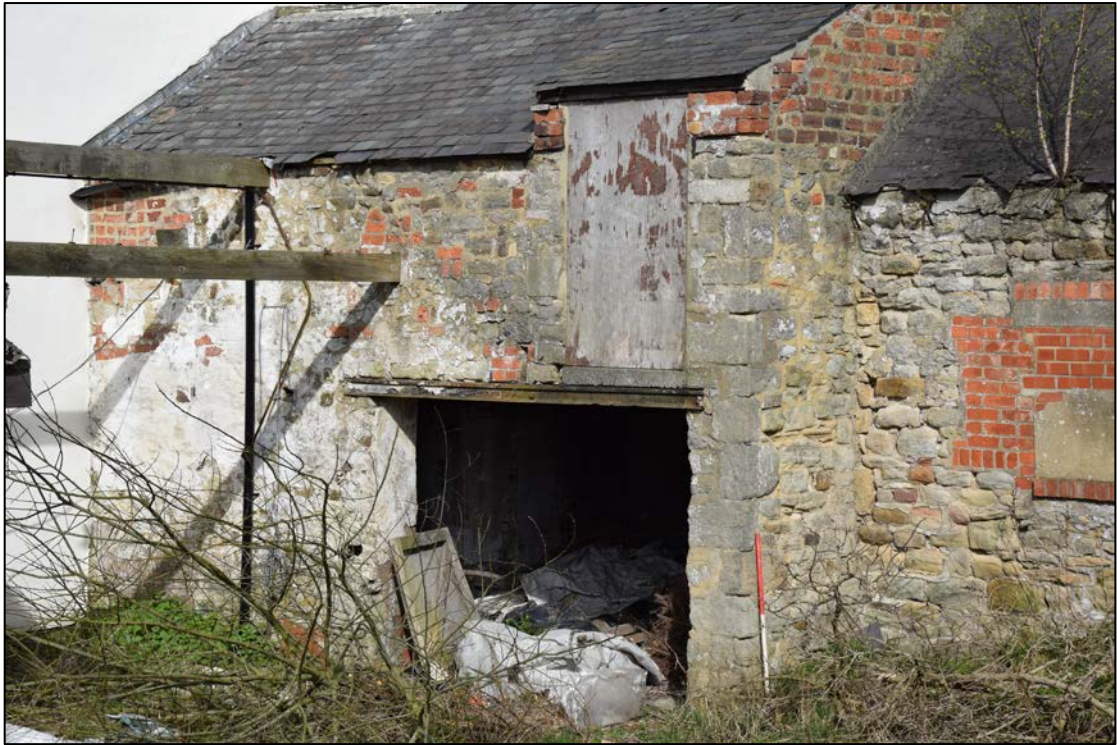
Photograph 9: The south face of building 1. Later brickwork, top right, accommodates the lower-pitched roof above an inserted loading door. The large horizontal timbers are the purlins of the vanished building 4
