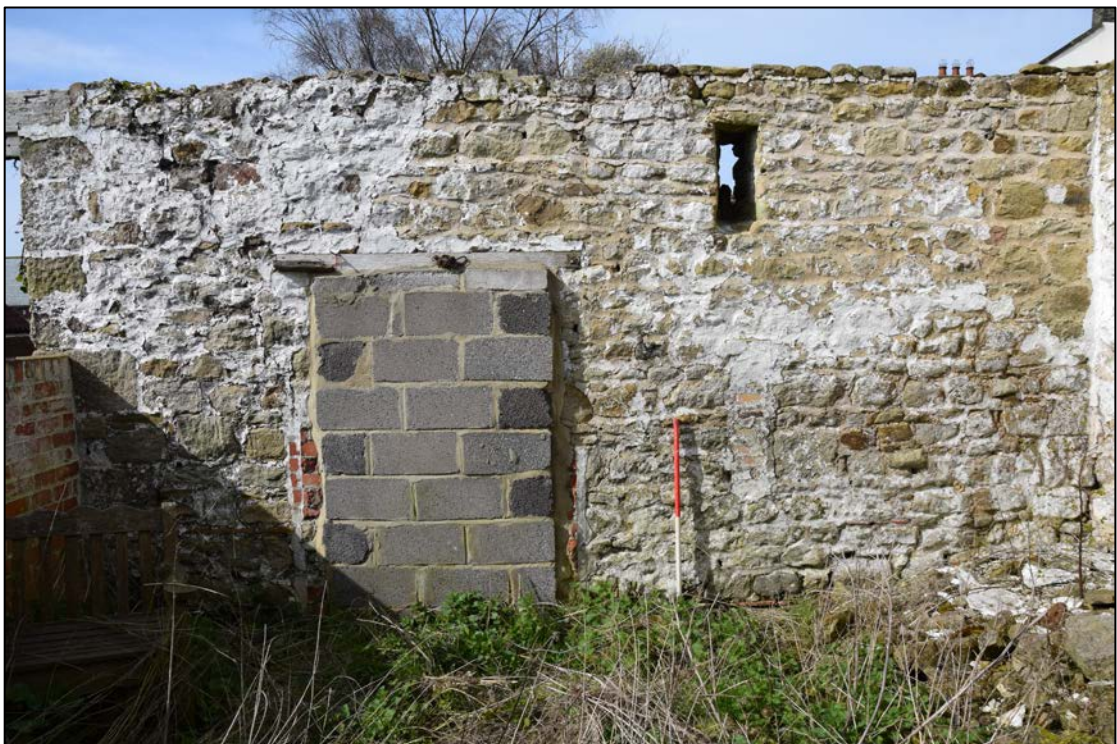
Photograph 28: The inside of the west wall of the old barn, building 11. Note the blocked breather below the open example, and the large quoins beside the door at the extreme left
