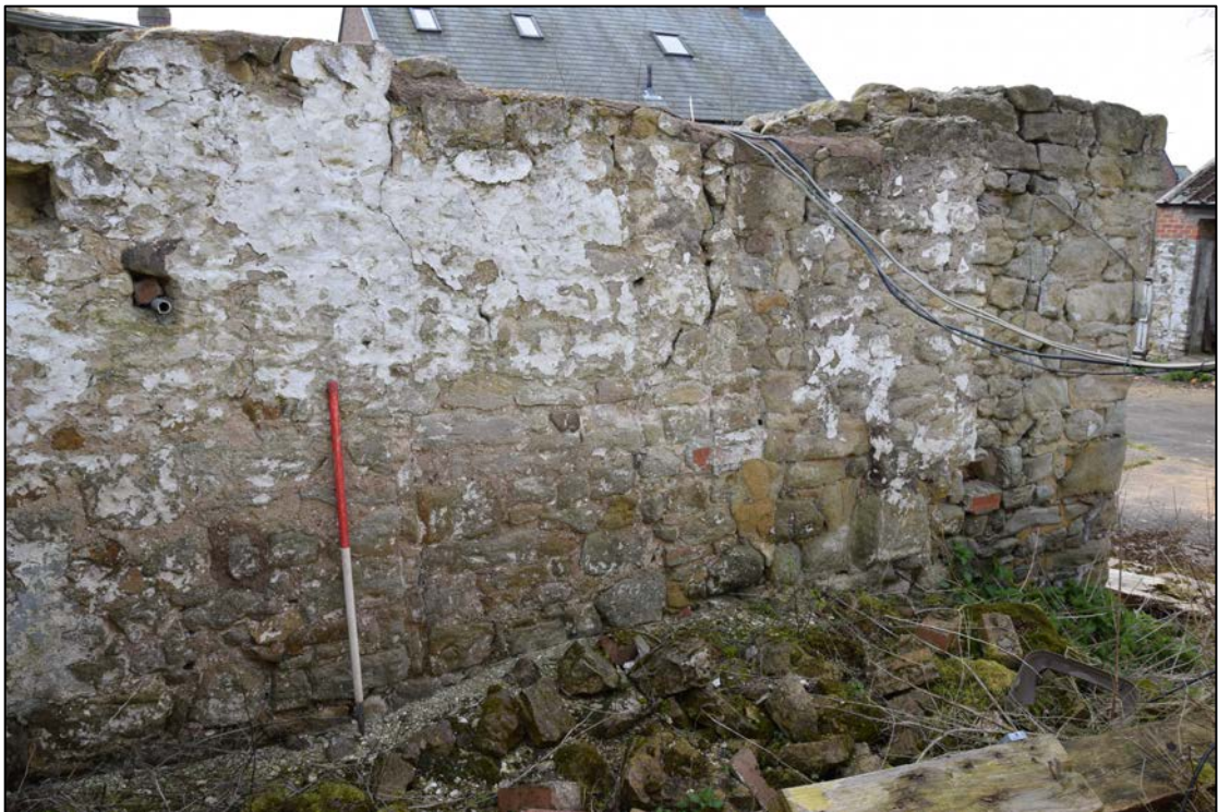
Photograph 26: The north end of building 11 seen from building 10. A blocked opening can be seen beside the scale
