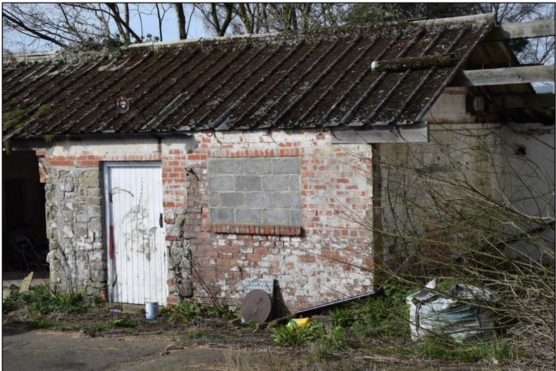
Photograph 40: Building 4, at the right side of this view, is now represented only by its roof purlins and door lintel. Building 5 is the brick structure at the centre and 6 is the passage entered by the white door
