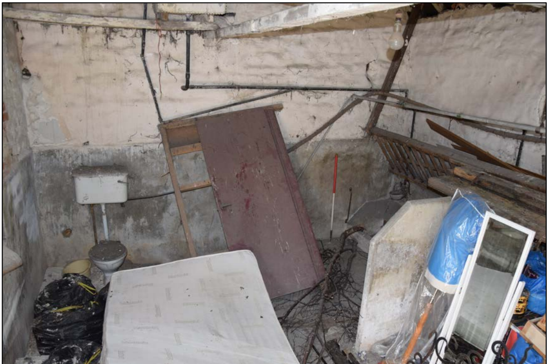
Photograph 16: The interior of building 2. The 20th-century render rises to about 1.3m above the floor and above this the masonry is whitewashed. Part of the trough and hay rack can be seen near the scale
