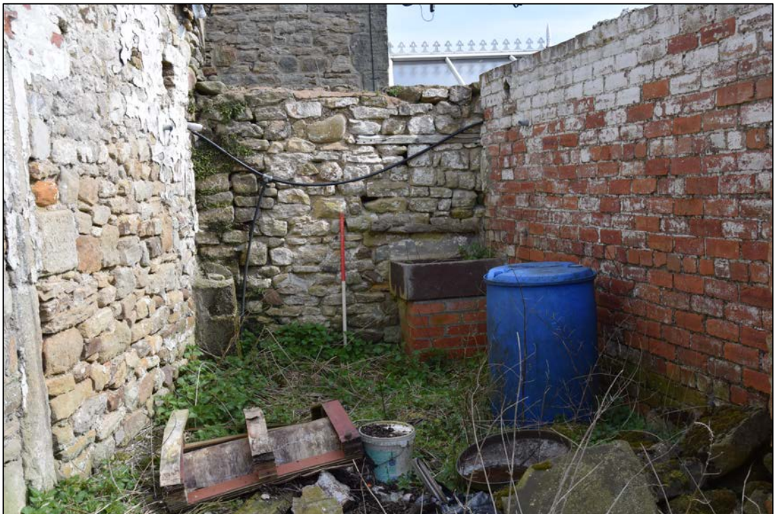
Photograph 22: The stone wall at the back of building 8 is part of an older shed. A blocked window can be seen above the brown ceramic trough
