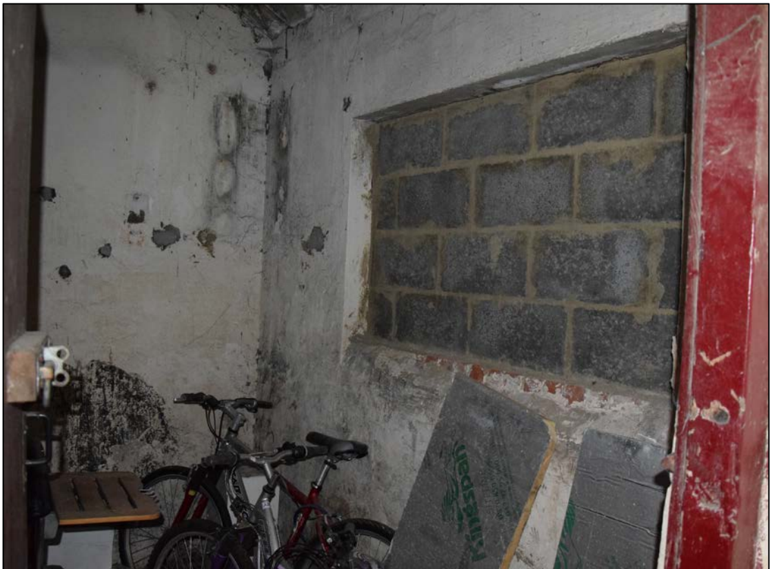
Photograph 46: The large blocked window at the east end of building 5
