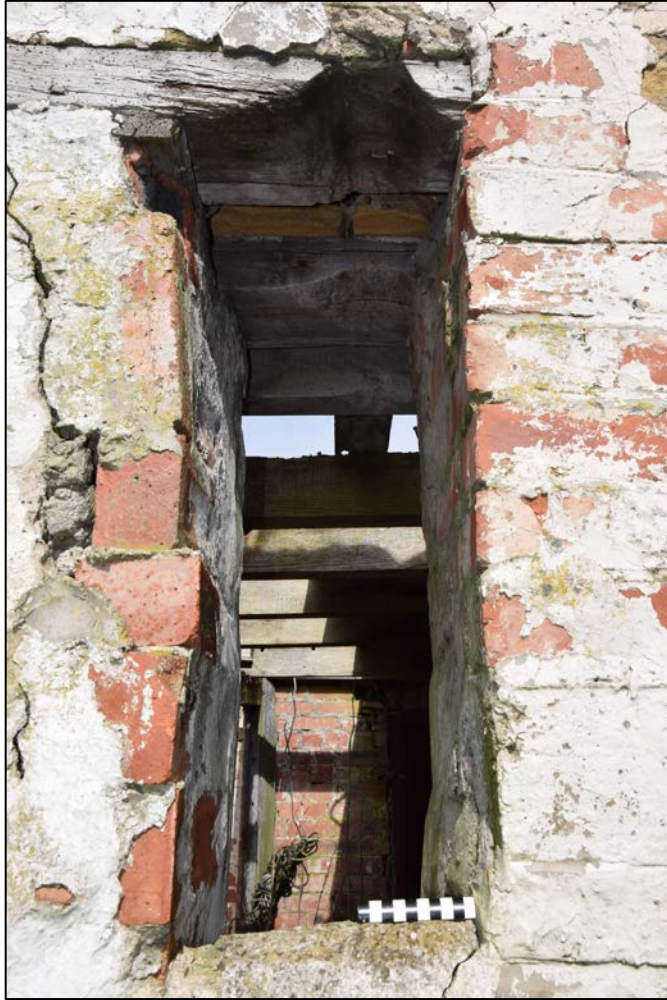
Photograph 35 (left): The timbers at the head of the belt slot have been cut away to increase clearance. A view looking north
