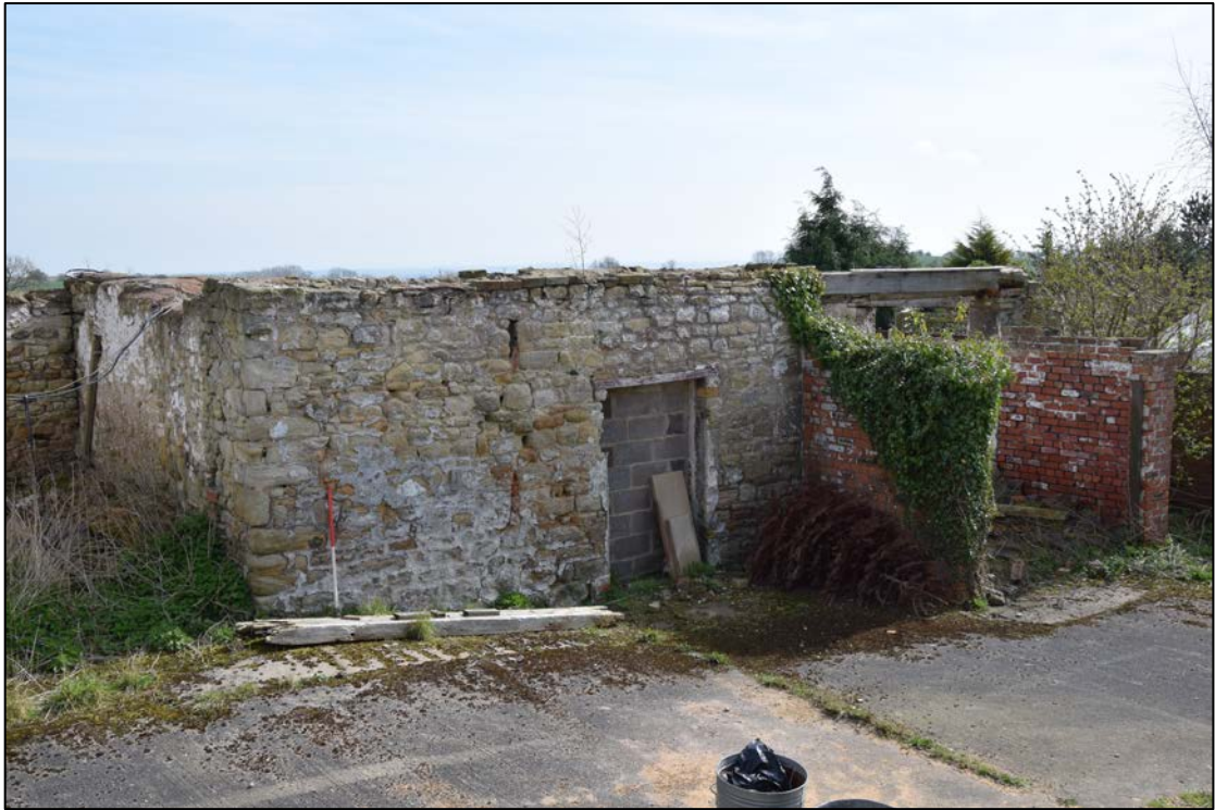
Photograph 25: Building 11/12/13, showing the brick porch added before 1920
