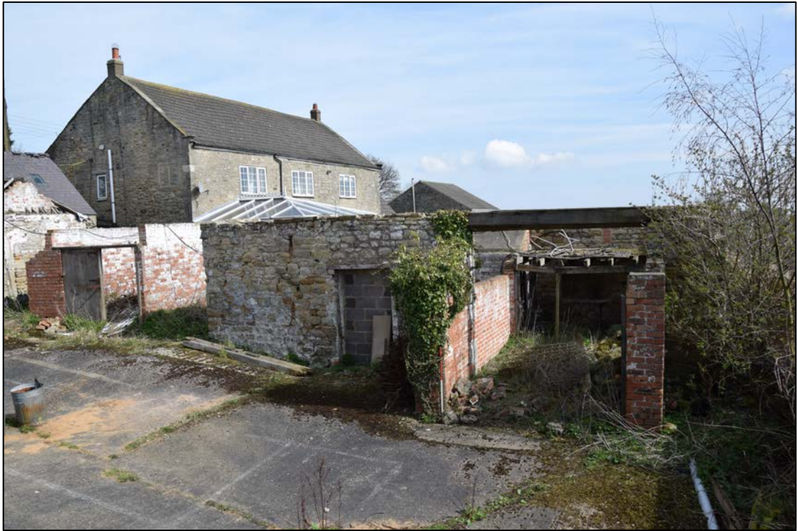
Photograph 7: The buildings of the east range. Note the blocked old window in the wall of the house beyond the yard
