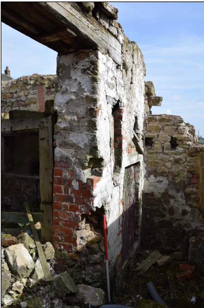
Photograph 37 (above): The south-west corner of building 13, showing the ragged masonry that faces the dressed stone shown in the previous picture
