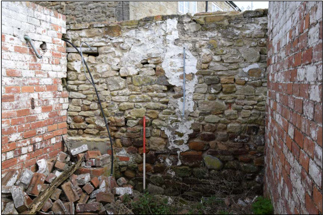
Photograph 23: Building 9, showing the middle of the old shed's back wall. A trough like that shown above stood in the left-hand corner. Above this, note the timber lintel seen in Photograph 22 emerging from behind the brick wall
