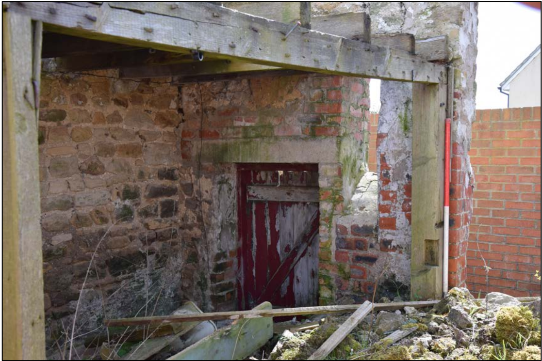
Photograph 33 (above): The door and the belt slot at the south-east corner of building 13
