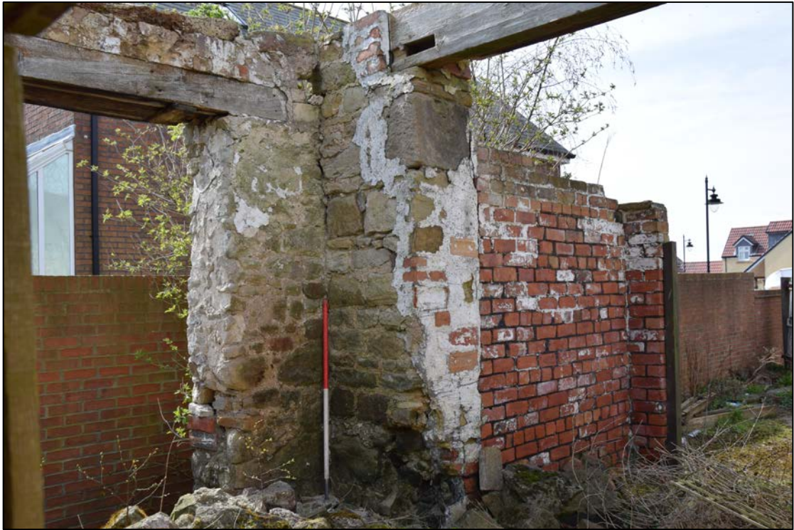
Photograph 37 (above): The south-west corner of building 13, showing the ragged masonry that faces the dressed stone shown in the previous picture
