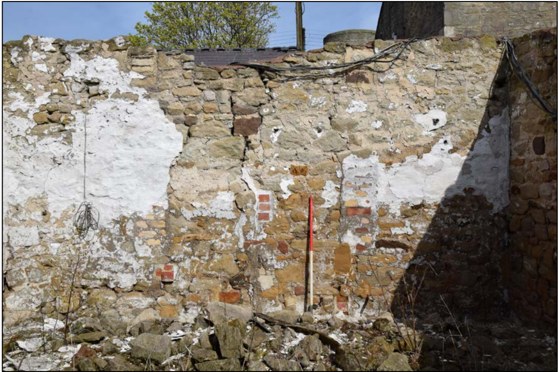
Photograph 29: The north wall in building 11, showing blocked openings
