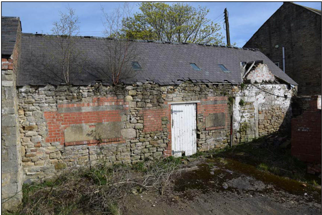
Photograph 14: The south face of building 2/3. Straight joints for a western door can be seen under the brick blocking of the left-hand window; its position mirrors that of a complete blocked door under the small gable at the right
