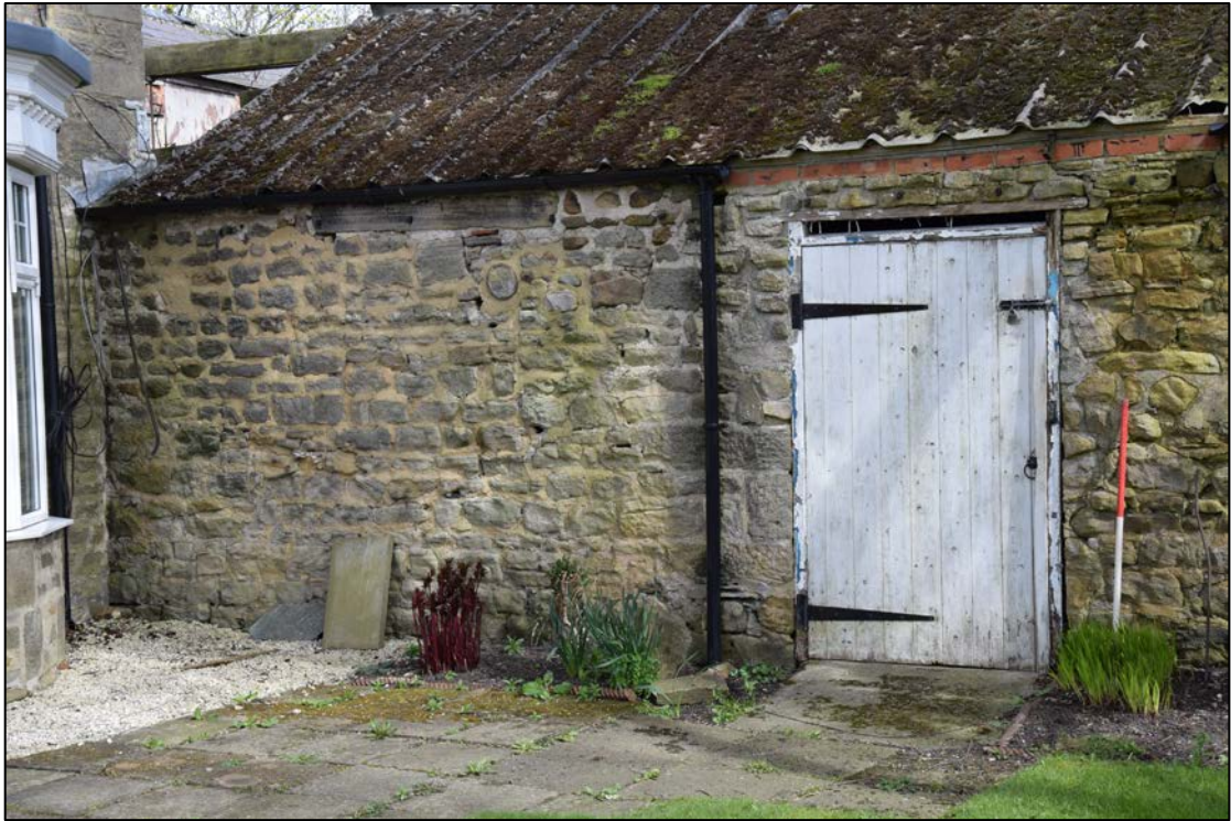
Photograph 43: Coursed rubble, a blocked window and a pipe ventilator in the west face of building 5. Note the difference between the stonework on either side of the door to building 6
