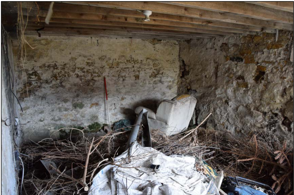
Photograph 10: Inside building 2; a view looking north-east. Note the batter in the lower part of the right-hand wall, which is the west end of building 2/3
