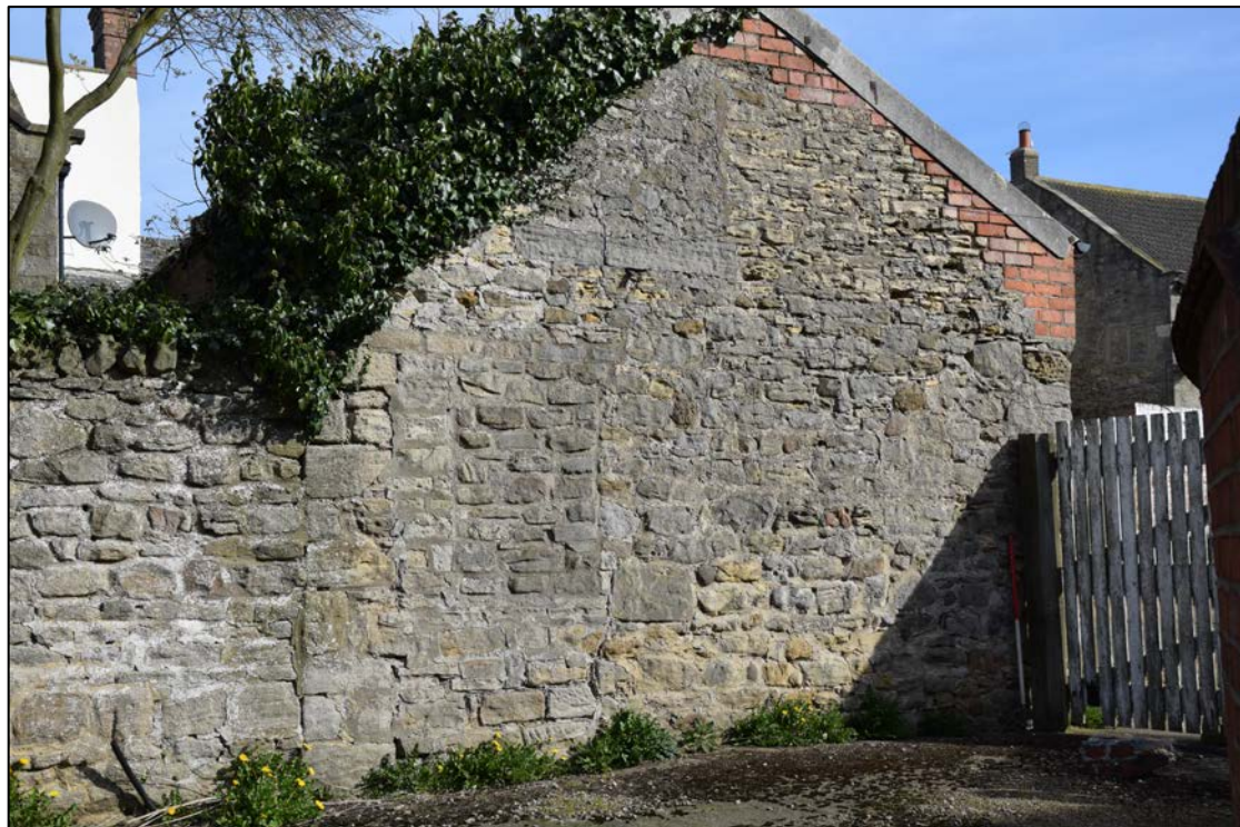
Photograph 50 (below): The south end of building 7 has blocked windows at two levels, left of centre. The roof line appears to have been raised at the east side, where brickwork has been added
