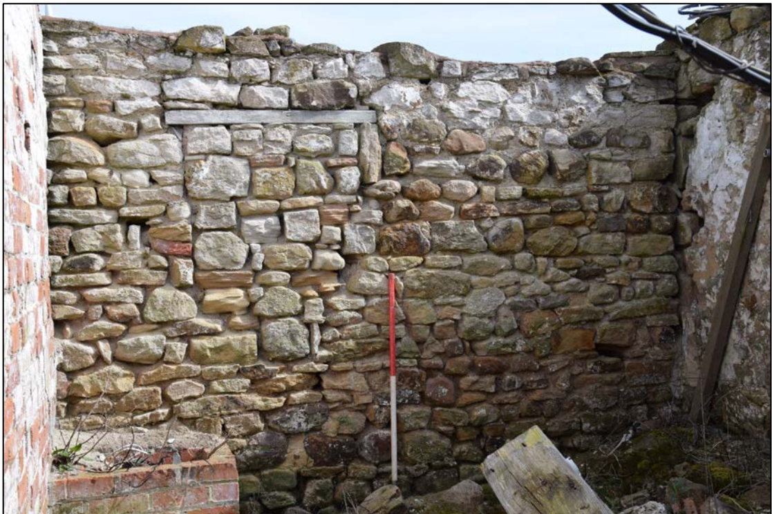
Photograph 24: Another blocked window in the back wall of building 10
