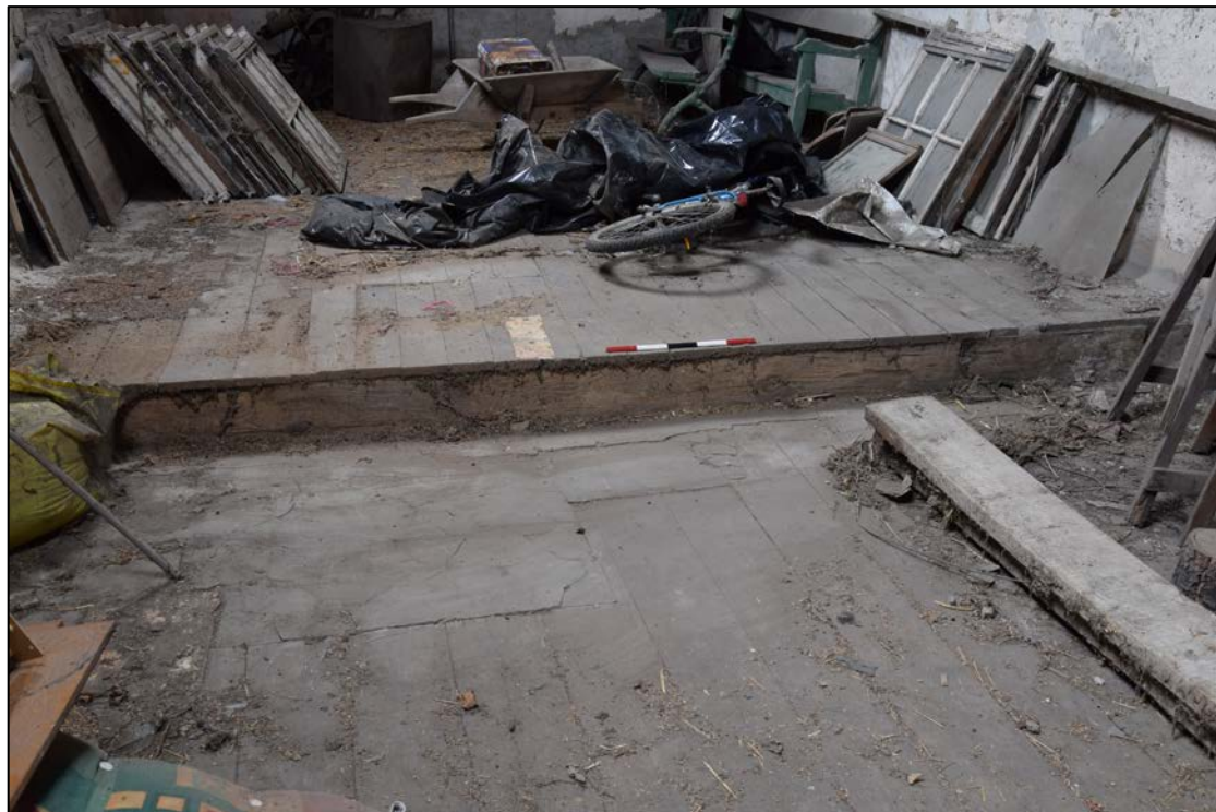
Photograph 30 (below): Detail of the step in the floor at the old internal wall. The area of mortar below the step at the left marks the cut-down chimney for the fireplace in the eastern room. The row of short floor boards just above the step fill the gap left by the removal of the old staircase
