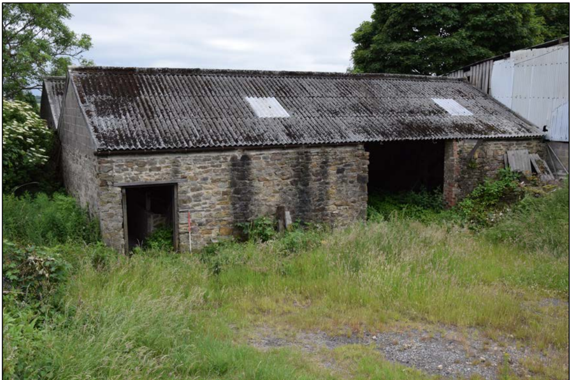
Photograph 6: The north face of the hemmel, building D
