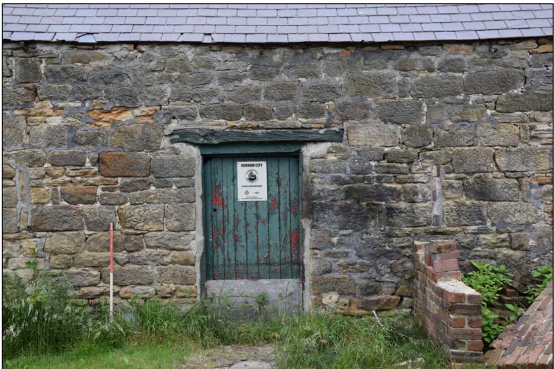
Photograph 52: The west door is set in large masonry. The brick piers at the right once supported a diesel tank
