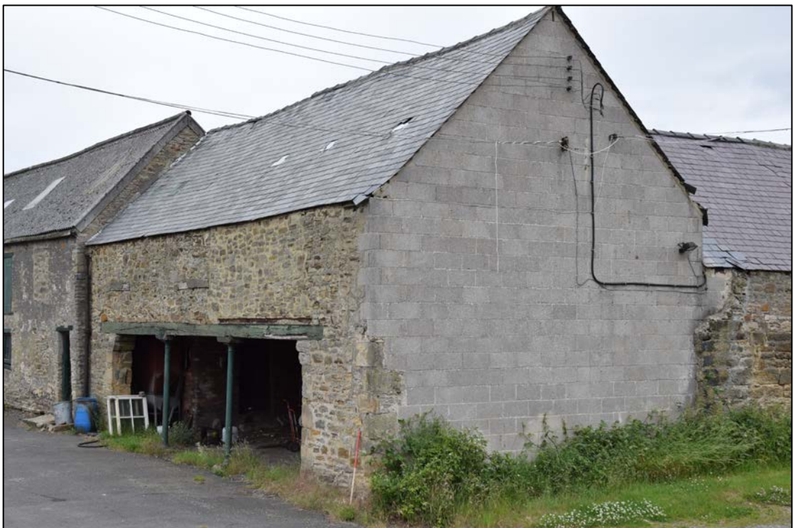
Photograph 38: The rebuilt east end of building B
