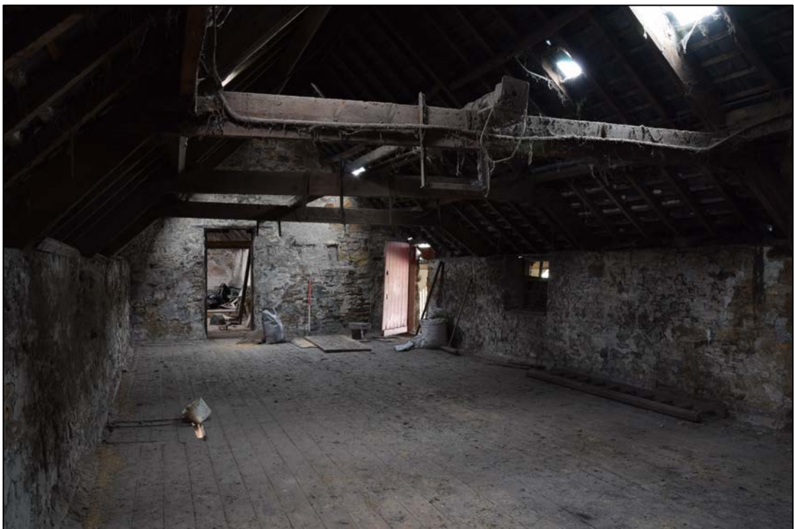
Photograph 48: Interior of the granary, seen from the south-east corner
