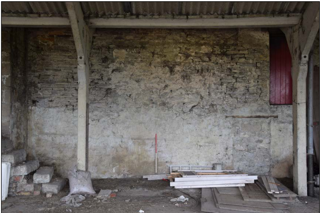
Photograph 10: North face of the old house; the east end, inside building G. The higher floor level in the modern building makes the blocked door (right) look very low. Note the offset in the face left of the first-floor door
