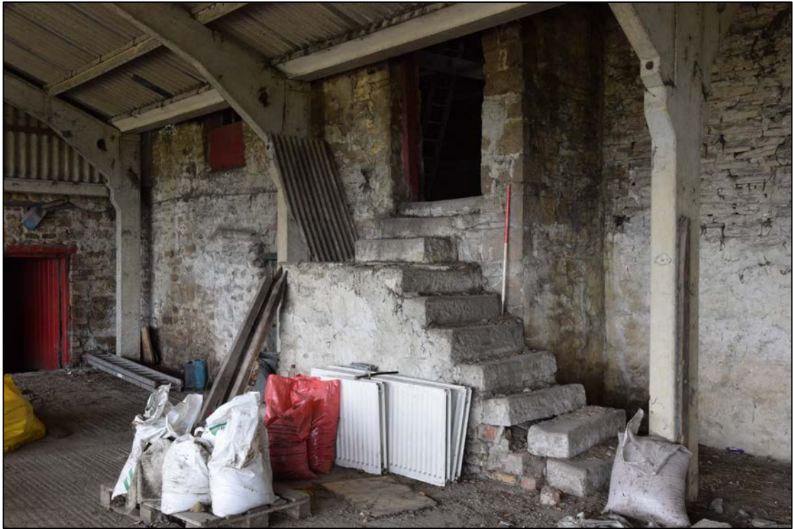
Photograph 39: The north-west corner of building B seen from inside the covered yard G
