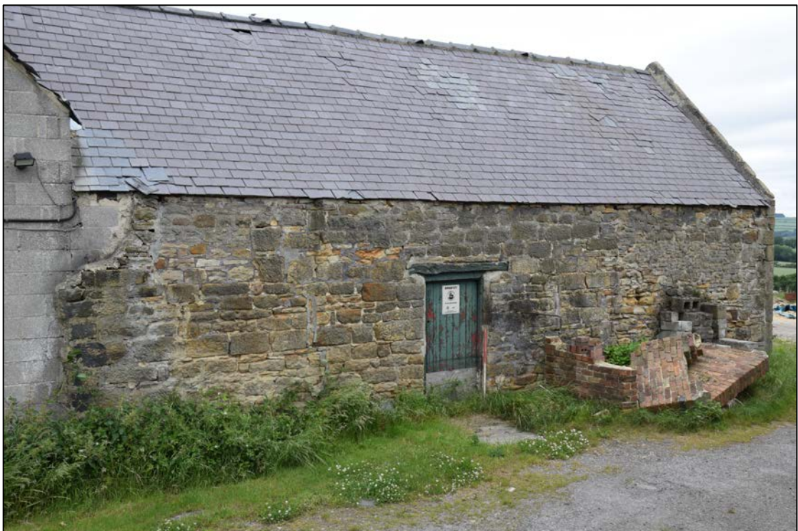
Photograph 50: East face of the threshing barn, building C
