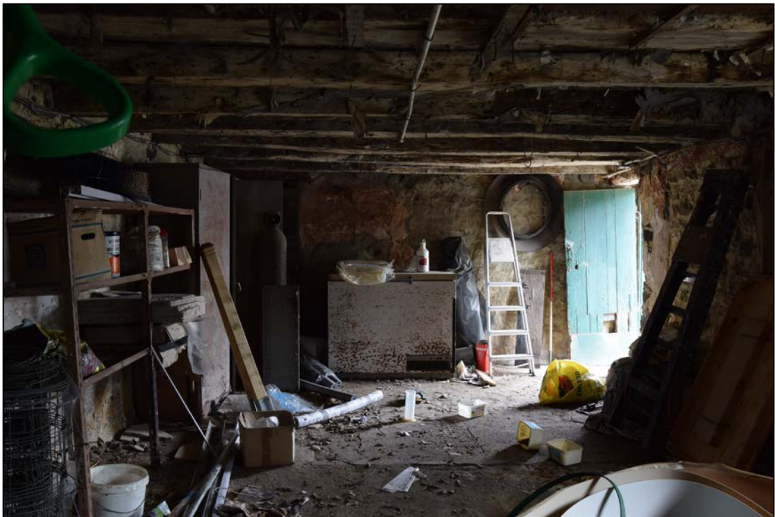
Photograph 24: A view looking east in the eastern room
