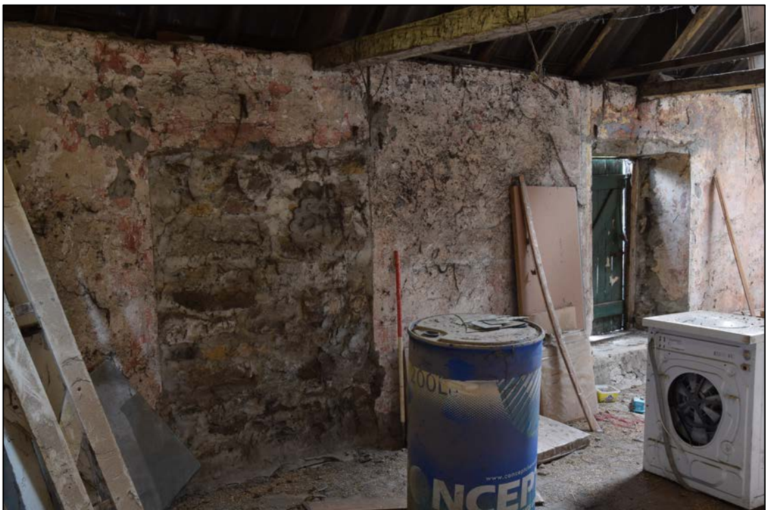
Photograph 34: The blocked east window
