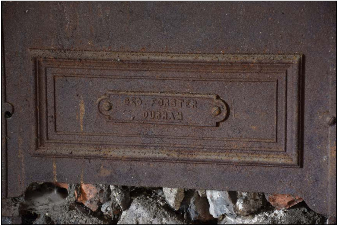
Photograph 23: Detail of the maker's plate above the blocked hearth
