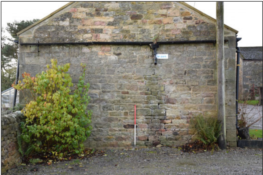
Photograph 10: Evidence of re-roofing can be seen in the re-set water table slabs on the gable. There is no trace of any building attached to this end of the structure
