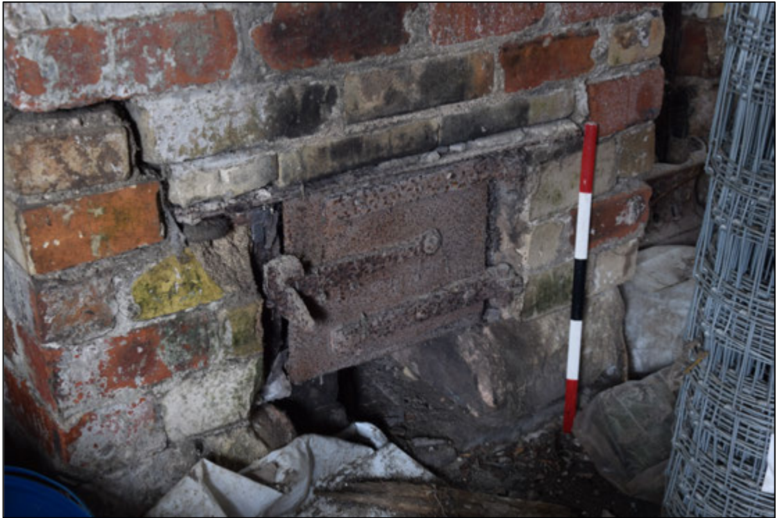
Photograph 23: Detail of the iron firebox door
