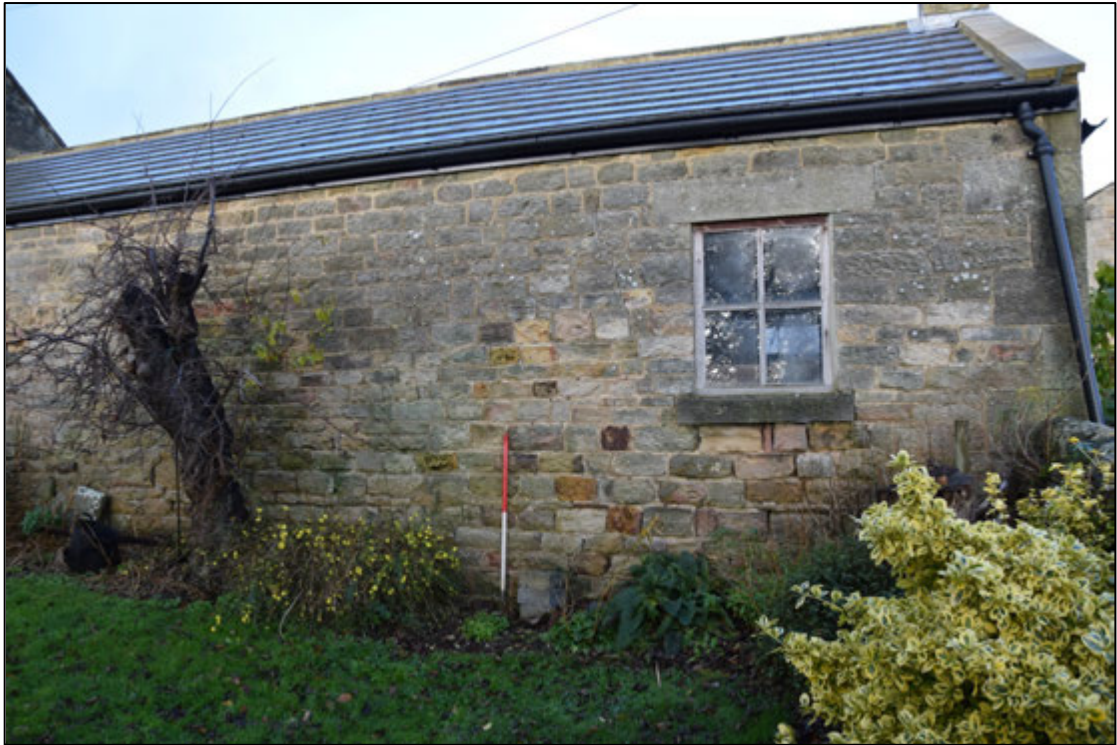
Photograph 11: Coursed masonry in the south face, with the window of the smithy
