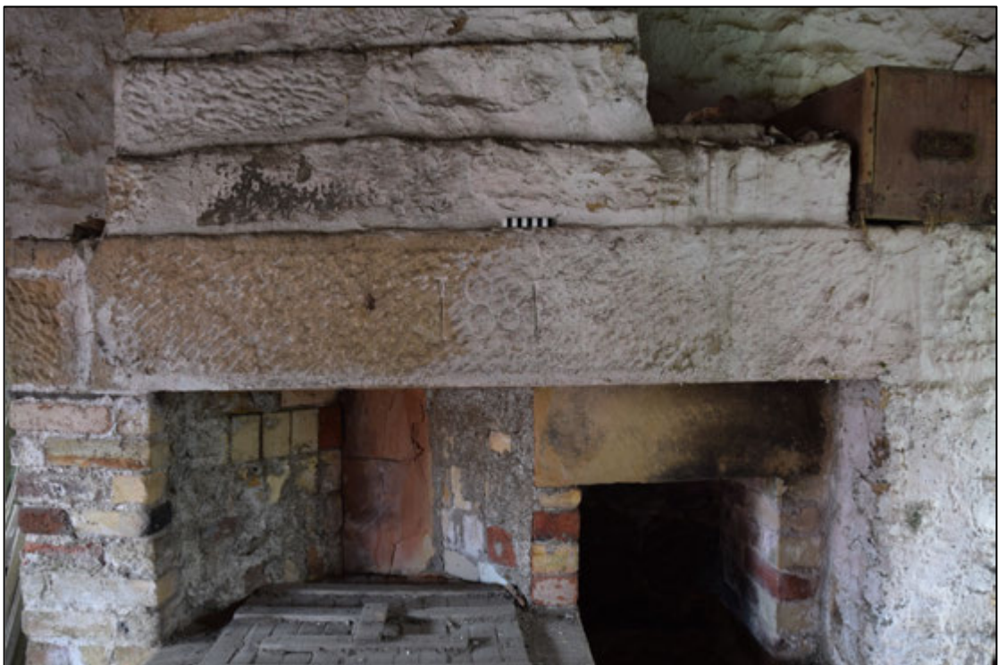
Photograph 20: The lintel of the former forge hearth, with the date 1881. Brickwork alterations, the wooden lid of the copper and the small southern hearth can be seen below
