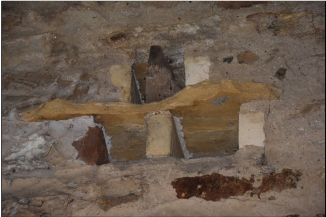
Photograph 29: Detail of the brick and sandstone pigeon holes
