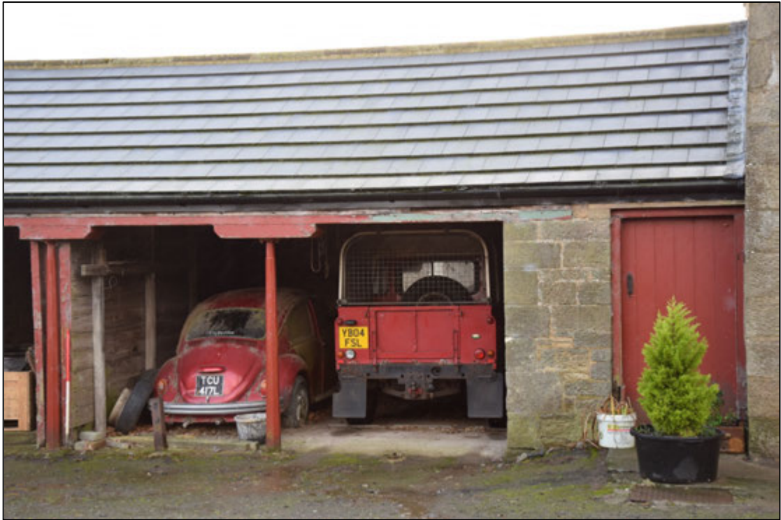
Photograph 7: Substantial masonry forms the pier between the open shed and the passage door, at the right
