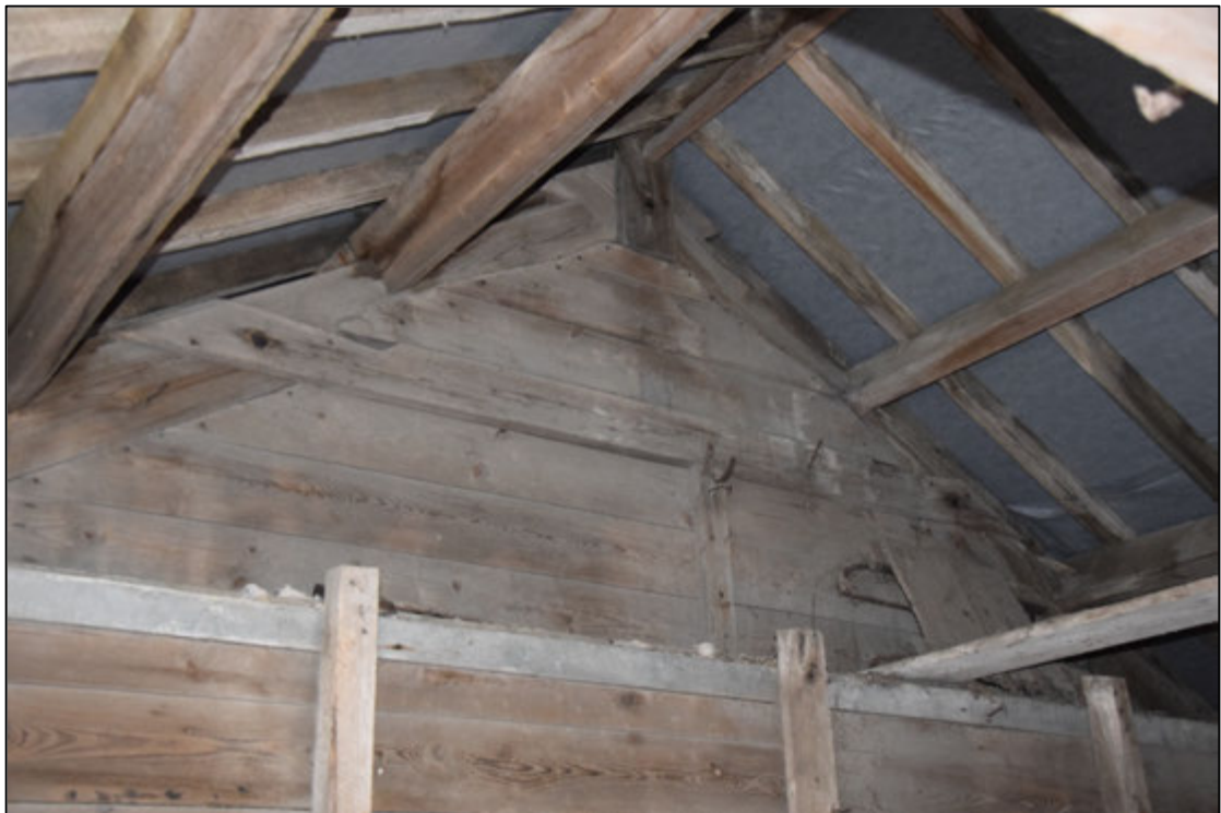
Photograph 30: The roof truss above the timber garage wall. The principal rafters and the collar beams are bolted together
