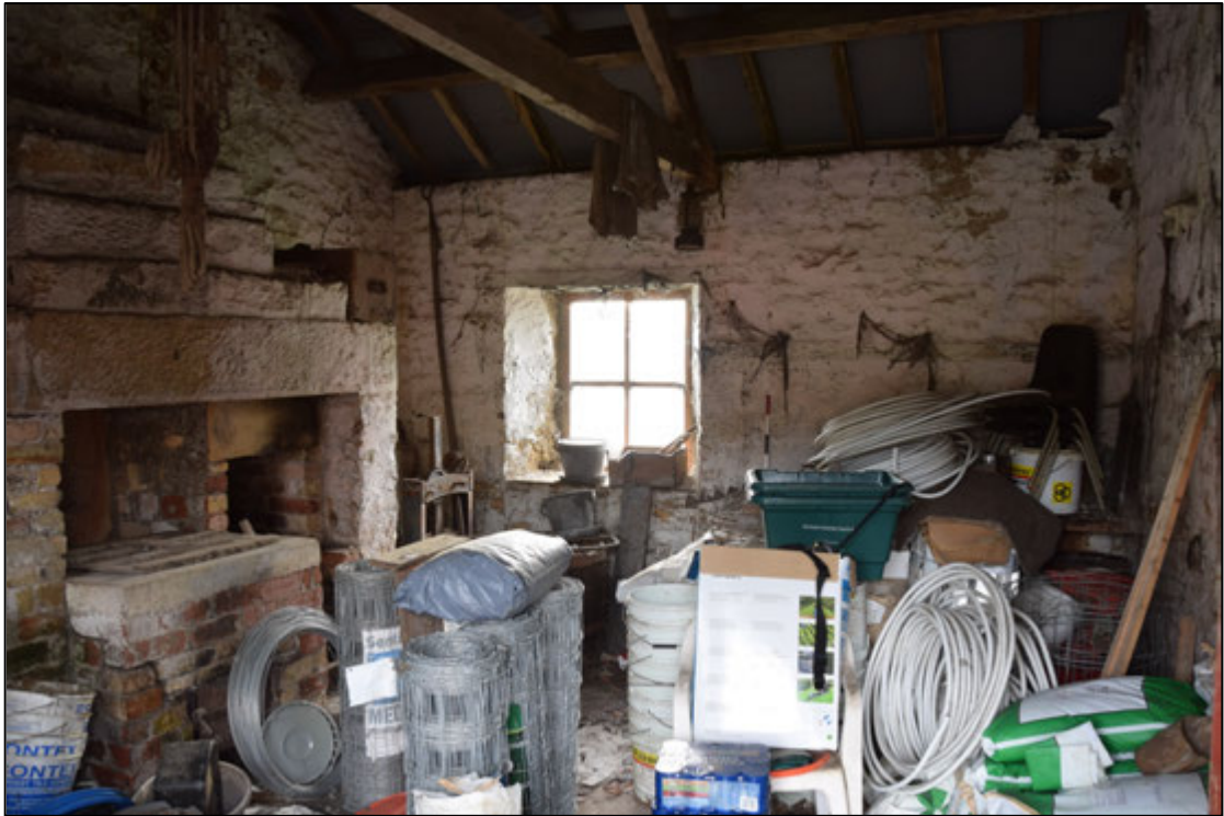
Photograph 19: The smithy / wash house seen from the doorway. Note the timbers set into the wall beside the window and at the extreme right
