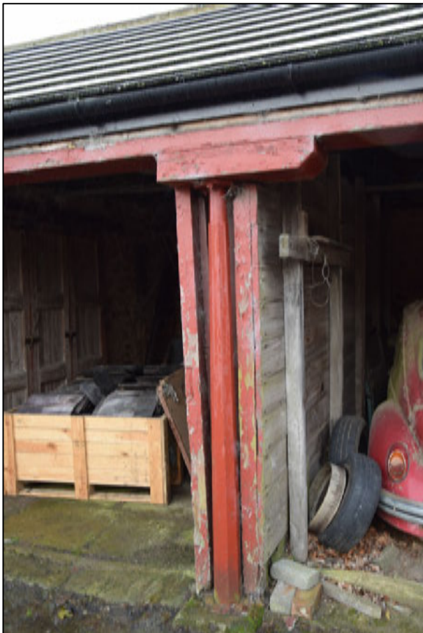
Photograph 16: The plank wall of the garage in the east bay of the shed. Note the alteration to the pad above the iron column
