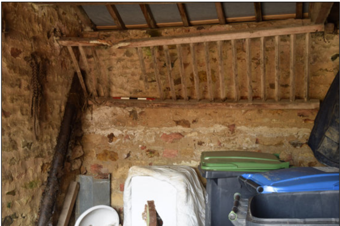
Photograph 18: A line of light grey mortar below the rack marks the position of a vanished manger
