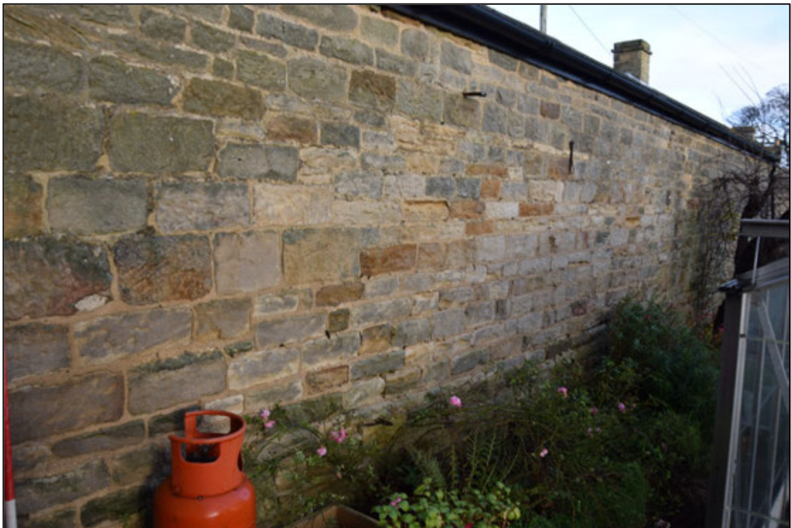
Photograph 12: Different mortar shows where stones have been re-set at the wall head during re-roofing work
