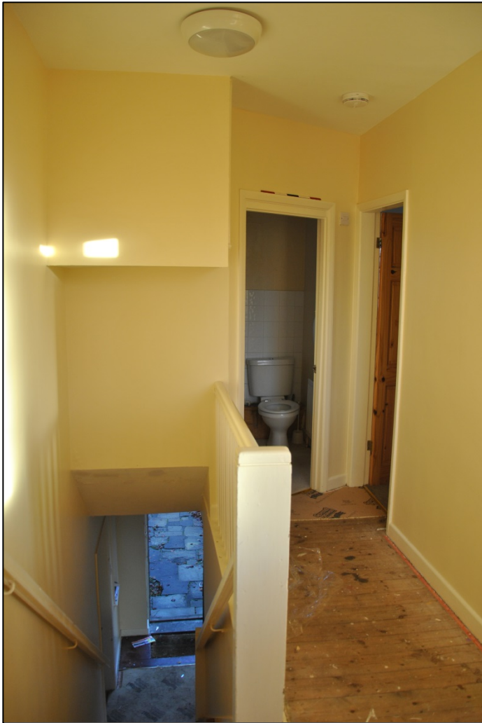
Photograph 13 (left): The landing [8] seen from the west. Before the insertion of the bathroom, the landing ran left beyond the stairs to the northern bedroom
