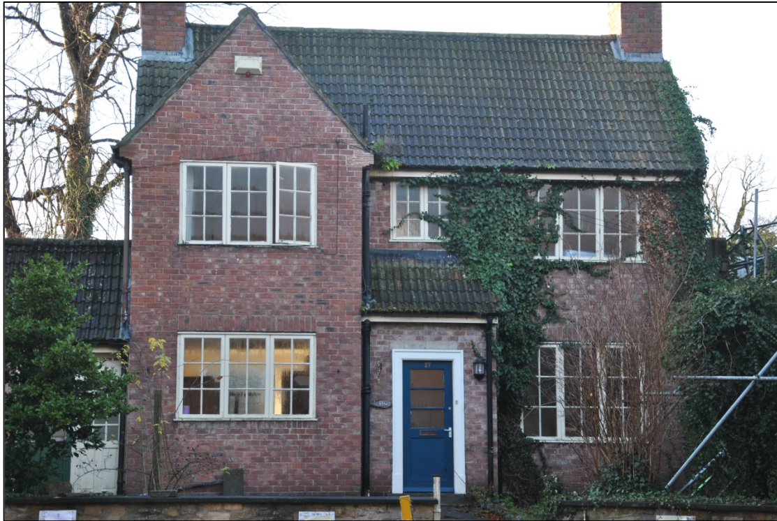
Photograph 3: The east face of no. 17. The porch is a slightly later addition
