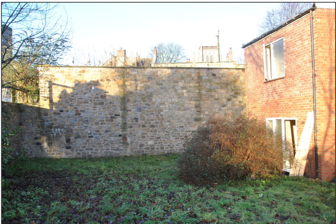
Photograph 6: The modern retaining wall at the north side of the site
