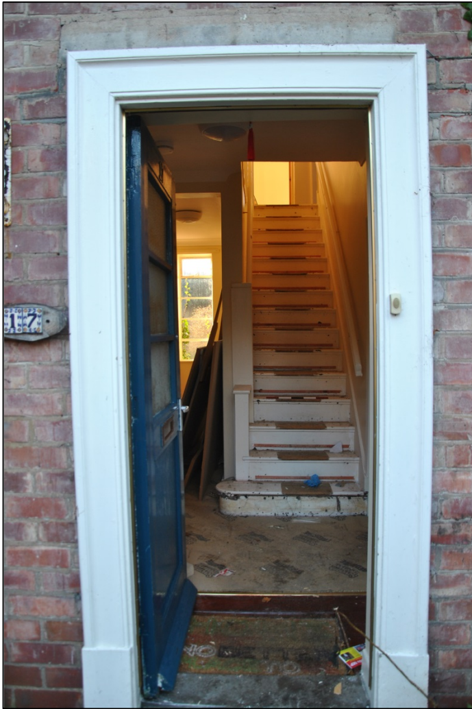
Photograph 7 (left): The staircase and hall seen from the front door
