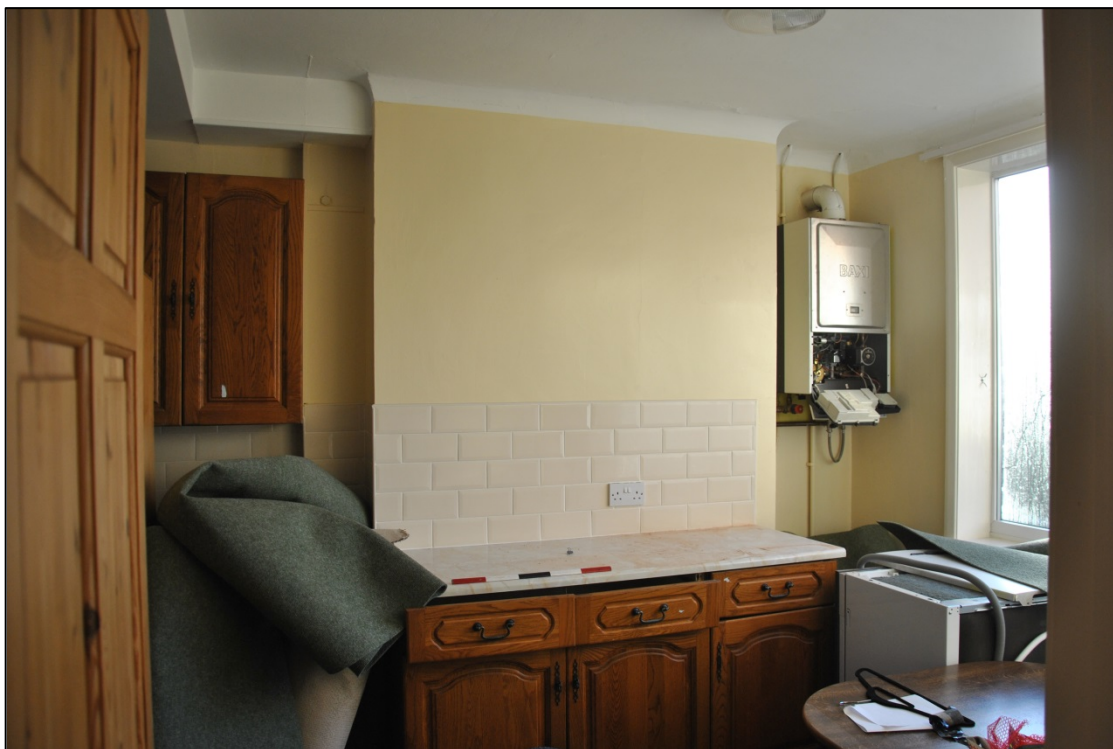
Photograph 8 (below): Looking south into the kitchen [4]. Note the blind chimney breast
