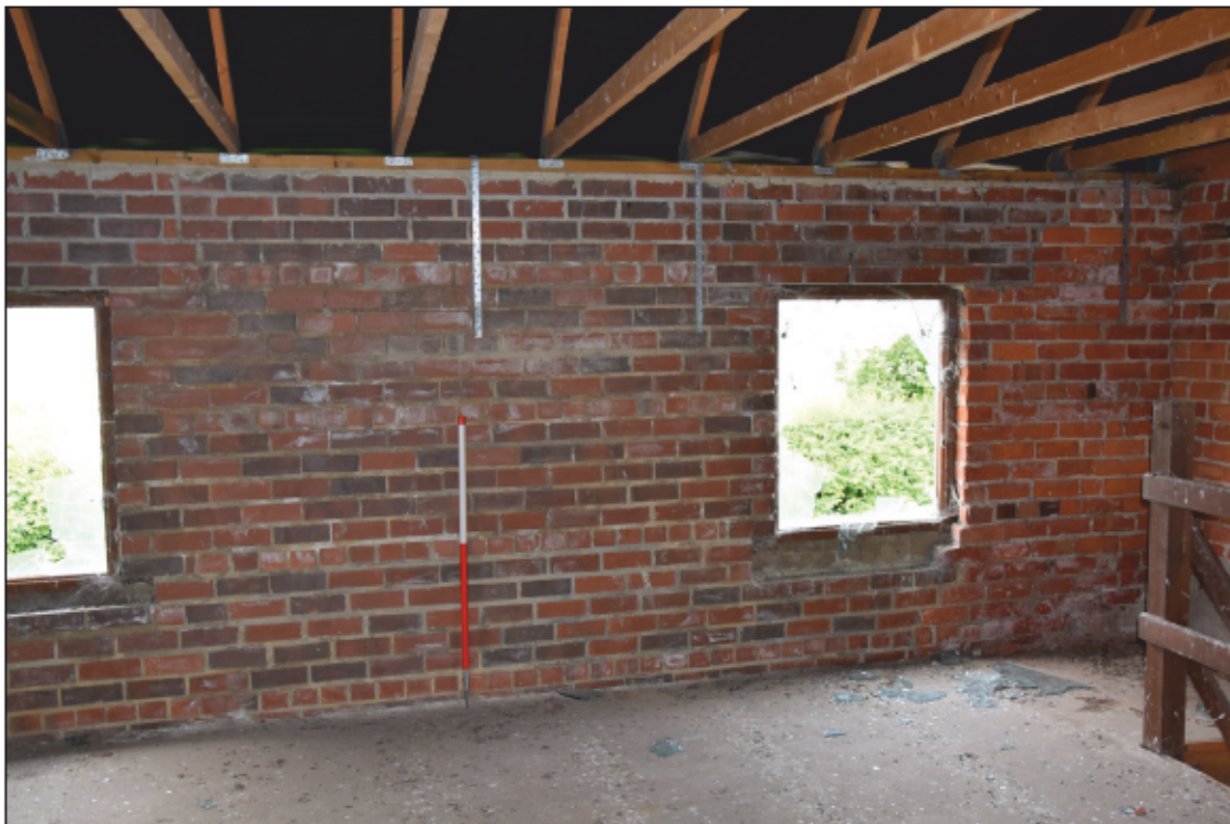
Photograph 60: New brickwork in the north-east wall
