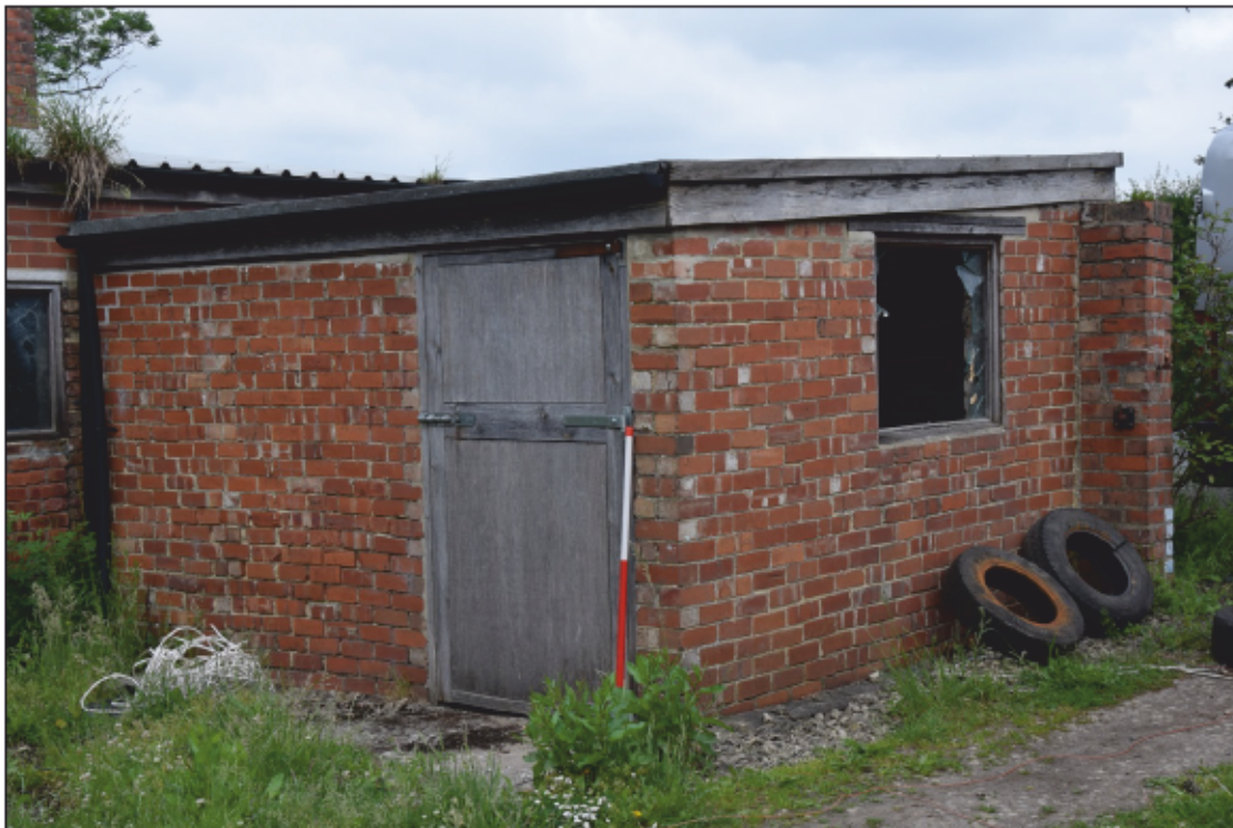
Photograph 38: The brick workshop seen from the yard
