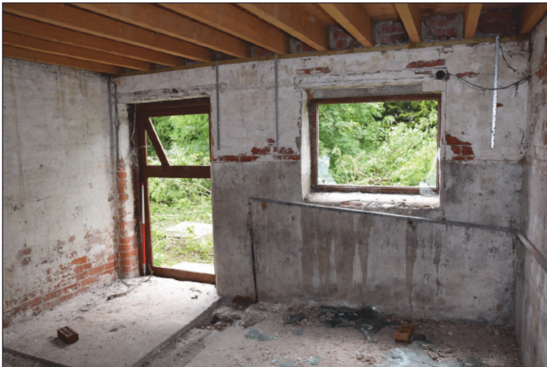
Photograph 56: Door and window in the north-west room
