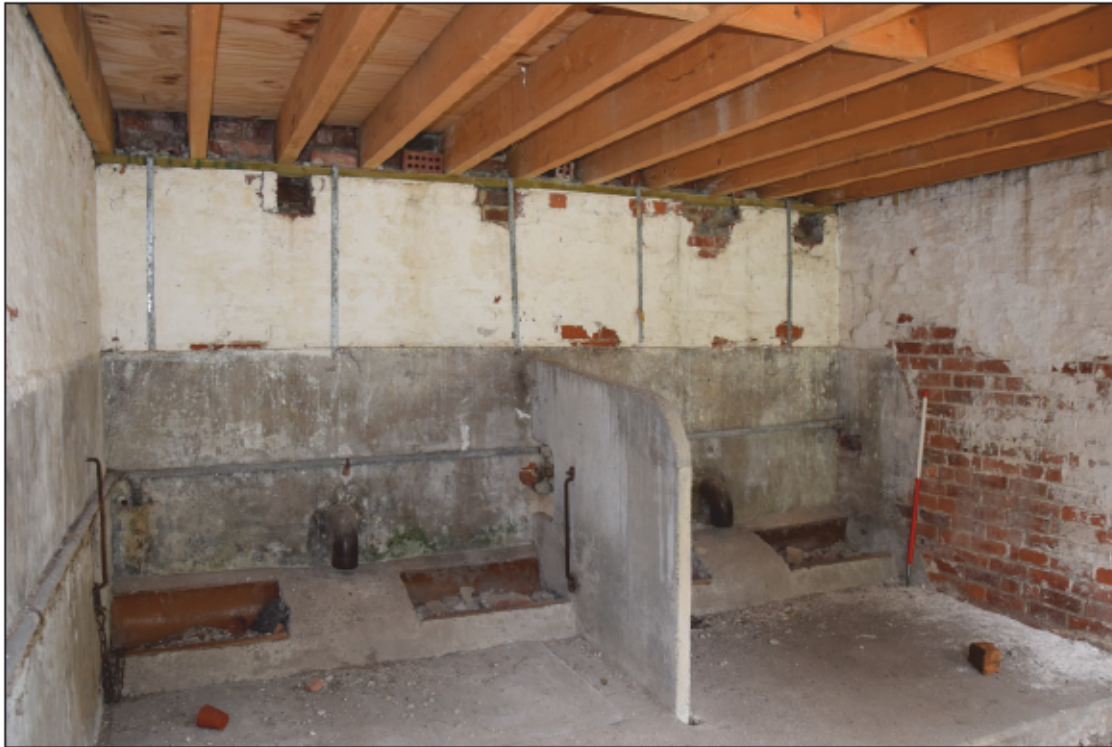
Photograph 55: Stalls in the small byre at the north-west end of the large building
