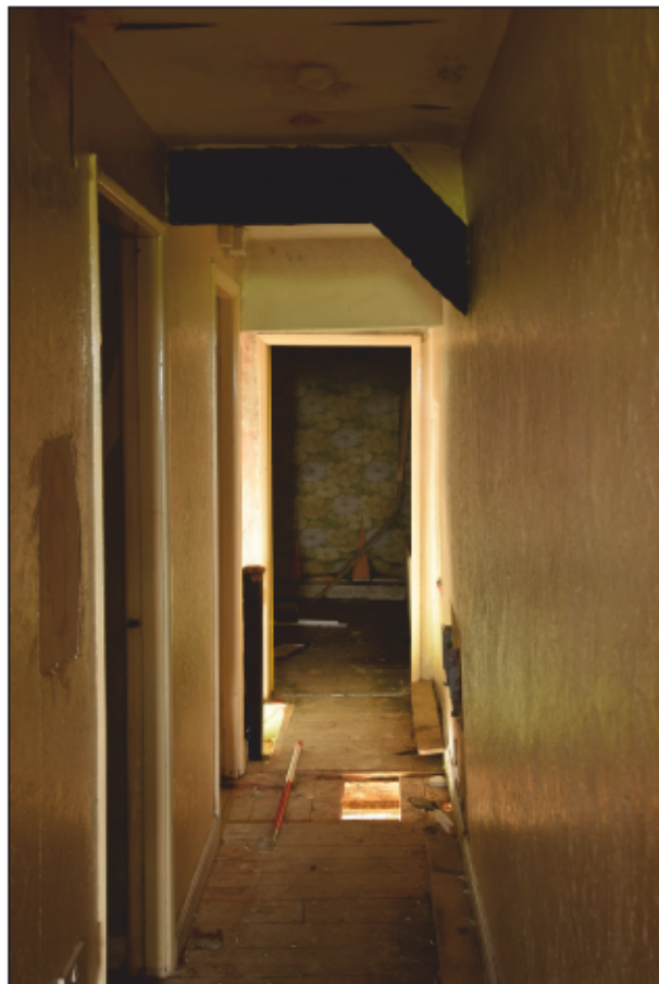
Photograph 32: The landing seen from the bedroom in the extension
