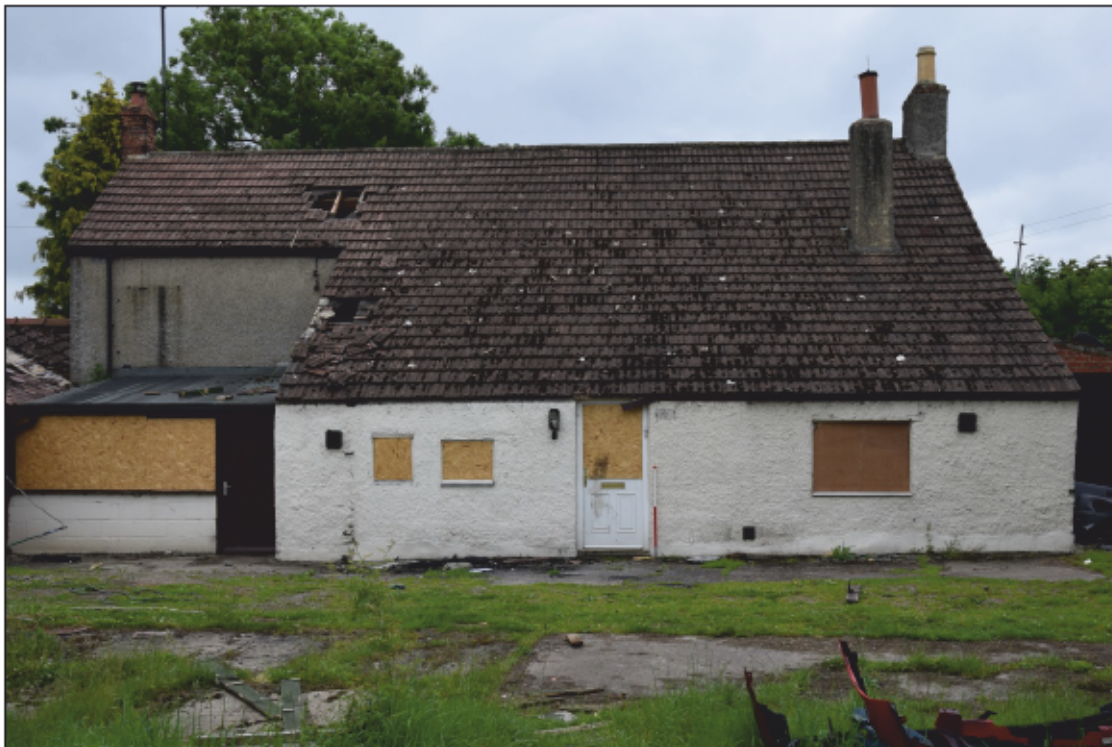
Photograph 10: The rear of the house, with the later extension visible as the grey wall at the left
