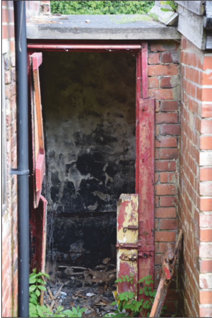
Photograph 41 (left): The coal shed. The mark of a timber privy seat can be seen in the back wall
