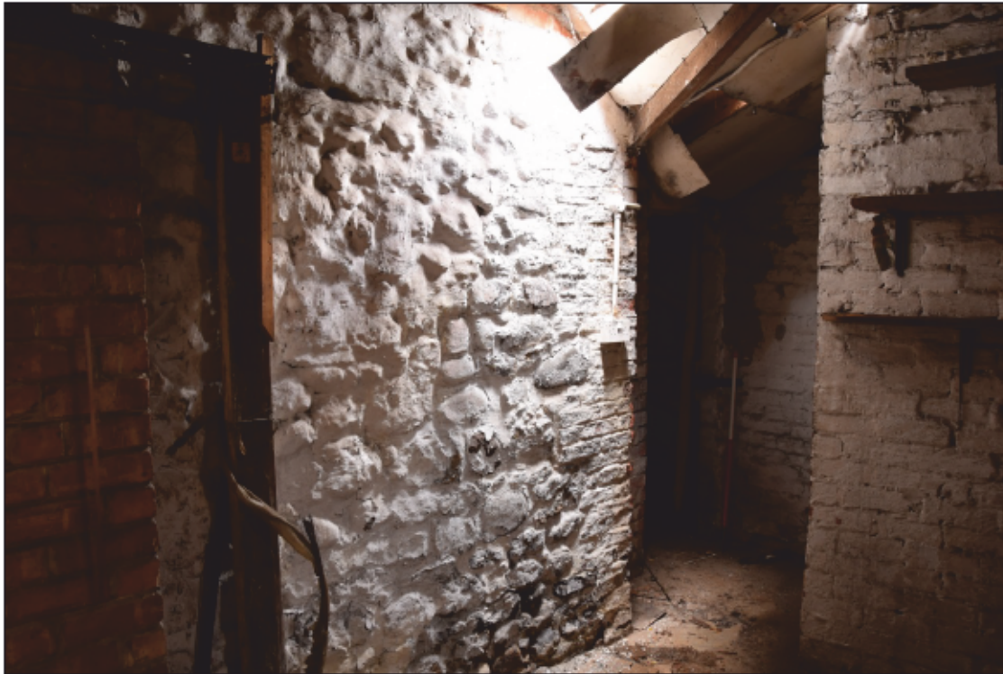
Photograph 29: The north corner of the house extension seen in the shed; note the brickwork at the angle
