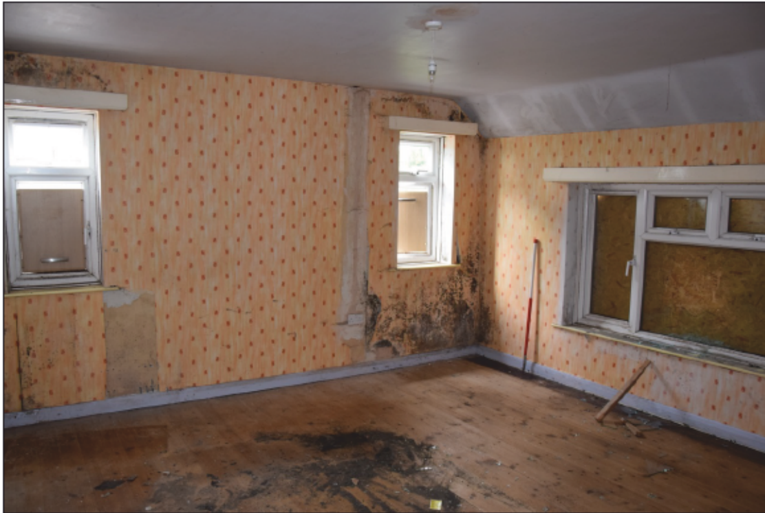
Photograph 37: The large north-east bedroom, with modern uPVC windows
