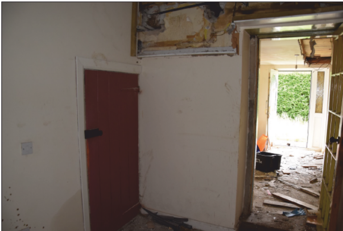
Photograph 22: The lobby and hall, with the old door to the passage
