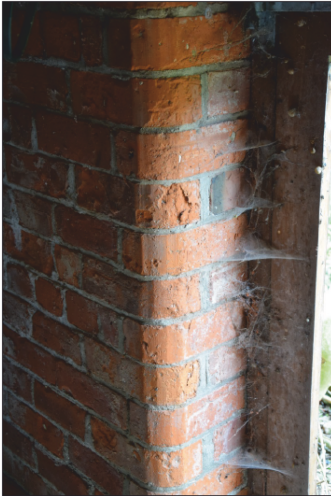
Photograph 57 (left): Detail of the rounded brick in the door jamb of the small byre
