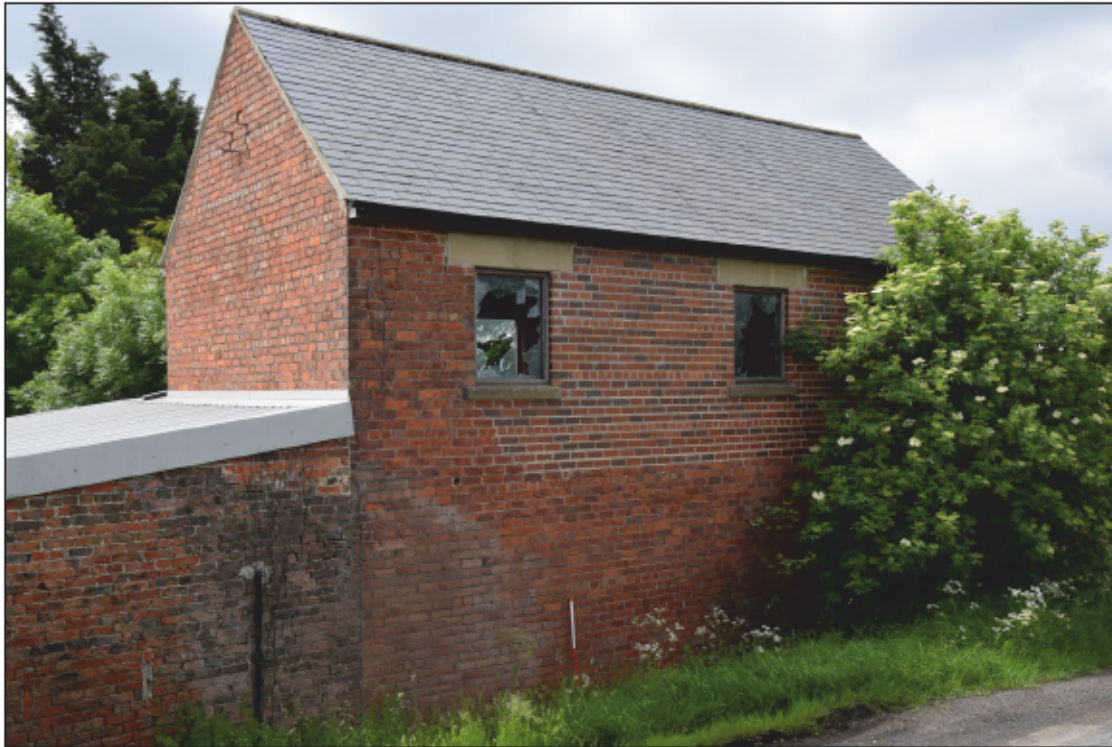
Photograph 51: The two-storey brick building seen from the east
