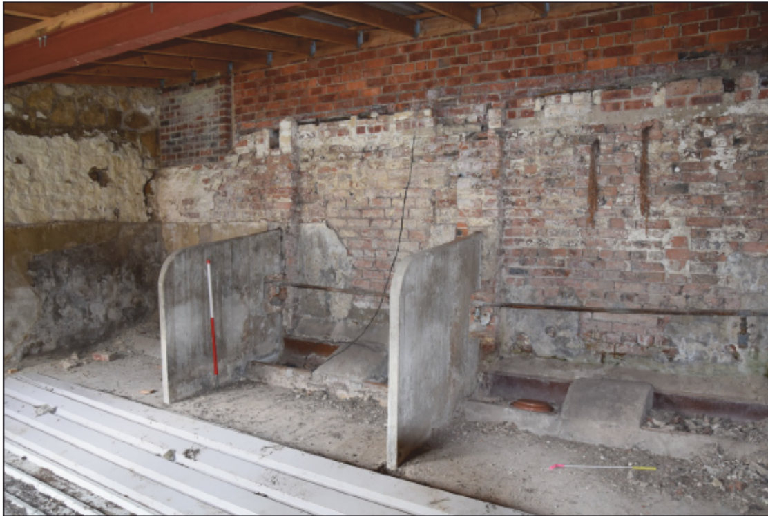
Photograph 47: Looking west in the brick byre
