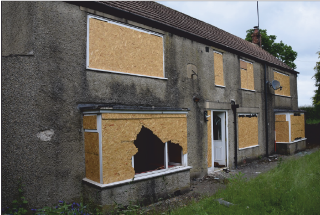
Photograph 7: The house seen from the south corner of the garden
