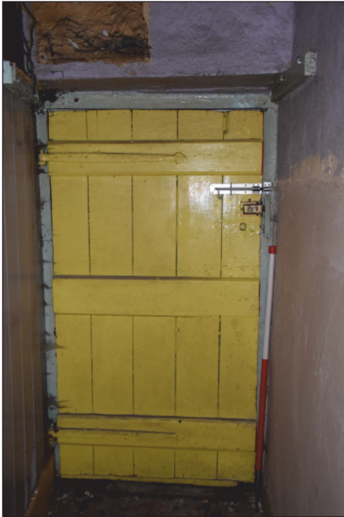
Photograph 25 (left): Old plank door at the north-east end of the passage
