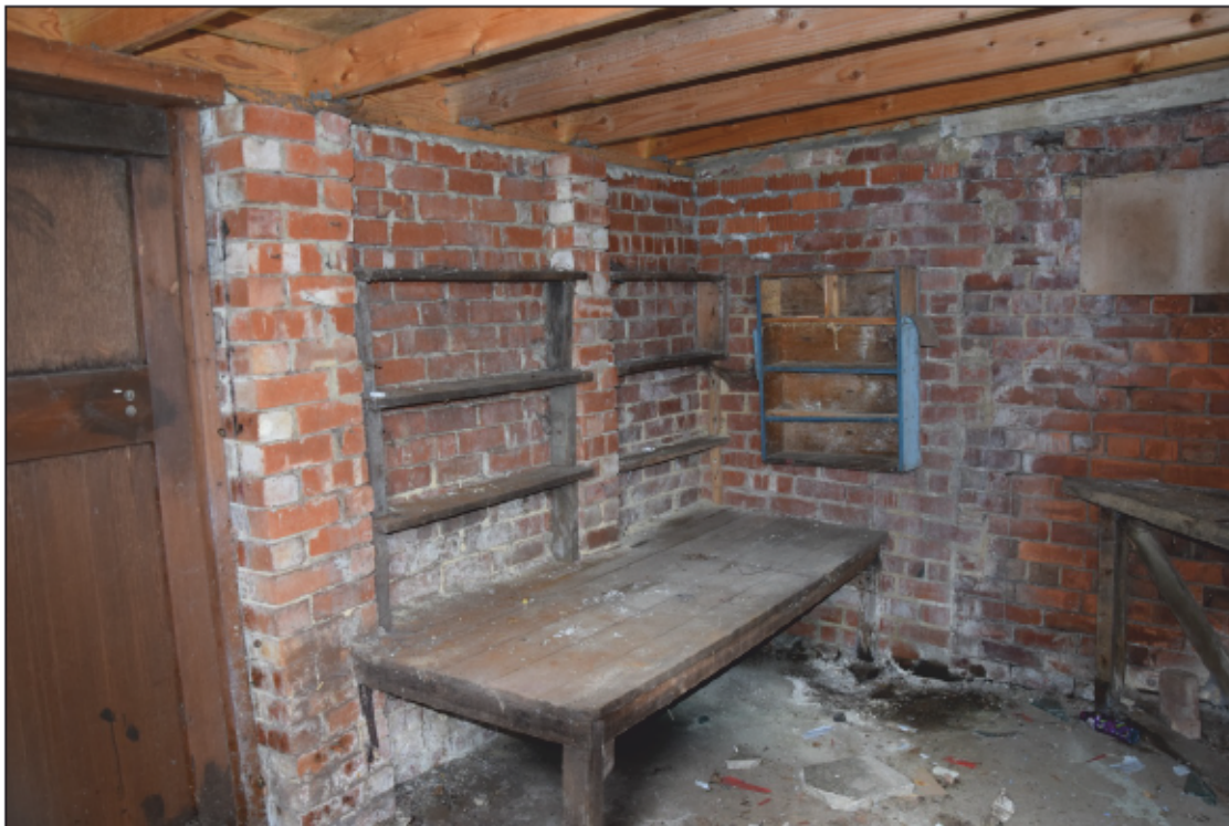
Photograph 40: Interior of the workshop
