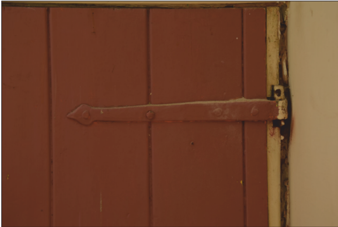
Photograph 23 (above): Detail of another old strap hinge on the lobby door
