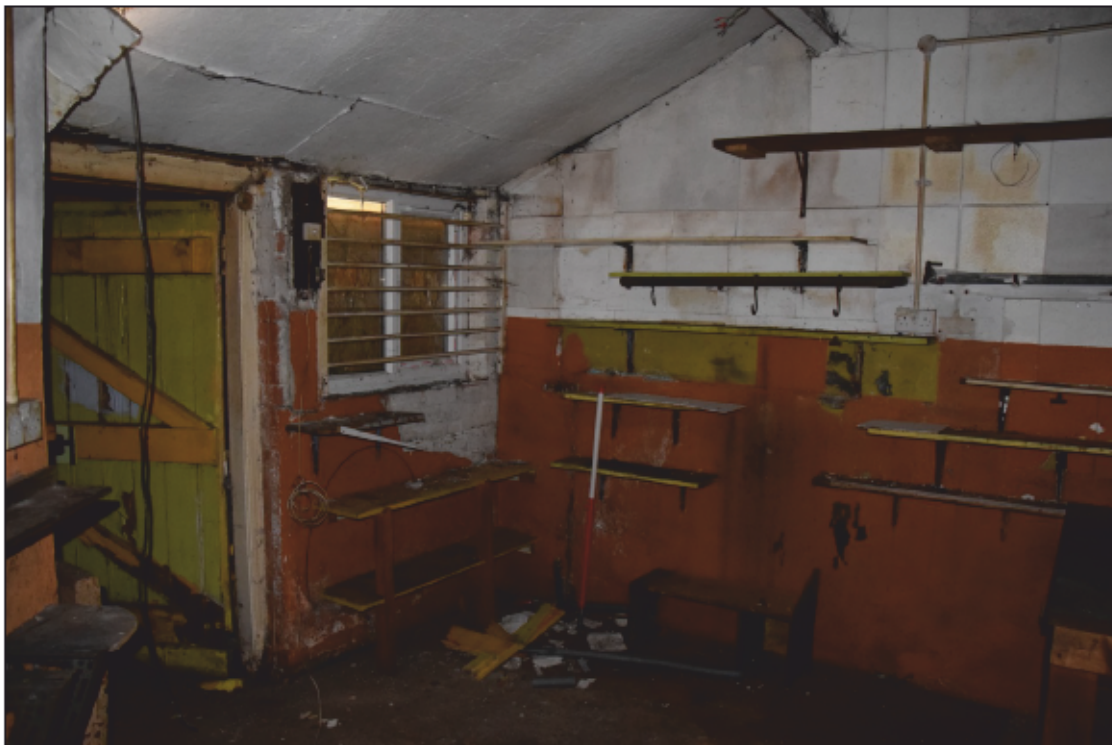
Photograph 30: The north-west shed
