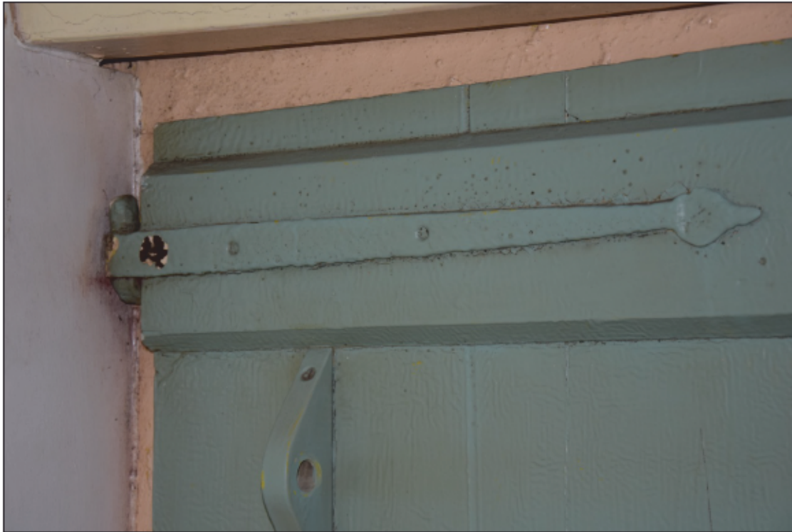
Photograph 21: Detail of the strap hinge and pintles of the kitchen door
