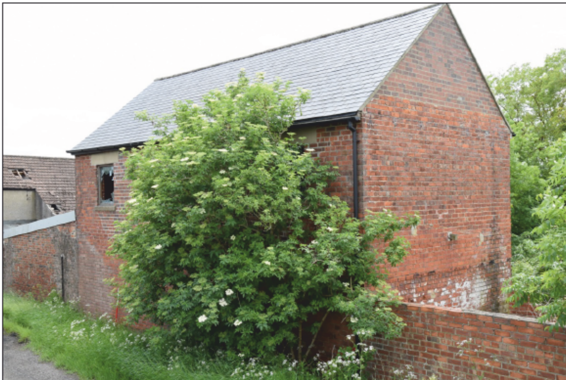
Photograph 52: The north-west gable, partly rebuilt
