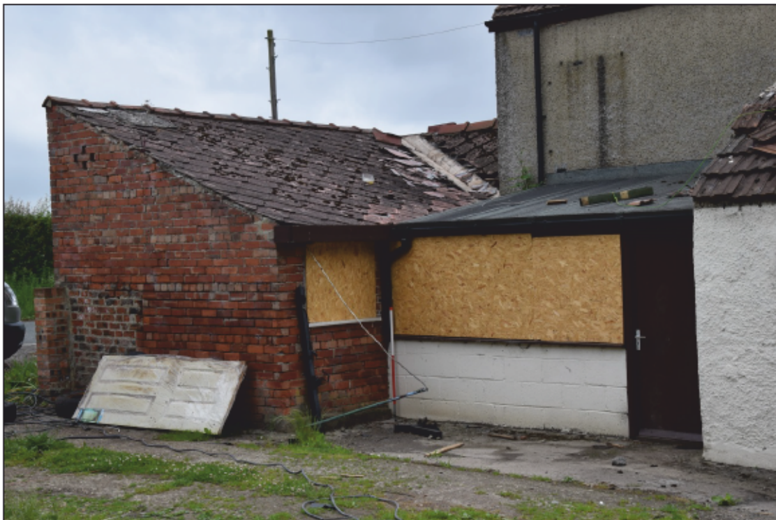
Photograph 12: The sheds at the north-east end of the house
