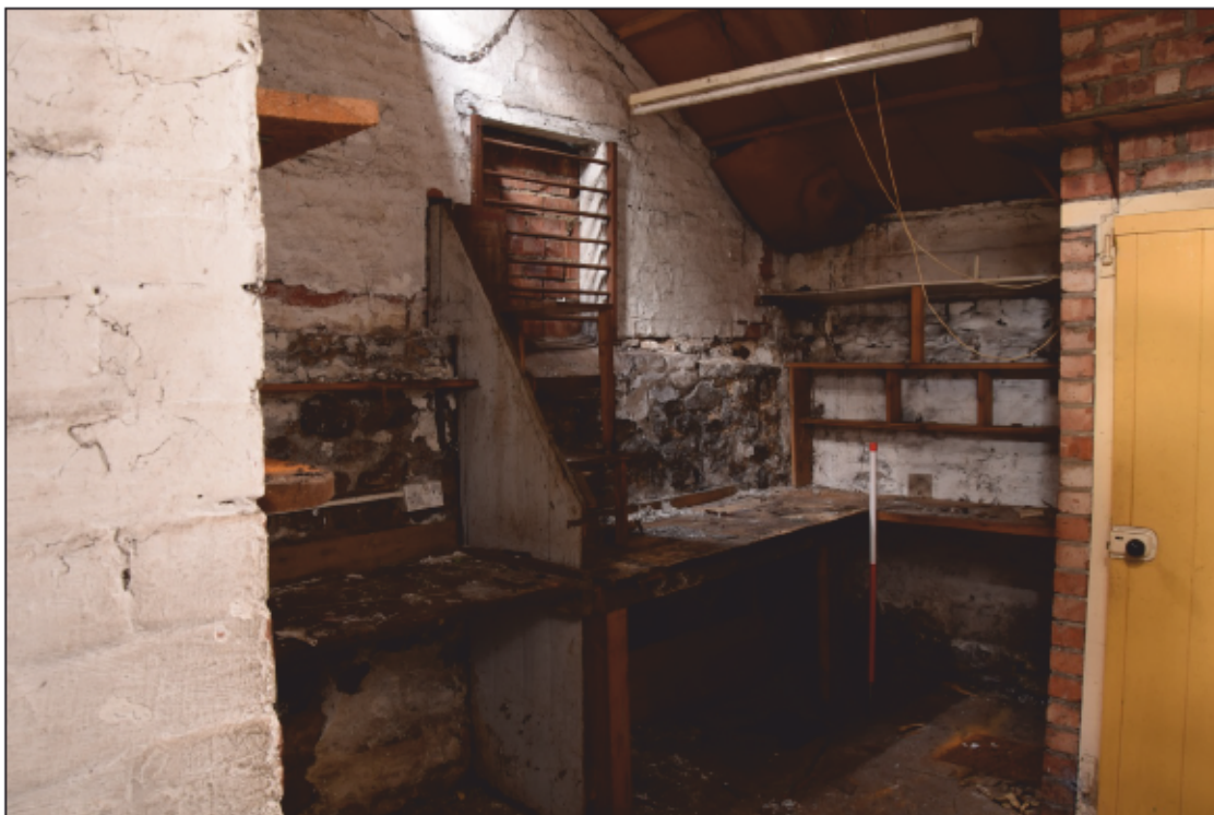
Photograph 28: The old shed at the south-east side; note the stonework of the lower walls, and the blocked window above
