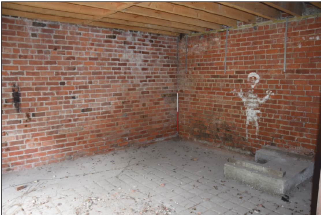
Photograph 54: Impressed concrete floor and machine plinth in the south-east room
