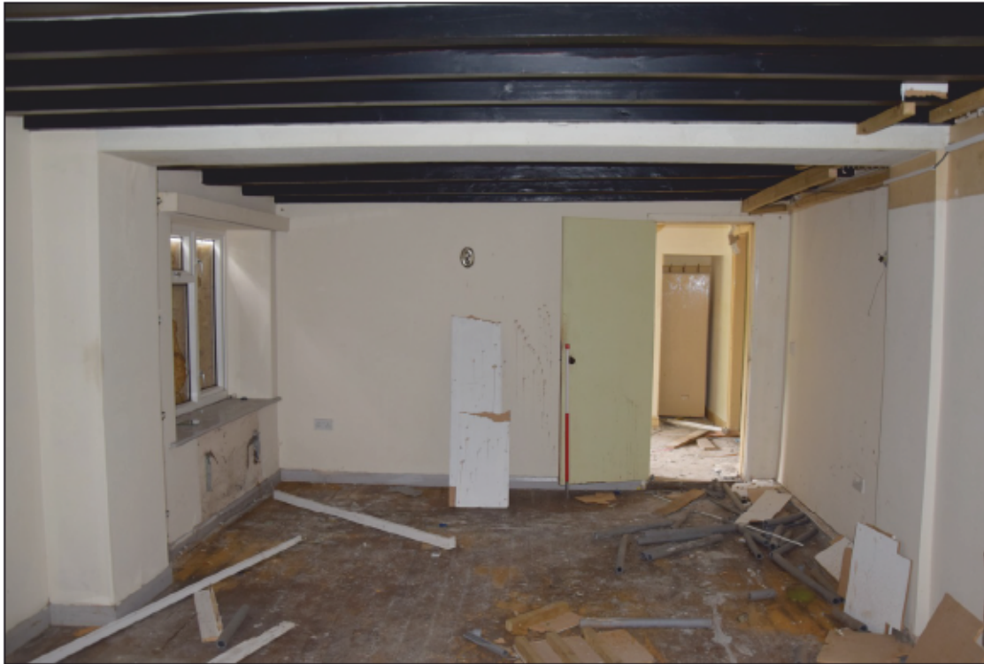
Photograph 17: The sitting room seen from the north-west end
