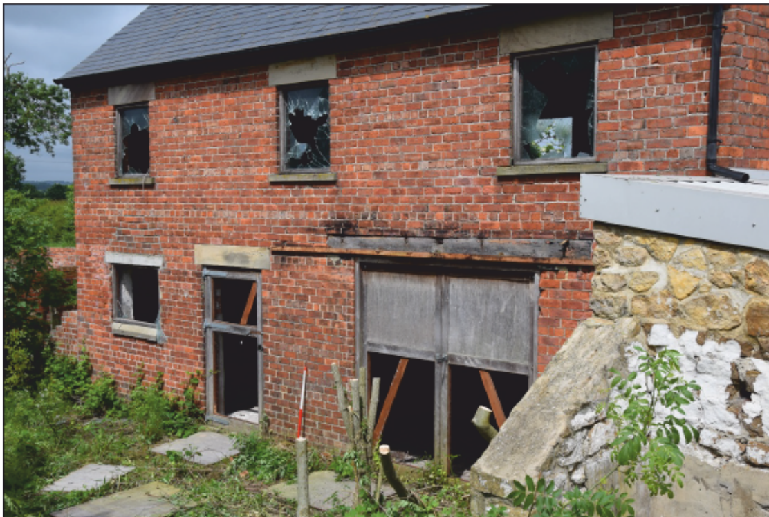
Photograph 50: The altered brick building at the north side
