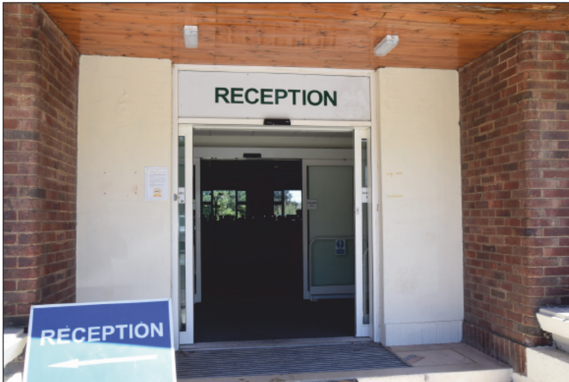
Photograph 21: Modern doors replace the original revolving door in the reception area 1
