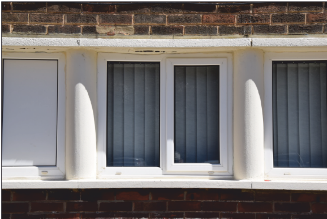
Photograph 10: Detail of the concrete slab sill and lintel, and the mullions
