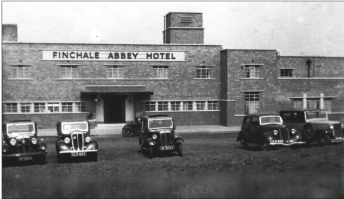
Photograph 1: The hotel and car park in the 1930s. Note the steel-framed windows throughout the façade. This photograph was kindly provided by Finchale College
