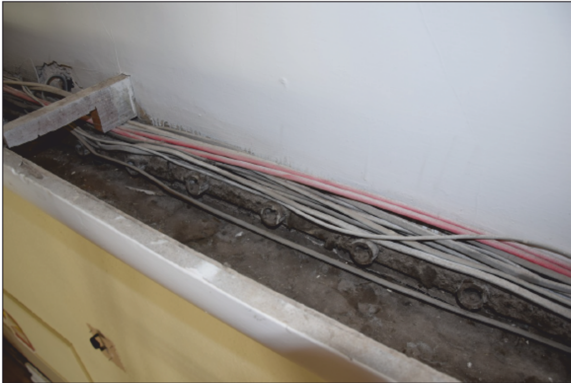
Photograph 49: Inside the plaster coving are battens and old ceramic lamp holders for concealed lights above the middle of the dance floor
