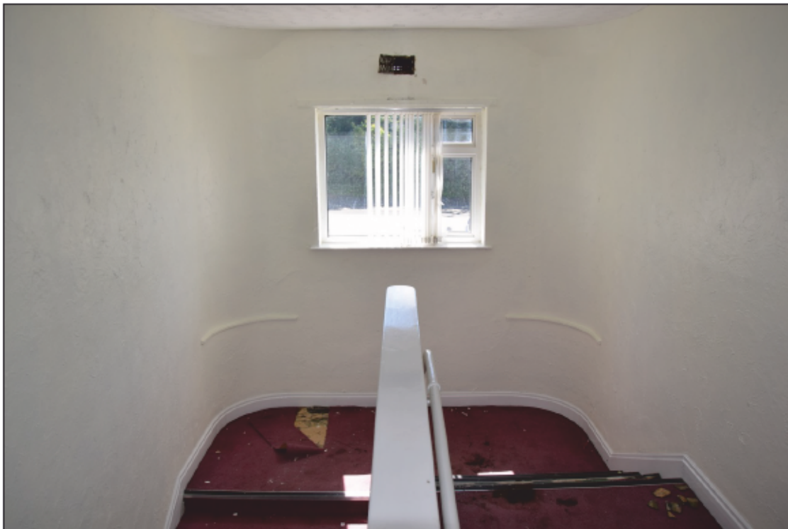
Photograph 54: The staircase seen from the landing
