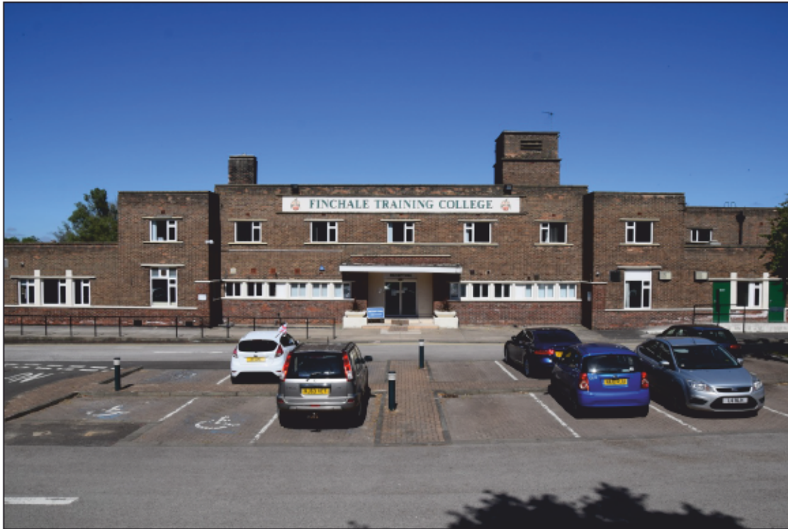
Photograph 5: The entrance front of the former hotel, showing the near-symmetrical arrangement and the strong horizontal emphasis of the building's design
