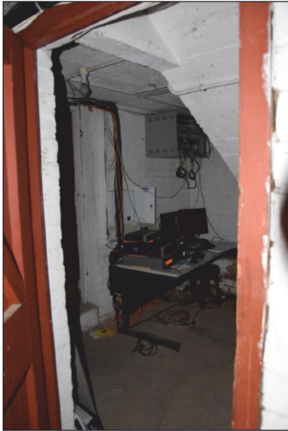
Photograph 39 (left): A bare brick and concrete room under the service staircase
