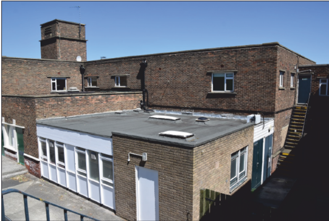
Photograph 15: The recent extension at the south-west corner of the building. The upper wall between the window and the fire escape door is part of the 1936 extension
