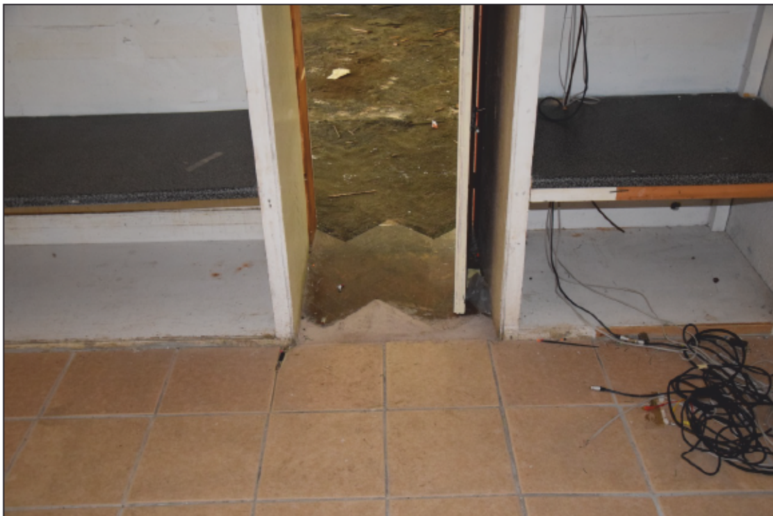
Photograph 36: The parquet floor of the dining room continues under the modern tiles of room 10
