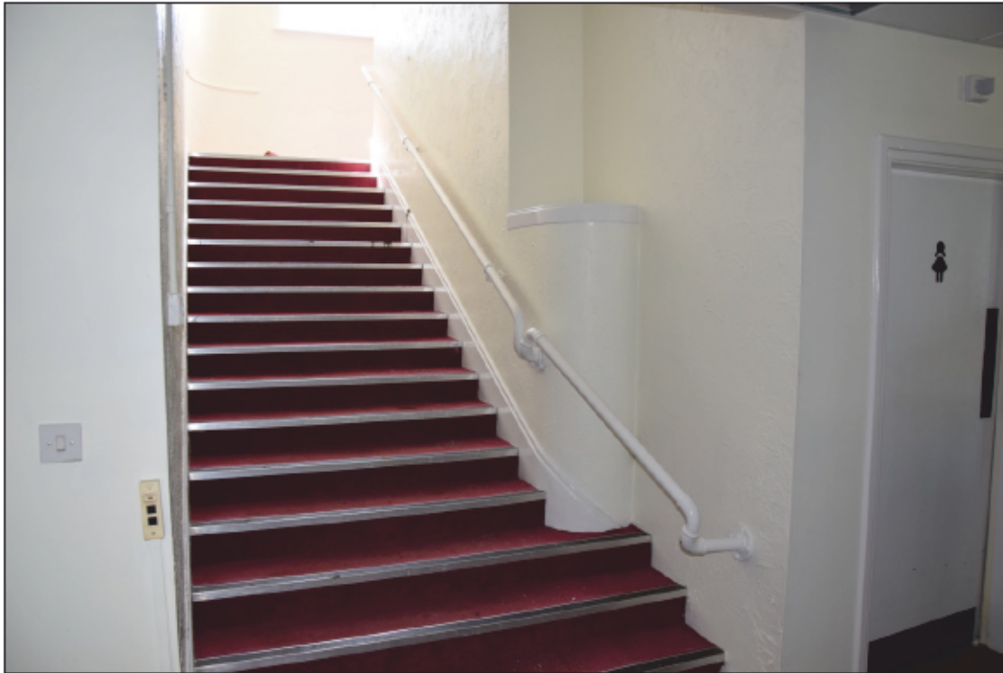
Photograph 53: The main staircase 18, with its incongruous steel-pipe handrail
