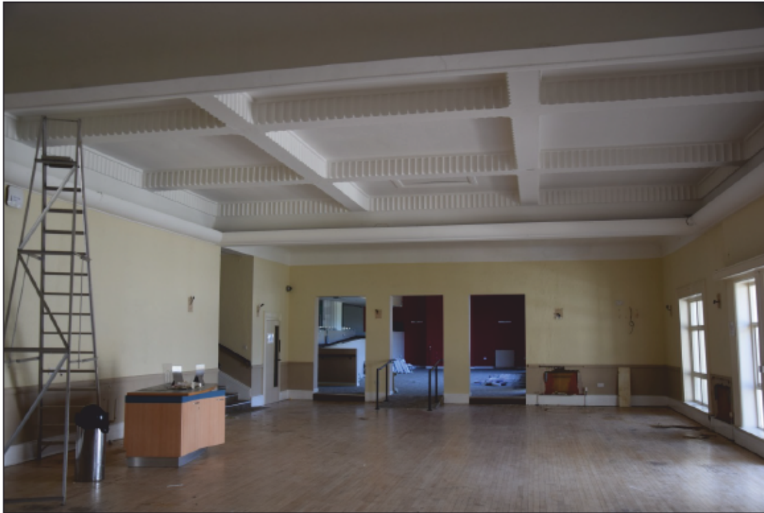
Photograph 47: The ballroom 15, seen from the south-east corner. The far wall was originally solid and the entrance was by way of the steps, left of centre
