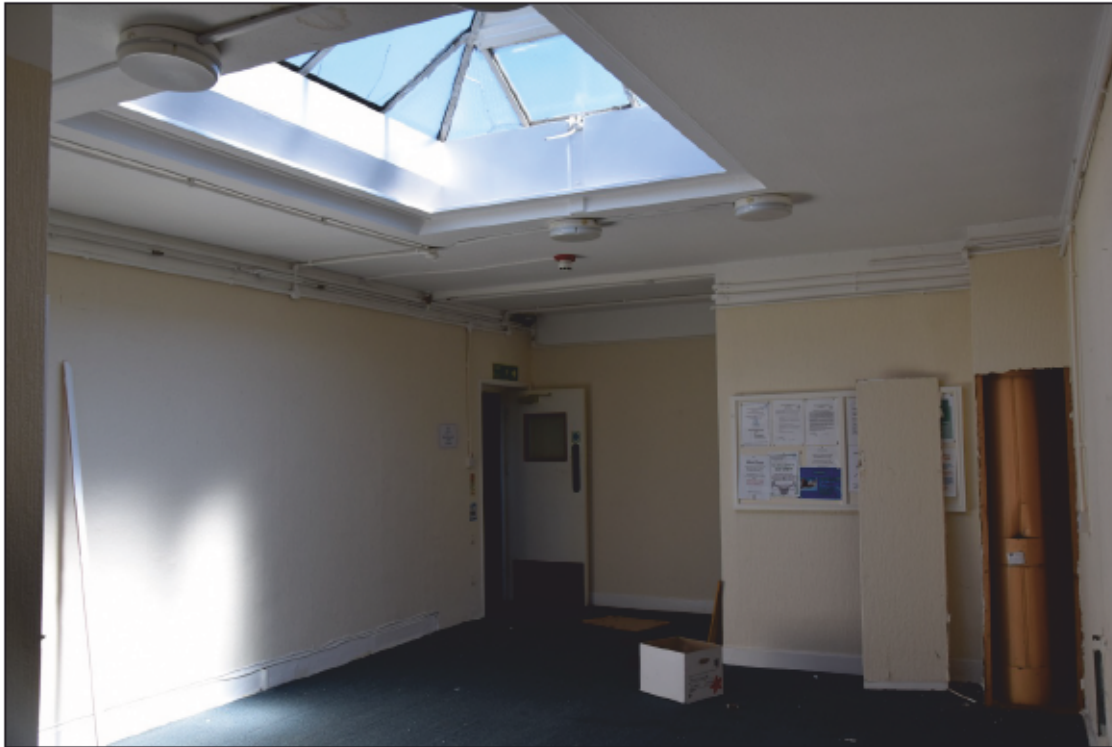
Photograph 67: The former kitchen 40, with the 1935 roof light and the 1936 extension
