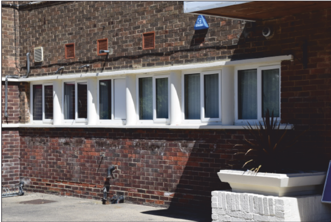
Photograph 9: Strip windows with semi-cylindrical concrete mullions, north of the entrance
