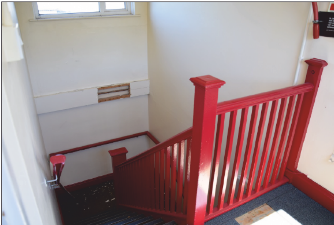
Photograph 66: The service staircase 39
