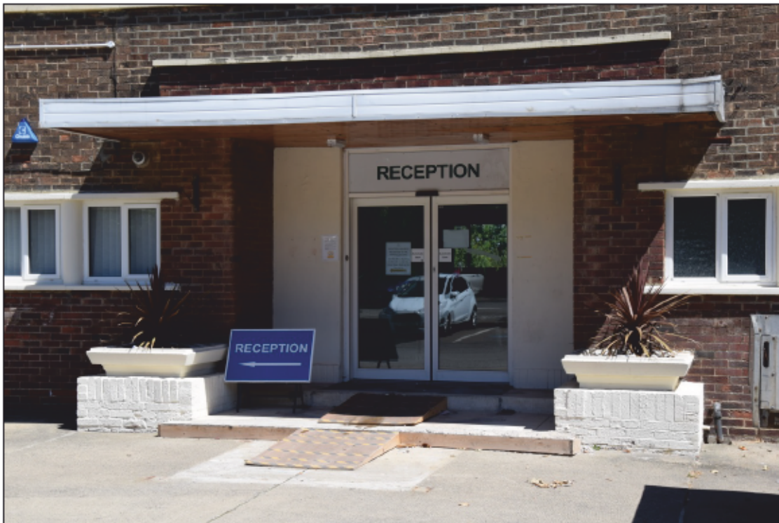
Photograph 14: The entrance with the brick plinths for planters. Modern cladding hides the concrete slab canopy
