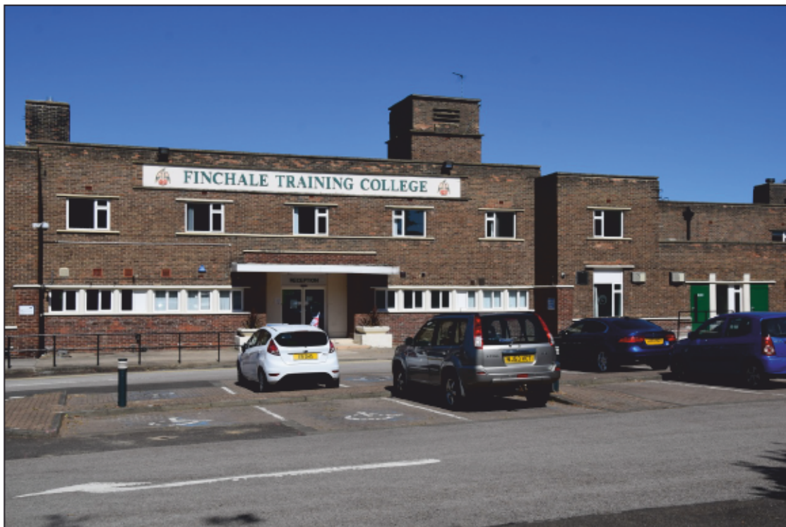
Photograph 2: The same view in 2018. All of the windows have been altered and vents, air bricks and other fittings have been added, but the façade is otherwise unchanged
