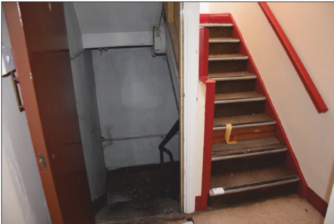
Photograph 38: The foot of the service stairs 39 and the steps down to the cellar. A view looking east
