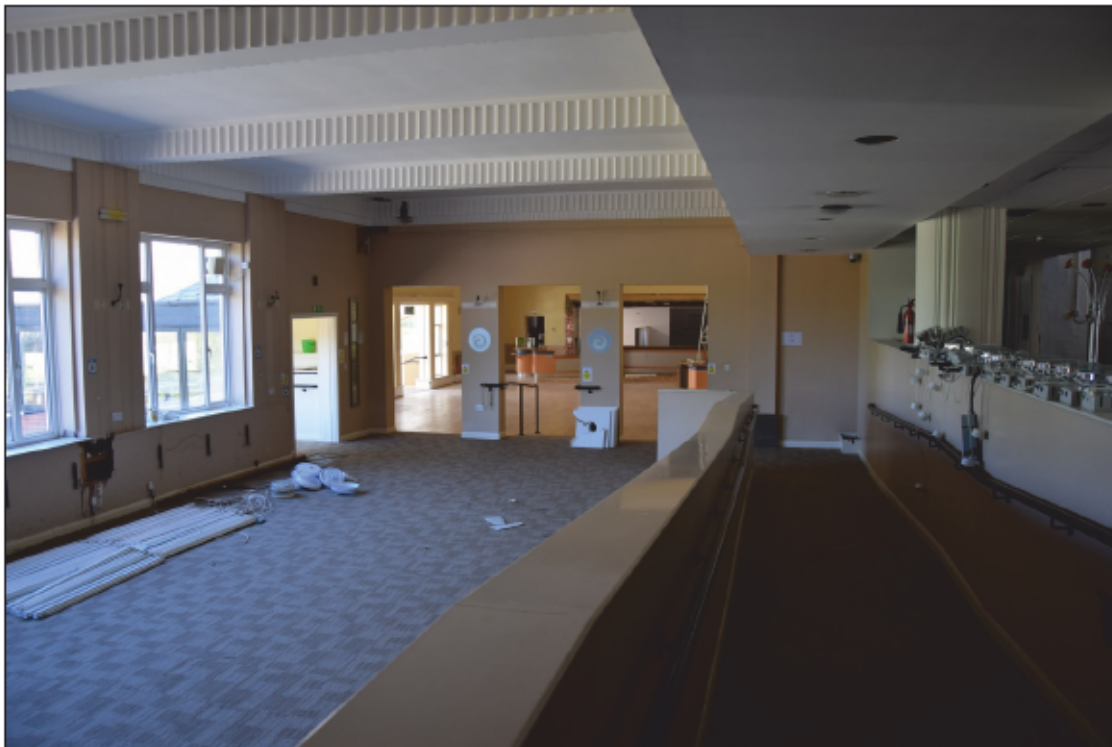
Photograph 42: The lounge 14 and ballroom 15, seen from the north end of the modern access ramp
