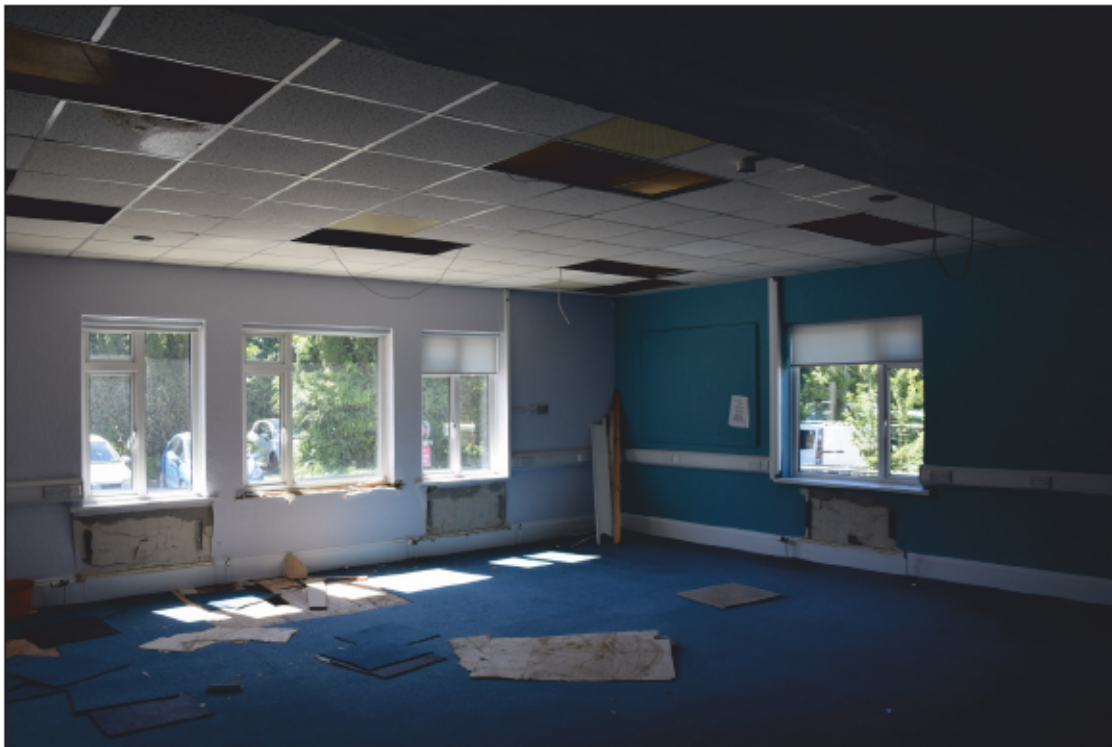
Photograph 30: The former bar, room 5
