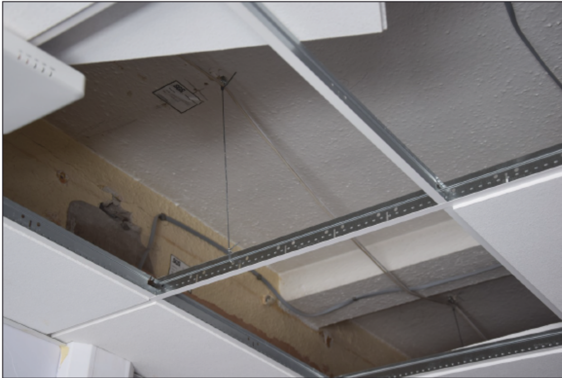
Photograph 29: Plain ceiling and beam above the modern suspended ceiling of room 4
