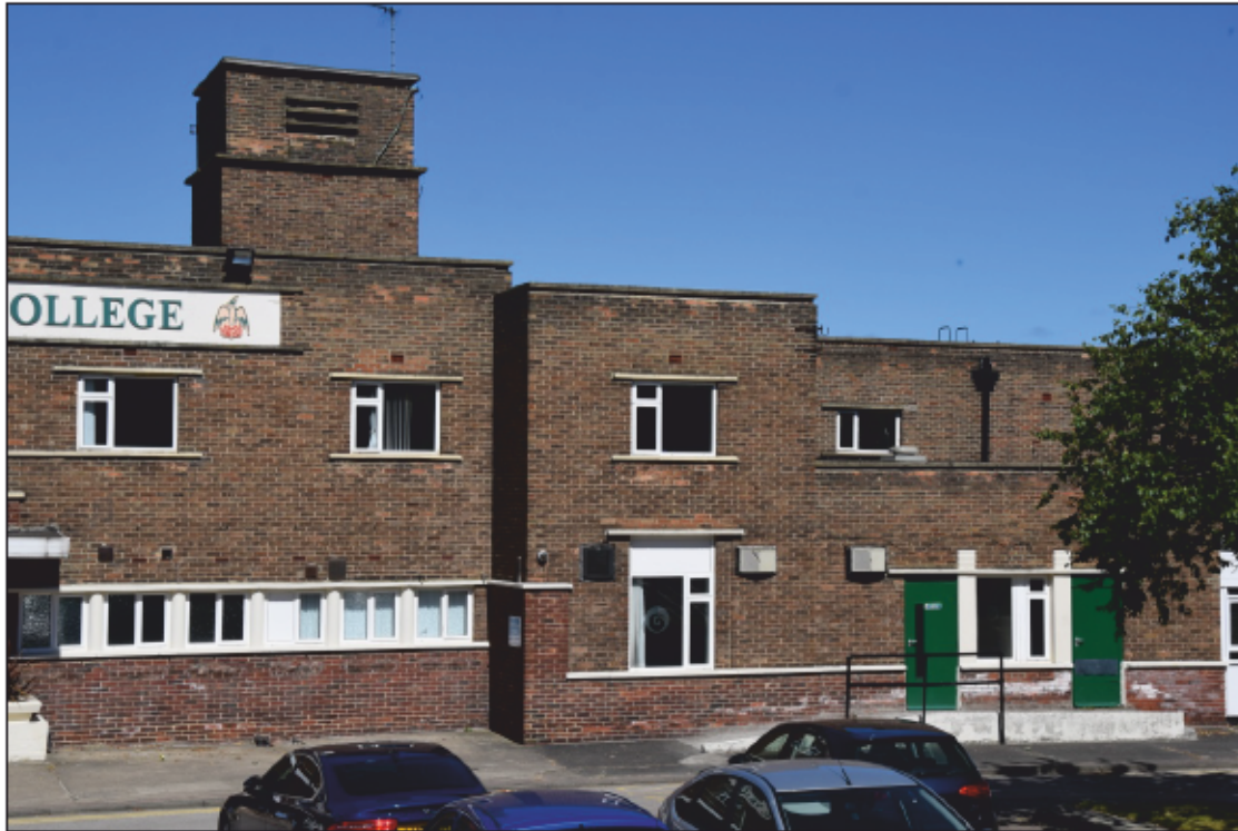
Photograph 7: The south wing, formerly the dining room and manager's quarters
