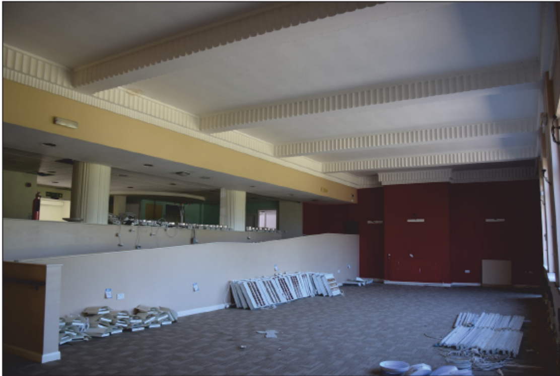
Photograph 41: The lounge 14, seen from the south-east corner
