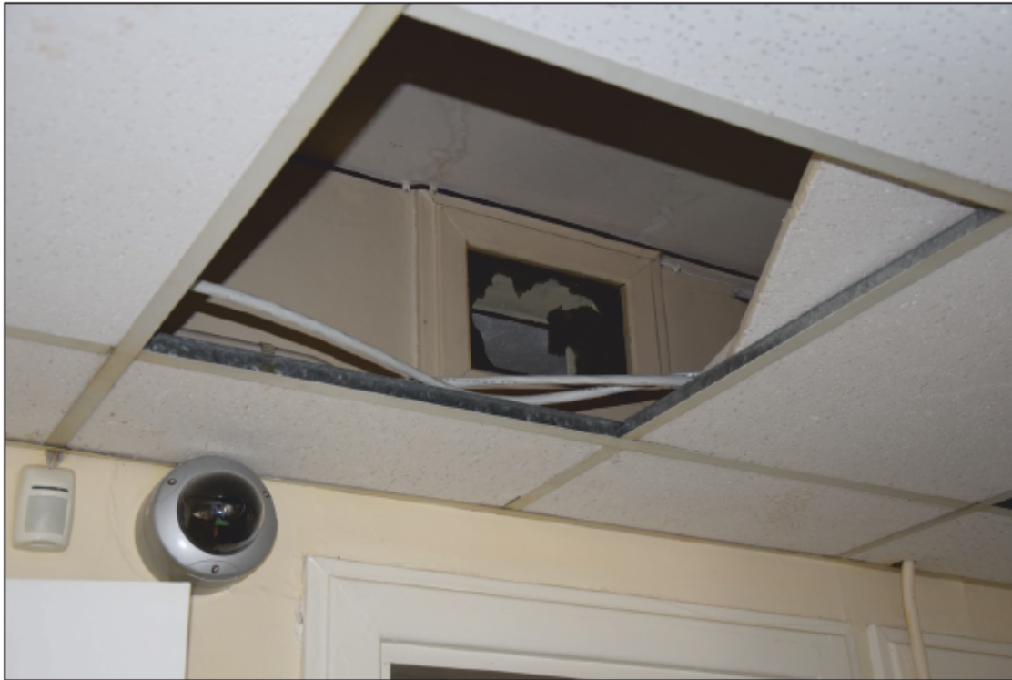
Photograph 63 (above): The suspended ceiling conceals a ventilator in the south end of the store room 26
