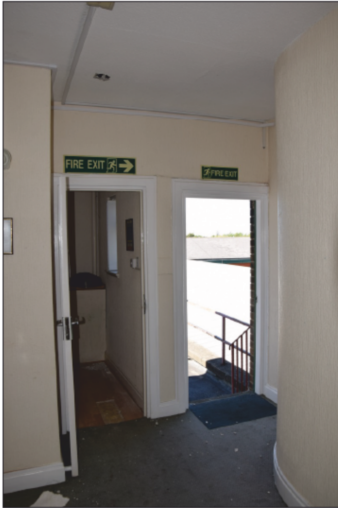
Photograph 57 (left): The former housemaids' cupboard 27 and fire escape at the end of the guest corridor
