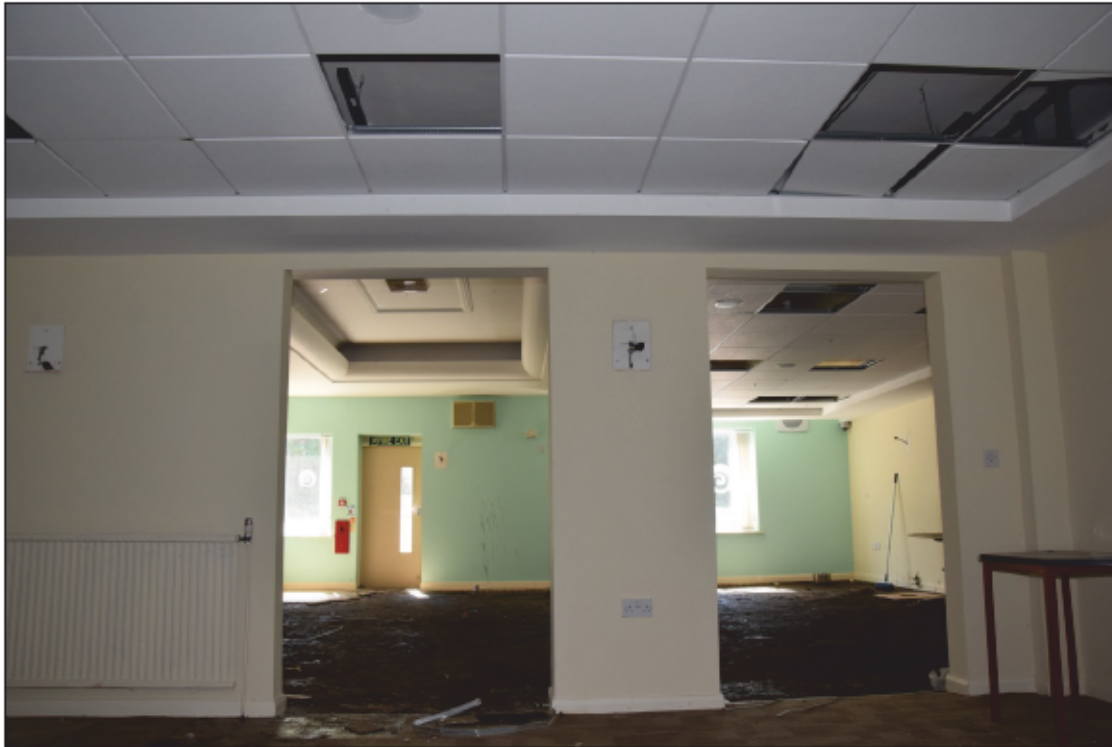
Photograph 37: A view from the buffet room 11 into the former dining room 9
