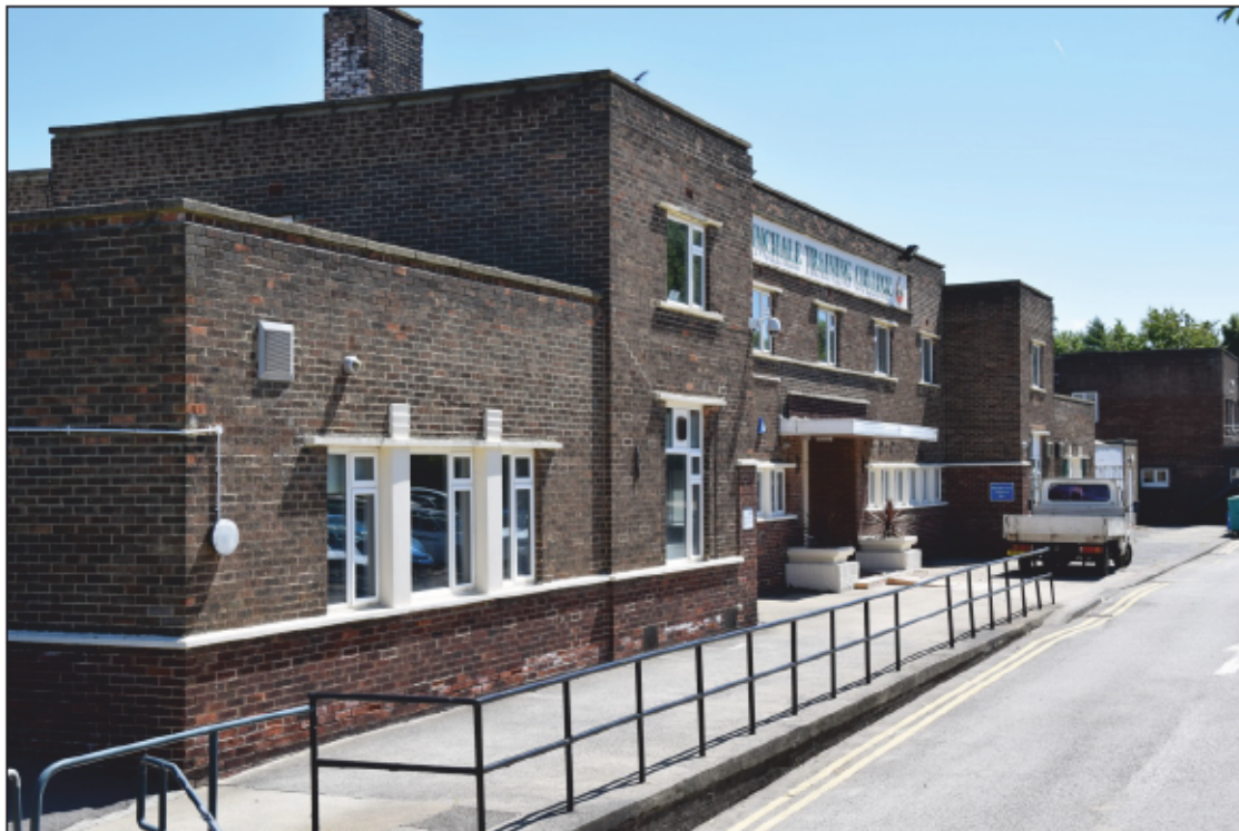
Photograph 8: The west face of the Priestman Building seen from the north-west
