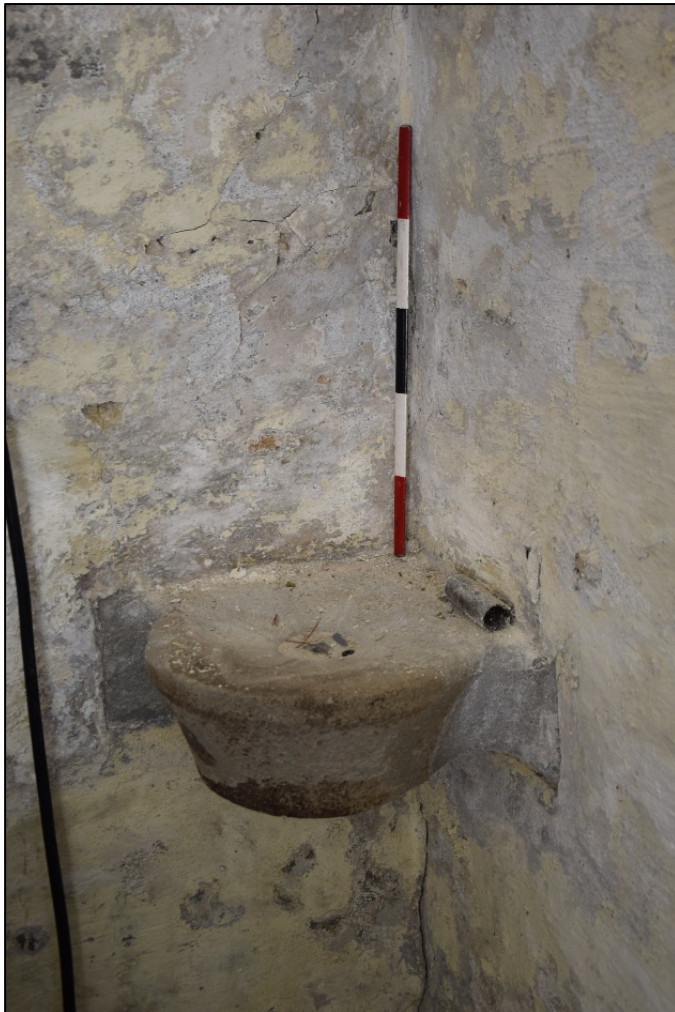
Photograph 39 (above): The east wall of the vestry, showing a recent hole for cable ducts and the damp-affected plasterwork
