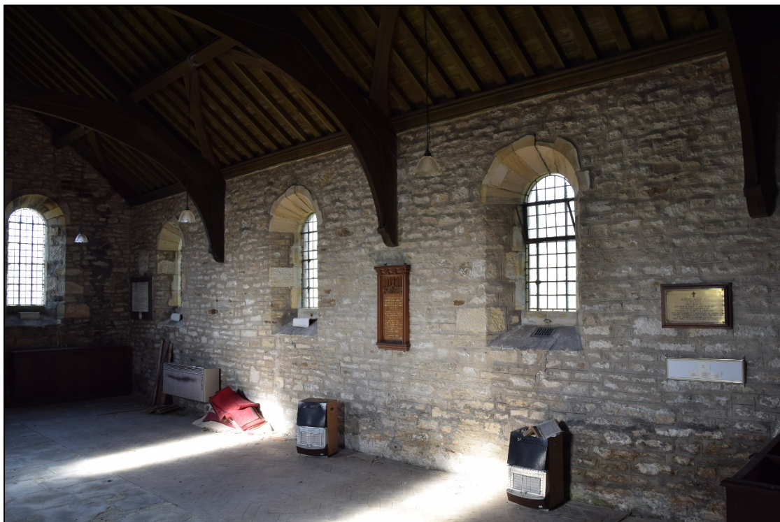
Photograph 24: The north wall of the nave
