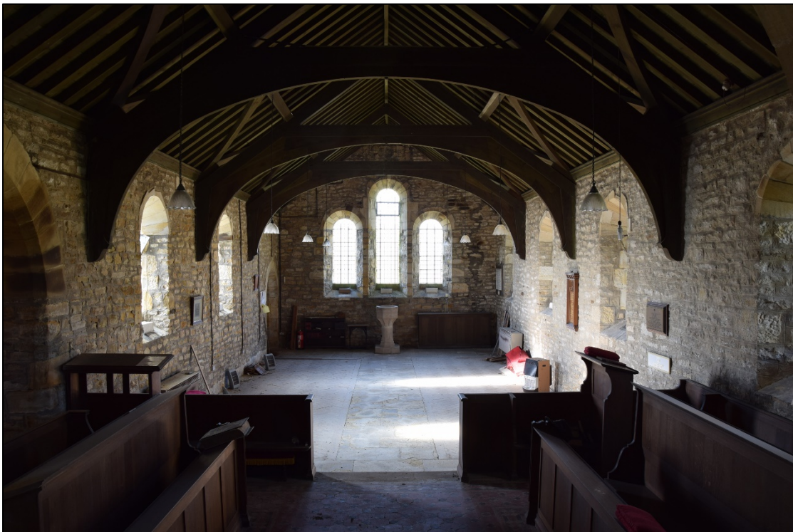
Photograph 26: The church seen from the east end. The stone flags at the centre of the nave are flanked by parquet where the pews stood
