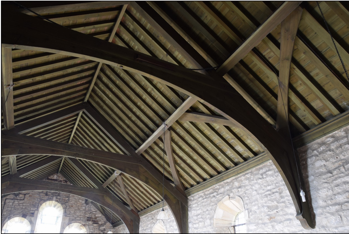
Photograph 35: The roof of the nave and choir. A view looking north-west
