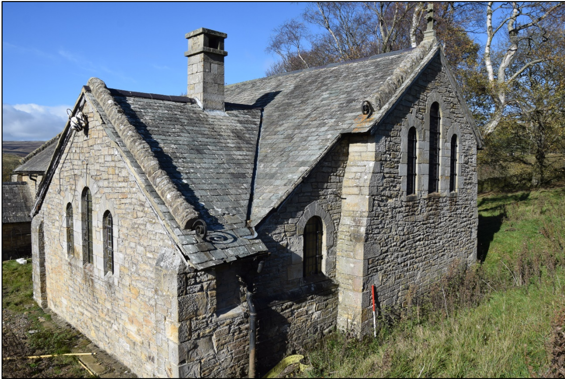
Photograph 9: The east end of the church is cut into the slope. The chimney served a stove in the vestry
