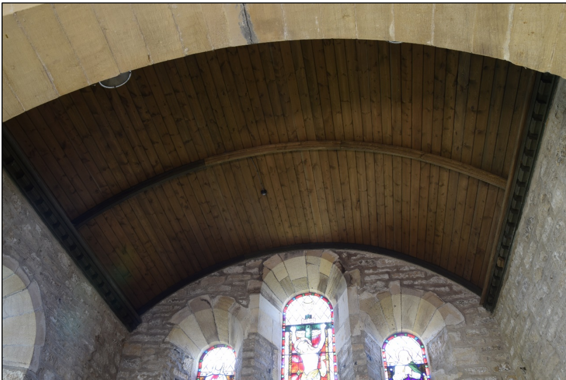
Photograph 36: The wagon roof over the chancel
