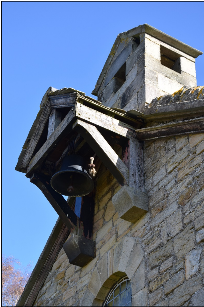
Photograph 17 (left): The ventilator on the west gable, with the bell cote below it
