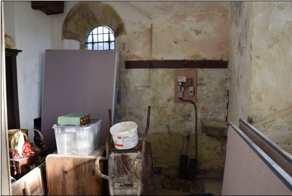
Photograph 39 (above): The east wall of the vestry, showing a recent hole for cable ducts and the damp-affected plasterwork
