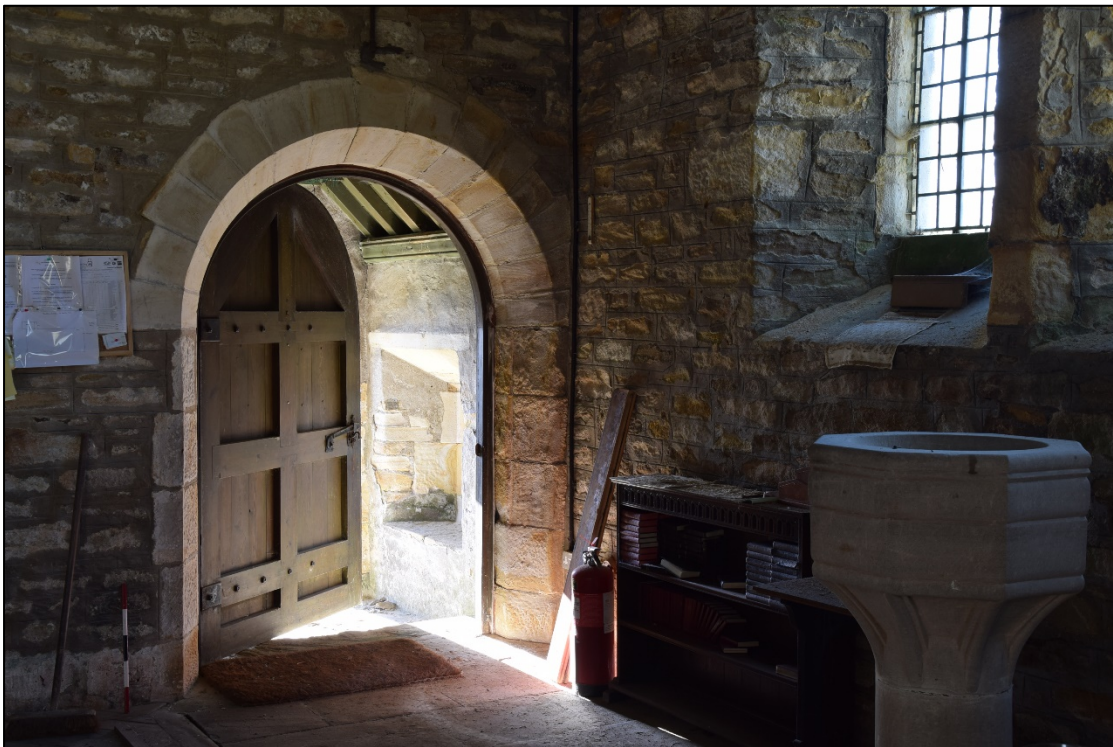
Photograph 22: The simply chamfered entrance and heavy door, seen from the nave. The scale is 0.5m long
