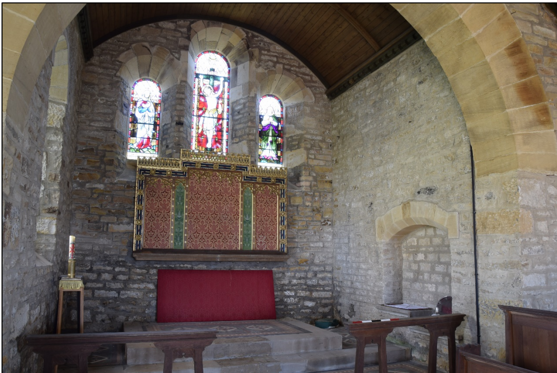
Photograph 30: The chancel. The small sedilia occupies the space where a south window might have been, but for the vestry on the other side of the wall
