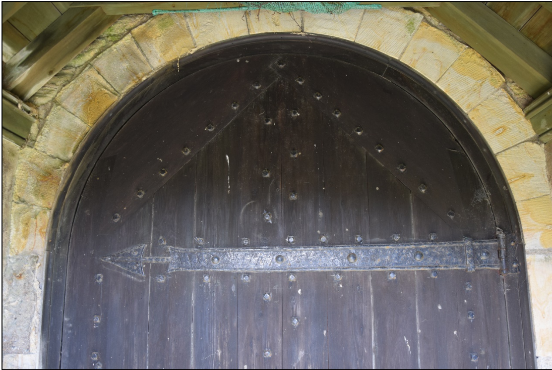
Photograph 21: Detail of the decorative hinge and nailing on the church door
