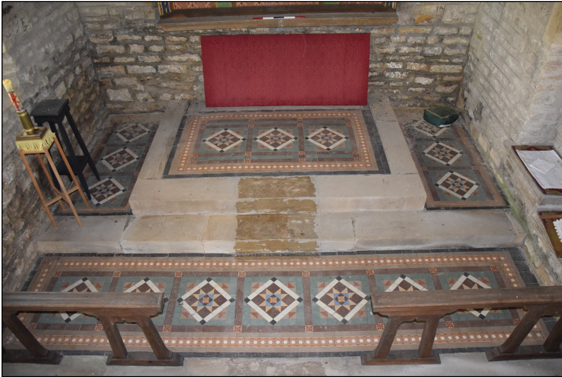
Photograph 33: The tiled floor and the steps in the chancel
