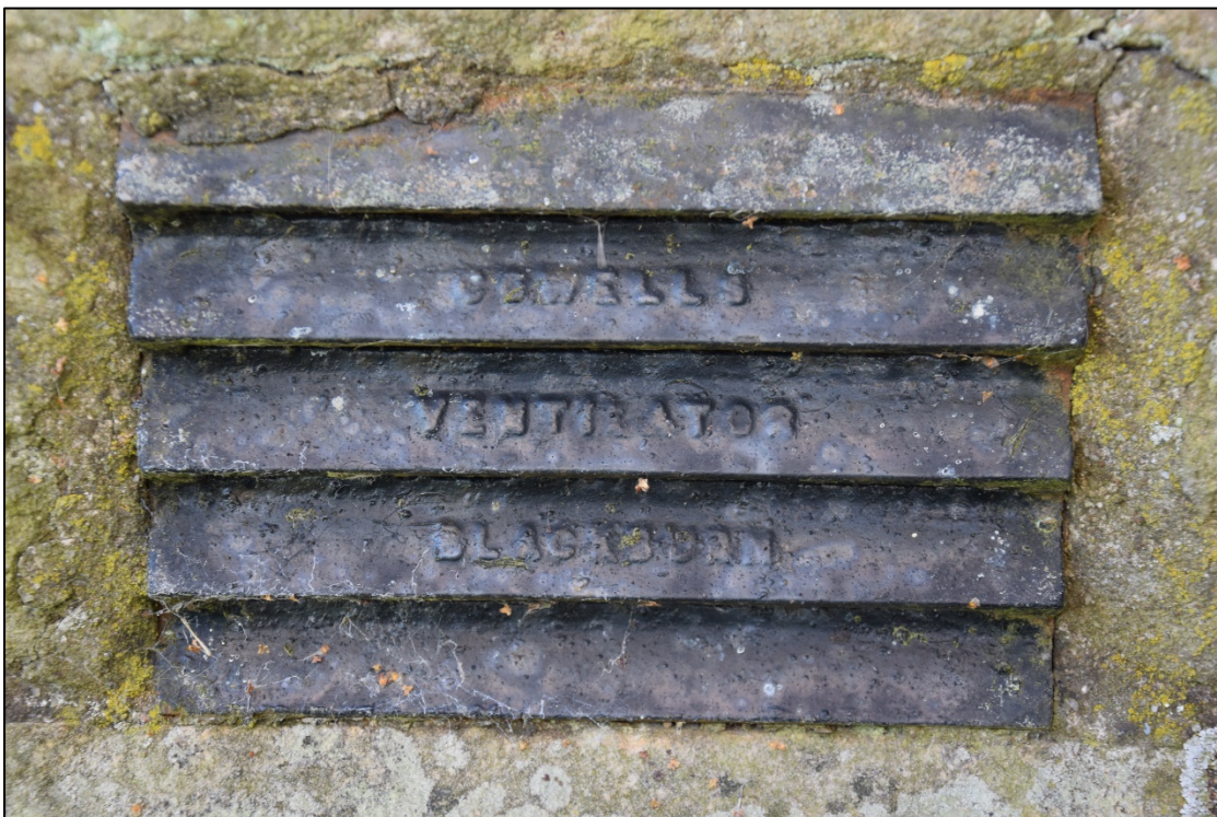
Photograph 12: One of the iron ventilators fitted below the windows
