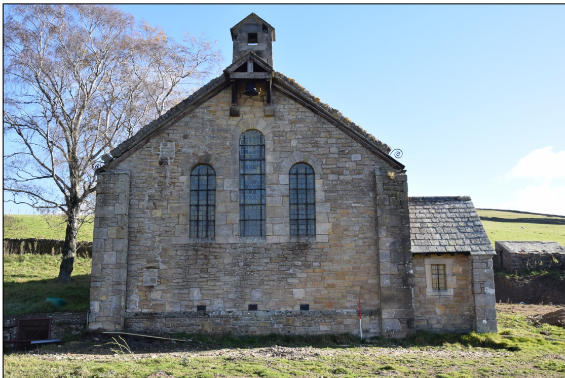
Photograph 16: The west end of the church, with signs of some recent excavation work in the grass
