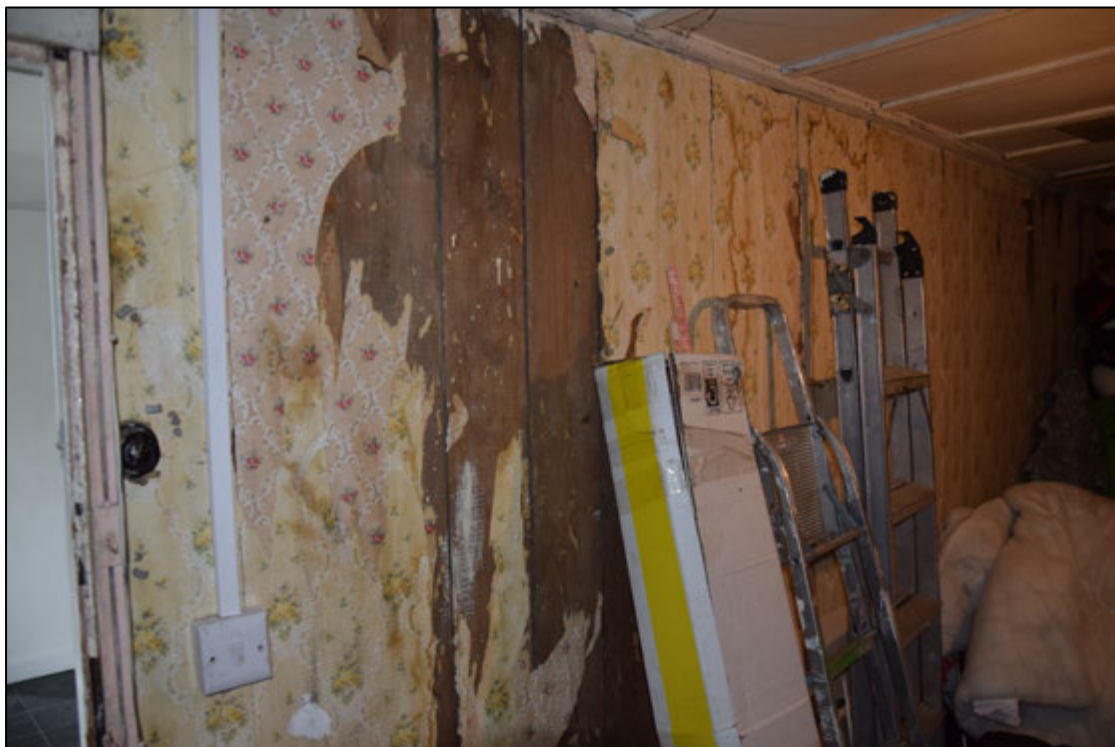
Photograph 28: The wooden wall of the bathroom store 11, with 20th-century wallpaper applied directly to the boards
