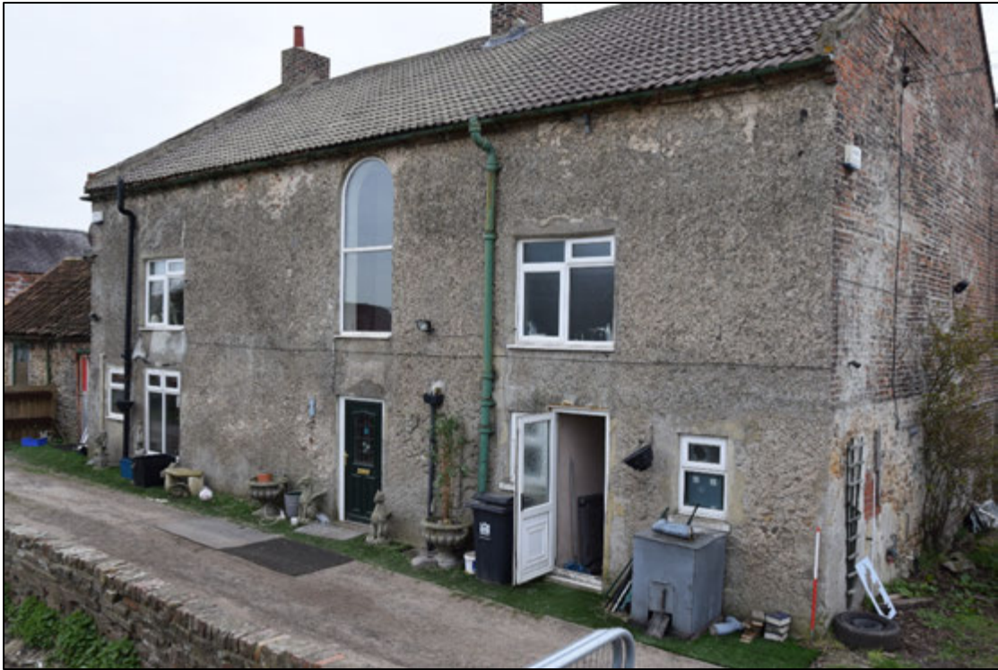
Photograph 7: The north wall of the house, covered with roughcast. Note the low windows on the first floor, reflecting the lower eaves of an earlier form
