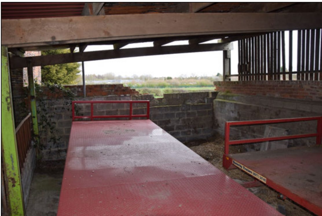
Photograph 88: Concrete block reinforcement conceals the inside of the old east building
