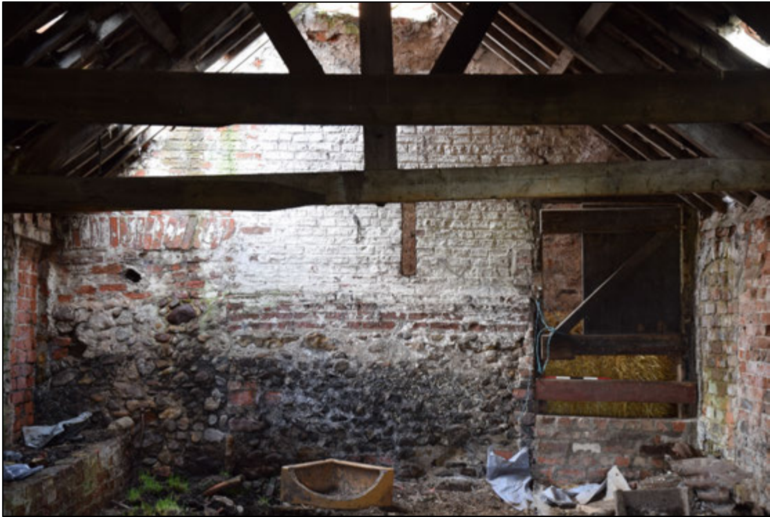
Photograph 73: The west face of the stable seen from the byre. The door at the left is blocked with a mixture of stone and brick, reflecting the old and later masonry of the wall
