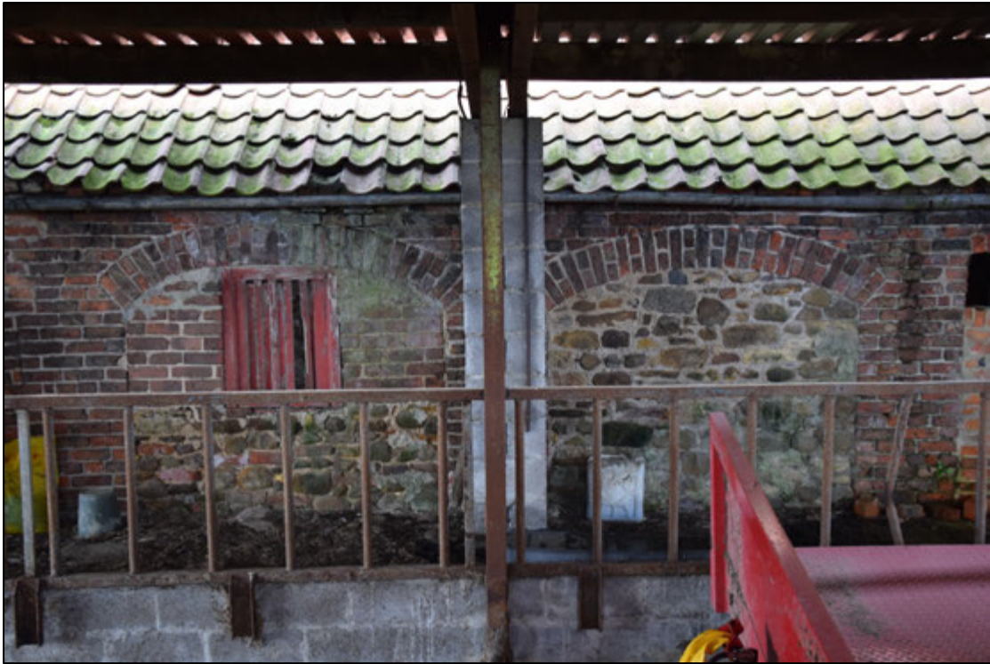
Photograph 81: The same openings seen from the outside
