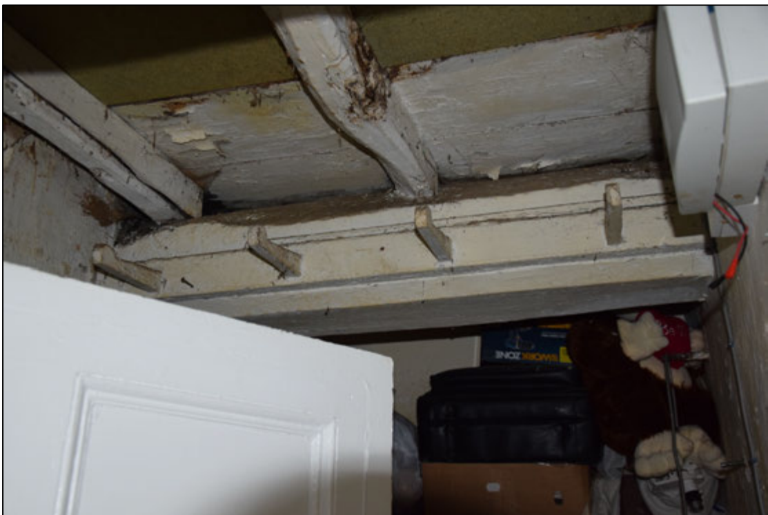
Photograph 18: The beam, joists and wooden hooks in the small store room 4
