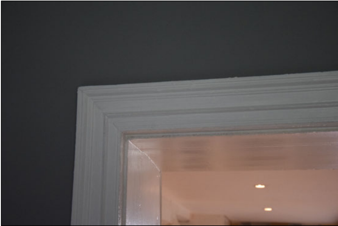
Photograph 15: The architrave on the south side of the same door has a more decorative moulding
