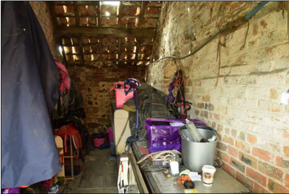
Photograph 53: Looking west into the tack room that occupies the south side of the surviving stable building. At the far end, the lintel of a blocked opening can be seen; this is the door shown in Photo 48
