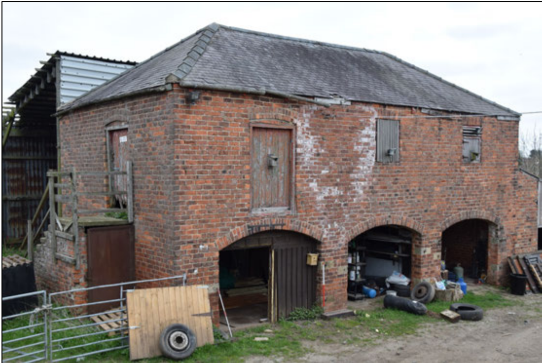
Photograph 93: The cart shed and granary, building I, seen from the north-west
