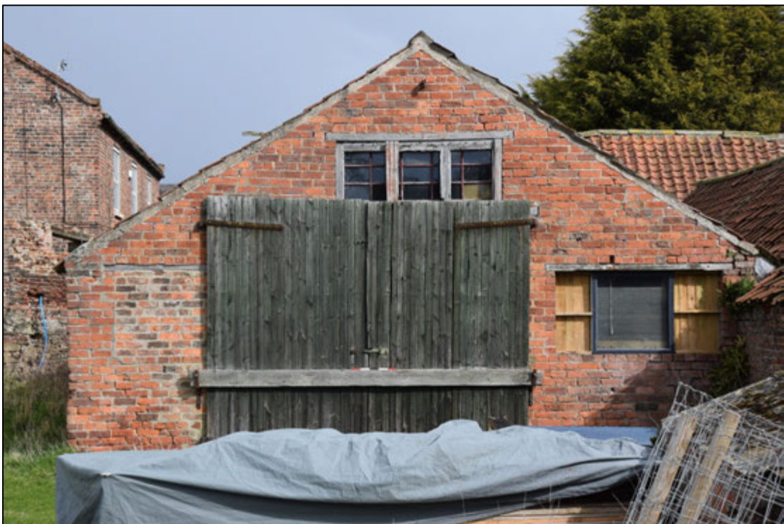
Photograph 90: The west face of the stable, building H
