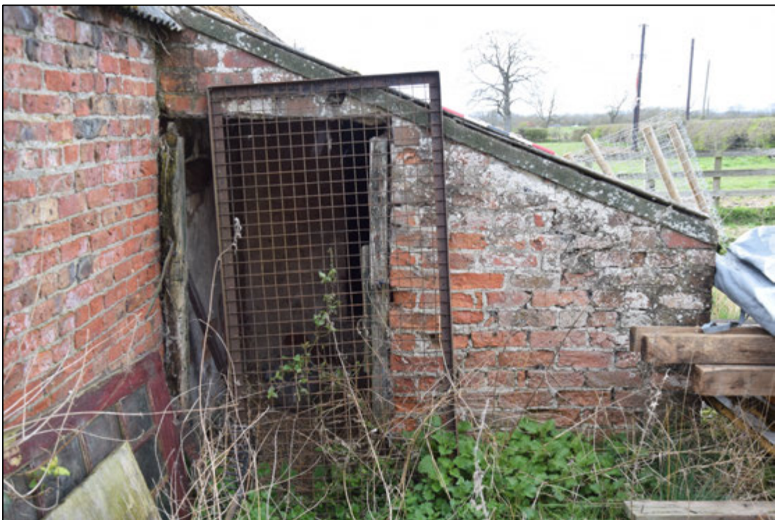
Photograph 84: The east face of shed F
