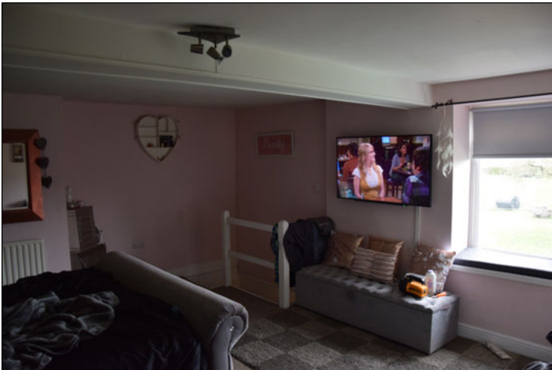
Photograph 26: Room 9 seen from the south-east corner. This view shows the top of the stair from the kitchen and the boxed-in ceiling beam
