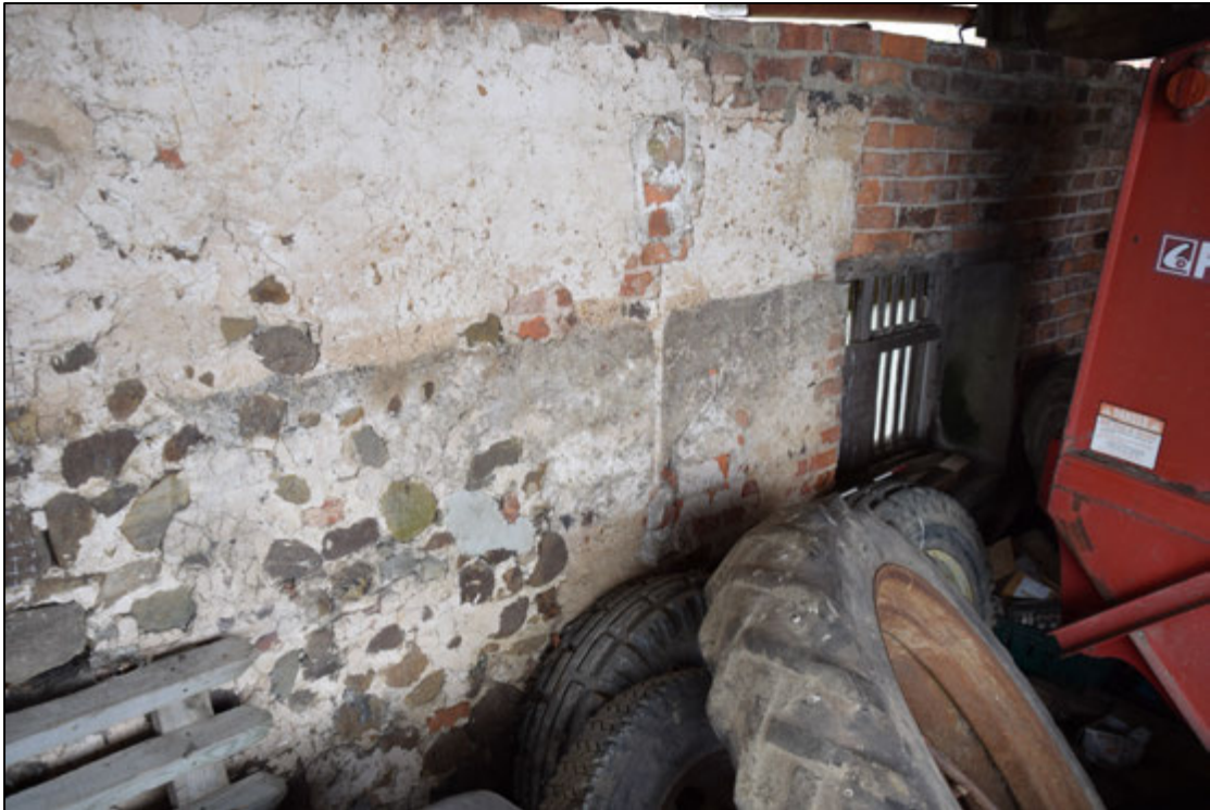
Photograph 57: The inside face of the west wall of the stable, inside the modern shelter. The window is set into a blocked door. There is a blocked triangular-headed niche above the tyres
