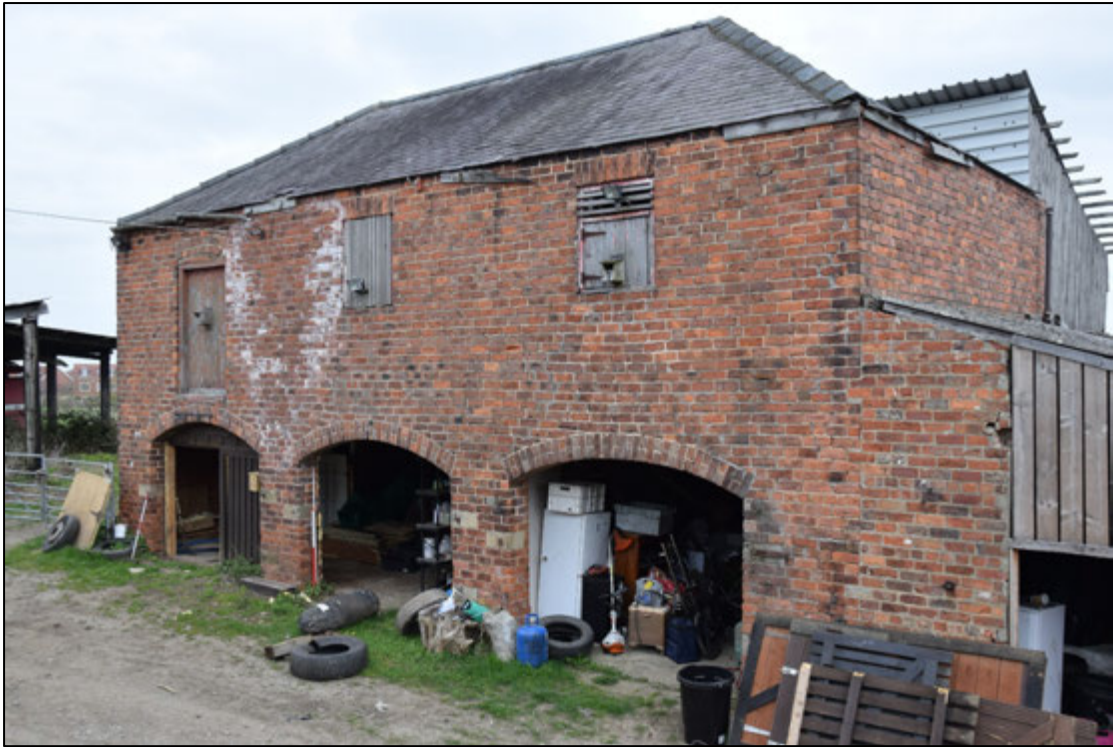
Photograph 95 (above): Building I seen from the south-west. The near arch and the brickwork above it are slightly distorted because of structural movement. The building at the right is a later lean-to shed
