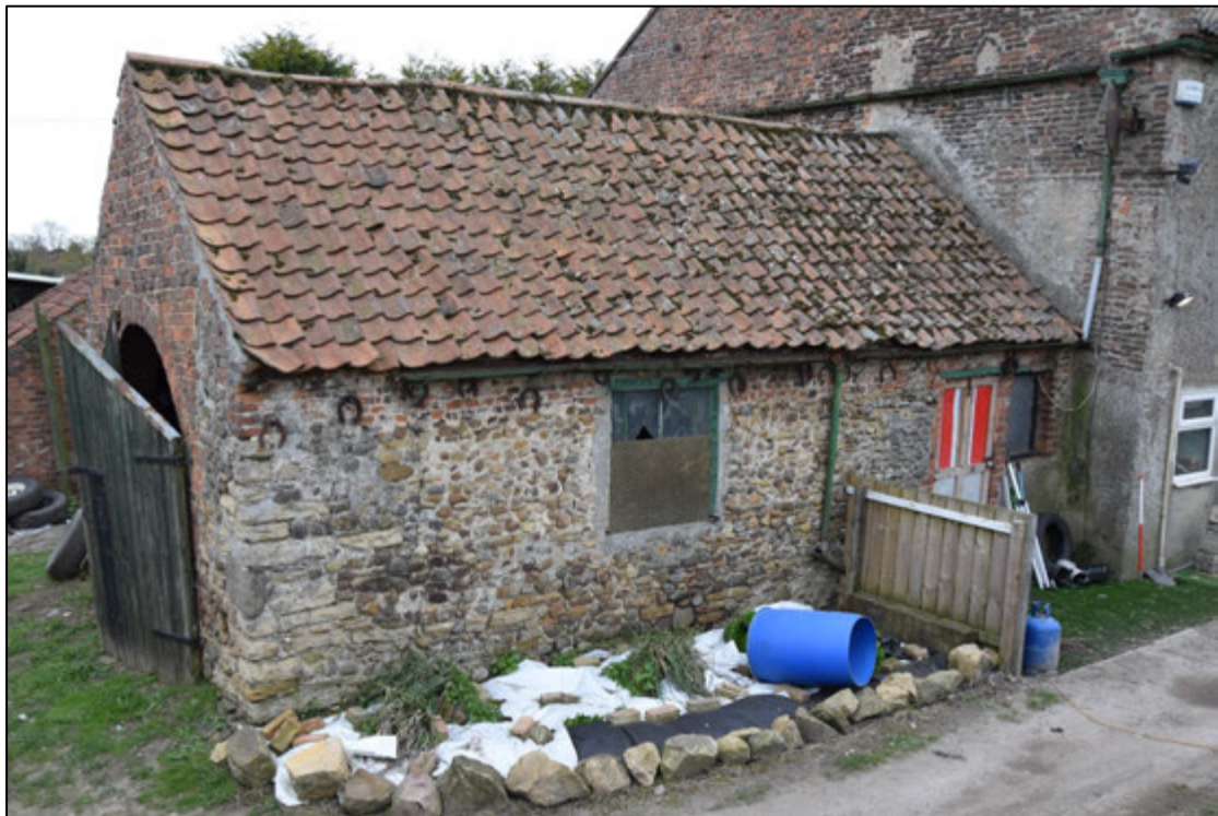
Photograph 36: The workshop, building B. Note the similarity between the stonework here and that in the west end of the house, seen in Photo 8. Brick courses used to raise the eaves can be seen here
