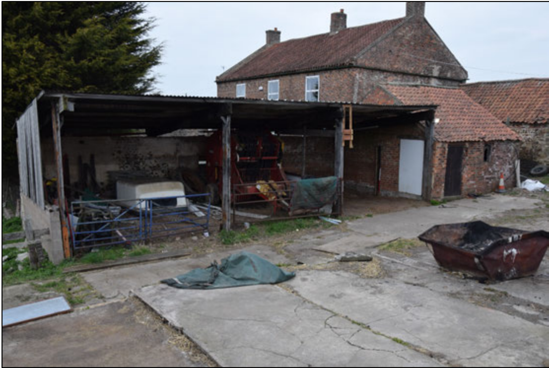
Photograph 43: The east face of the stable, most of which has been replaced by a simple open shelter. The wall with the white door is a modern addition
