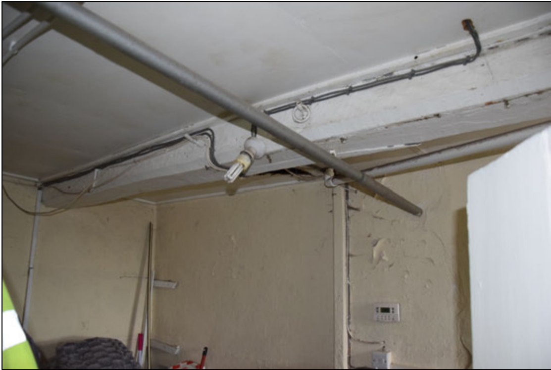
Photograph 17: A heavy ceiling beam with a rough chamfer in the store room 3, west of the old through-passage
