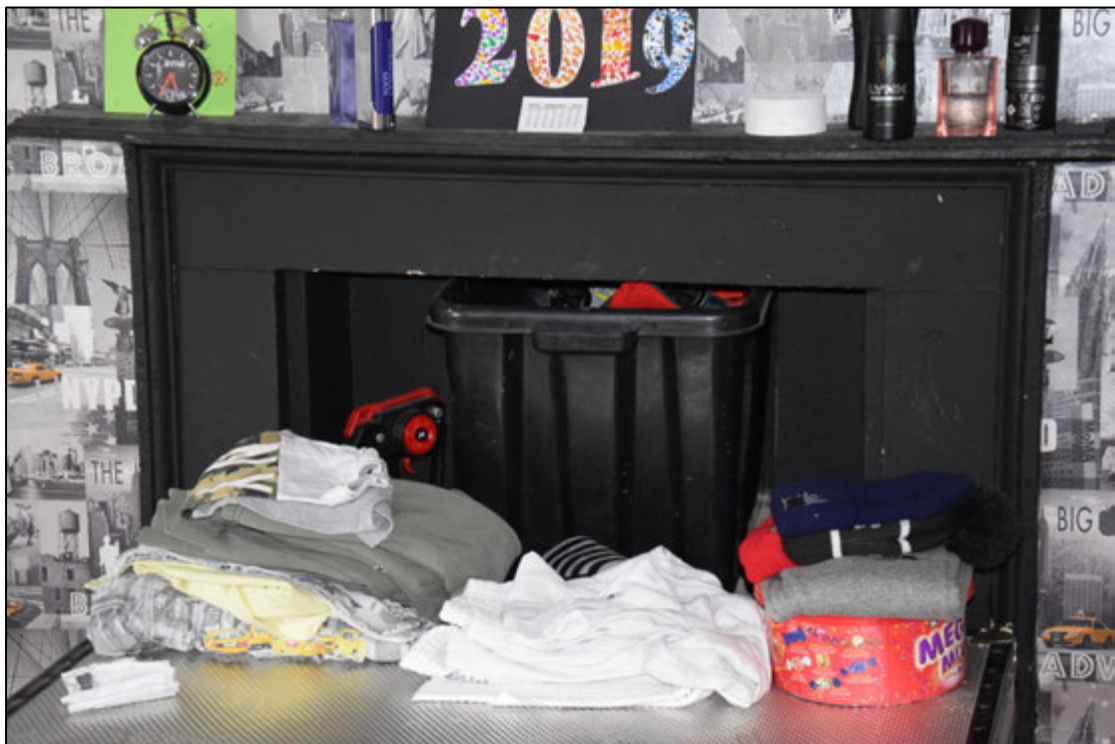
Photograph 34: Detail of the simple stone fireplace in room 14
