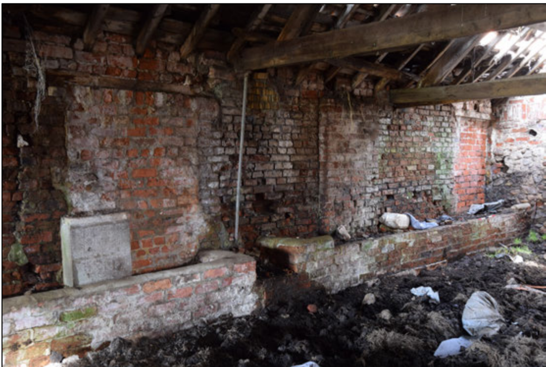
Photograph 76: Blocked doors and a brick trough in the north wall of the byre. The thicker section of wall, right of centre, is probably part of a pier from the vanished gin-gang
