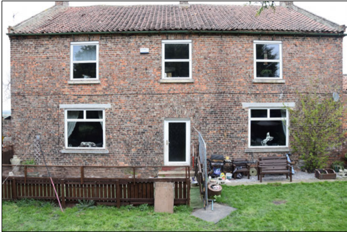
Photograph 5: The south face of the house, with new windows and door. The ground-floor windows have been widened
