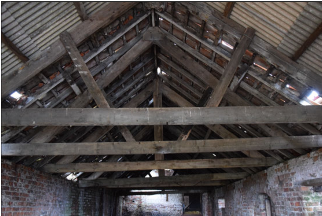
Photograph 82: Old roof trusses contrast with cruder examples in the foreground, at the west end of the byre
