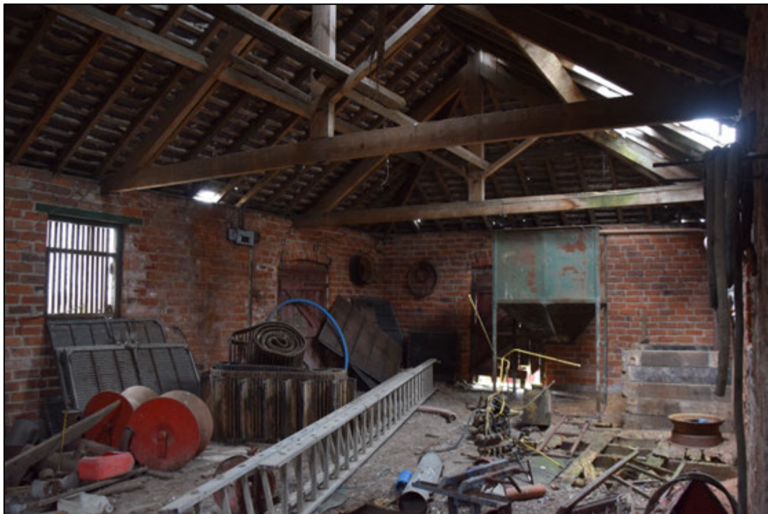
Photograph 100 (below): The interior of the granary, seen from the south-east window
