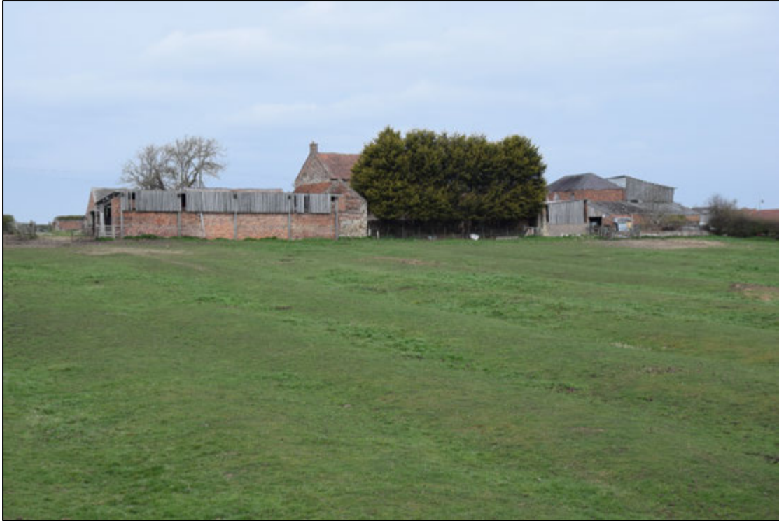
Photograph 1: The Mount Pleasant steading seen from the south-west. The house is screened by conifers at the end of the garden. Note the well-marked ridge and furrow in the field
