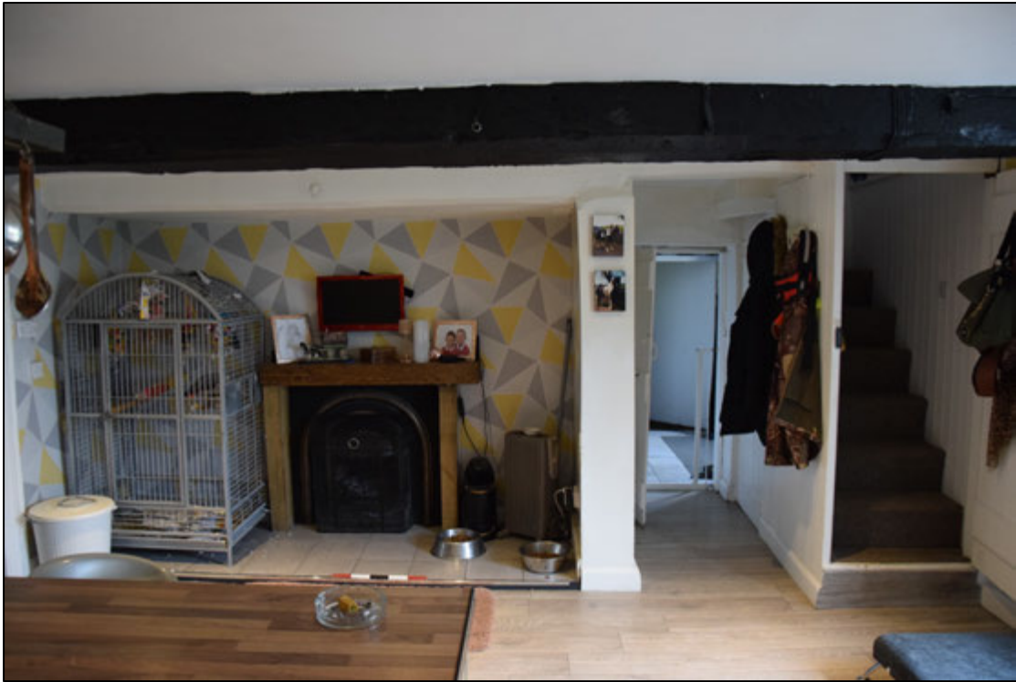
Photograph 11: A view looking west in the kitchen, room 1. The inglenook has a modern fireplace but the heck screen and fire beam are still in place, both covered with plaster. The wall at the left-hand end is a possible site for a fire window. The box stair rises to bedroom 9
