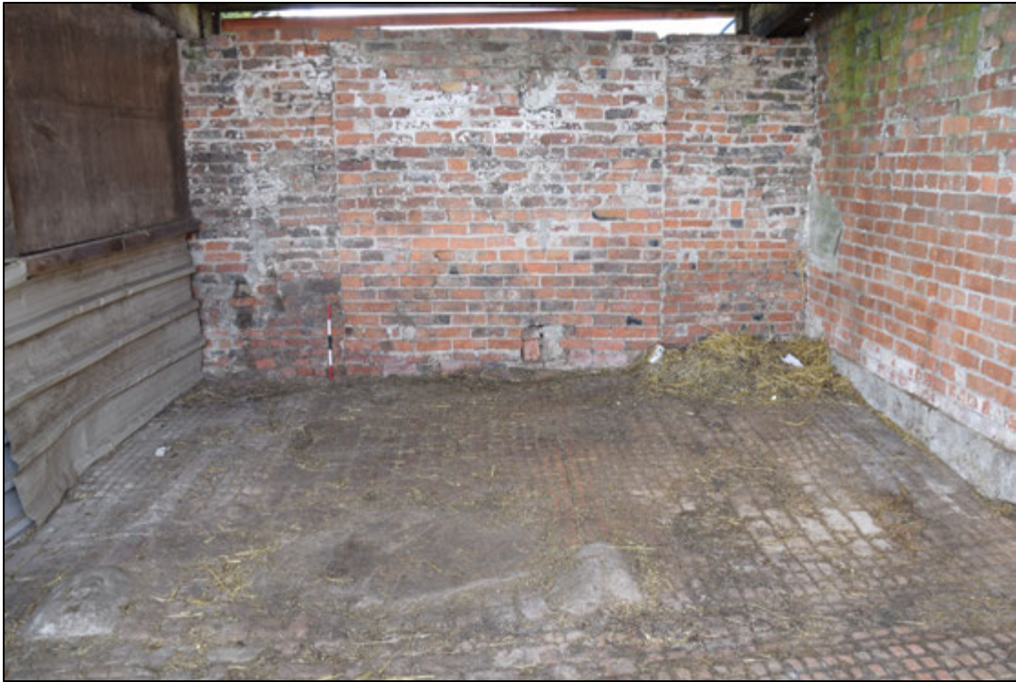
Photograph 55: The marks of stalls can still be seen in the stable floor. The wall at the right is the modern insertion. Note the small blocked rectangular niche near the right-hand end of the far wall. A view looking west
