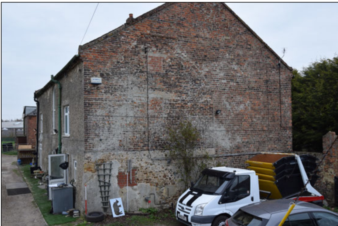
Photograph 8: The west gable. The outline of the older brick house can be seen in the left-hand half of the wall, with rough stone masonry in its lower section
