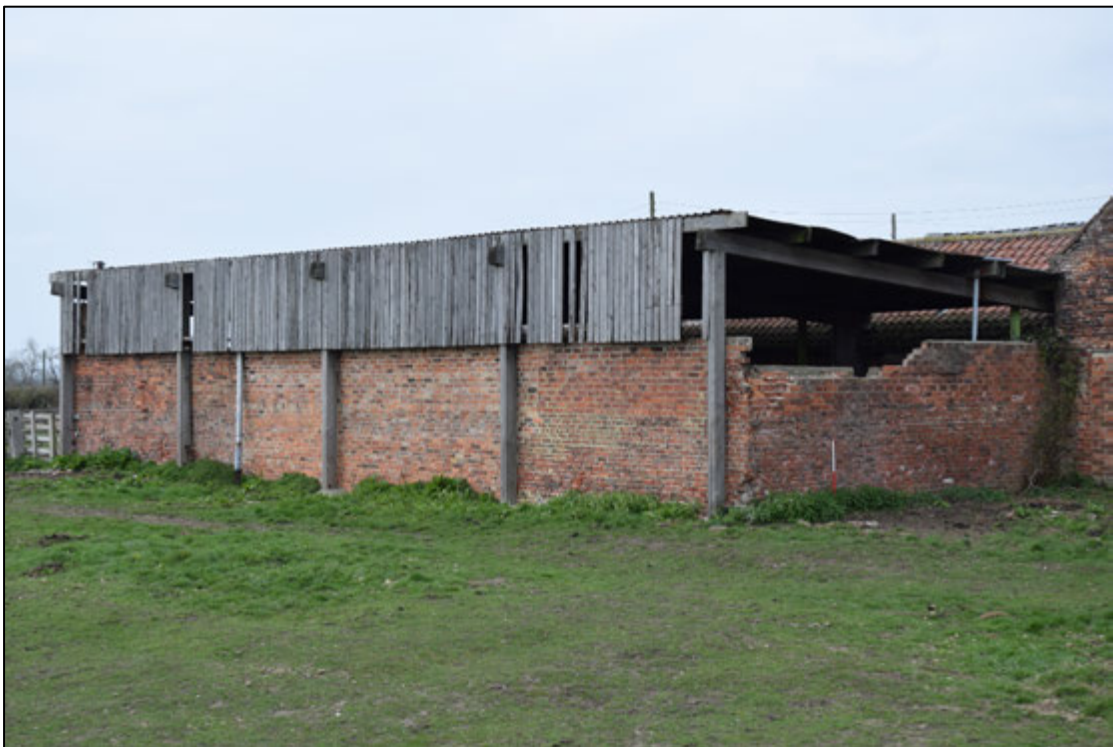
Photograph 86: Building G retains some traces of the two brick buildings that stood here until after the Second World War
