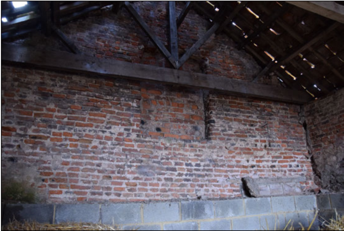
Photograph 65: The pitching door in the south gable. The head of the blocked door seen in Photo 60 is just visible above the later concrete block lining at this end of the building
