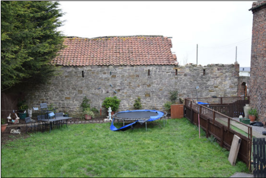
Photograph 59: The east wall of the barn, building D. Note the better quality of the stonework in this wall, which has no parallel elsewhere on the farmstead
