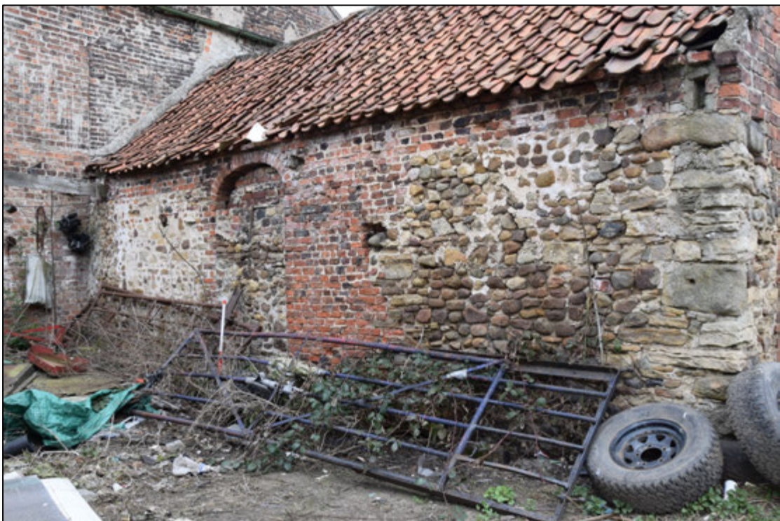
Photograph 38: The south face is a mixture of brick and stone
