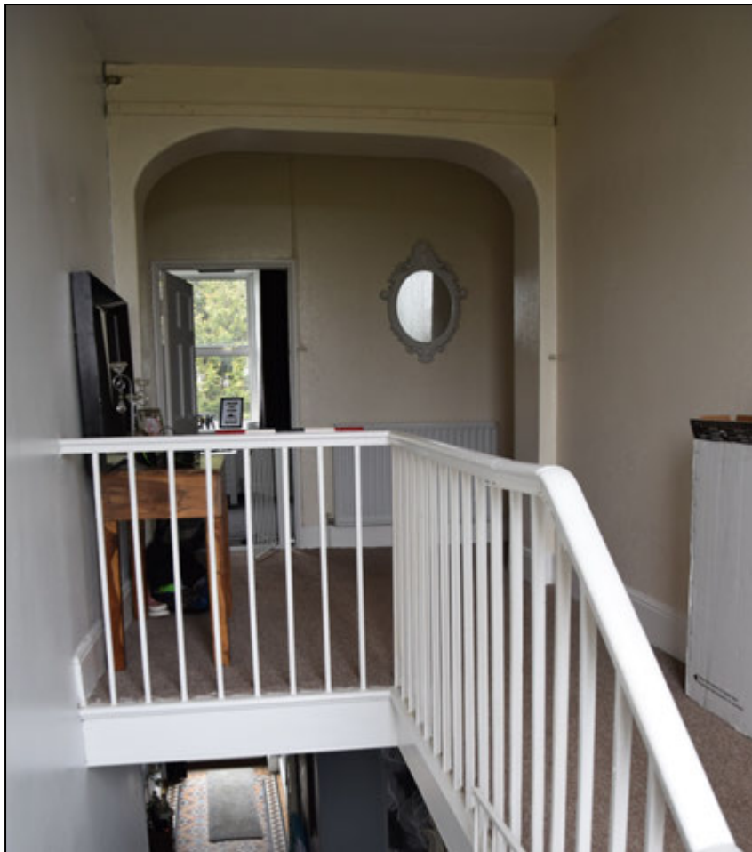
Photograph 31 (left): The plaster arch on the landing 12 marks the line of the old south face of the house.
