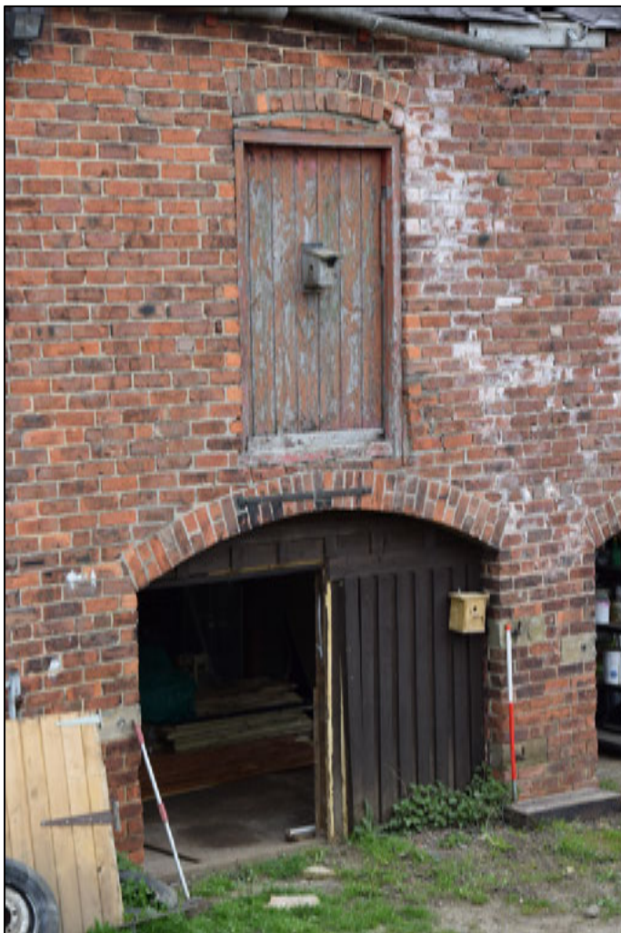
Photograph 95 (above): Building I seen from the south-west. The near arch and the brickwork above it are slightly distorted because of structural movement. The building at the right is a later lean-to shed
