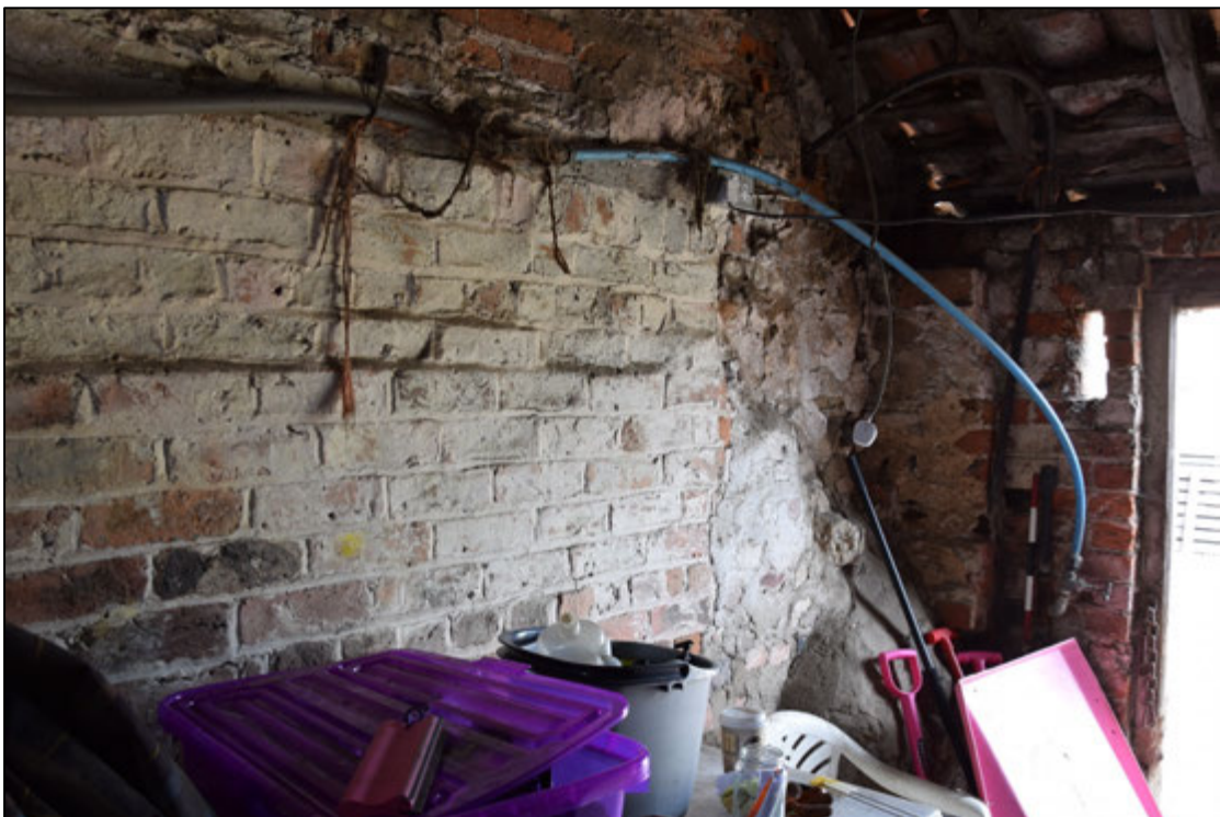
Photograph 54: Mixed brick and stone at the north-east corner of the tack room. The brickwork fills the old door seen in Photo 52
