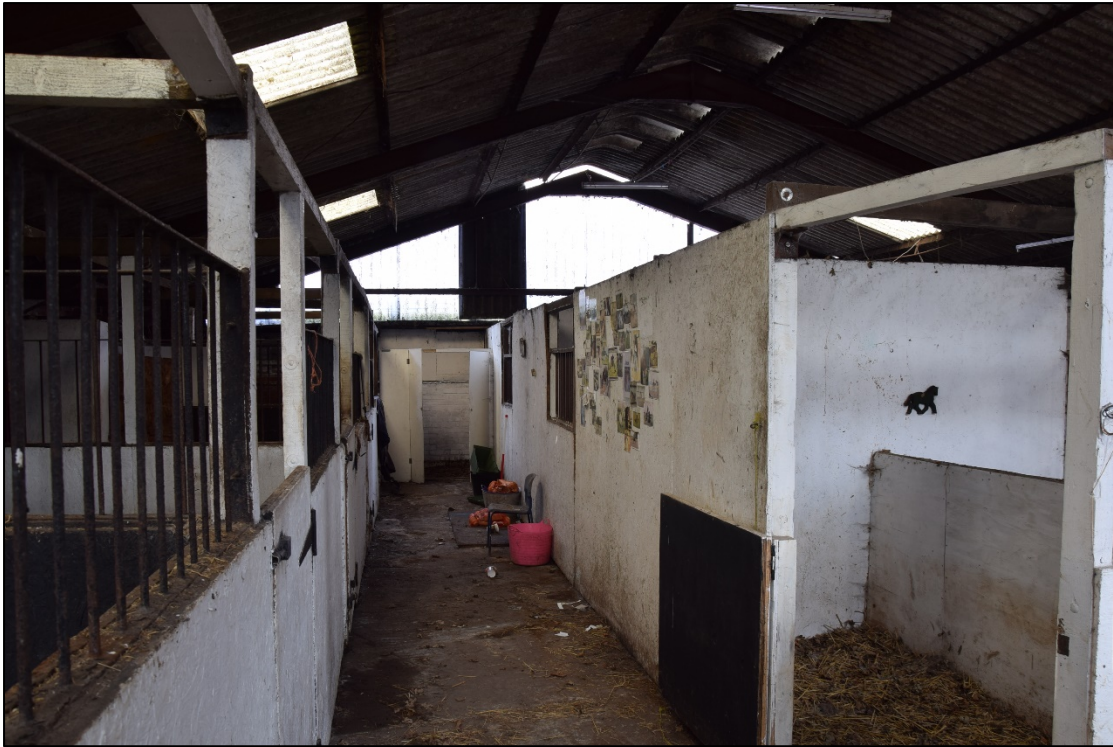
Photograph 63: The interior of the yard [16] is filled with loose boxes and lockers. A view looking north
