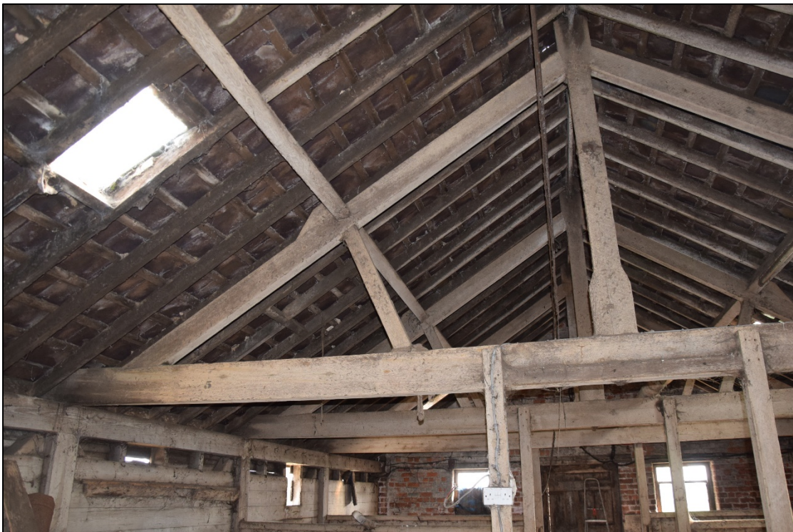
Photograph 36: The roof truss in the granary
