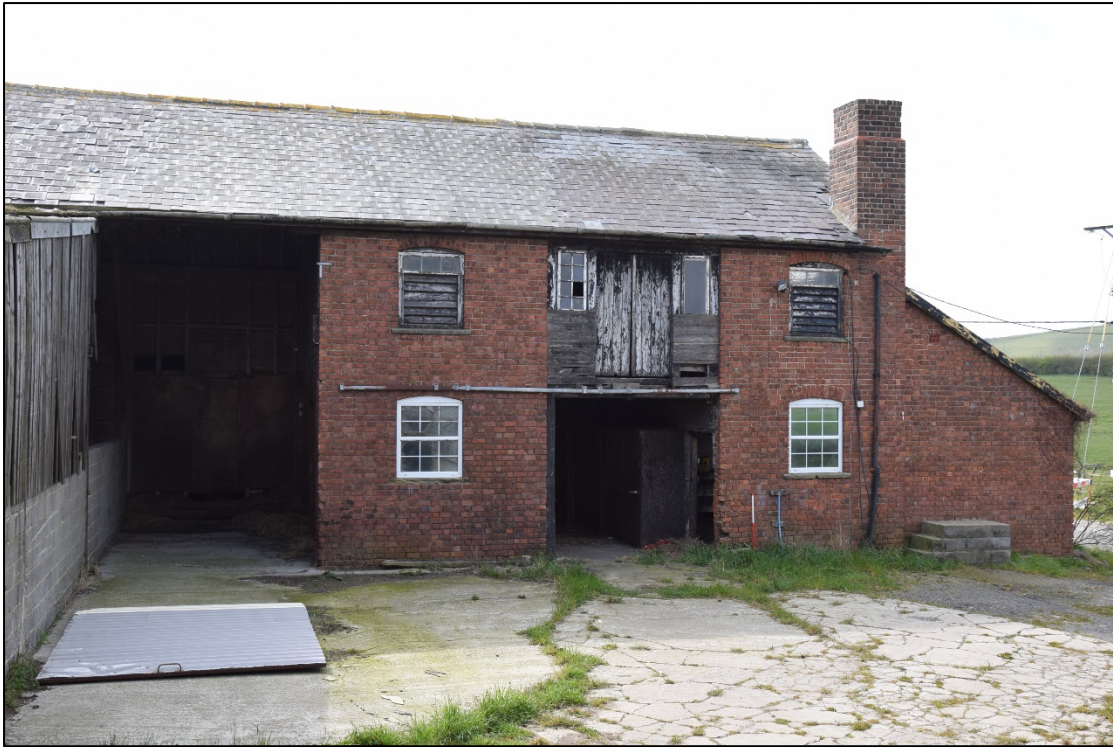
Photograph 9: The north face of the west block. The opening at the left is the end of the hay barn [9]. The chimney has been truncated and capped
