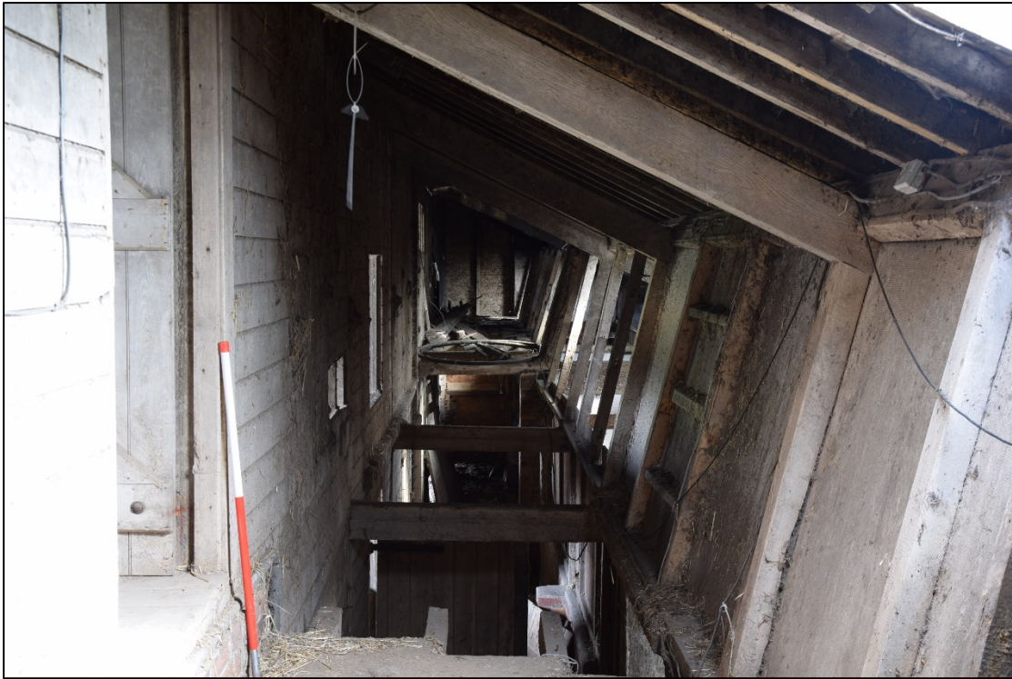
Photograph 27: The upper passage has lost most of its floor. A view looking east from the door to room [6]
