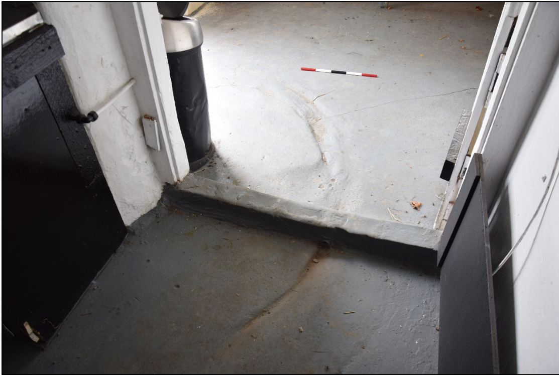
Photograph 13: The crude floor drains between rooms [2] and [3]
