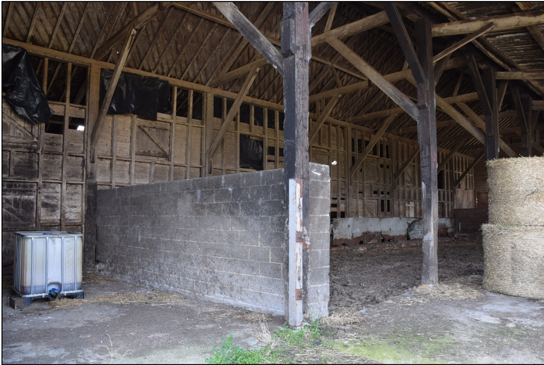
Photograph 37: A view looking south-west into the hay barn [9]. The concrete wall is part of the late pole barn [1]
