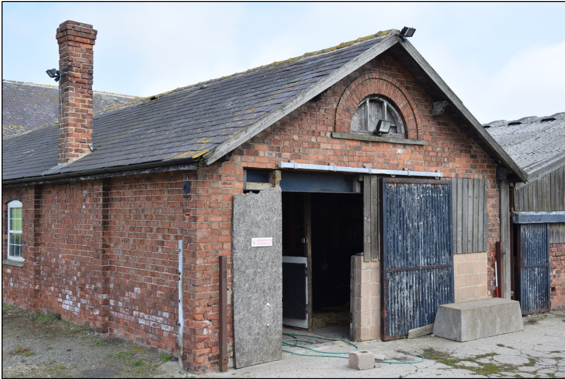
Photograph 51: The west range [13]. As on the other south faces, there are plain barge boards and shaped purlin ends
