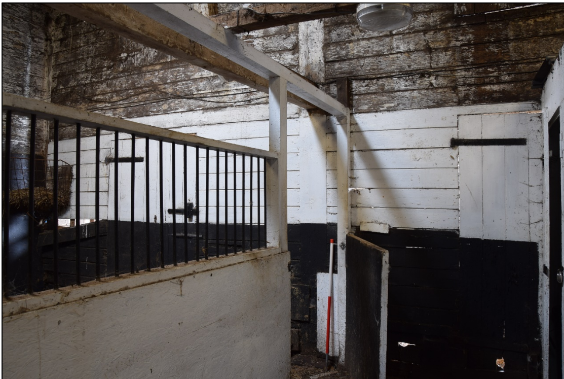
Photograph 66: Two of the feeding doors from the hay barn, seen at the north end of yard [17]
