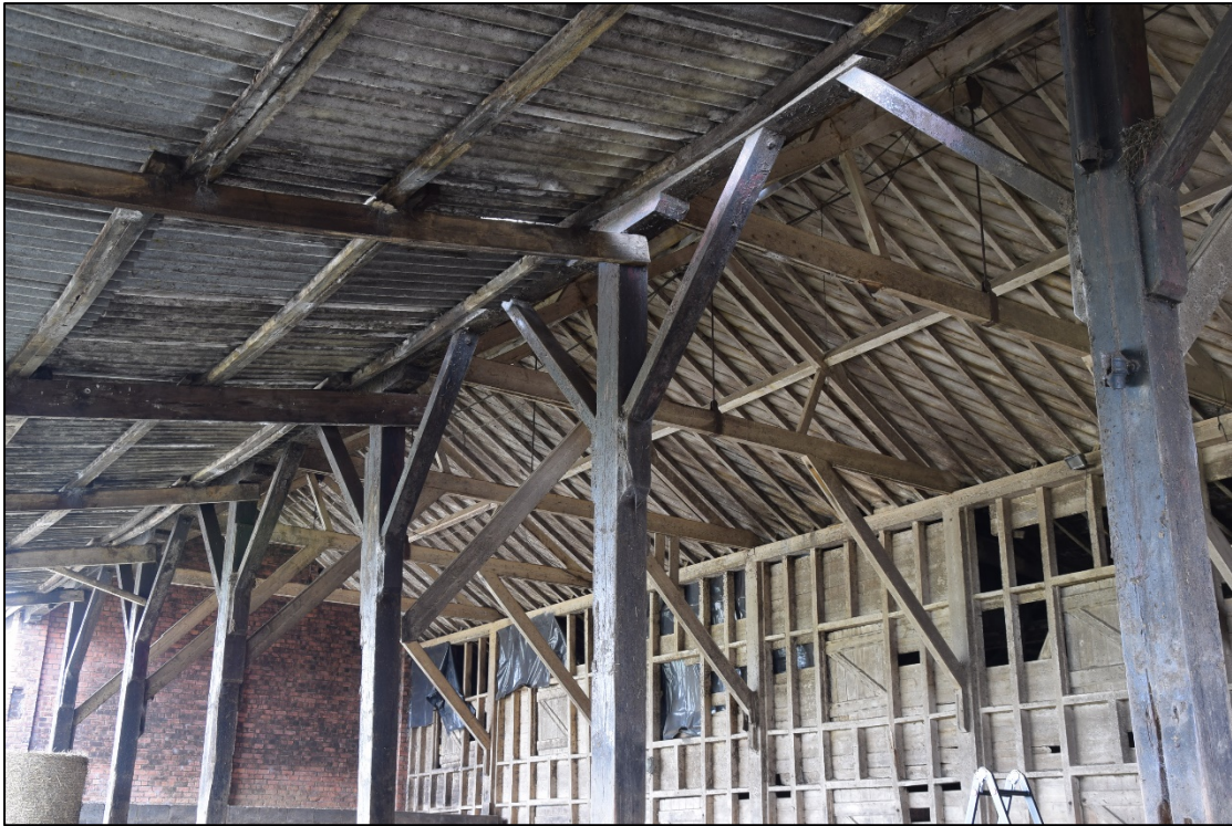
Photograph 39: Posts and braces on the north wall of the hay barn
