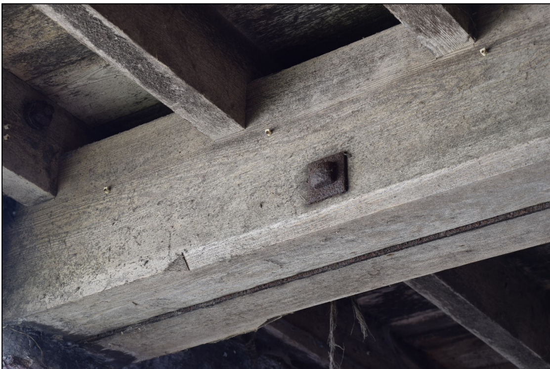
Photograph 16: Detail of the heavy flitched ceiling beam in room [4]
