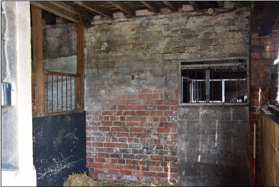
Photograph 53: A blocked door at the south-east corner of the byre [13]
