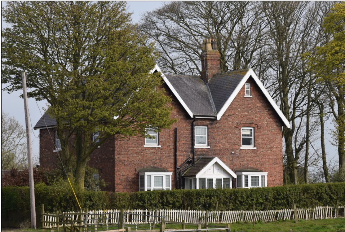
Photograph 3: The farmhouse is contemporary with the main building and shares some of its features, such as shallow arches over the windows
