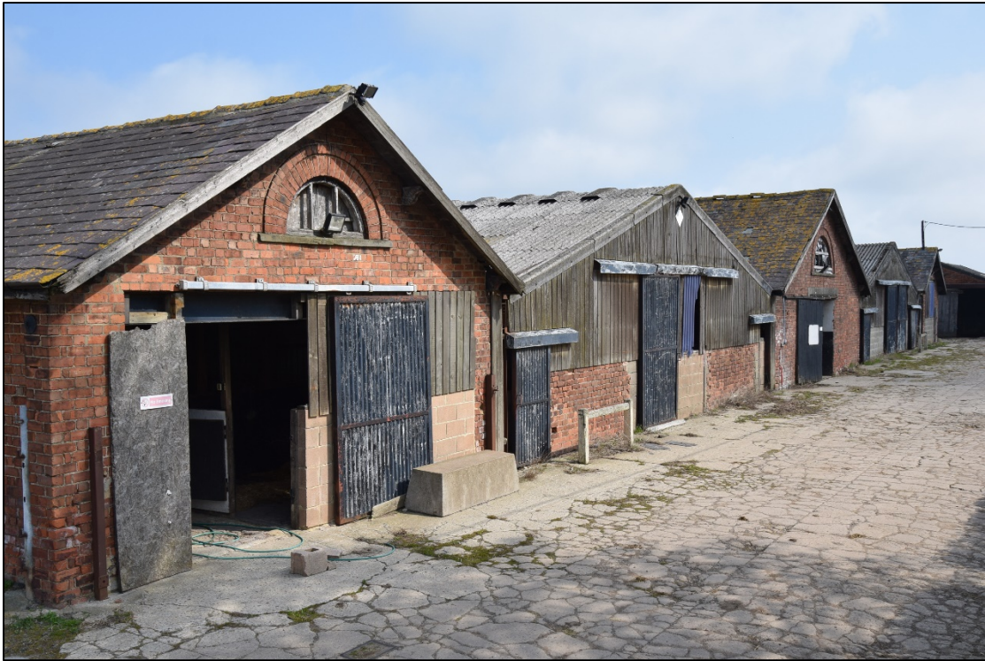
Photograph 7: The south face, with three original brick-built byres separated by later covered yards
