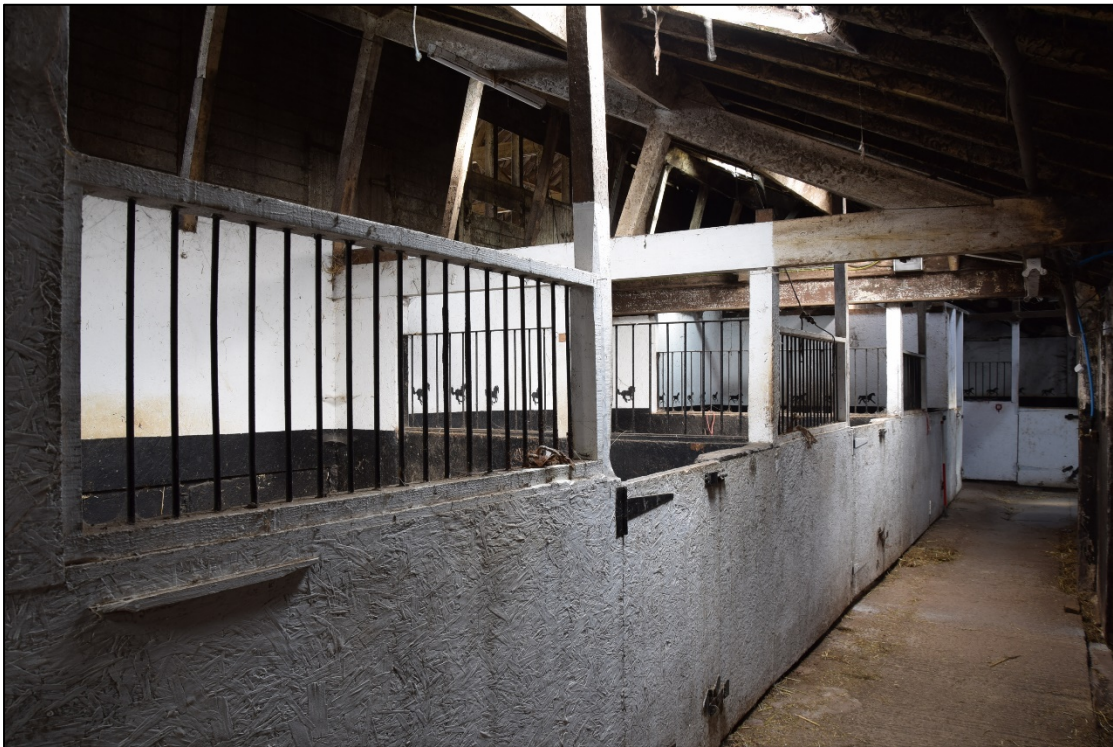
Photograph 48: Loose boxes in the east-west stable [12]; the upper feeding passage can be seen at the top
