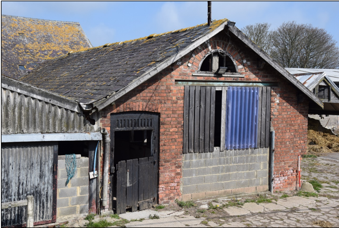
Photograph 59: The east range [15], with the old timber door frame
