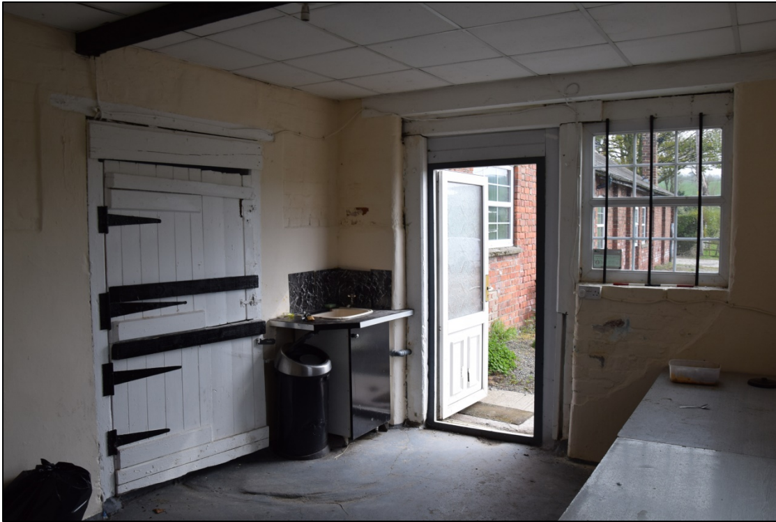
Photograph 11: The canteen [2], showing the door to the kitchen inside the main block
