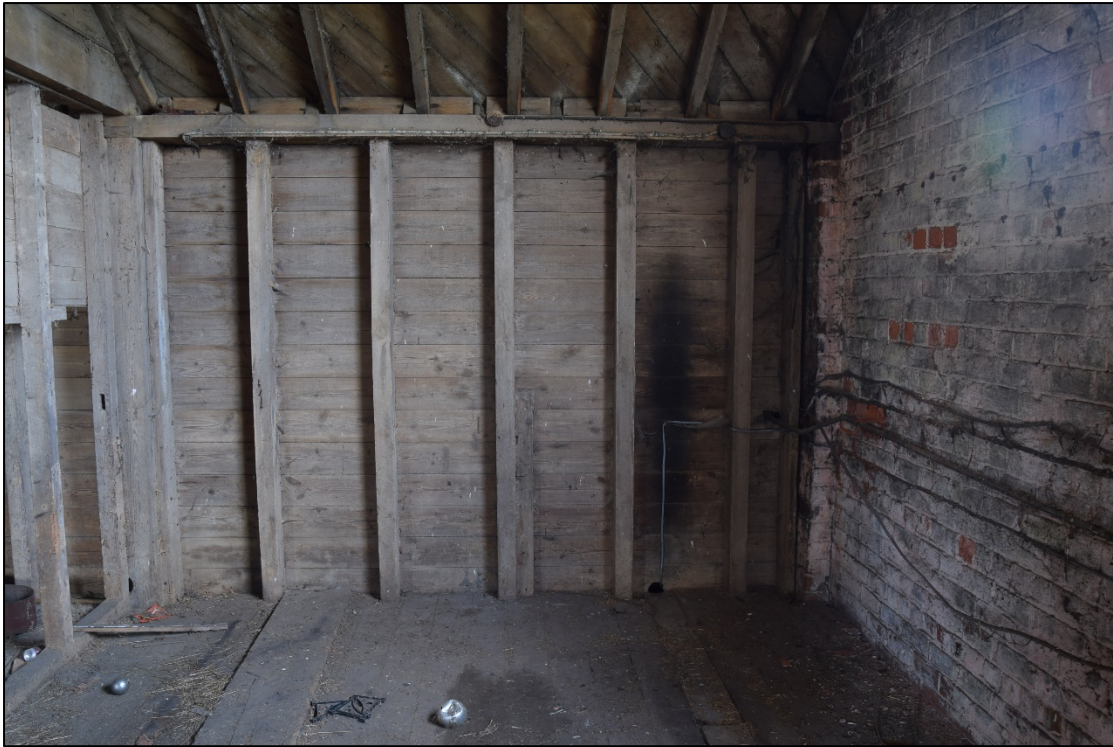
Photograph 23: An oil mark on the south wall of room [6] indicates the position of some vanished piece of machinery. The timber at the left is the side of a former hopper
