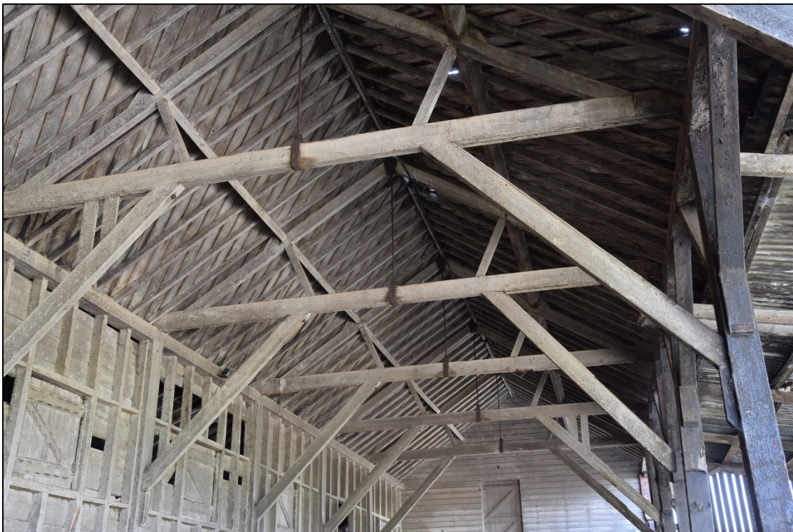
Photograph 40: Detail of the roof trusses in the barn [9]
