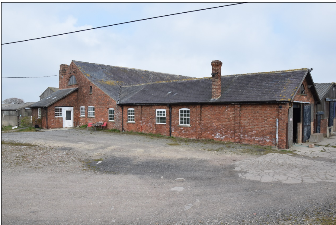
Photograph 8: The west face. Note the altered doors in the single-storey byre, the chimneys and the lean-to that formerly housed an engine
