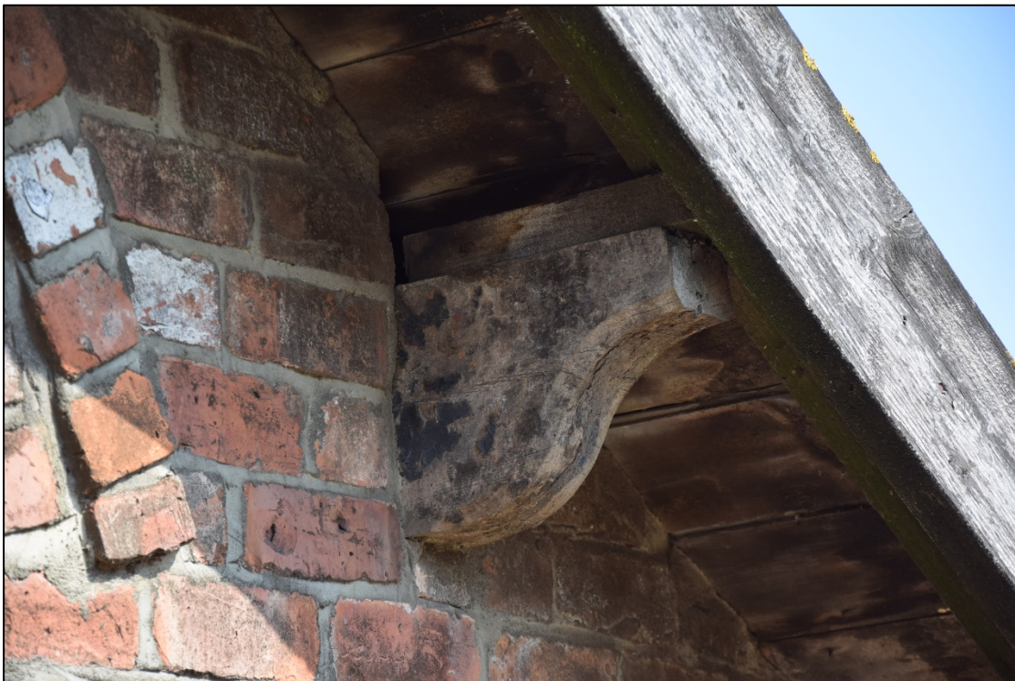
Photograph 60: Detail of one of the shaped purlin ends
