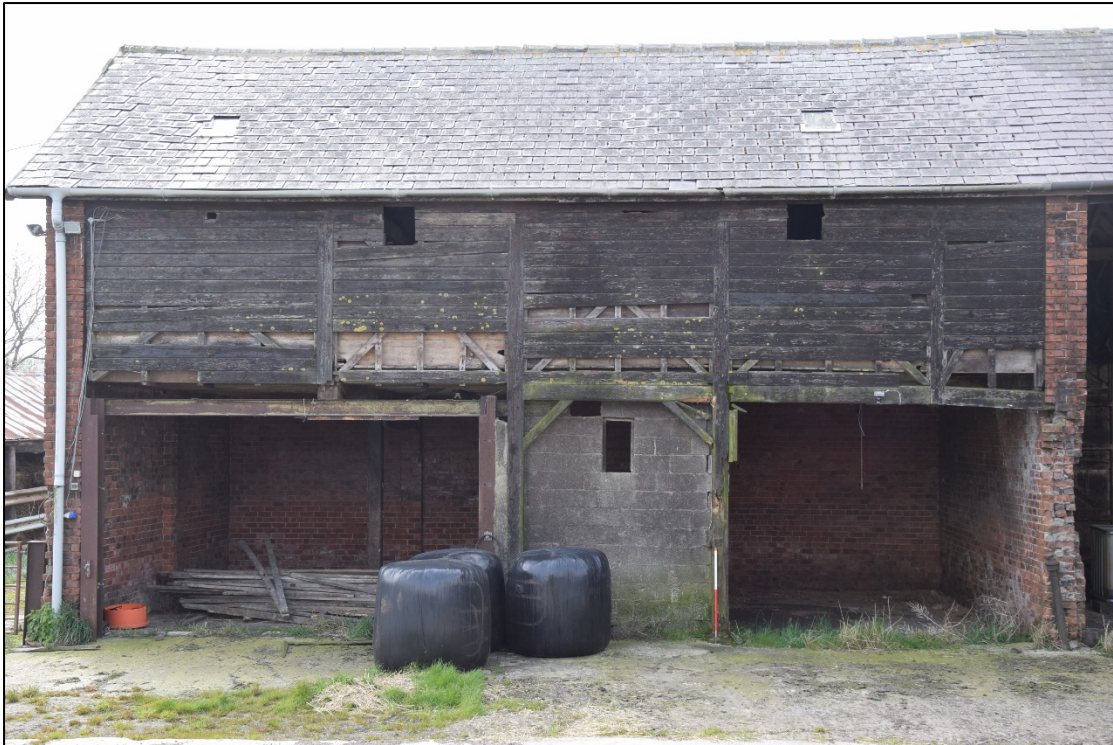
Photograph 29: The north face of the east block, with its timber-fronted granary
