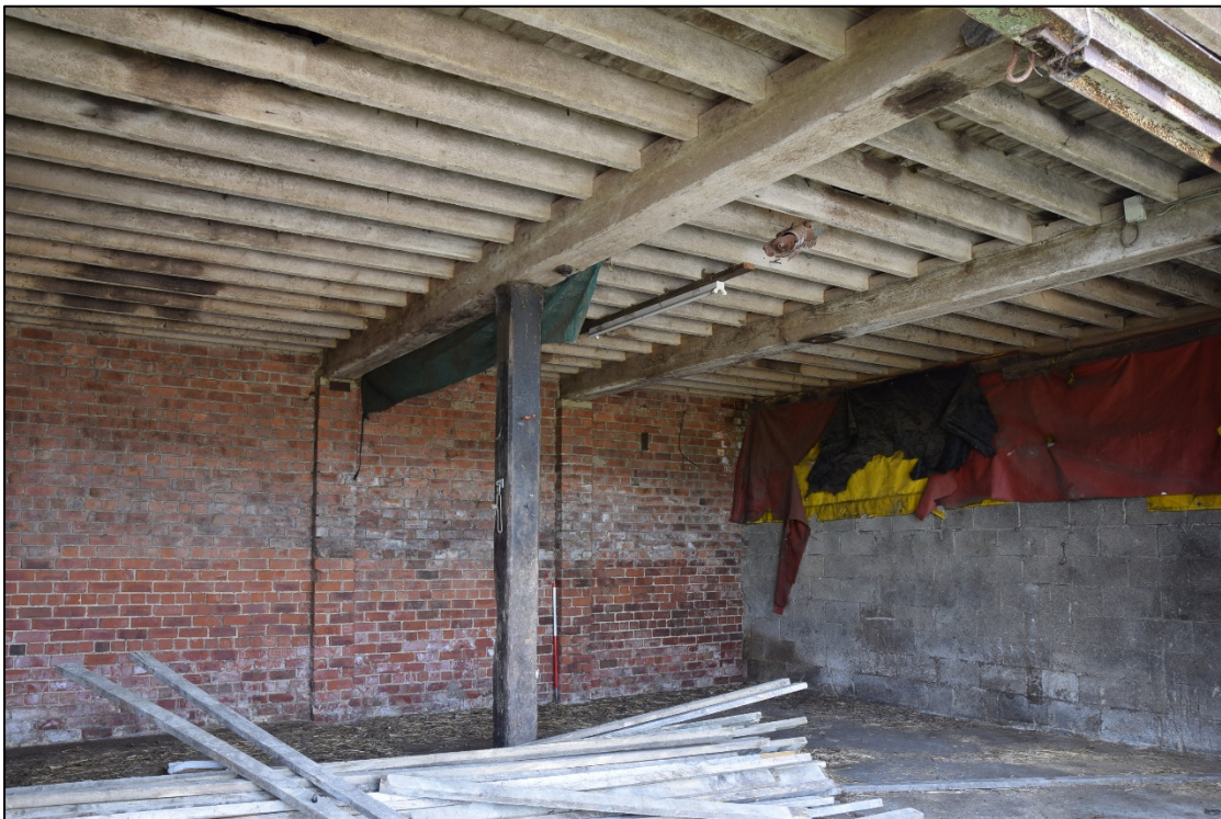
Photograph 30: The open-fronted shed [7] under the granary. Dark marks and mortices on the underside of the ceiling beams show the position of timber posts like the one in the centre of the picture
