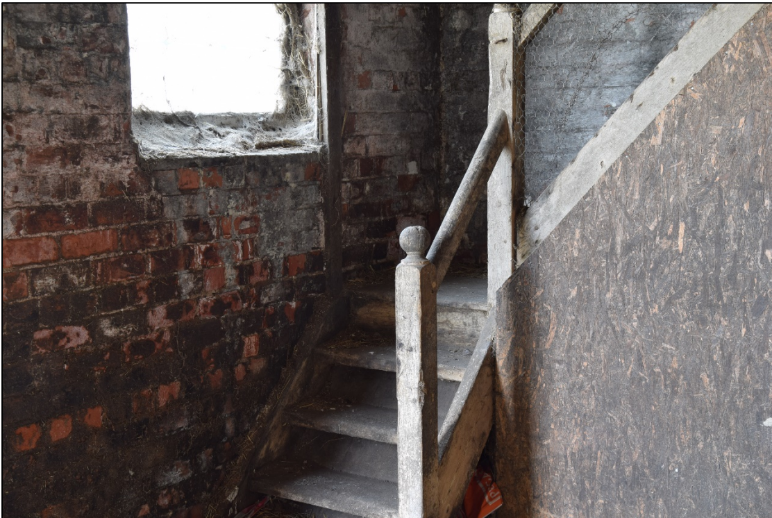
Photograph 20 (below): The staircase at the north-east corner of room [4]
